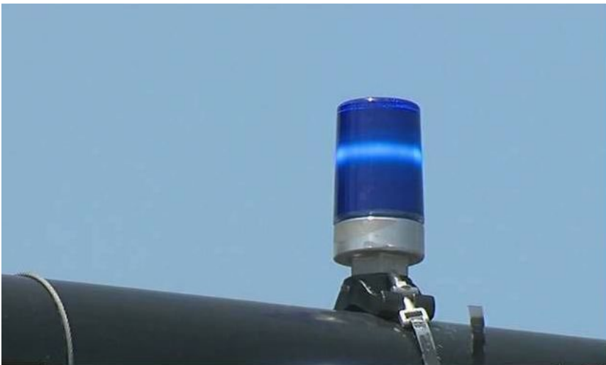
Confirmation Light Retrofit onto a Traffic Signal (Source: City of Bismarck)
