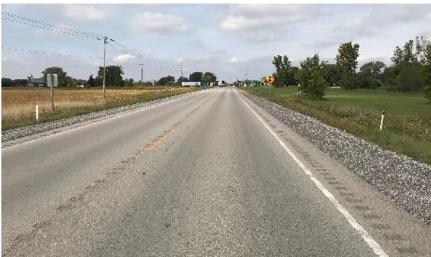
Shoulder Rumble Strip and Centerline Rumble 2
