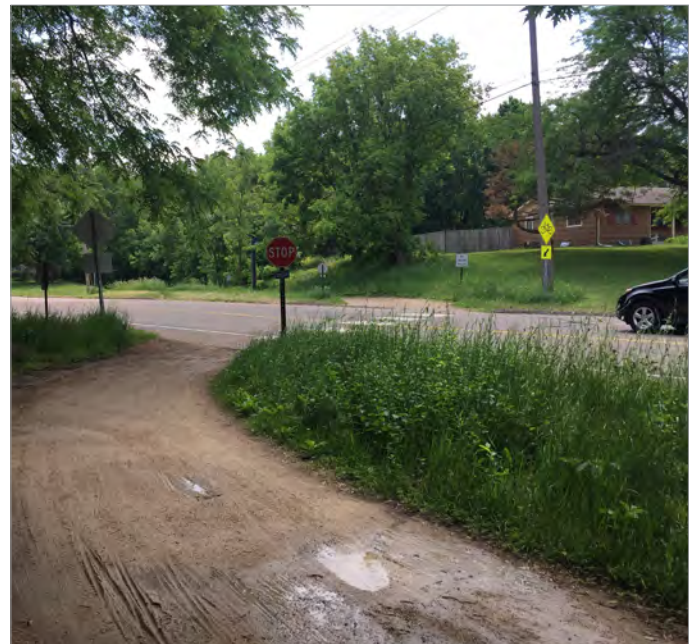
The current Minnetonka Mills Road crossing has poor sight lines and alignment. Photo credit: SRF Consulting Group
