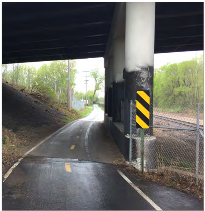
The tight railroad right-of-way creates clear zone compliance issues, as seen here under the Louisiana Avenue bridge overpass. Photo credit: Park District & SRF Consulting Group
