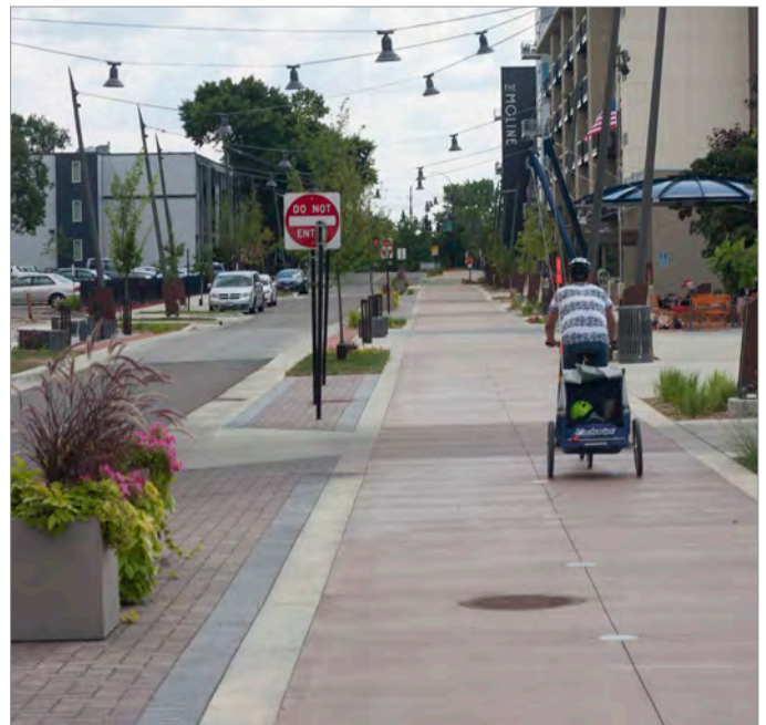
The regional trail is incorporated into the Hopkins Artery streetscape as a cycle track. Photo credit: SRF Consulting Group
