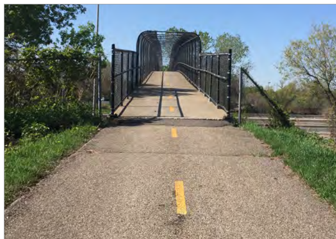
Shingle Creek Regional Trail passes over I-94/694 in Brooklyn Center. Photo credit: SRF Consulting Group
