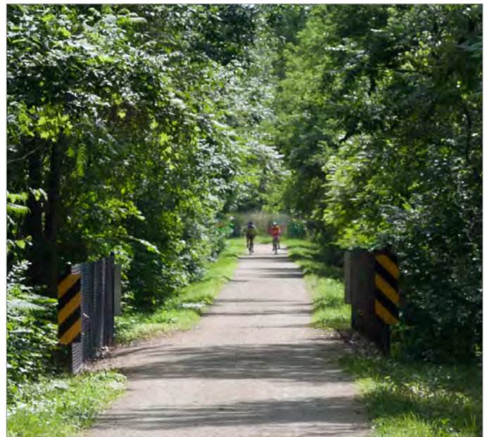
The regional trail passes over Riley Creek with a small bridge, which creates an ideal setting for a rest stop.
