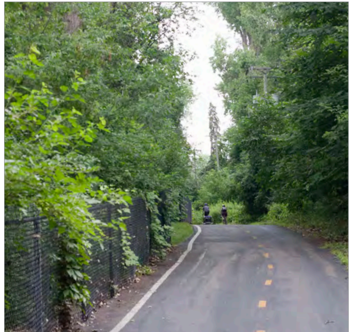
Luce Line Regional Trail route near Schaper Park. Photo credit: SRF Consulting Group
