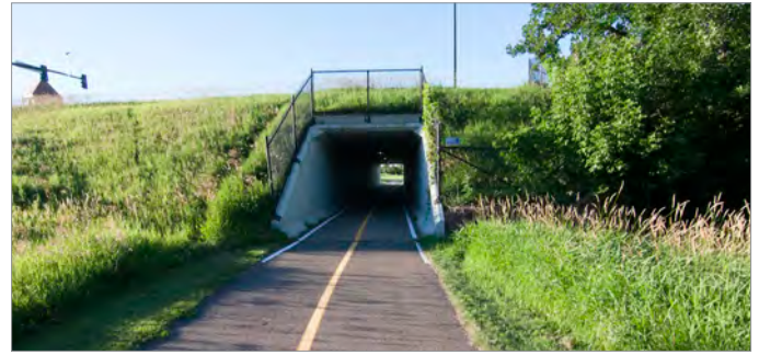
A grade-separated underpass allows regional trail users safe travel underneath CR 30. Photo credit: SRF Consulting Group
