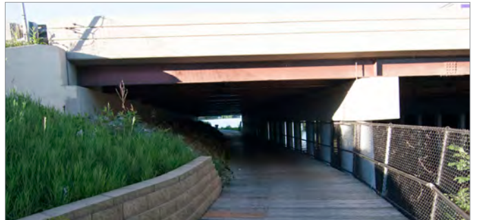
The regional trail travels underneath multiple lanes of I-94 traffic in Maple Grove. Photo credit: SRF Consulting Group
