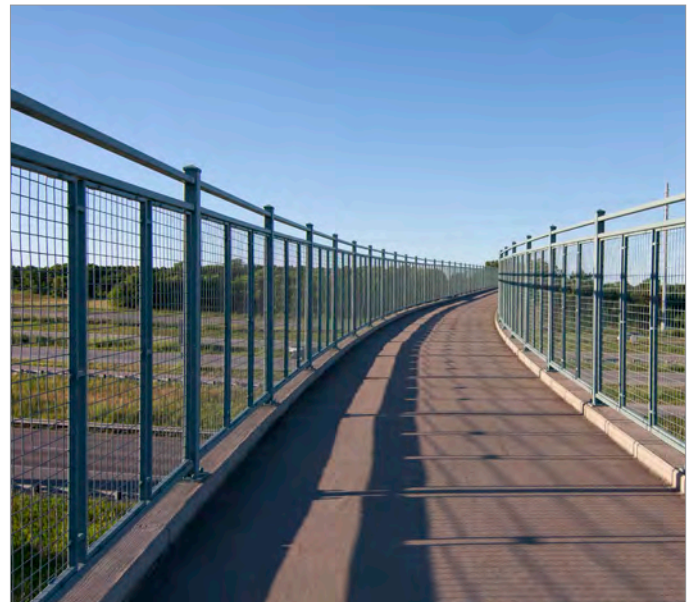
The grade-separated Medicine Lake Regional Trail bridge crosses multiple lanes of Highways 610 and 81 through Maple Grove. Photo credit: SRF Consulting Group
