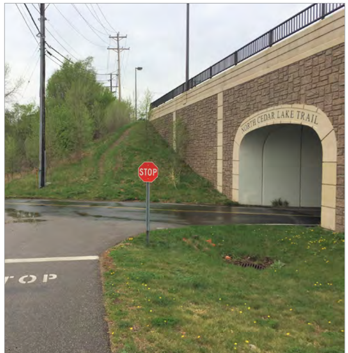
Local trail spur has poor sight lines when connecting to the North Cedar Lake Regional Trail so close to the Minnetonka Blvd underpass tunnel . Photo credit: SRF Consulting Group
