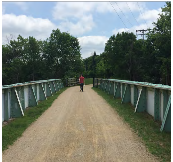
The regional trail is grade-separated by a bridge crossing over Highway 7. Photo credit: SRF Consulting Group
