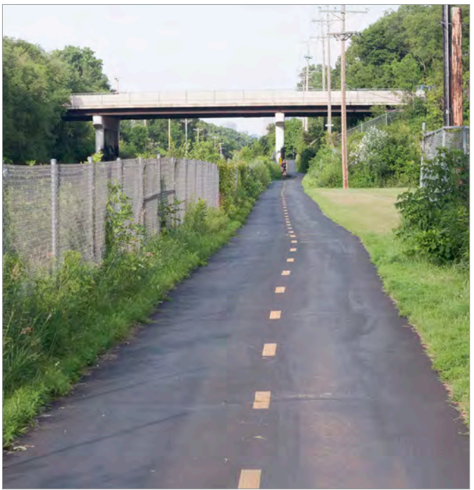
The tight railroad right-of-way creates clear zone compliance issues, as seen here under the Louisiana Avenue bridge overpass. Photo credit: Park District & SRF Consulting Group
