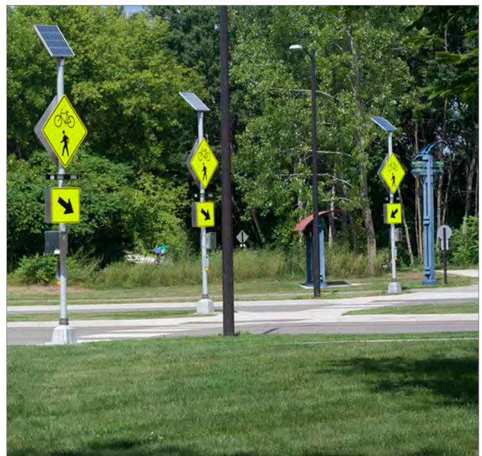
Recent crossing improvements have improved safety at the Dell Road intersection. Photo credit: SRF Consulting Group
