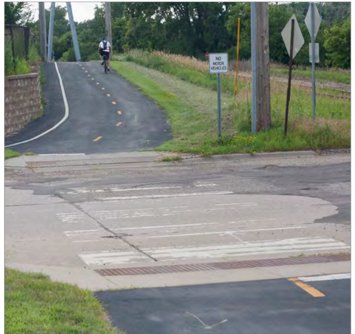
Intersection improvements needed at the crossing of Zane Avenue N. Photo credit: SRF Consulting Group
