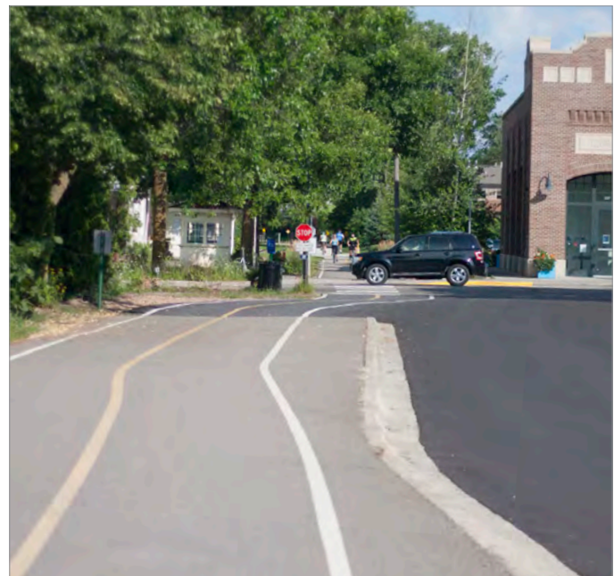
A small segment of the regional trail is currently paved through downtown Excelsior. Photo credit: SRF Consulting Group
