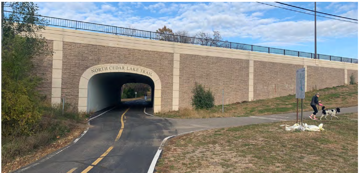
North Cedar Lake Regional Trail has several grade separated road and railway crossings. Photo credit: Park District
