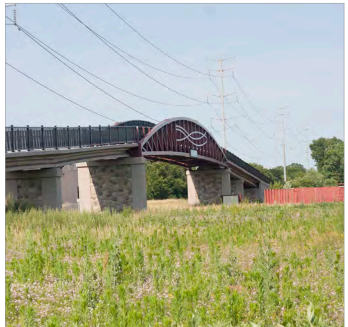
Recently constructed grade-separated bridge crossing of Xenium Lane North. Photo credit: SRF Consulting Group
