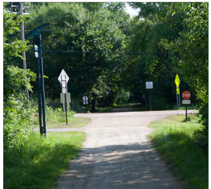
The intersection of CSAH 13 and Lake Minnetonka LRT Regional Trail recently underwent upgrades including tree removal and RRFB installation. Photo credit: SRF Consulting Group
