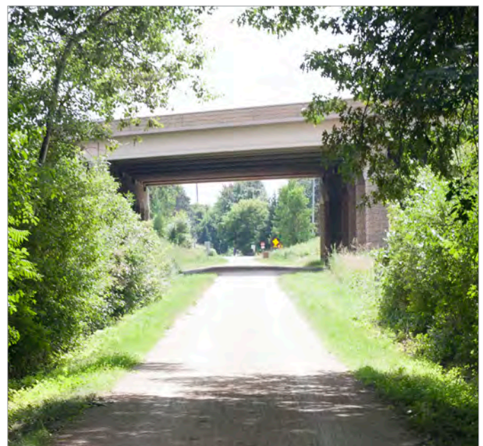
The regional trail travels under I-494. Photo credit: SRF Consulting Group
