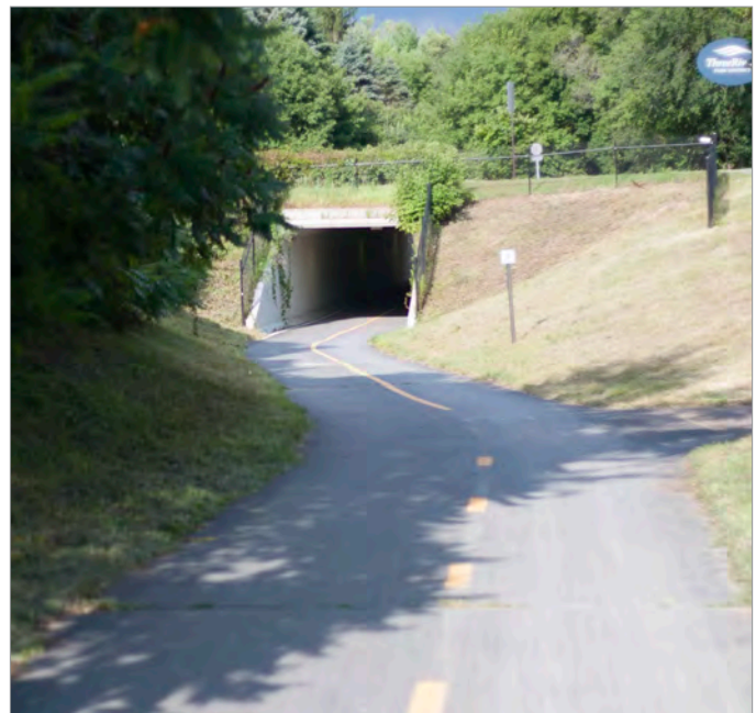
Existing grade-separated underpass of CR 101. Photo credit: SRF Consulting Group
