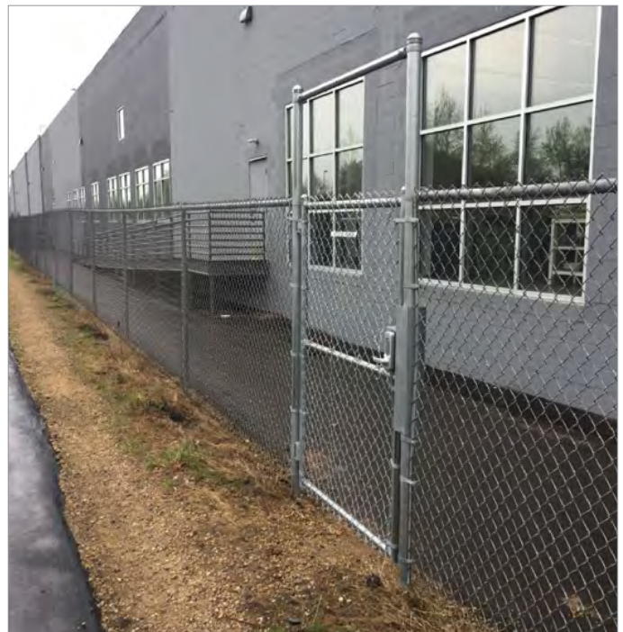
To allow greater regional trail access to and from adjacent businesses, coded gates are utilized in coordination with the Park District. Photo credit: SRF Consulting Group
