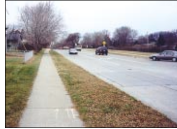
70th Street at Lynmar, looking west
