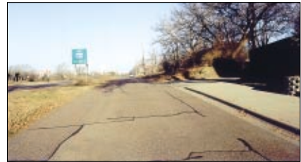
Lakeview Avenue at Twin Oak Drive, looking north
