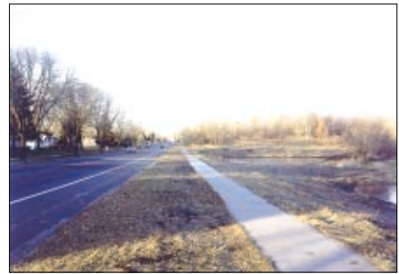
Boone Avenue south at 40 1/2 Avenue, looking north
