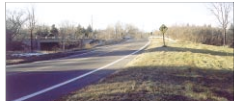
Broadway Avenue Bridge over TH 100, looking north
