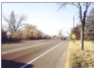
Broadway Avenue at 44 1/2 Avenue North, looking north
