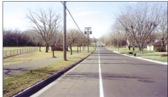
32nd Avenue at Basset Creek Park, looking west
