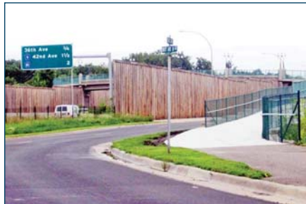
The existing TH 100 pedestrian bridge between Crystal and Golden Valley overcomes a major physical barrier to multi-modal movement.
