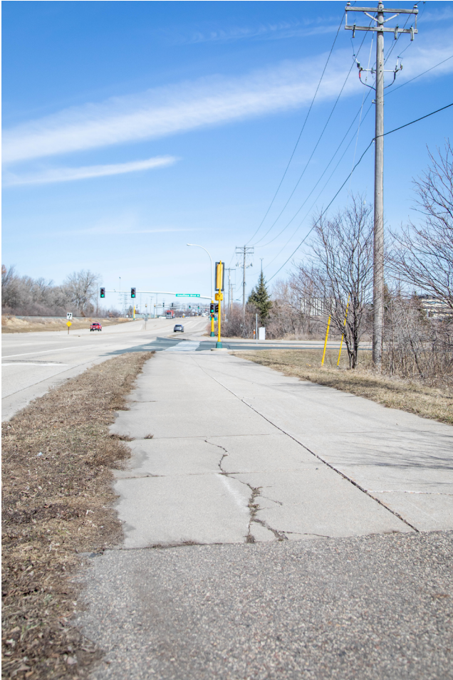
Figure 11 Discontinuous surface on CP Rail Regional Trail
