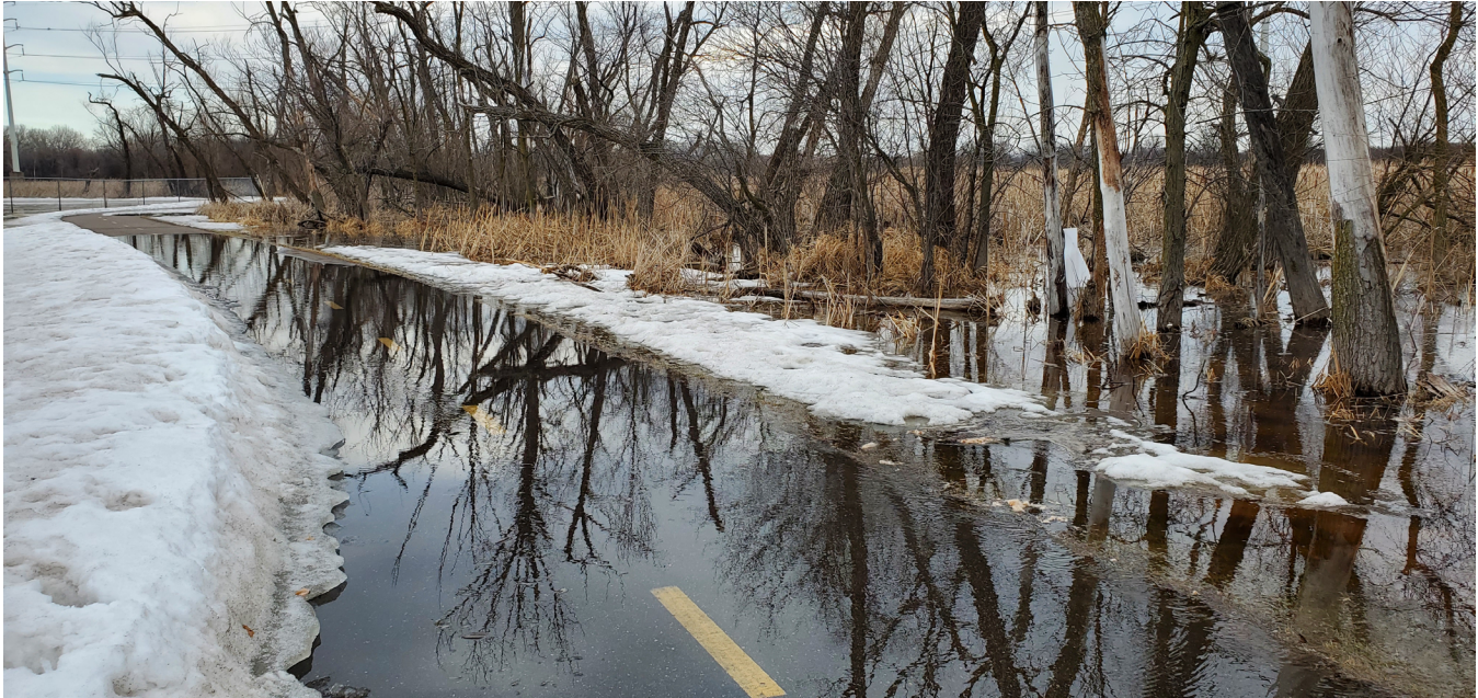
Figure 10 Shingle Creek Regional Trail Seasonal Flooding
