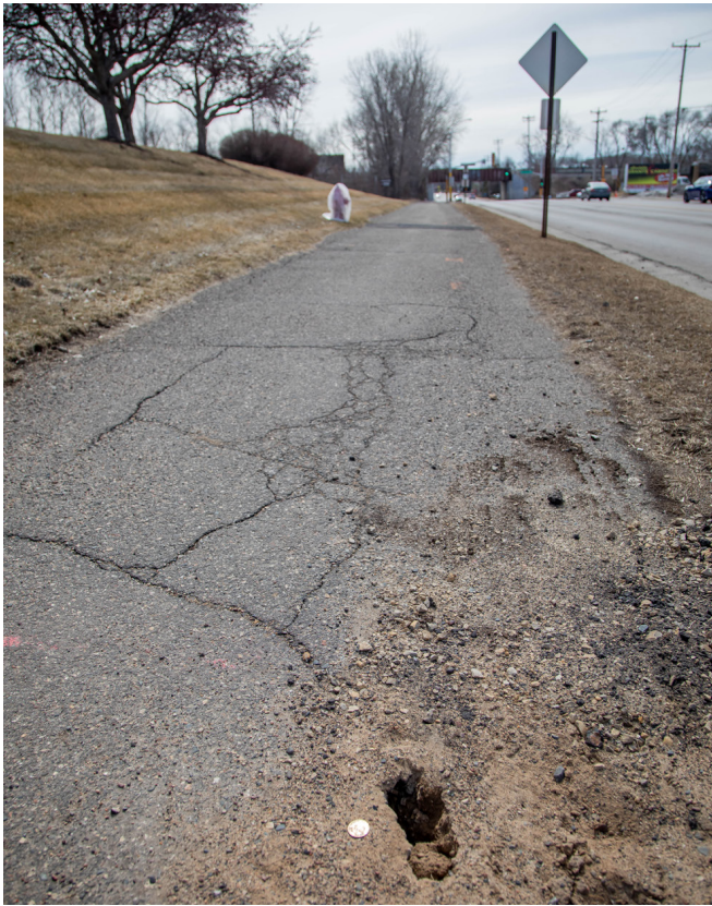
Figure 13 Typical cracking and pothole on Three Rivers’ trails at the end of the useful life
