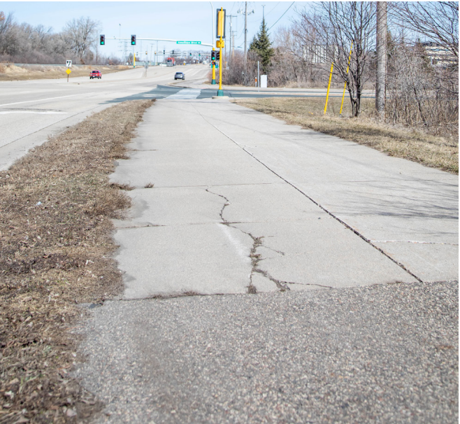
Figure 12 Typical discontinuous surface on Three Rivers’ trails
