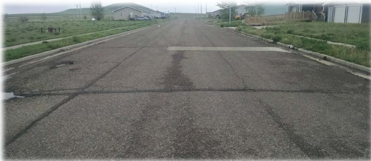
Photo of a PASER Rating 5 Road on the Standing Rock Reservation
