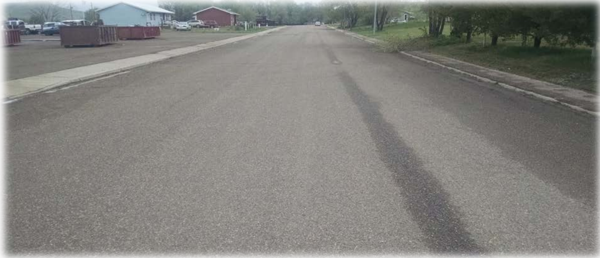
Photo of a PASER Rating 7 Road on the Standing Rock Reservation
