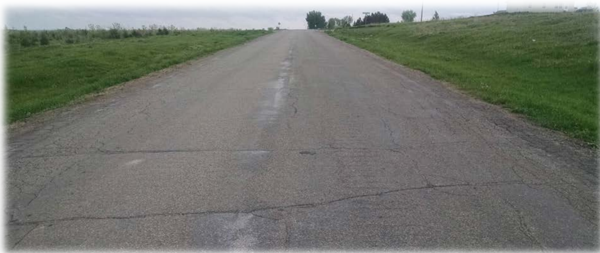
Photo of a PASER Rating 4 Road on the Standing Rock Reservation
