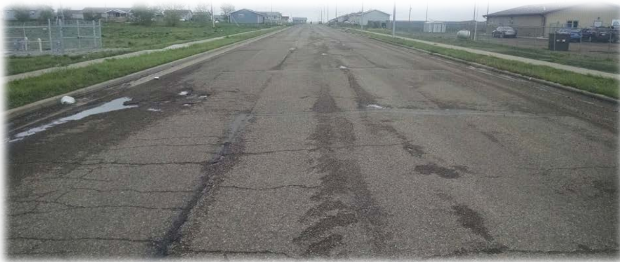
Photo of a PASER Rating 3 Road on the Standing Rock Reservation
