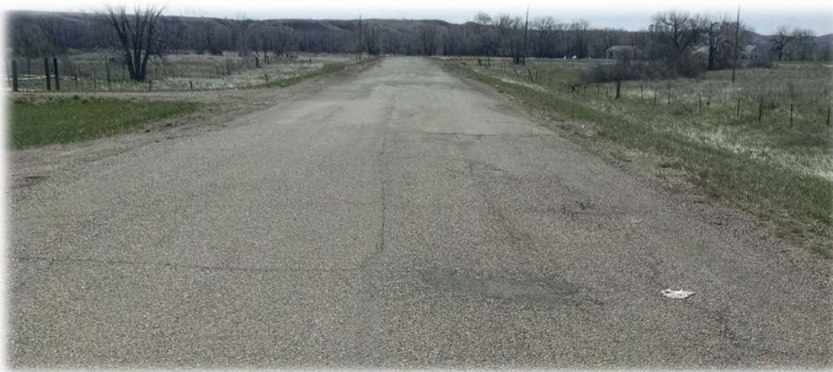
Photo of a PASER Rating 4 Road on the Standing Rock Reservation
