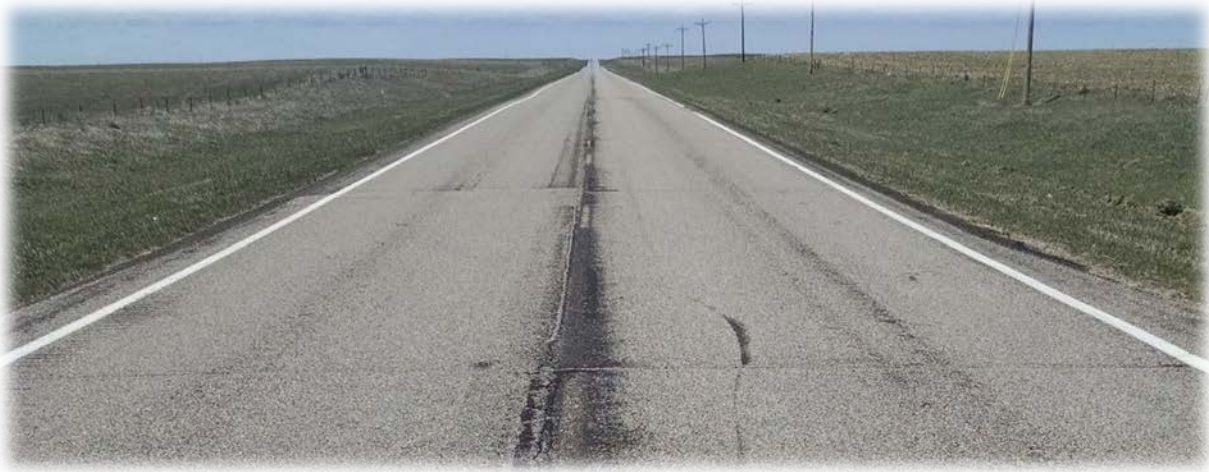
Photo of a PASER Rating 7 Road on the Standing Rock Reservation
