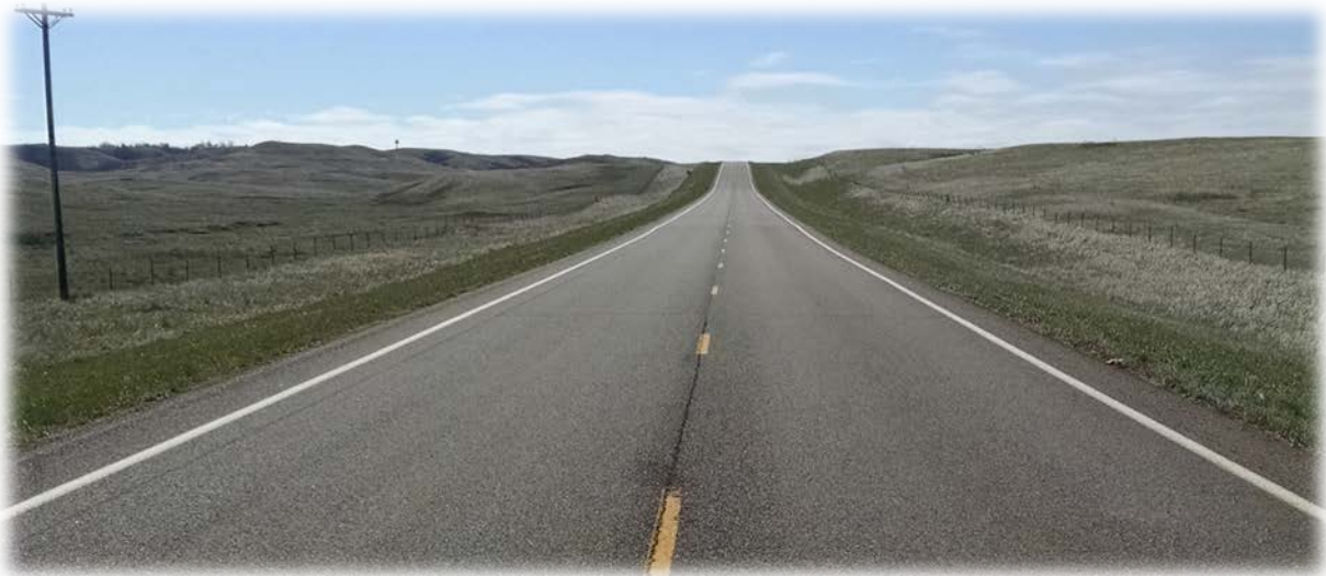
Photo of a PASER Rating 8 Road on the Standing Rock Reservation
