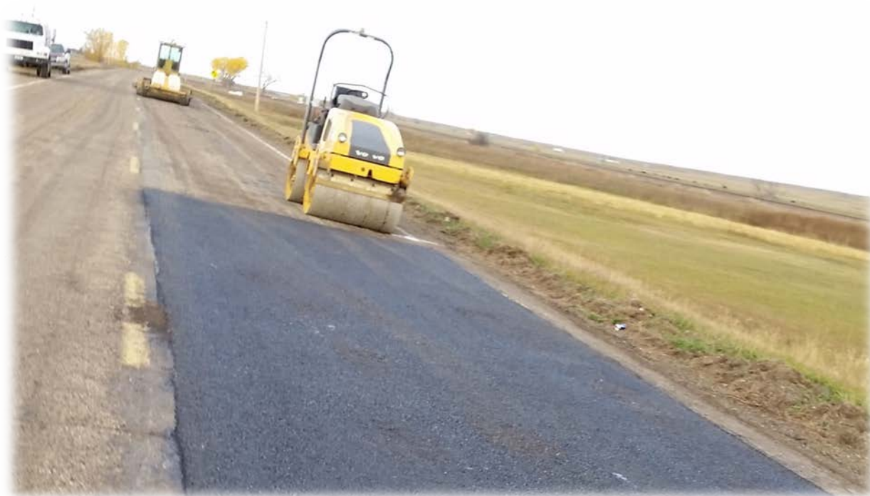
Example Photo of Road Maintenance Activities
