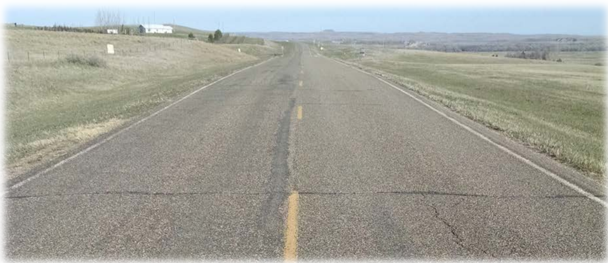
Photo of a PASER Rating 6 Road on the Standing Rock Reservation
