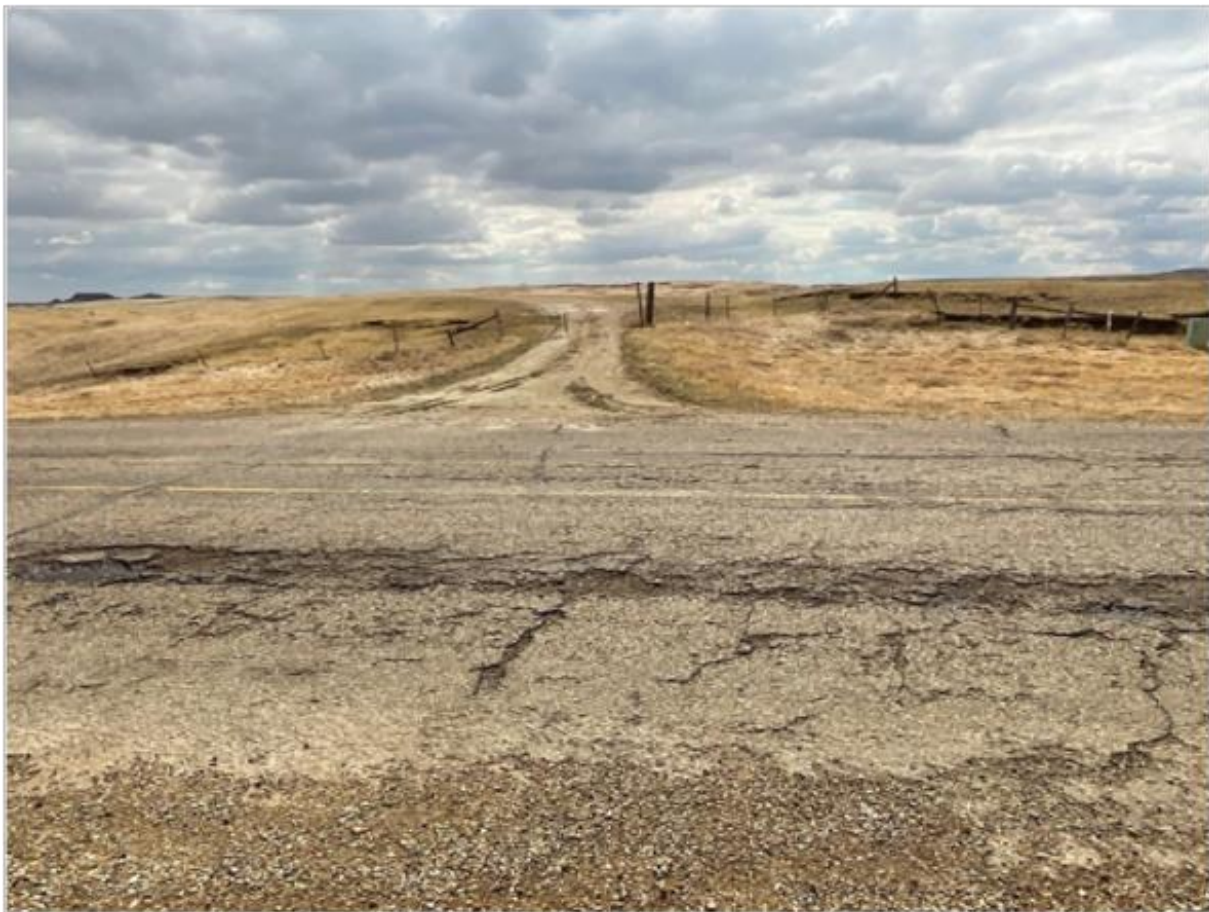
Figure 2. Existing Pavement Condition on BIA
