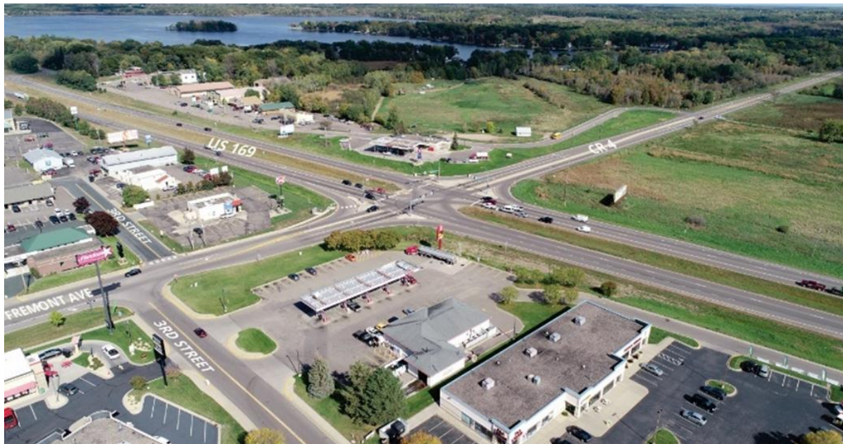
Figure 1. 169 and CR 4 Intersection Existing Conditions
