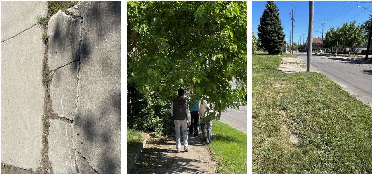
Figure 2 Existing Condition of Sidewalk
