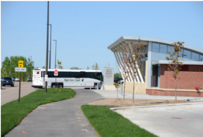
Figure 14 Existing Transit Station Adjacent to the Project
