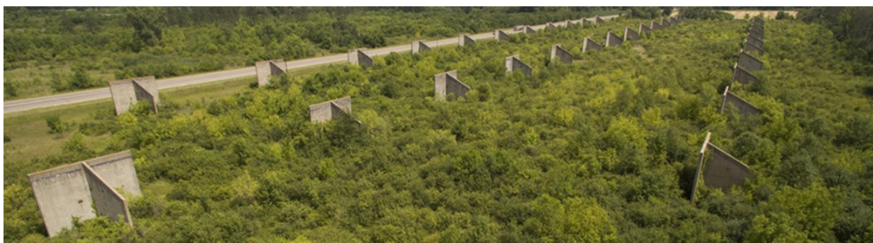
Figure 13 T Walls from Old WWII Gunpowder Manufacturing Site within Project Area.
