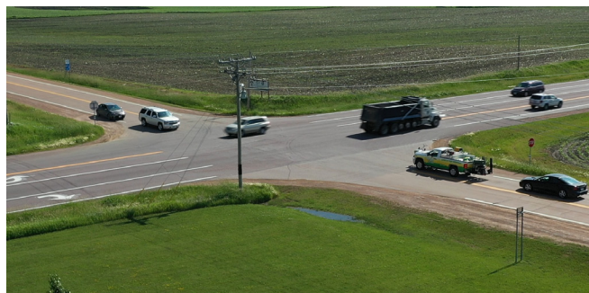
Inadequate turning radii for trucks at intersection
