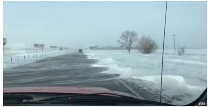
Dash cam footage (above) showing the difference in roadway conditions between a portion of I-94 near Moorhead with (left) and without (right) standing corn row snow fences, during the same blowing snow event with winds of 30 miles per hour (January 29, 2019). During this event, one foot snow drifts formed rapidly on roadways that were not protected by snow fencing.
