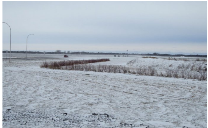
Living snow fencing with berm with snow catch points.
