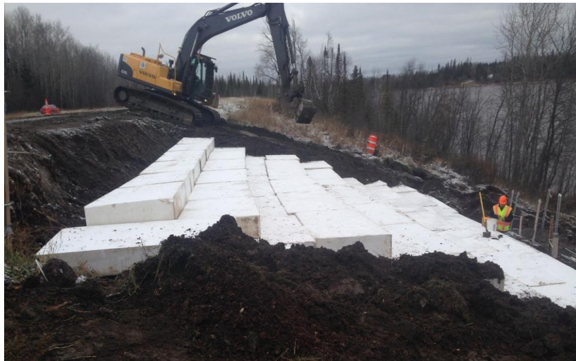
Figure 3. Foam Installation for Slope Stability
