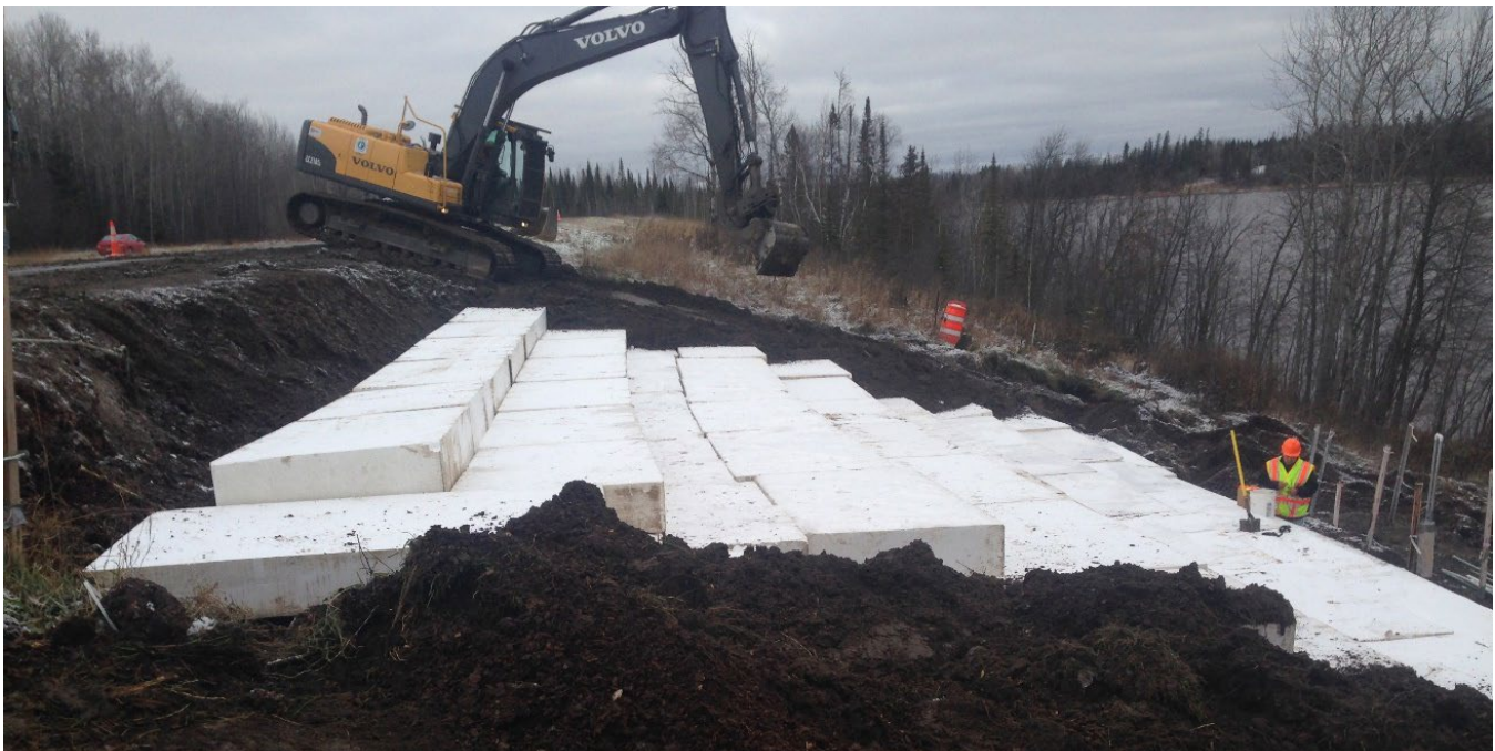
Foam installation to help stabilize the southern slide.
