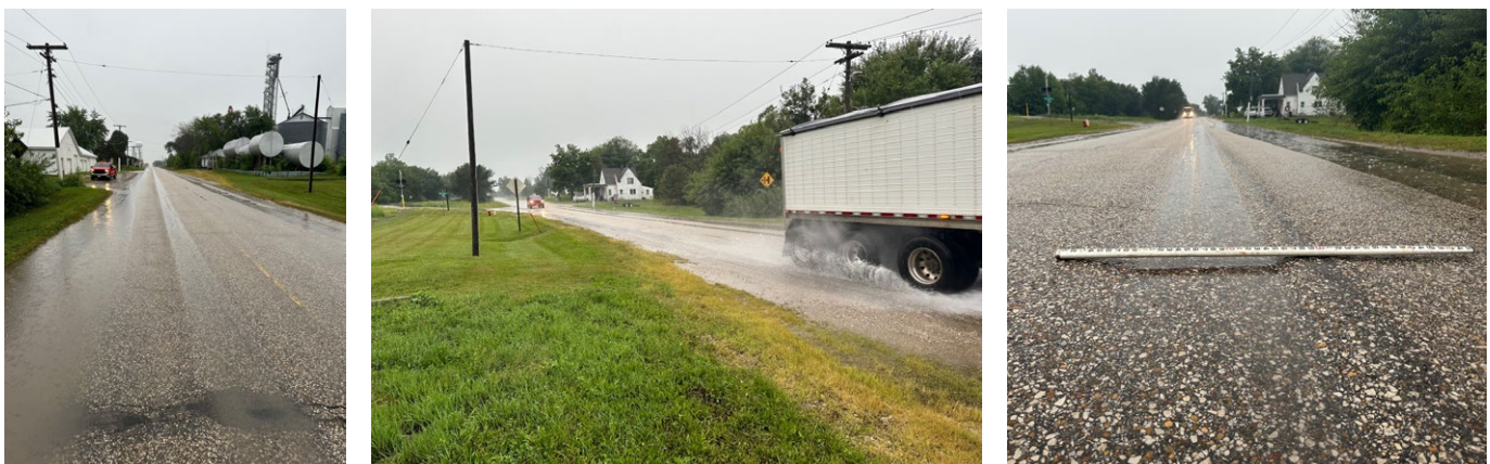
Figure 8 Drainage issues along F65 in Guthrie County
