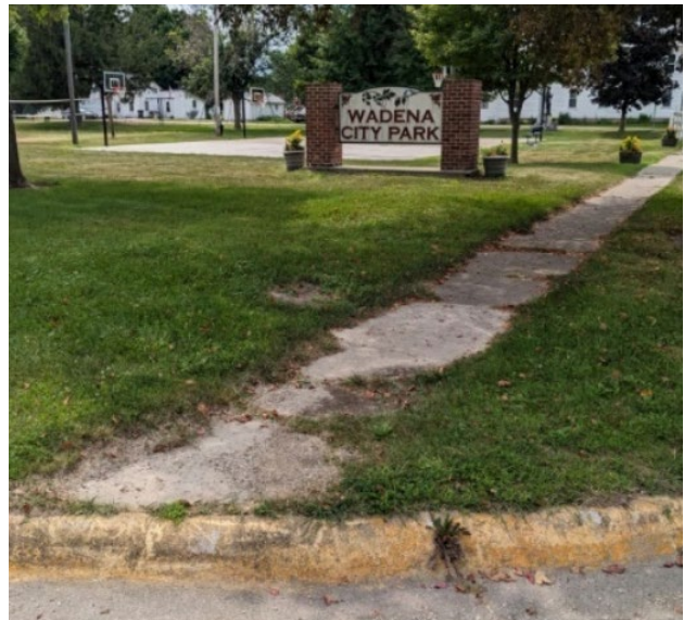
Figure 10 Fayette County W51 Project
