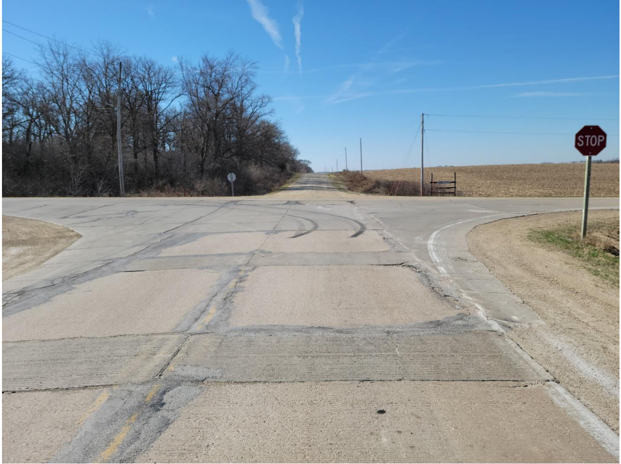
Figure 50: V18/Fayette Ave. intersection with 110th St./V18 (Facing South)
