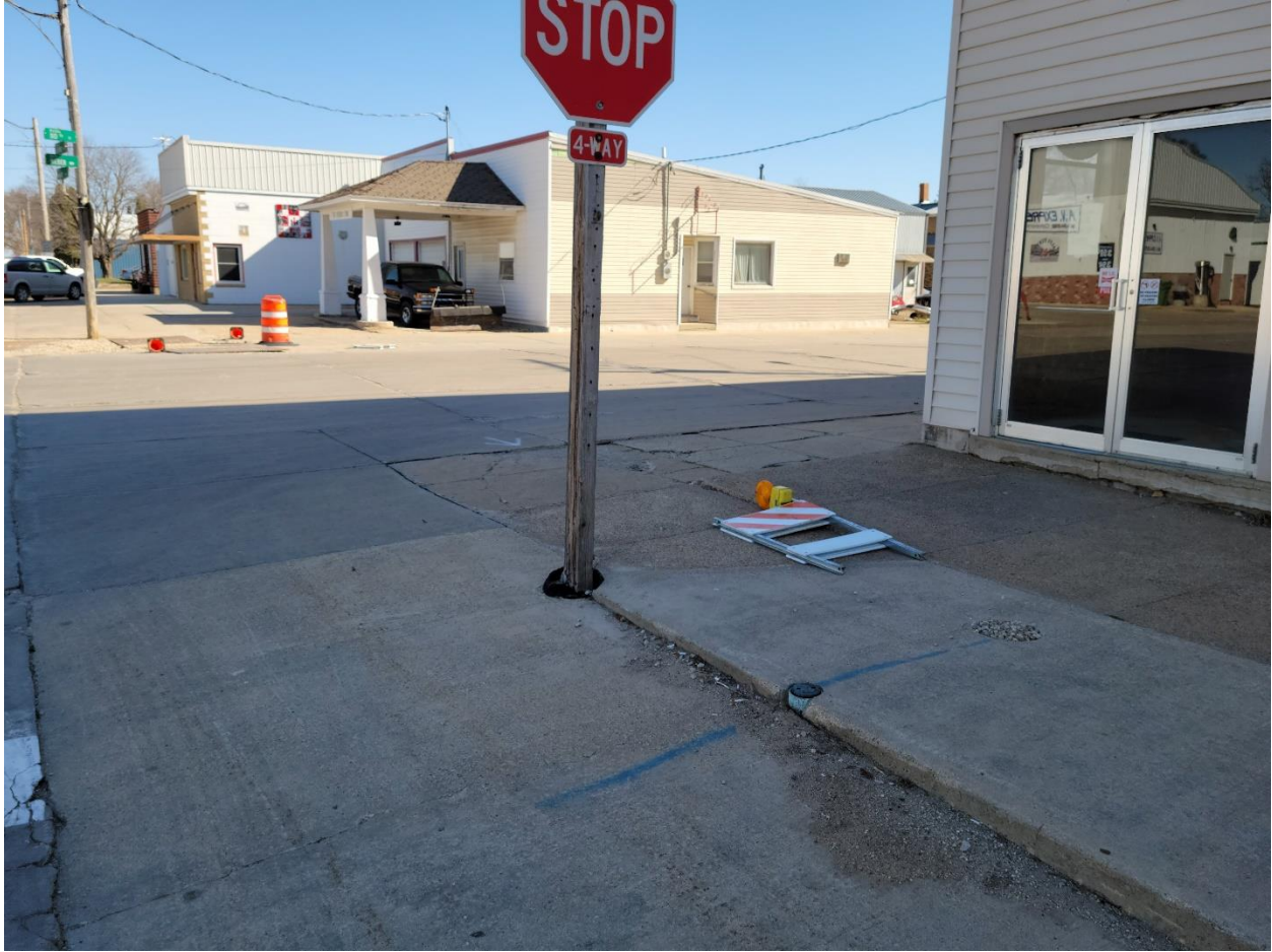
Figure 30: Existing sidewalk/curb at Southeast corner of South White St./Weber St. Intersection next to Schuckys Bar & Grill (Facing Northeast)
