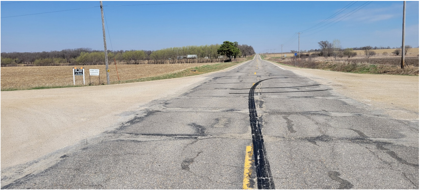
Intersection with 100 th St. Looking North.
