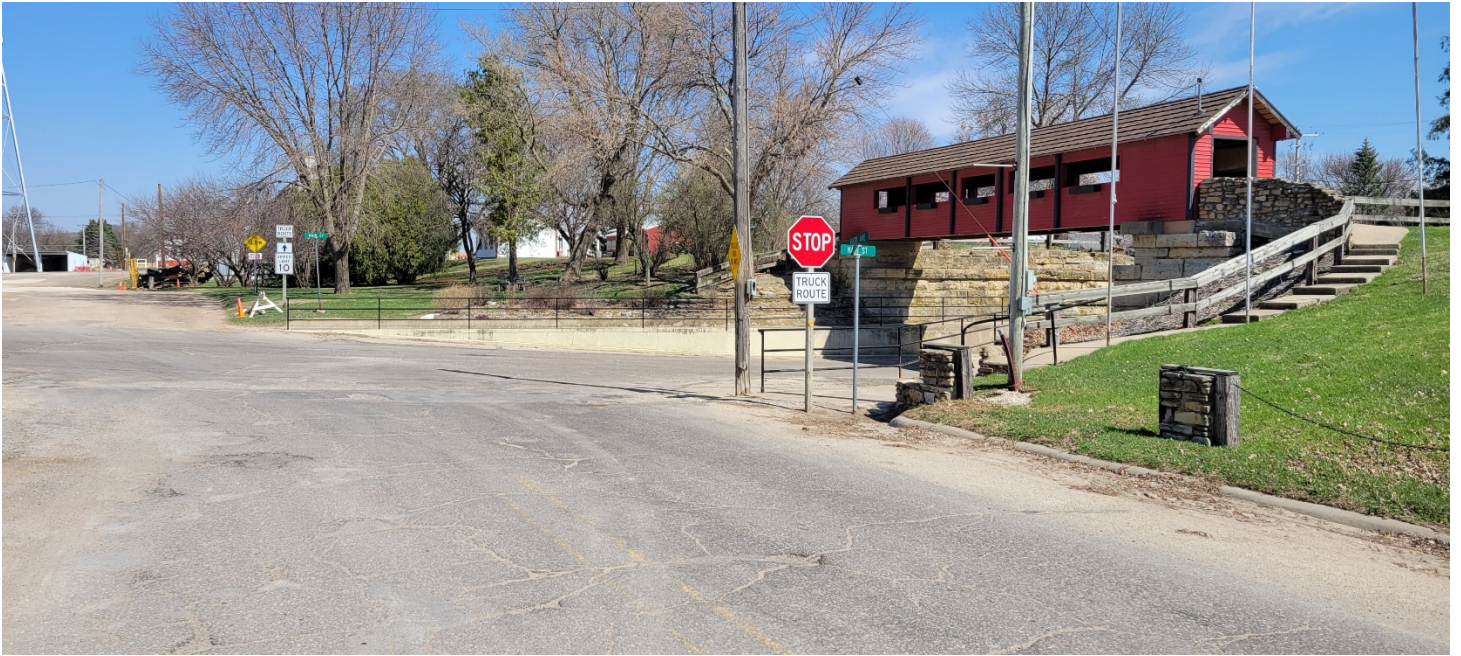
End of Project. Looking North
