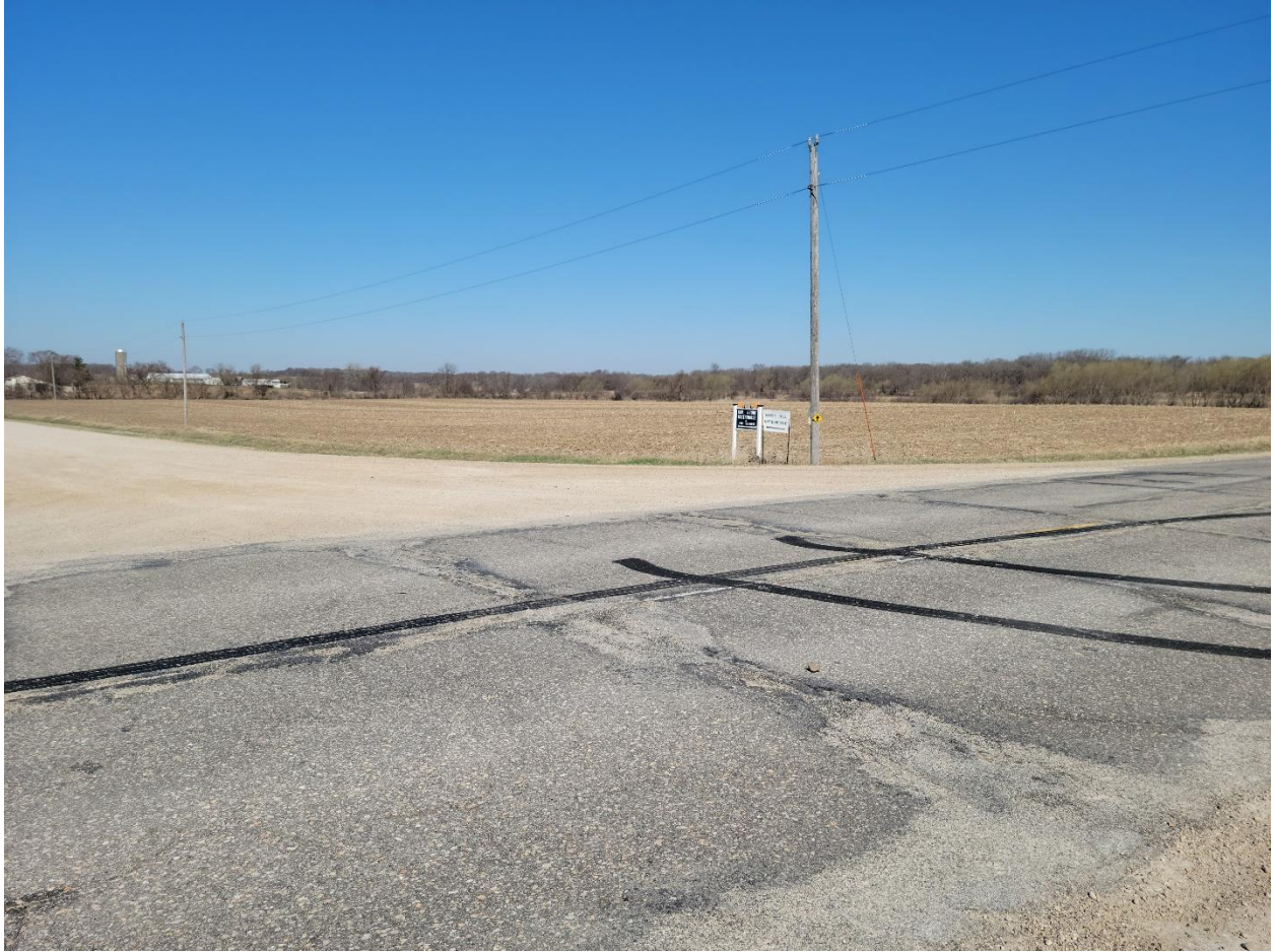
Figure 53: V18/Fayette Ave. at Chickasaw/Howard County Line (Facing Northwest)
