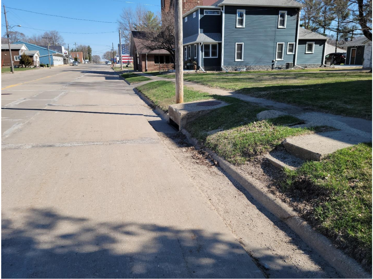
Figure 15: South White St. East side existing sidewalk, curb/gutter and intake (Facing North)
