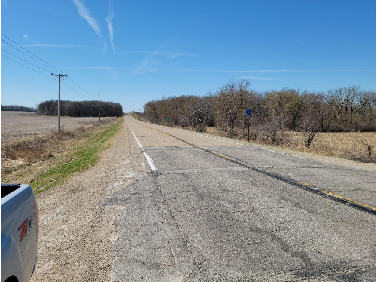
Figure 54: V18/Fayette Ave. at Chickasaw/Howard County Line (Facing South)
