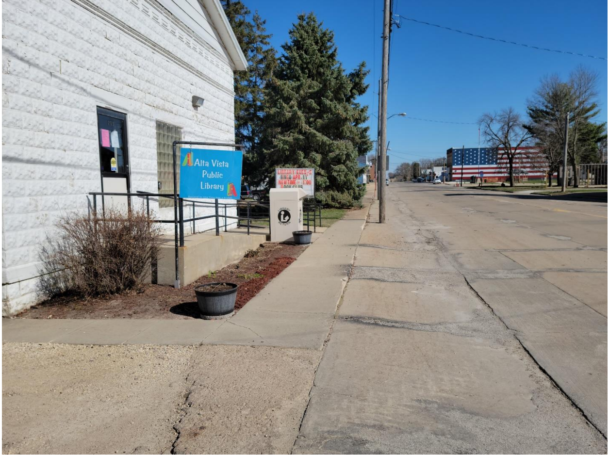
Figure 17:South White St. West side existing sidewalk next to Public Library (Facing North)
