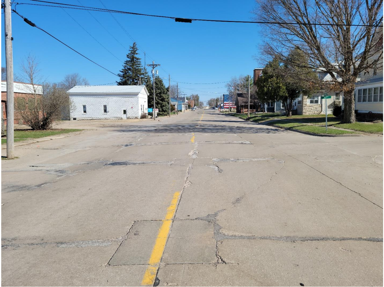
Figure 14: South White St./Alt St. Intersection (Facing North)
