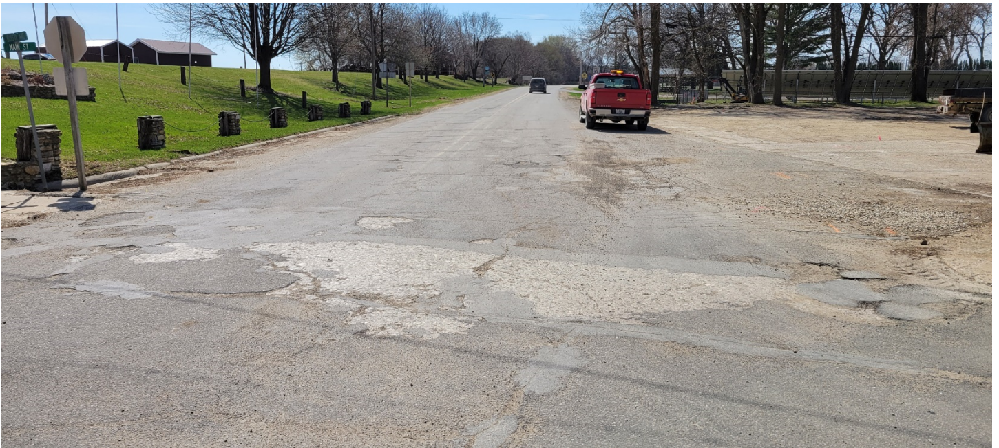
End of Project. Looking South
