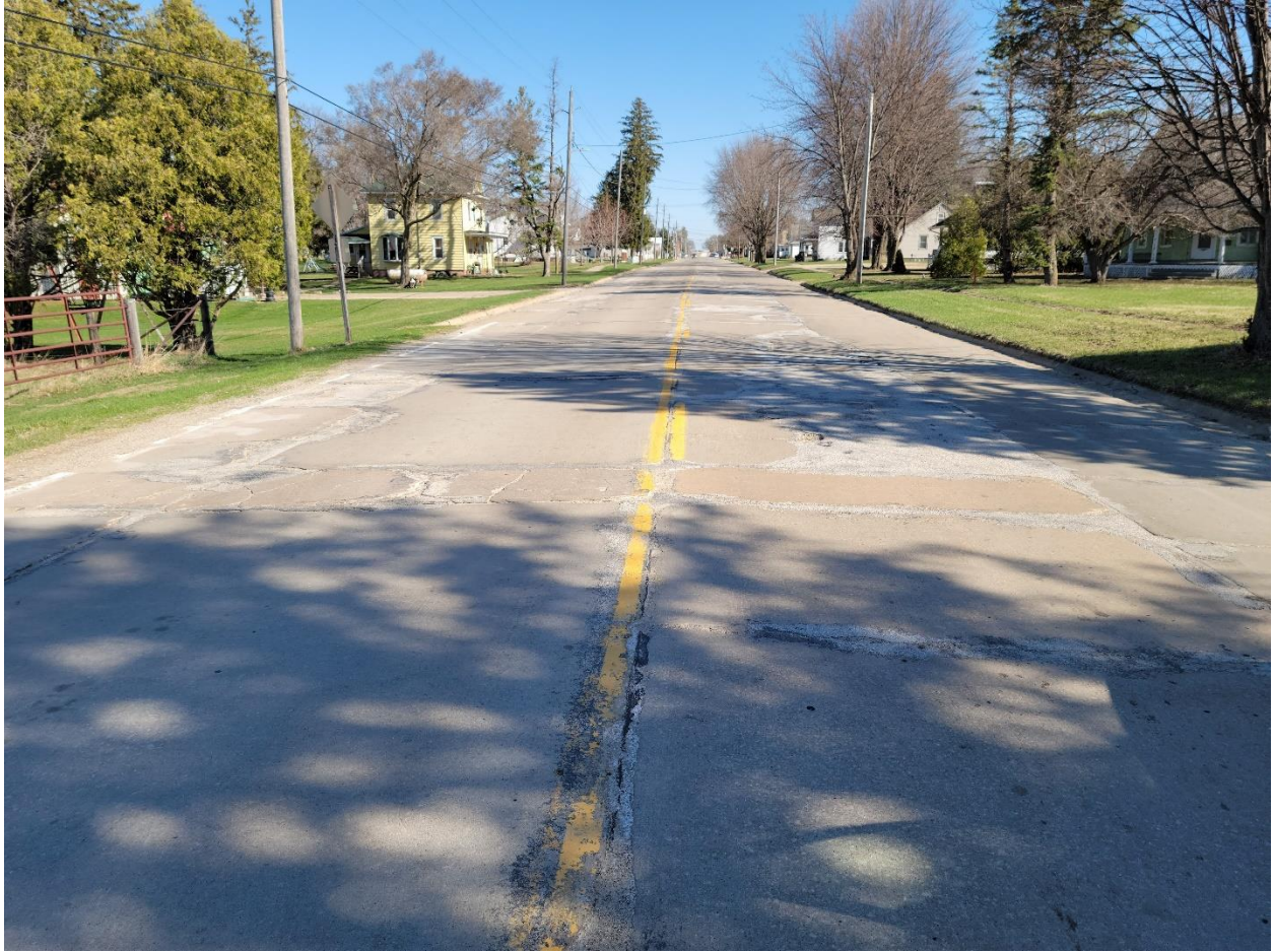
Figure 4:South White St. (Facing North)
