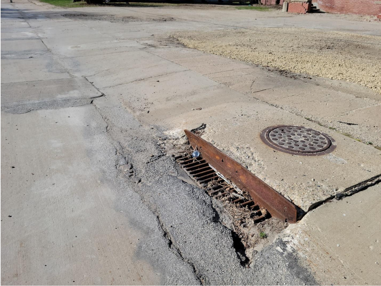
Figure 18: South White St. West side existing intake (Facing Southwest)
