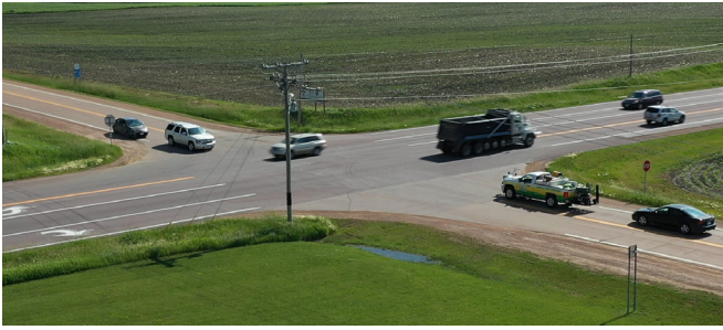
Inadequate turning radii for trucks at intersection
