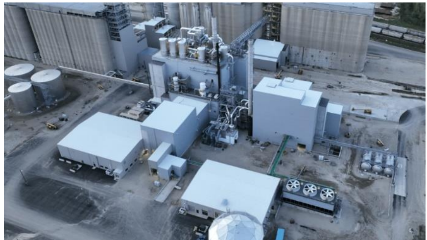
Figure 4. Green Bison Soybean Processing Plant
