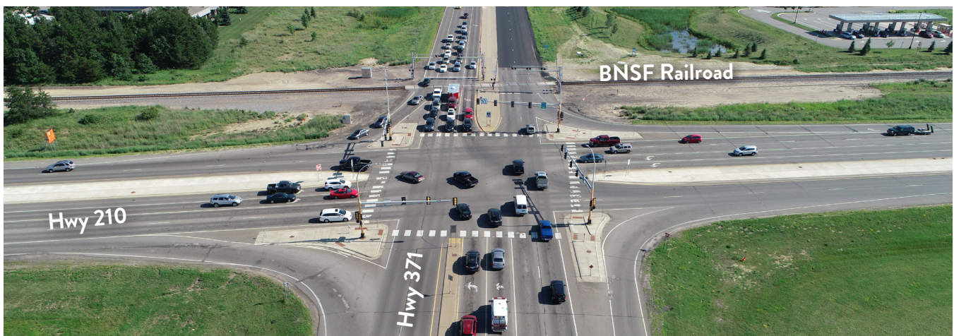
Figure 2 Congestion along Hwy 371 at the BNSF railroad at-grade crossing (Source: KLJ)
