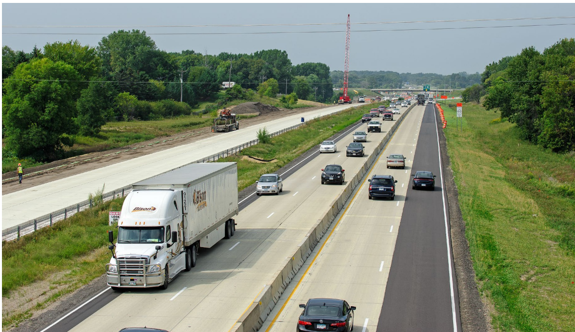
Construction along I-94 near TH 241. Source: District 3 Staff
