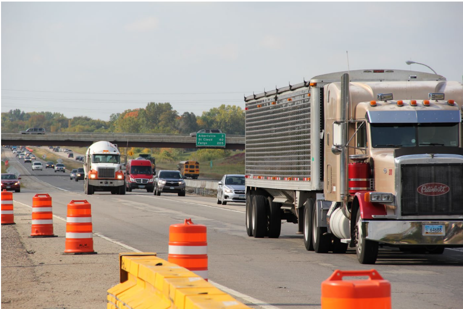
Construction on I-94 near Albertville. Source: MnDOT District 3 Staff
