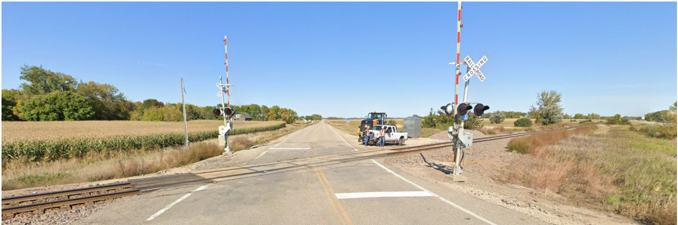
Railroad crossing at CSAH 55
