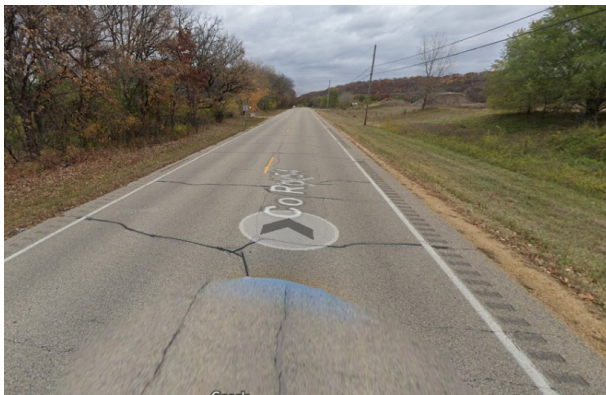
Figure 14 Cracking along CSAH 54.
