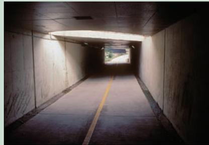
**Contrast of sightlines.** Both of these box culverts provide adequate light for visitor safety. The light opening in the center of the box culvert in the right photo greatly improves visibility and will be more accepted by the user. Notably, in both of these cases the shoulder is minimal due to site limitations. For this not to be an issue, visual cues, adequate sightlines, and signage before entering the tunnels are important to alert trail users to a narrowed section.
