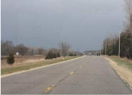
(Looking south) Ravenna Trail from Hastings to the junction of County Road 18 does not have an adequate shoulder to accommodate a bike route.
