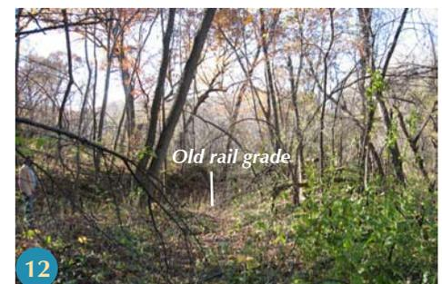
(Looking southeast) As with much of the old rail grade, brush removal and remedial grading will be necessary to prepare the grade for building the trail.
