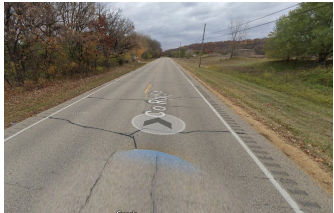
Figure 15 Cracking along CSAH 54.
