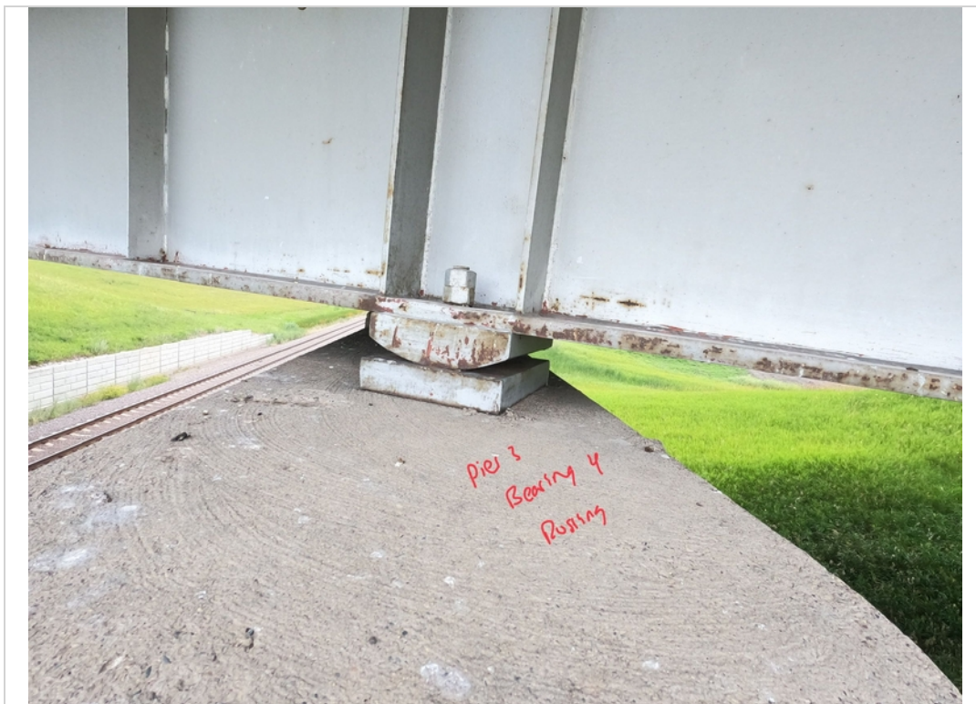
Facing North. Rusting to Pier 3 Bearing 4.
