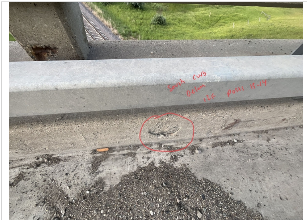
Facing South. Delamination to South Curb in-between Posts 14 and 15.
