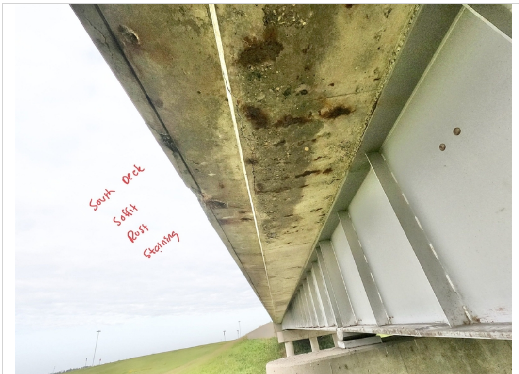
Facing West and Upwards. Rust Stains to South Soffit.
