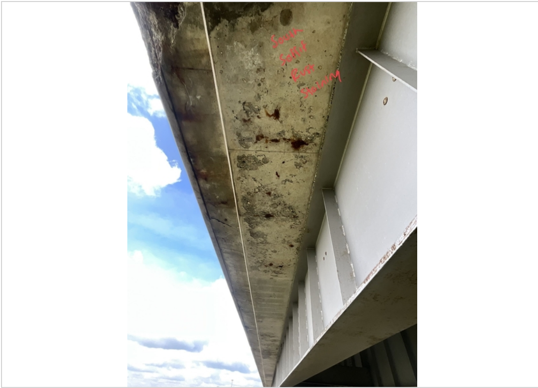
Facing West and Upwards. Rust Staining to South Deck Soffit in Span 3.
