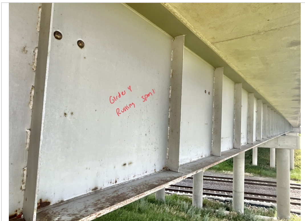
Facing NW. Rusting to Girder 4 in Span 1.
