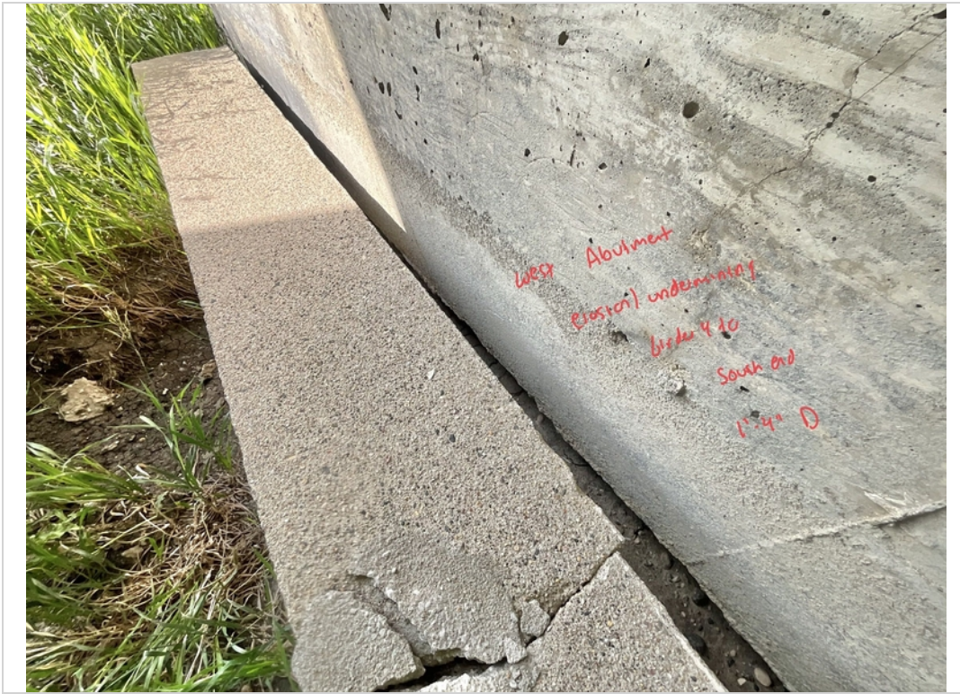
Facing SW and Downward. Erosion and Undermining along West Abutment South End.
