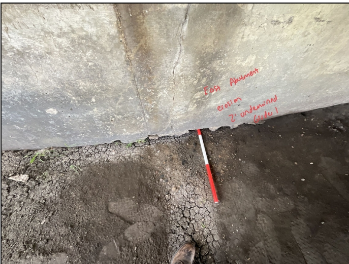
Facing East and Downward. Erosion and Undermining to East Abutment in-between Girders 1 and 2.
