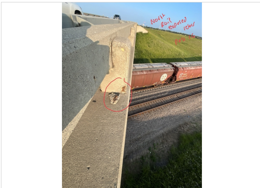
Facing West. Exposed Rebar to North Railing at Post 16.
