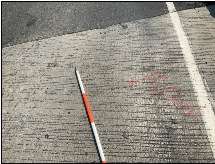
Facing East and Downward. Various cracking to Deck Wearing Surface in the EB Lane near East End.
