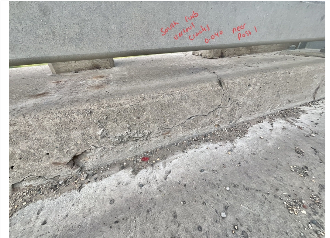
Facing SW. Horizontal Crack to South Curb near Post 1.
