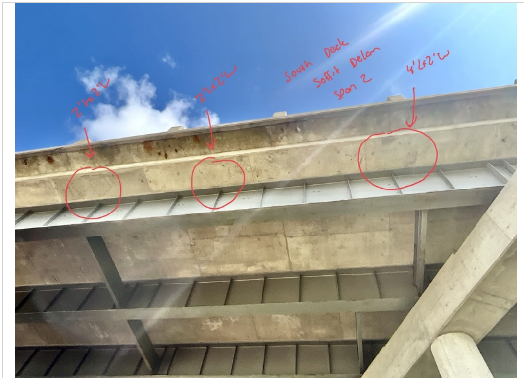
Facing North and Upwards. Areas of Delamination to South Deck Soffit in Span 2.
