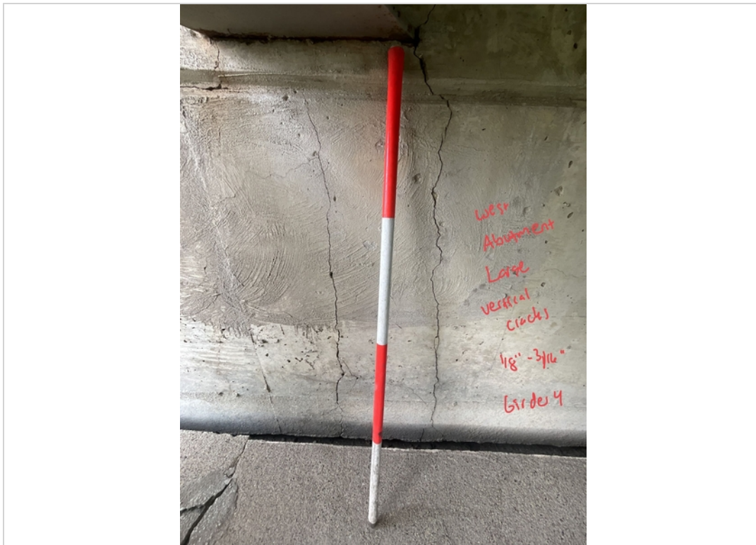
Facing West. Large Vertical Cracks to West Abutment under Girder 4.
