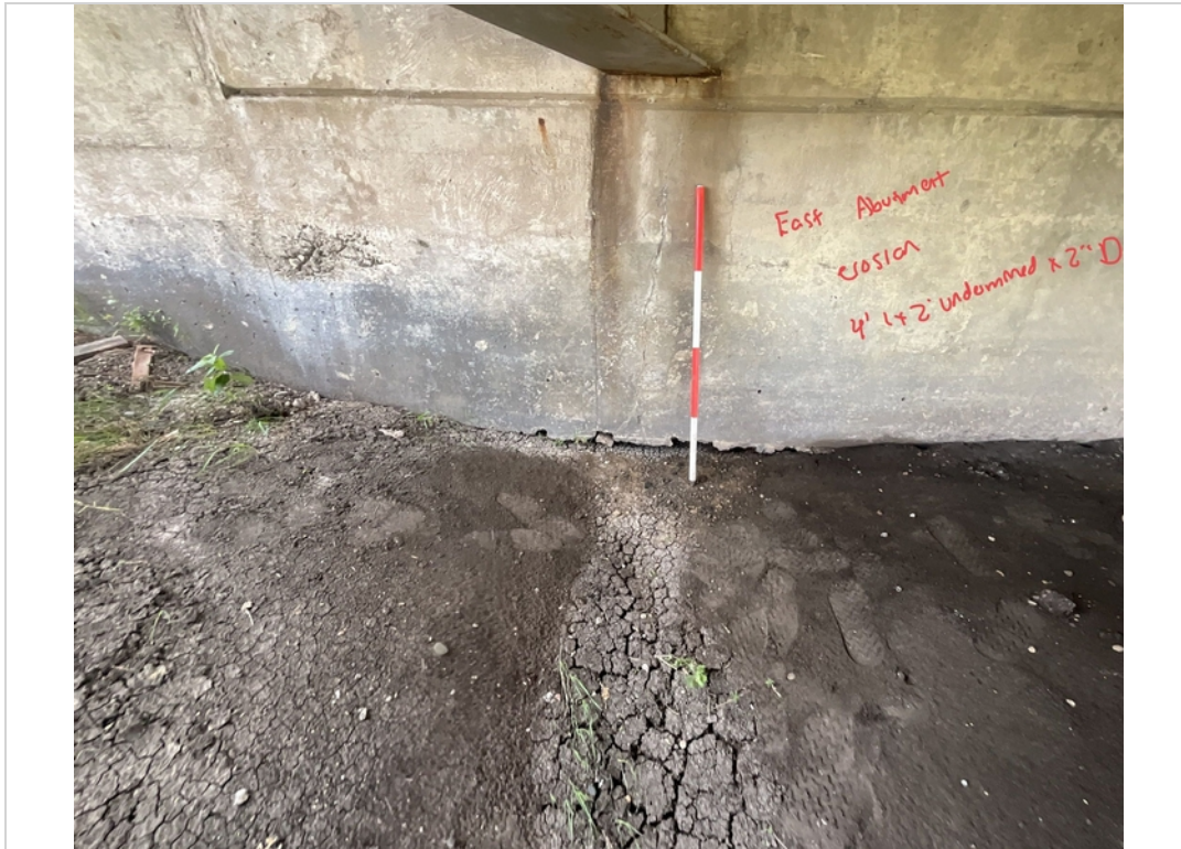
Facing East. General area of Erosion along East Embankment Slope in-between Girders 1 and 2.
