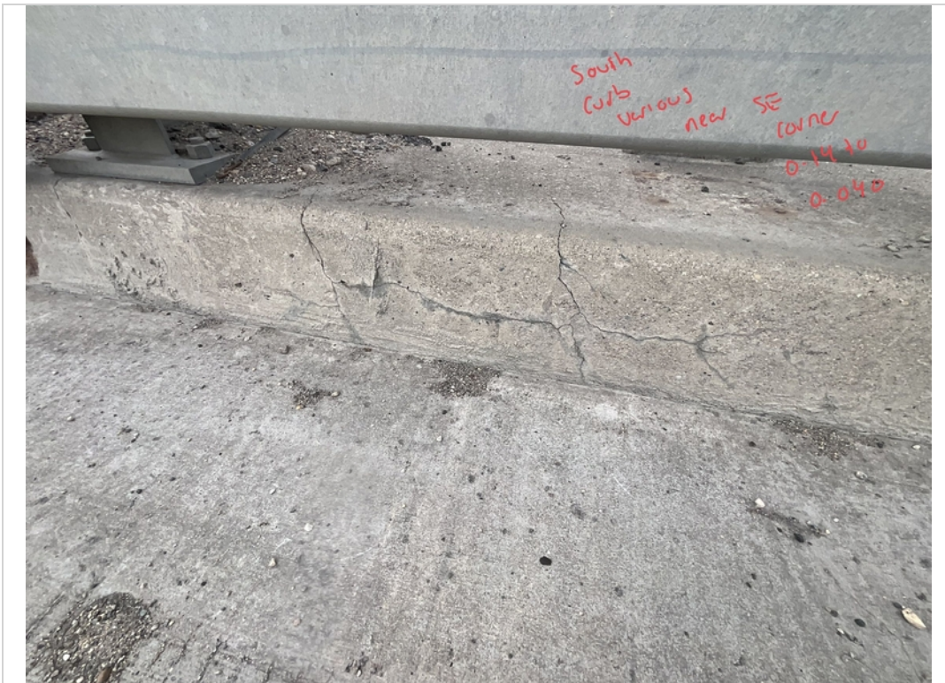
Facing South and Downward. Various Cracking to South Curb near SE Corner.
