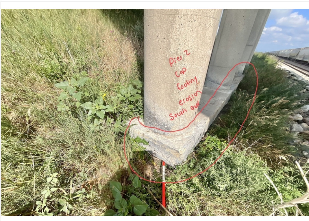
Facing NW and Downward. Erosion and Undermining area along Pier 2 Cap Footing South End.
