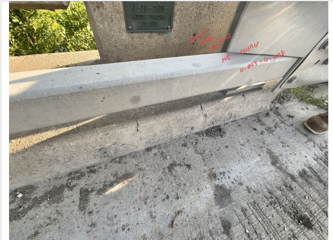
Facing North. Cracking to North Curb near NE Corner.
