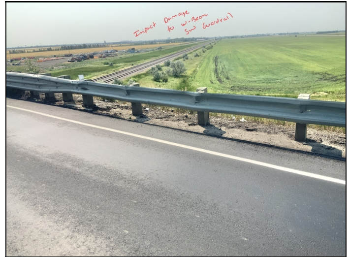
Facing SE. Another View of the Vehicle Impact to the W-Beam with the SW Quadrant.
