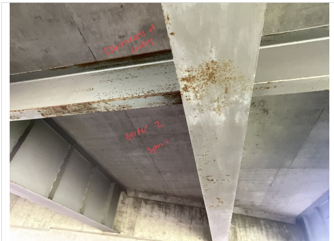
Facing West and Upwards. Effectiveness of Coating underside bottom flange of Girder in Span 1
