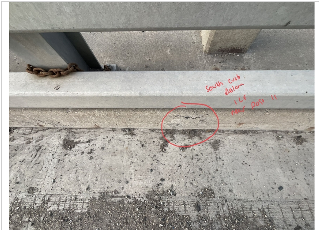
Facing South. Delamination to South Curb at Post 11.
