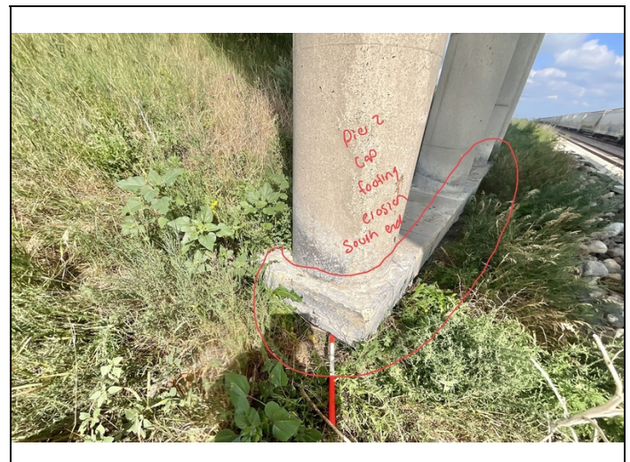
Facing NW and Downward. Erosion and Undermining area along Pier 2 Cap Footing South End.
