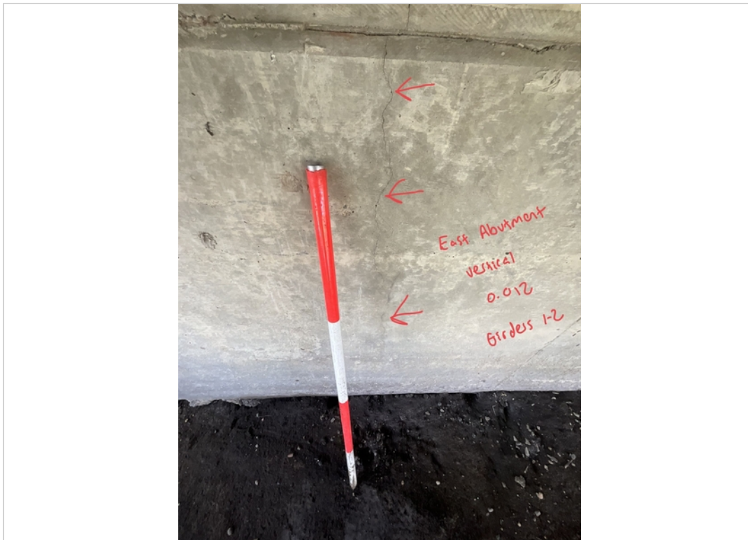
Facing East. Vertical Crack to East Abutment in-between Girders 1 and 2.
