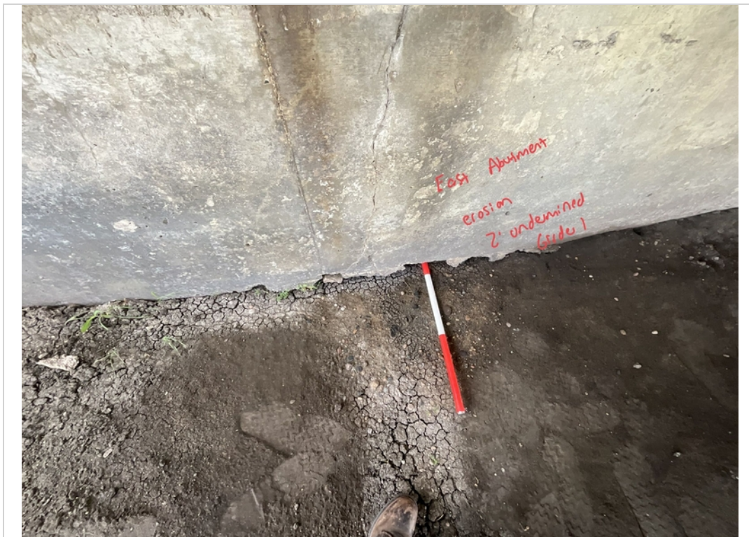
Facing East and Downward. Erosion and Undermining to East Abutment in-between Girders 1 and 2.
