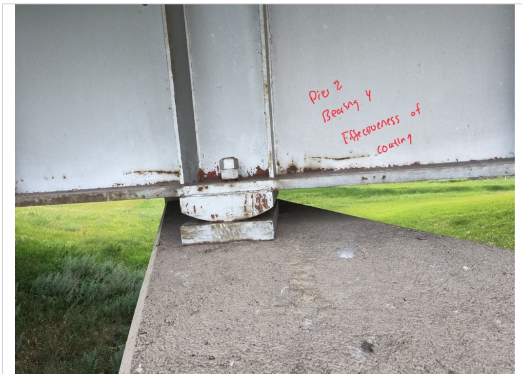
Facing North. Effectiveness of Coating to Pier 2 Bearing 4.
