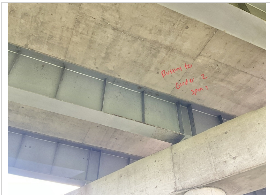
Facing NE and Upwards. Rusting to Girder 2 near Pier 2.
