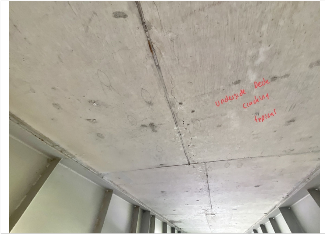
Facing West and Upwards. Underside Deck Cracking throughout. Typical.
