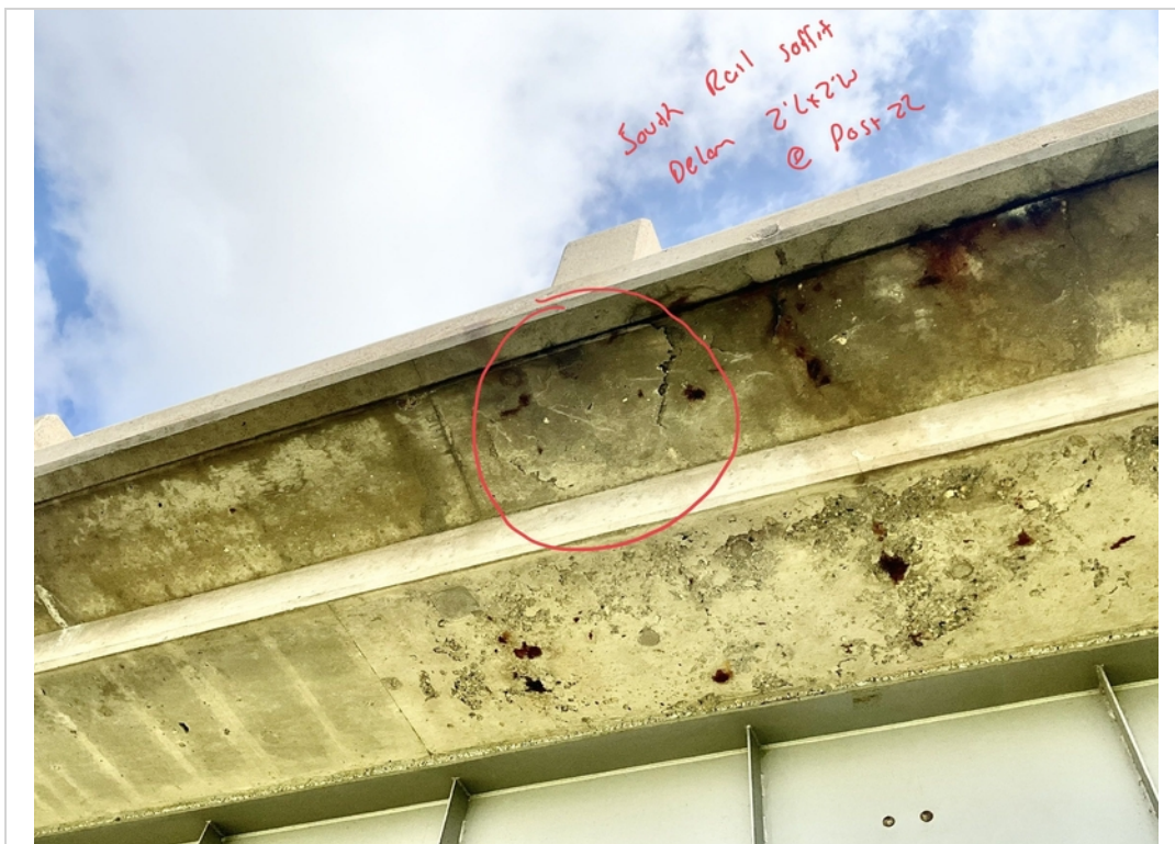
Facing NW and Upwards. Delamination to South Railing Soffit at Post 22.
