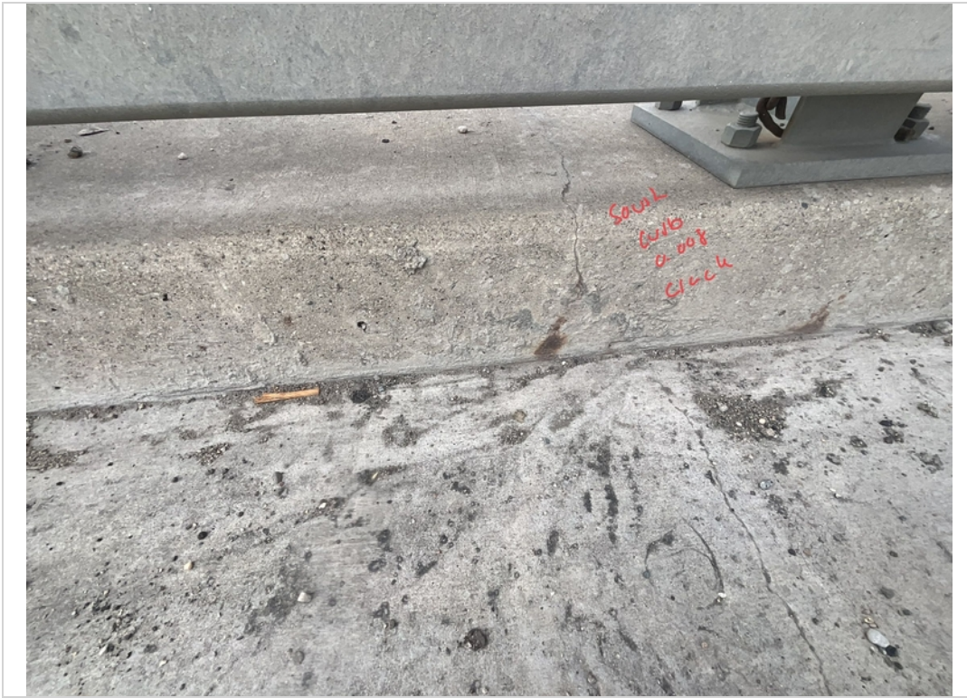
Facing South. Crack to South Curb.
