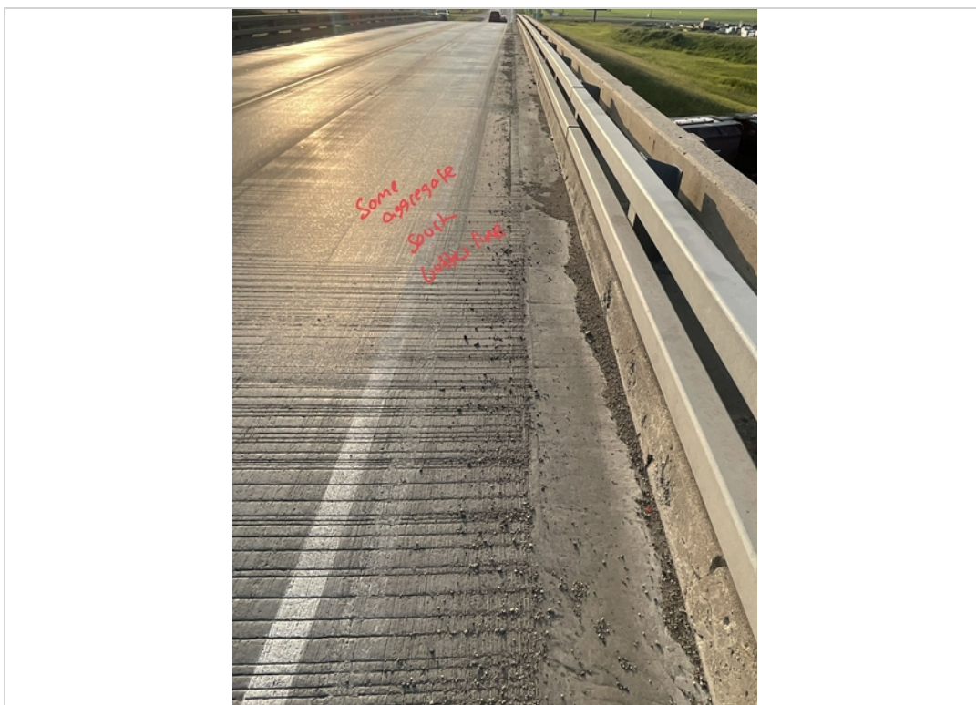
Facing East and Downward. Aggregate along South Gutter Line.
