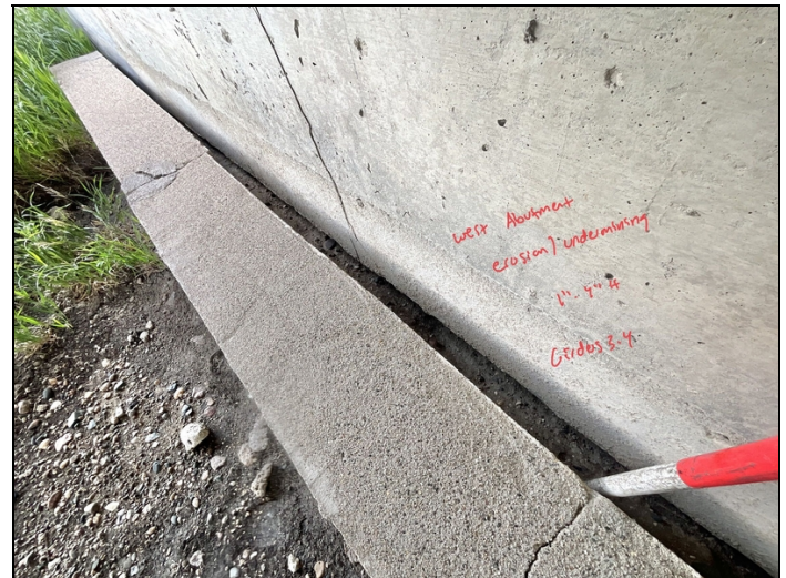
Facing SW and Downward. Continued Erosion along West Abutment from Girders 3 to 4.
