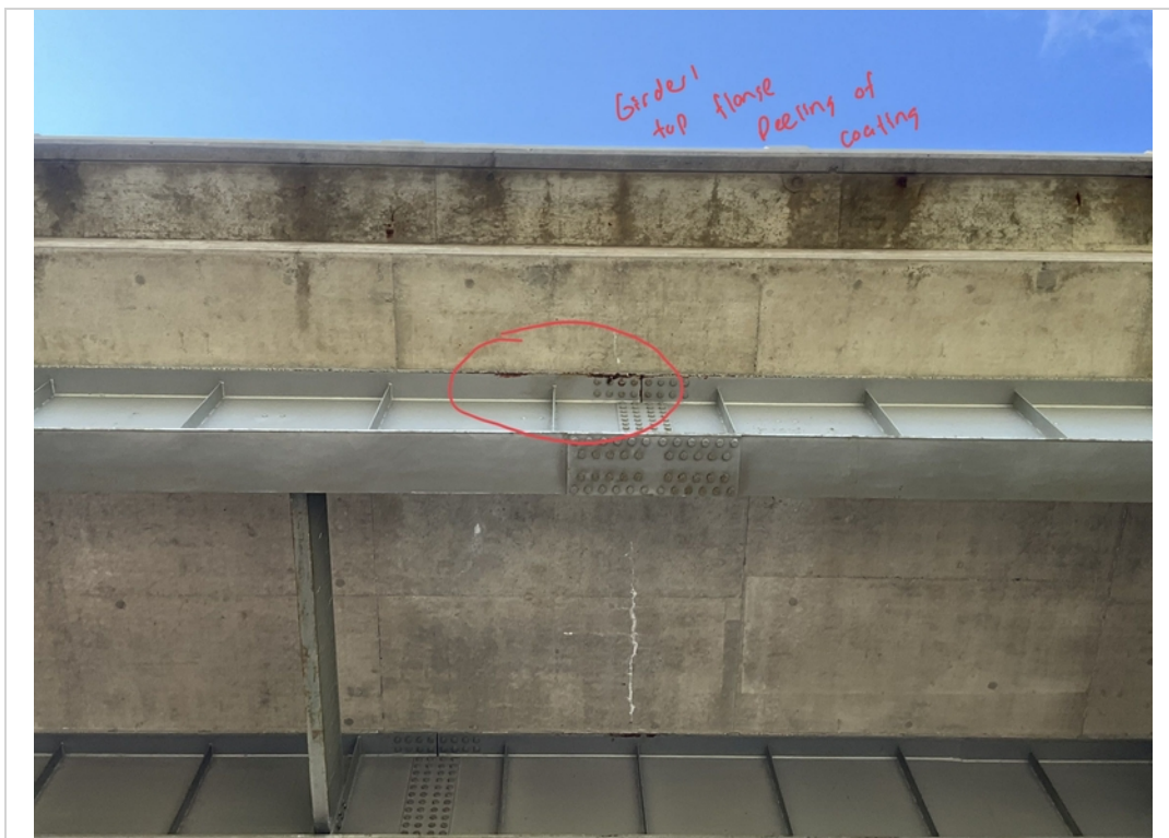
Facing South and Upwards. Peeling of Coating to Girder 1 Top Flange in Span 2.
