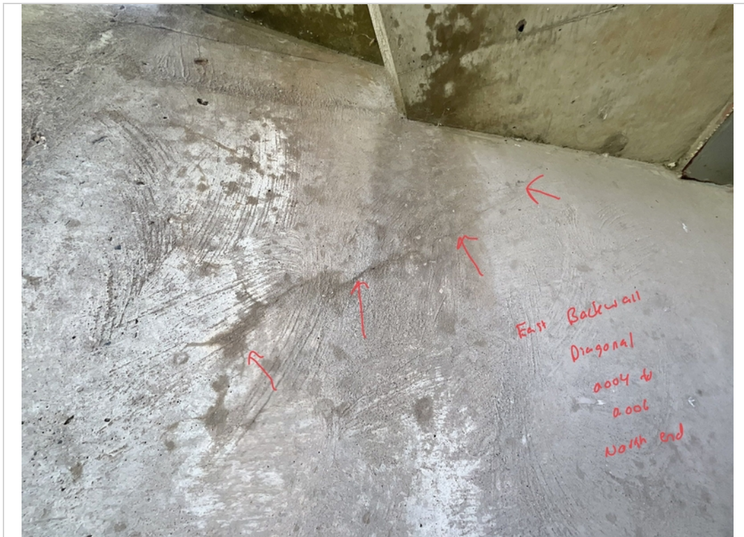
Facing East and Upwards. Diagonal Crack to East Backwall North of Girder.
