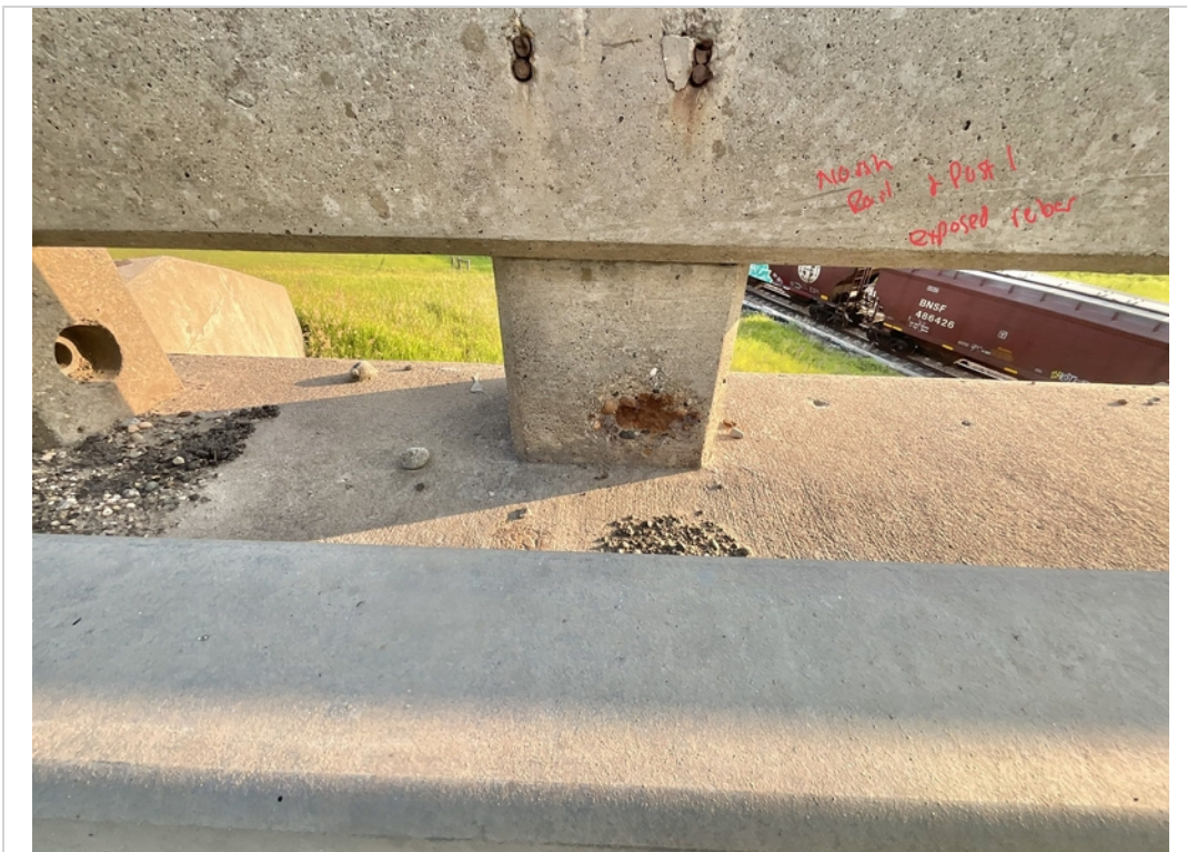
Facing North. Exposed Rebar to North Railing at Post 1.
