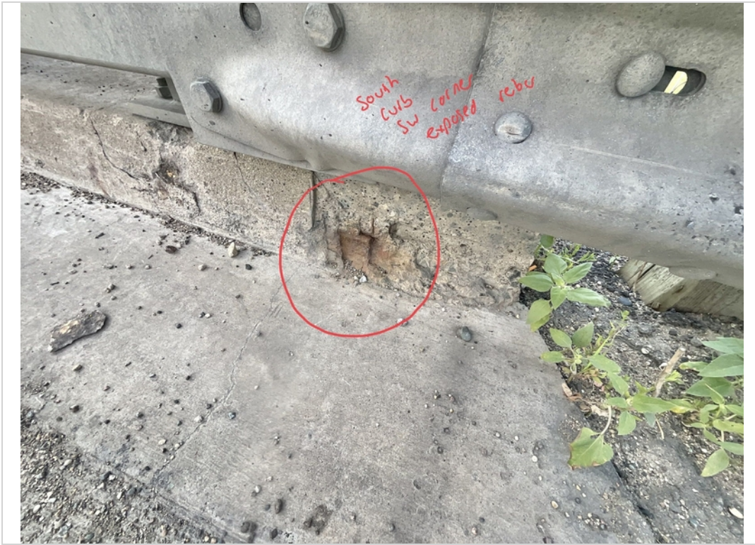
Facing South. Exposed Rebar to South Curb near SW Corner.
