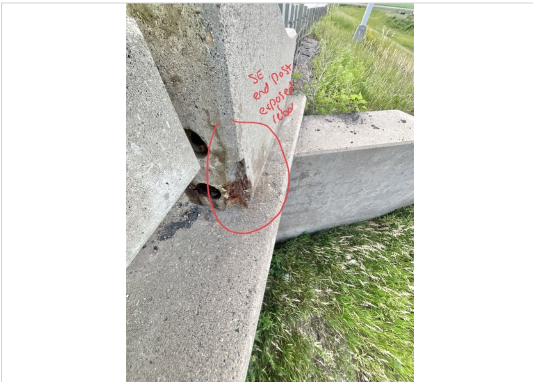
Facing East. Exposed Rebar to SE End Post.
