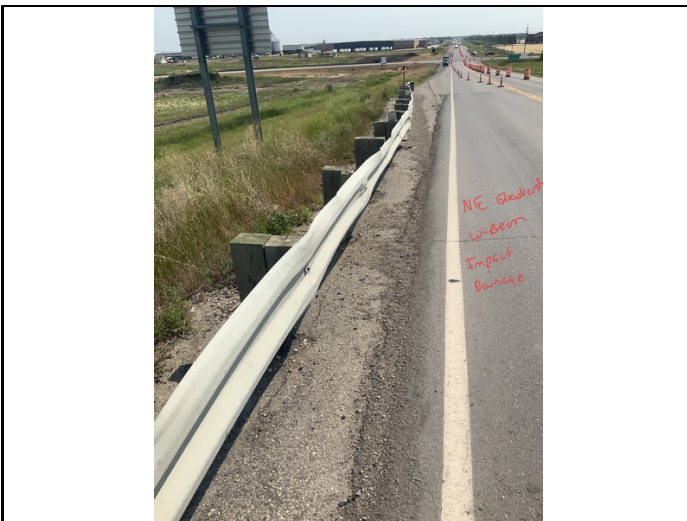
Facing East. Guardrail impact Damage to W-Beam within the NE Quadrant.
