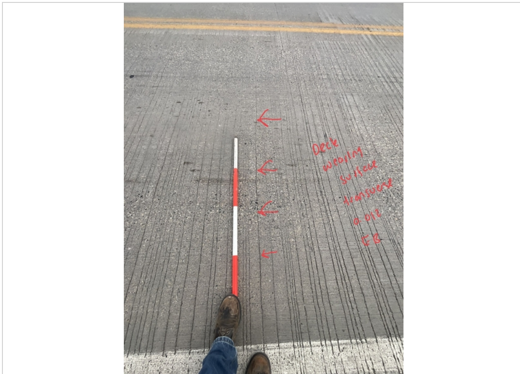
Facing North and Downward. Transverse Crack to Deck Wearing Surface EB Lane.
