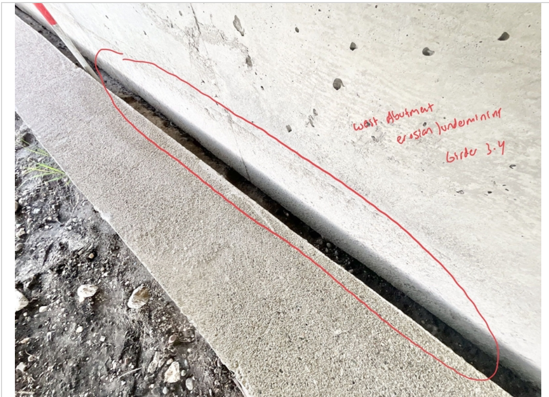
Facing SW and Downward. Area of Erosion and Undermining along Lower Portion of West Abutment from Girder 3 to 4.
