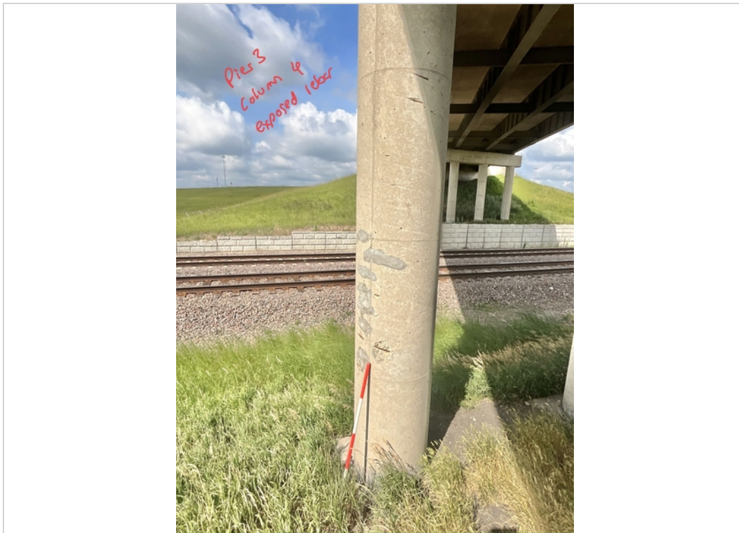
Facing West. Exposed Rebar to Pier 2 Column 4.
