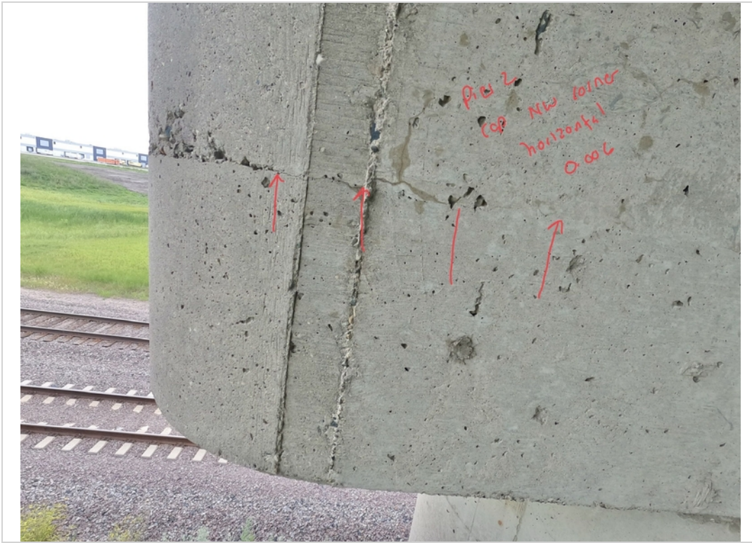
Facing East. Minor Horizontal Crack to Pier 2 Cap North of Bearing 1.
