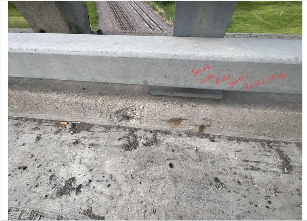
Facing South. Rust Stains to South Curb from Posts 15-16
