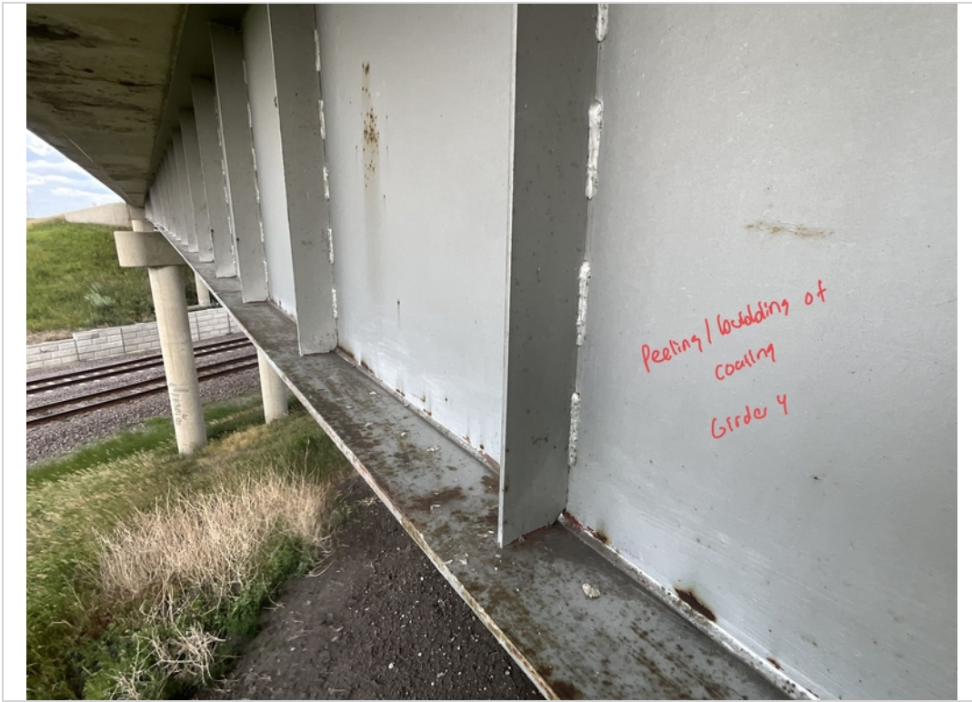
Facing SW. Peeling and Some bubbling of Coating to bottom flange of Girder 1 in Span 3.
