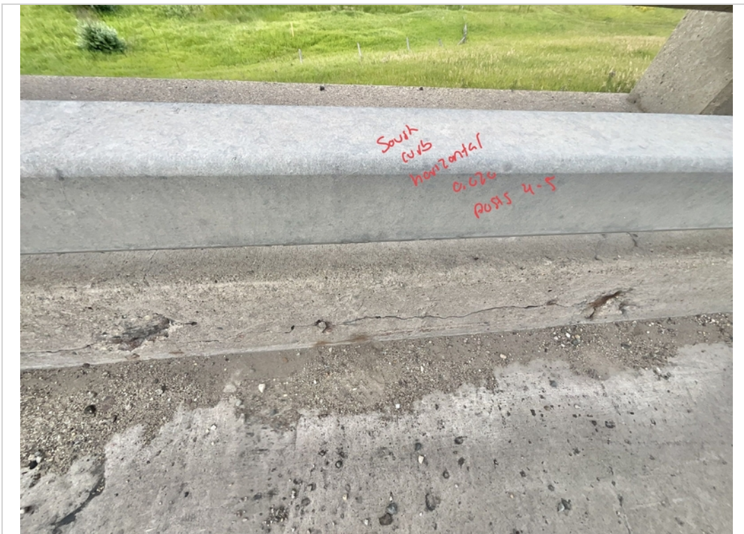
Facing South. Horizontal Crack to South Curb from Posts 4-5
