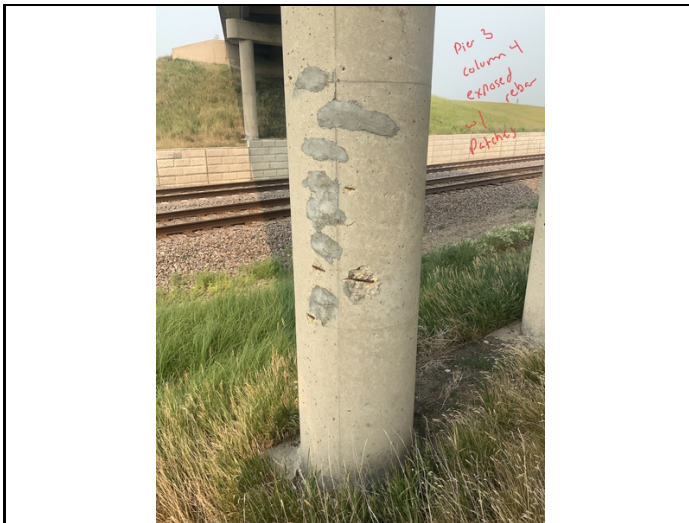
Facing NW. Exposed Rebar to Pier 3 Column 4.
