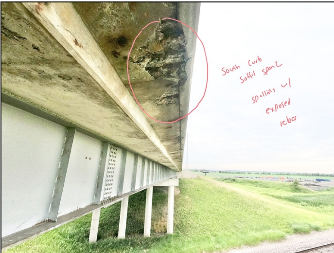
Facing East and Upwards. South Curb Soffit with Spalling and Exposed Rebar in Span 2.
