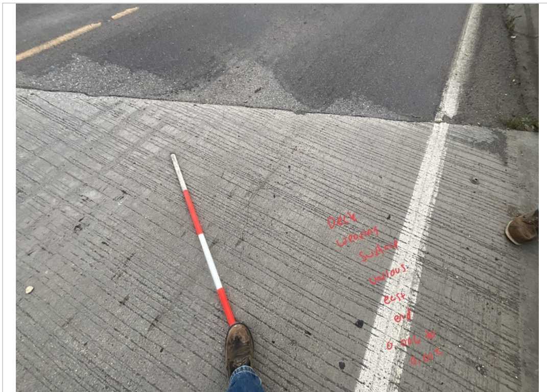
Facing East and Downward. Various Cracking to Deck Wearing Surface East End.
