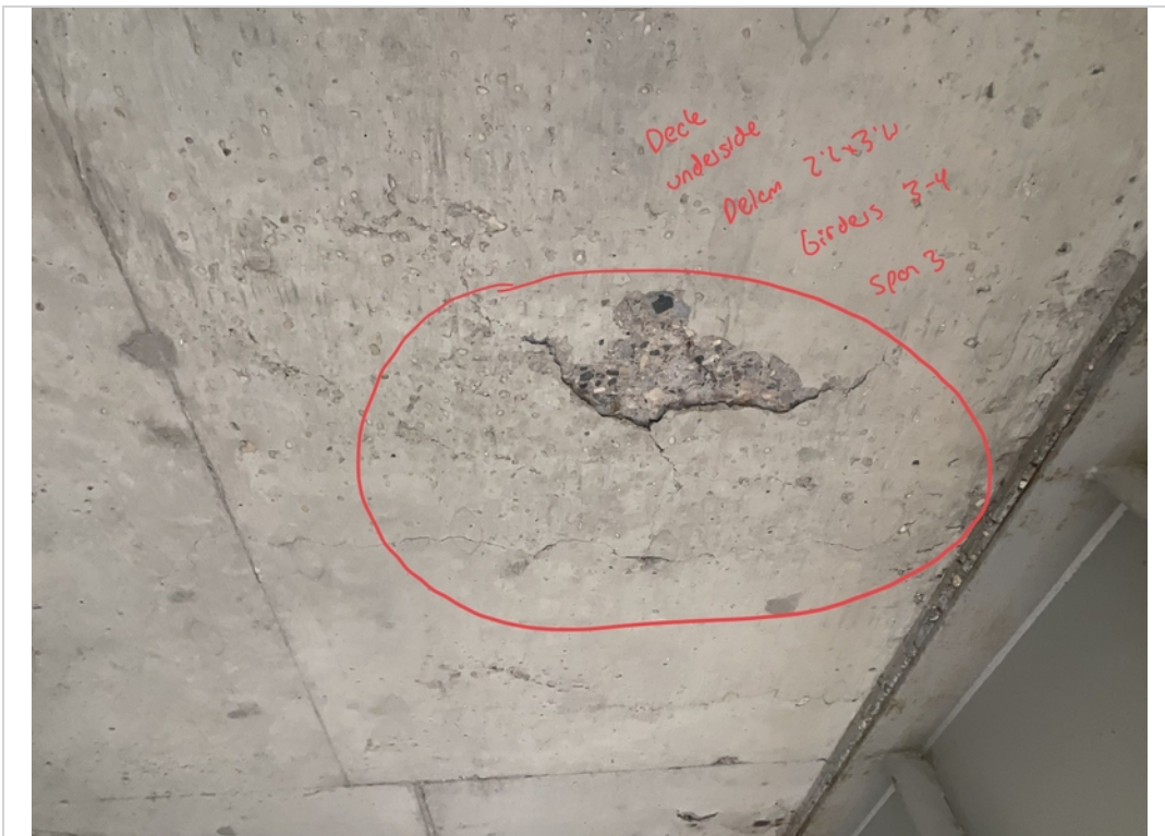
Facing East and Upwards. Underside Deck Delamination in-between Girders 3 and 4 near East End.
