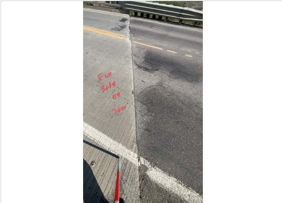
Facing North and Downward. East Bridge End Joint.
