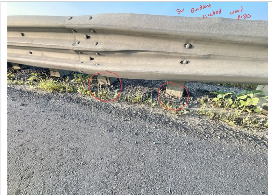
Facing South. Cracked Wood Posts within SW Guardrail Quadrant.
