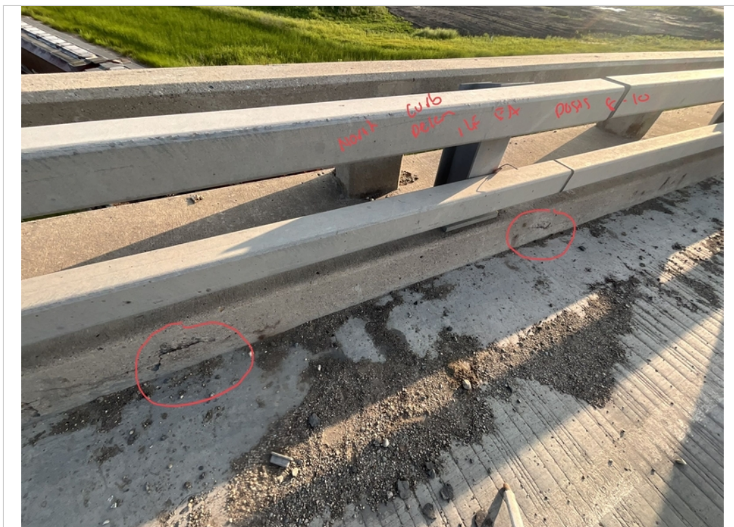
Facing NE. Delamination to North Curb from Posts 8-10.
