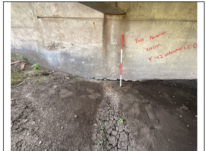
Facing East. General area of Erosion along East Embankment Slope in-between Girders 1 and 2.
