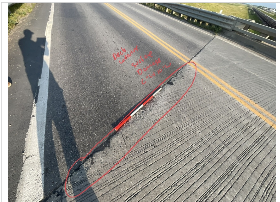
Facing NW and Downward. Blade Damage to Deck Wearing Surface EB Lane West End.
