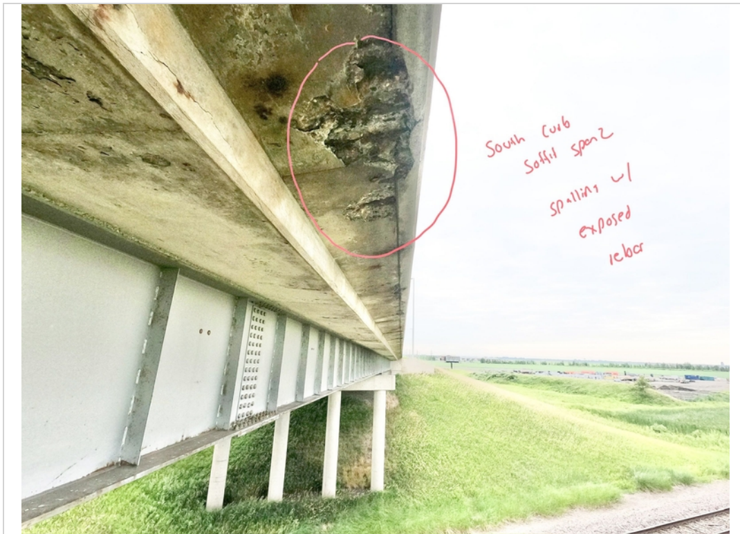
Facing East and Upwards. South Curb Soffit with Spalling and Exposed Rebar in Span 2.
