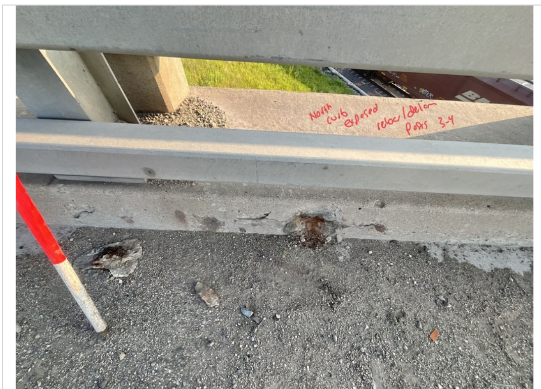
Facing North. Delamination with Exposed Rebar to North Curb in-between Posts 3 and 4.
