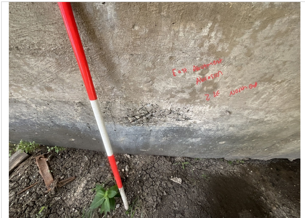
Facing East. Abrasion to East Abutment near North End.
