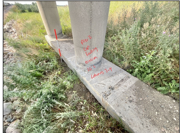
Facing SW. Erosion area along Pier 2 Cap Footing from Columns 3 to 4.
