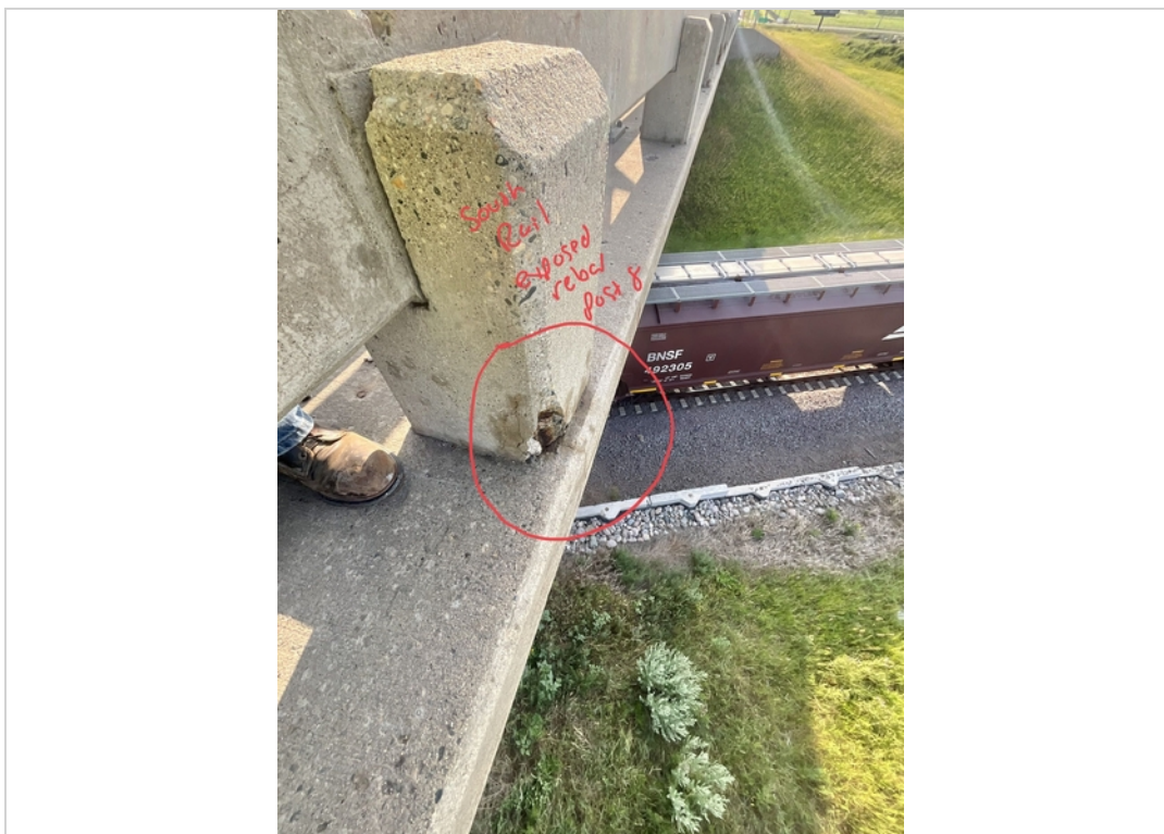
Facing NE. Exposed Rebar to South Railing Post 8.
