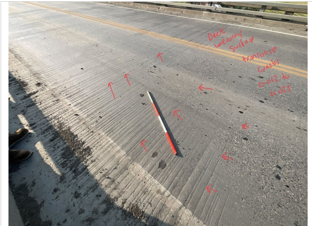
Facing SE and Downward. Transverse Cracks to Deck Wearing Surface WB Lane.
