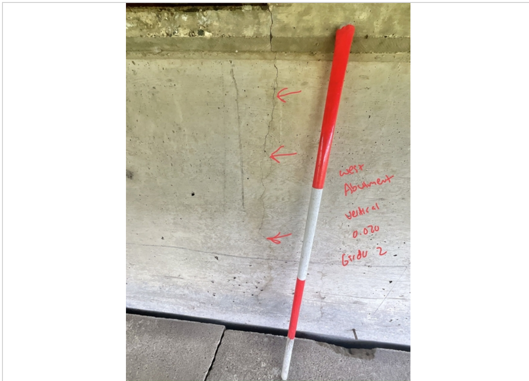
Facing West. Vertical Crack to West Abutment under Girder 2.
