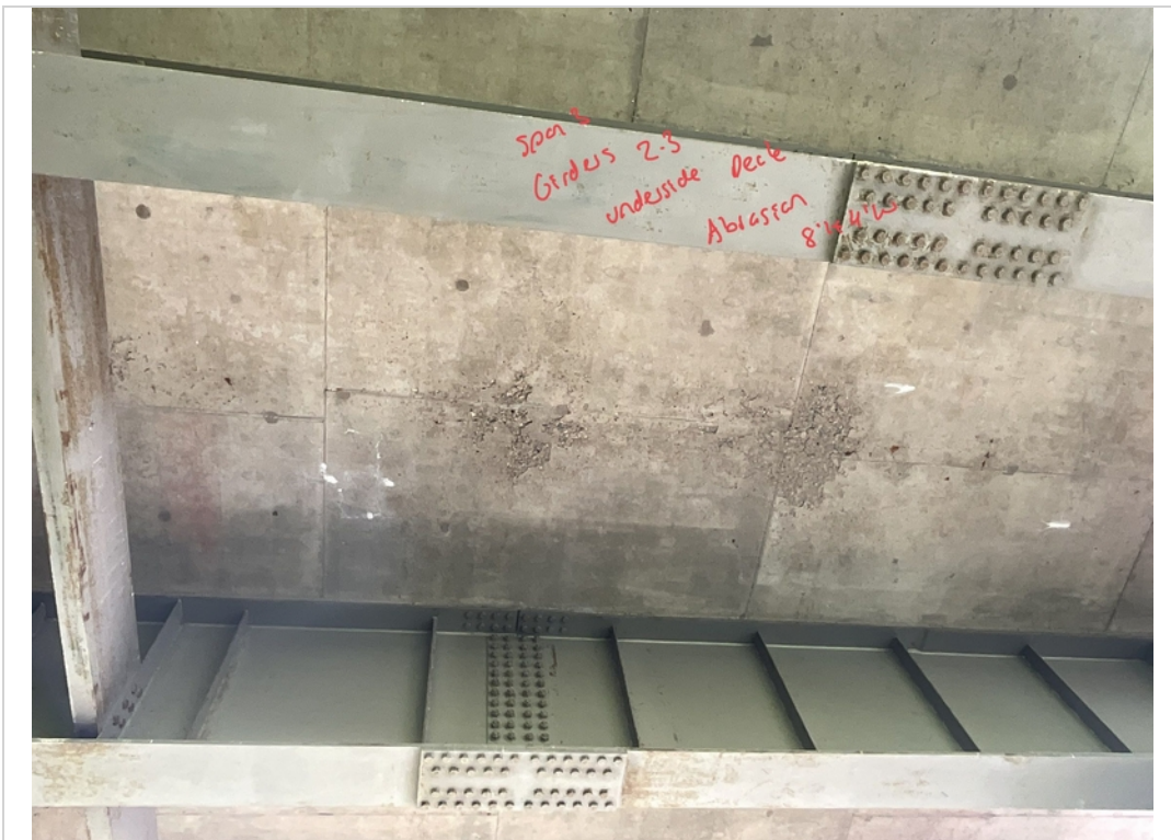
Facing South and Upwards. Abrasion to Underside Deck in Span 3 in-between Girders 2 and 3.
