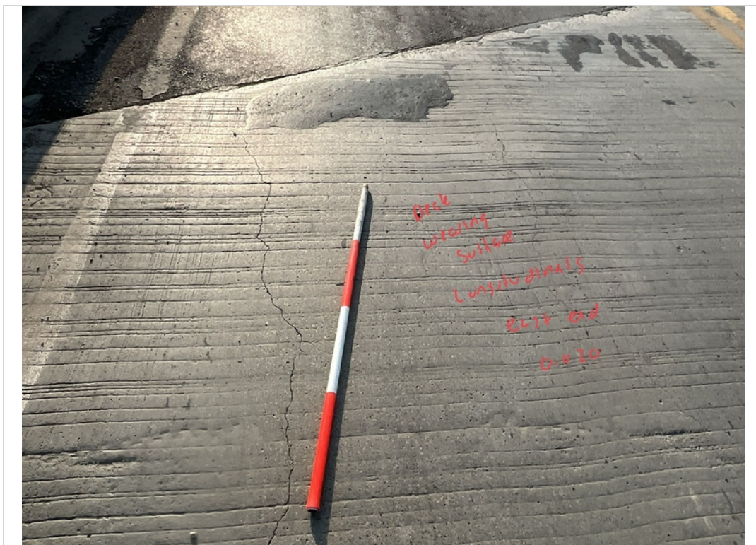
Facing East and Downward. Longitudinal Cracks to Deck Wearing Surface East End.
