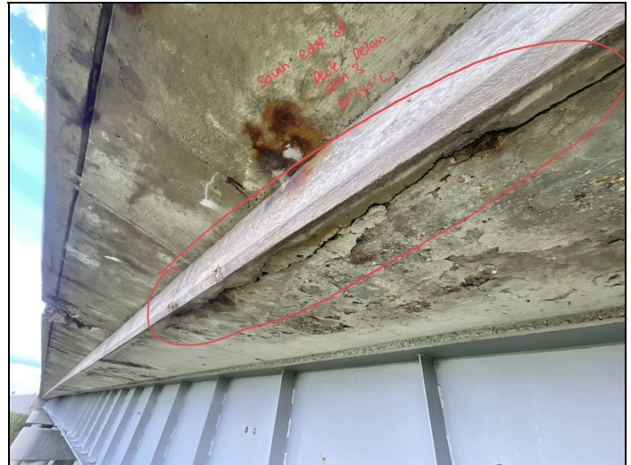
Facing NW. Moderate area of Cracking with Delamination to South Edge of Deck near East End.
