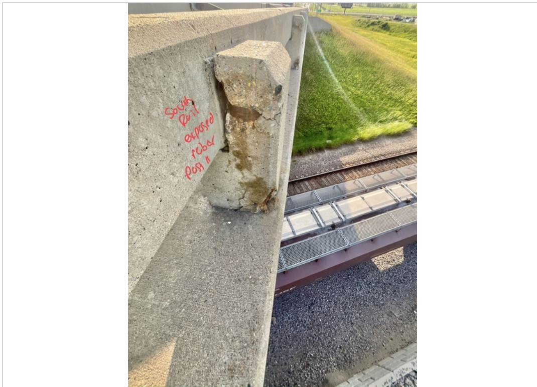
Facing East. Exposed Rebar to South Railing Post 11.
