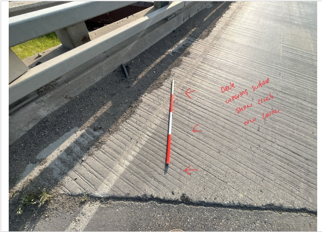
Facing East and Downward. Shear Crack to Deck Wearing Surface near NW Corner.
