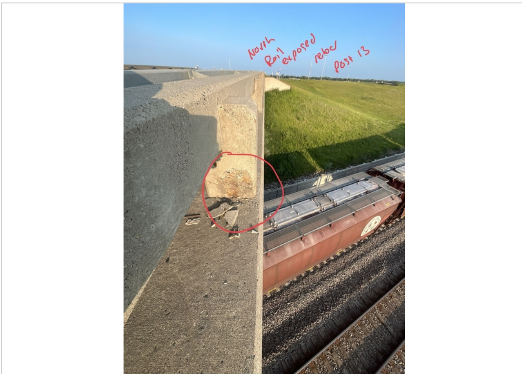
Facing West. Exposed Rebar to North Railing at Post 13.
