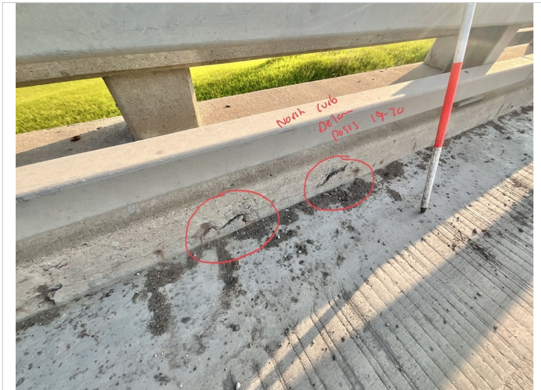
Facing NE. Delamination to North Curb in-between Posts 19-20.
