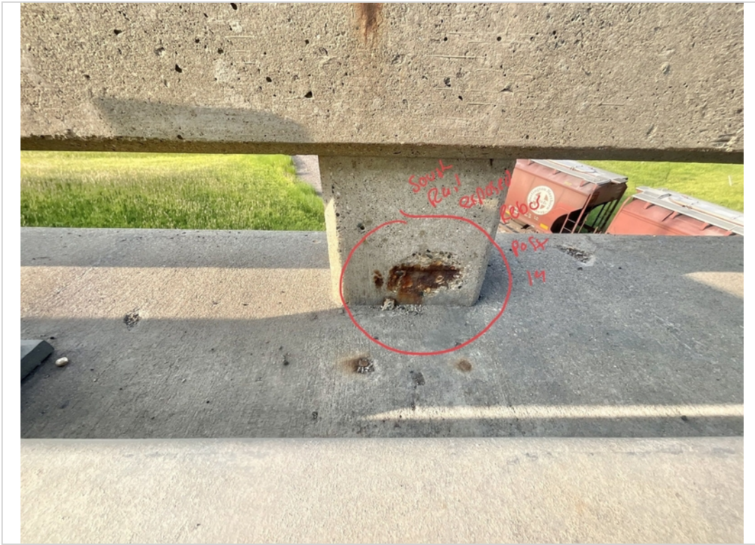
Facing South. Exposed Rear to South Railing Post 19.
