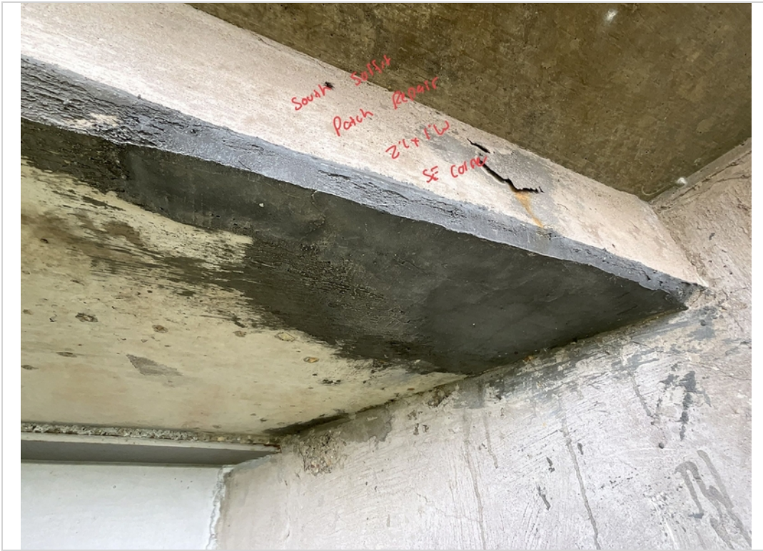
Facing NE. Patch Repair to South Soffit near SE Corner.
