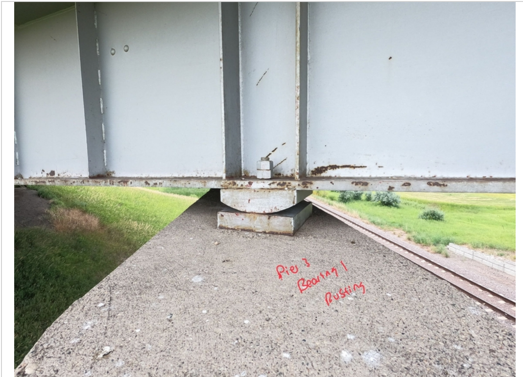
Facing South. Pier 3 Bearing 1 Rusting with Limited Effectiveness of Coating.
