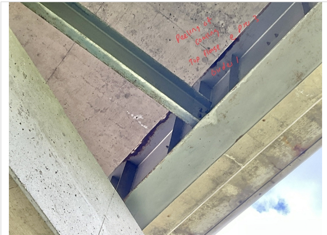
Facing NW and Upwards. Peeling of Coating down to bare metal along top flange of Girder 1 near Pier 3.
