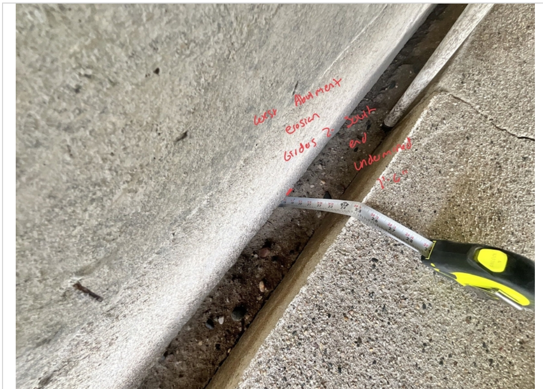
Facing NW and Downward. Erosion and Undermining Depth to West Abutment.
