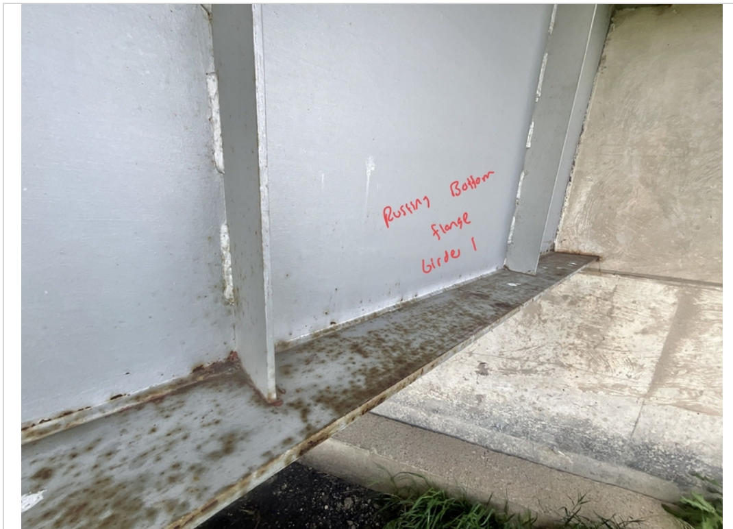
Facing SW. Freckled Rusting to Bottom Flange of Girders near West End.
