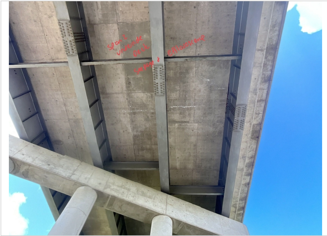
Facing West and Upwards. Underside Deck Seepage and Efflorescence in Span 2.
