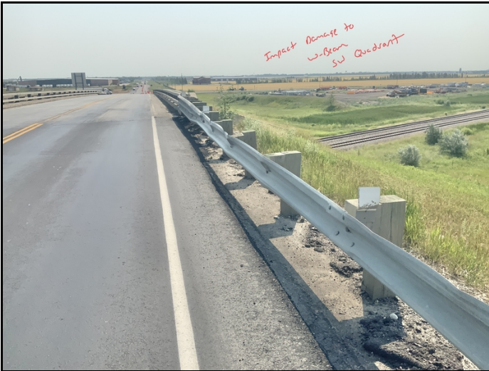
Facing East. Vehicle Impact to W-Beam within SW Quadrant.
