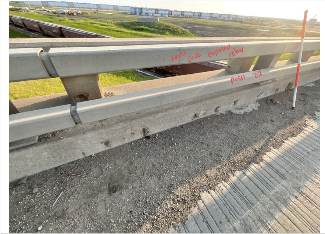
Facing NE. Exposed Rebar to North Curb from Posts 2 and 3.
