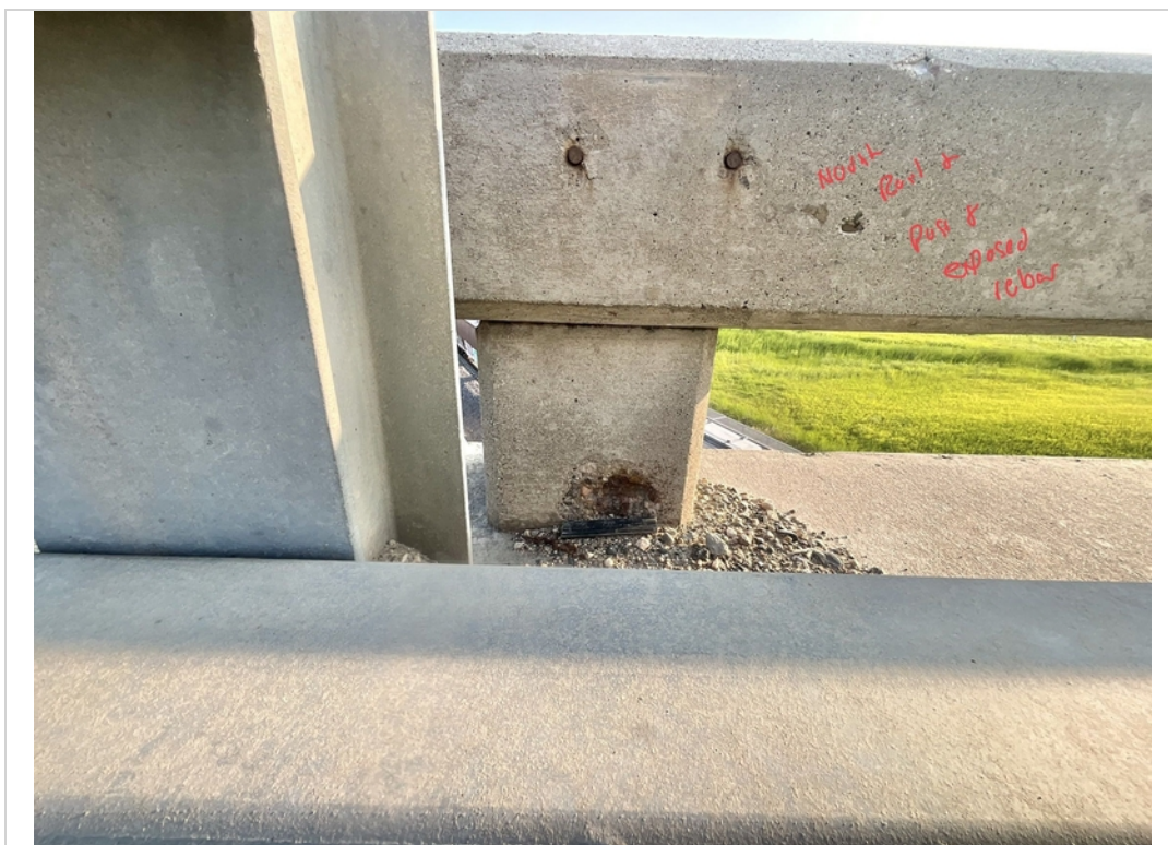
Facing North. Exposed Rebar to North Railing Post 8.
