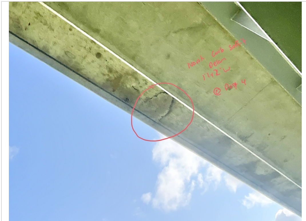
Facing NW and Upwards. Delamination to North curb Soffit in Span 1.
