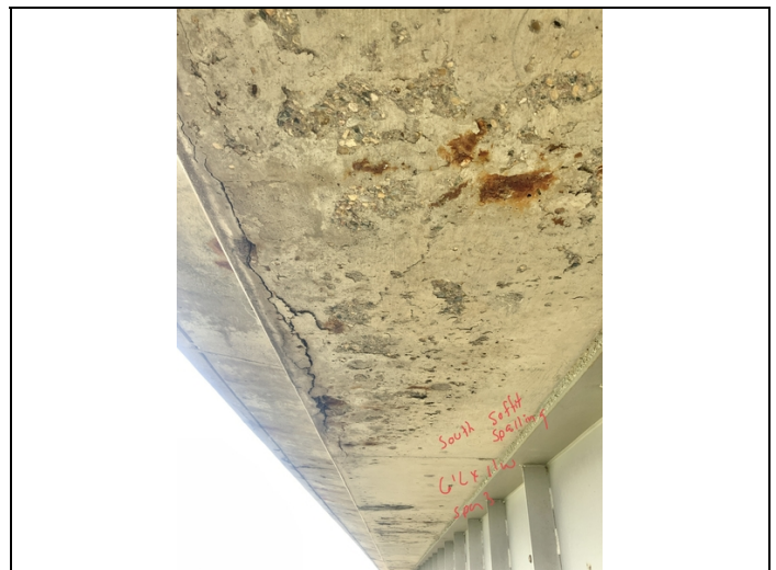
Facing West. Areas of Spalling along South Edge of Deck in span 3.
