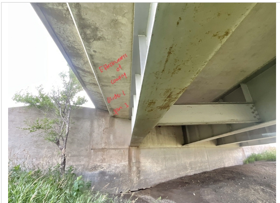
Facing East. Effectiveness of Coating to underside Girder 1 in Span 3.
