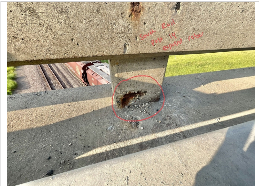
Facing South. Exposed Rebar to South Railing Post 14.
