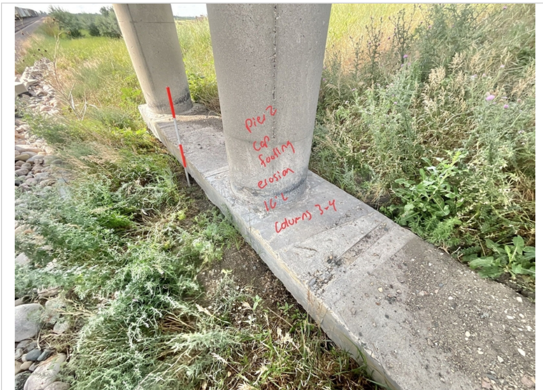
Facing SW. Erosion area along Pier 2 Cap Footing from Columns 3 to 4.
