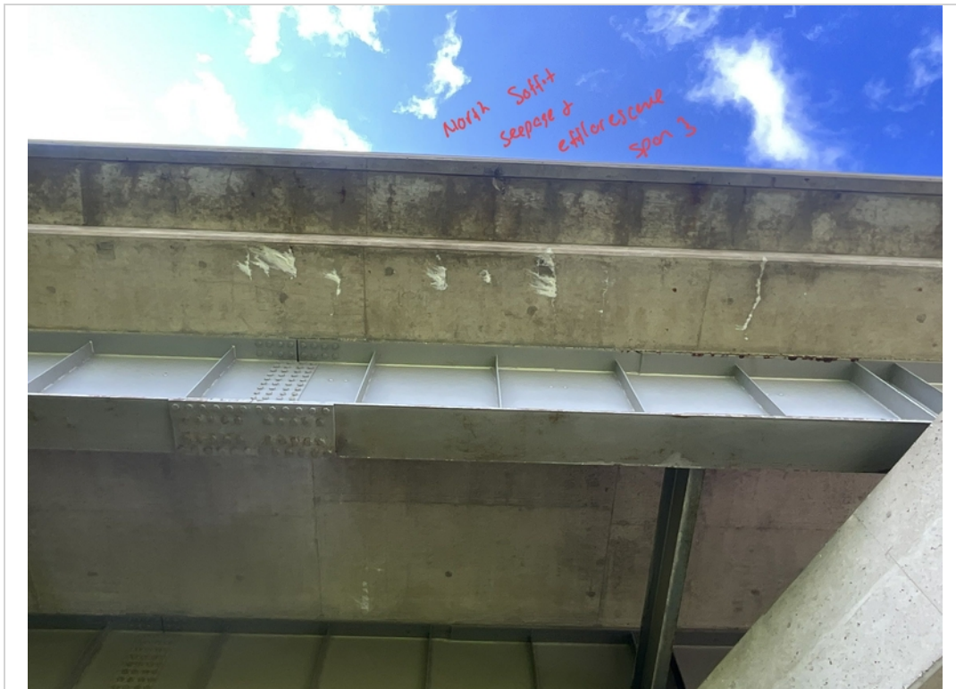
Facing South and Upwards. North Deck Soffit with Seepage and Efflorescence in Span 3.
