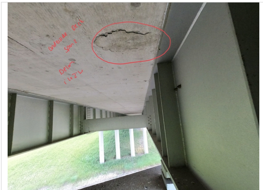
Facing East and Downward. Delamination to Underside Deck Span 1
