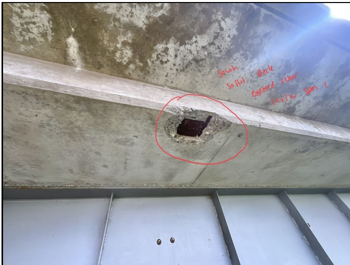
Facing South and Upwards. Exposed Rebar to South Deck Soffit in Span 1.
