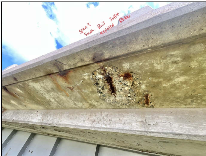
Facing NW and Upwards. South Curb Soffit Exposed Rebar in Span 3.
