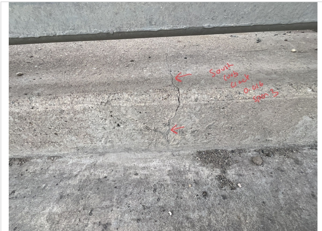
Facing South. Crack to South Curb in Span 3.
