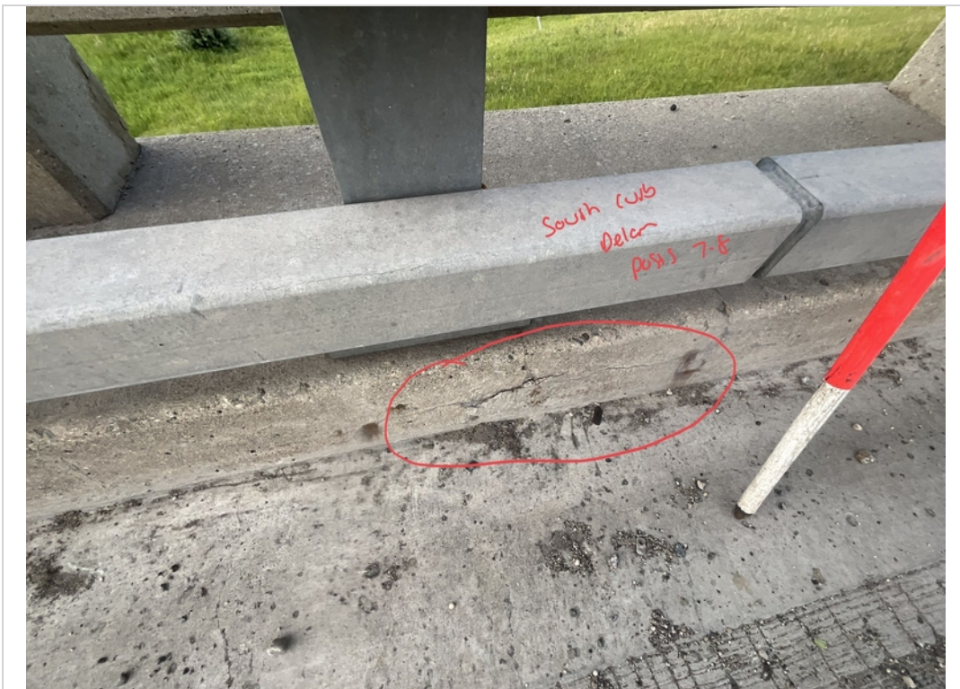
Facing South. Delamination to South Curb Posts 7 and 8.
