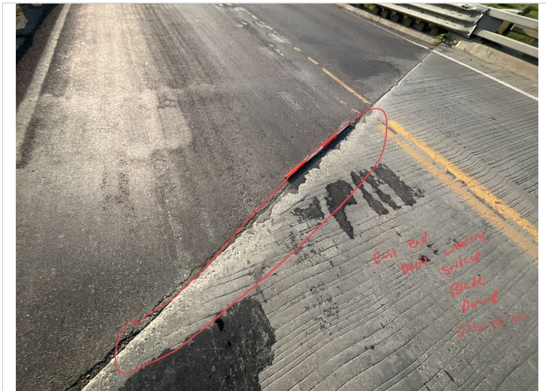
Facing SE and Downward. Blade Damage to Deck Wearing Surface East End WB Lane.
