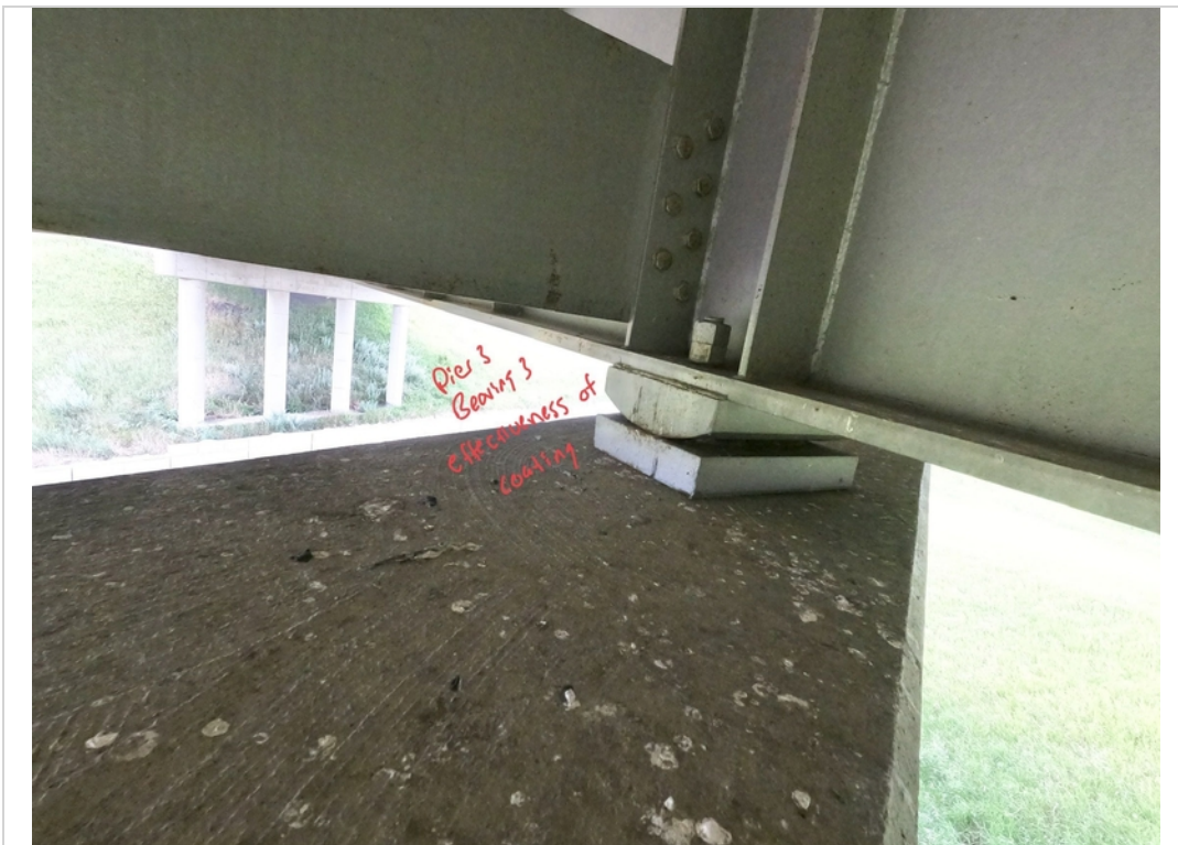
Facing NW. Effectiveness of Coating to Pier 3 Bearing 3.
