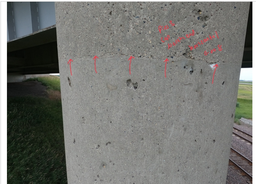
Facing South. Horizontal Crack to North End of Pier 3 Cap.
