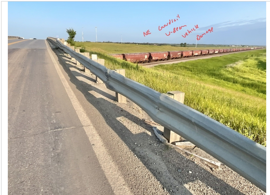
Facing West. Vehicle Impact to W-beam in NE Quadrant.
