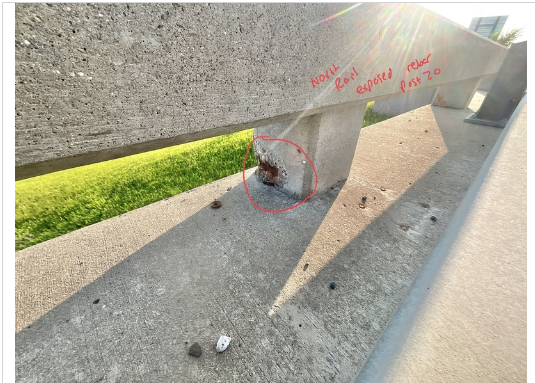
Facing NE. Exposed Rebar to North Railing Post 20.
