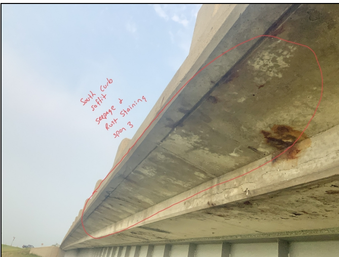
Facing West. Areas of Seepage and Rusting staining to underside South Curb in Span 3.
