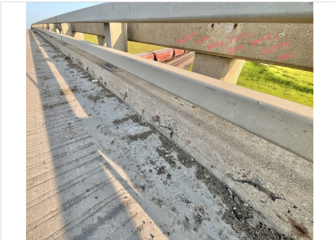
Facing SW. Cracking with Rust Staining to North Curb from Posts 17-20.
