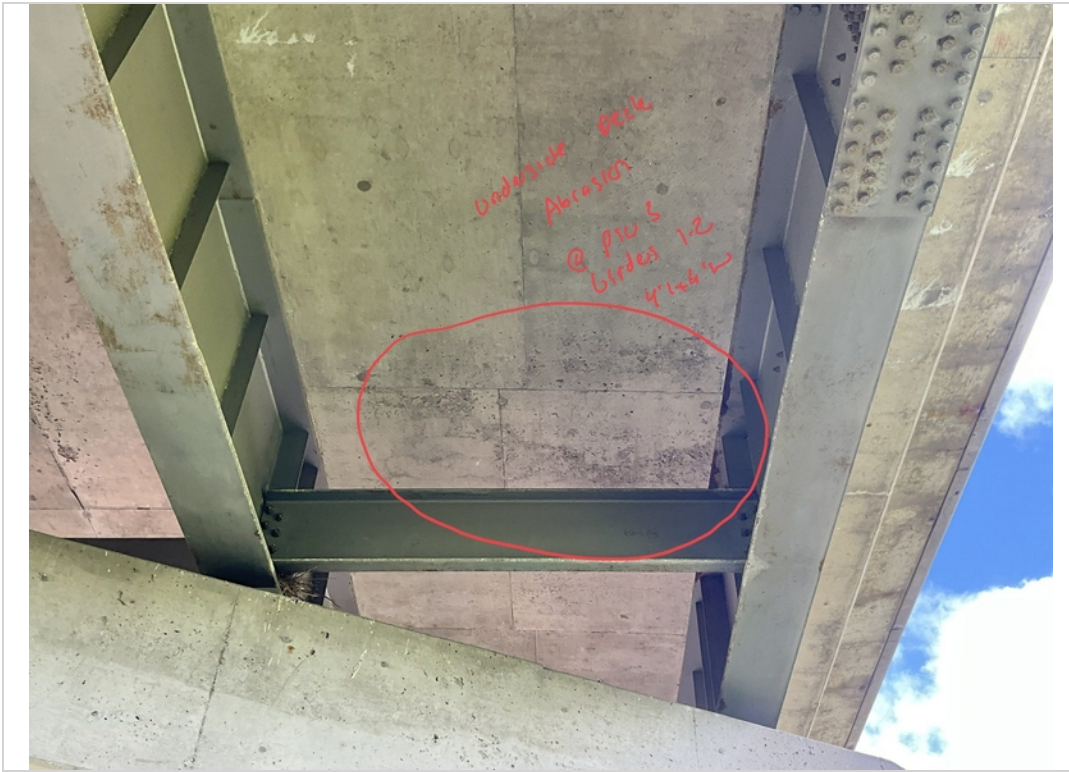
Facing West and Upwards. Abrasion with some honeycombing to underside of deck near Pier 3.
