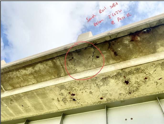
Facing NW and Upwards. Delamination to South Railing Soffit at Post 22.
