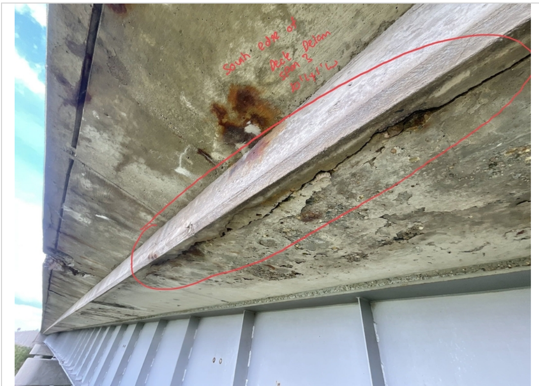
Facing NW. Moderate area of Cracking with Delamination to South Edge of Deck near East End.
