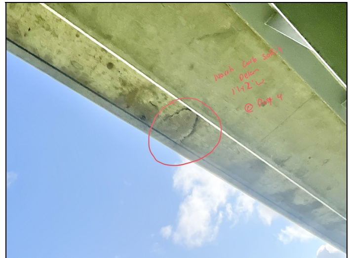
Facing NW and Upwards. Delamination to North curb Soffit in Span 1.
