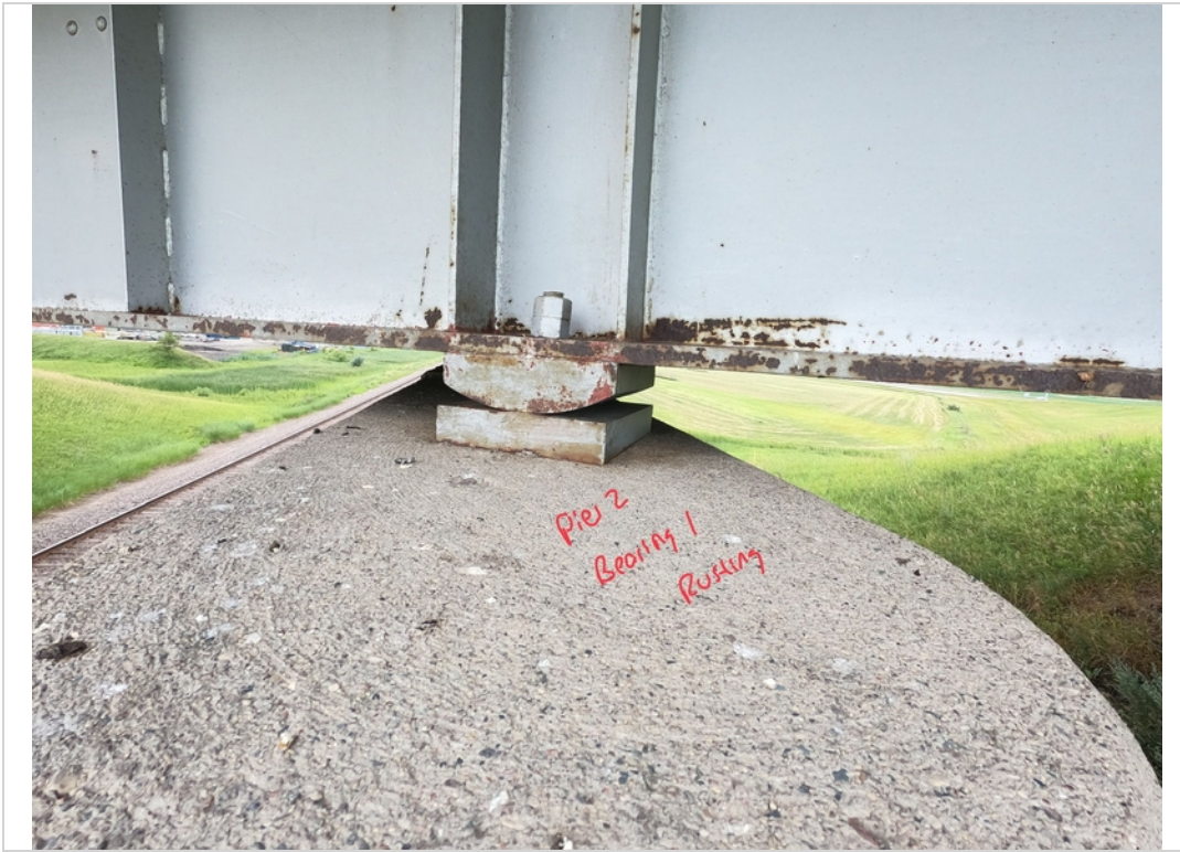
Facing South. Rusting to Pier 2 Bearing 1.
