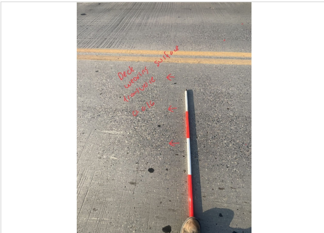
Facing South and Downward. Transverse Crack to Deck Wearing Surface WB Lane.
