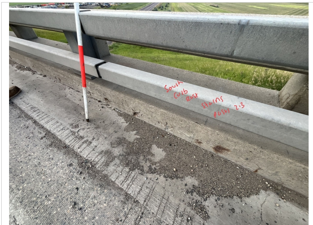
Facing South. Rust Stains to South Curb from Posts 2-3
