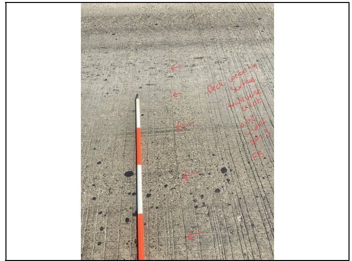
Facing North and Downward. Transverse crack to Deck Wearing Surface in Span 3 of the EB Lane.
