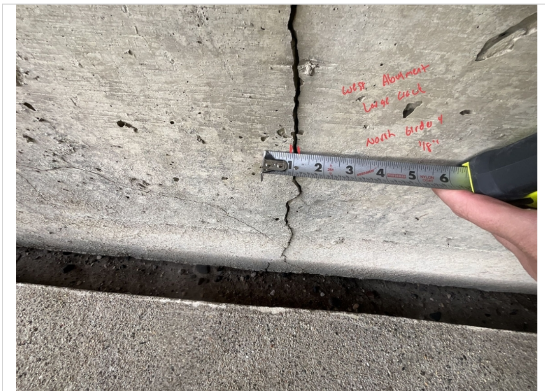
Facing West and Downward. Large Vertical Crack Opening to West Abutment.
