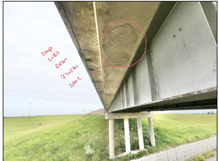
Facing West. Delamination to South Soffit in Span 2.
