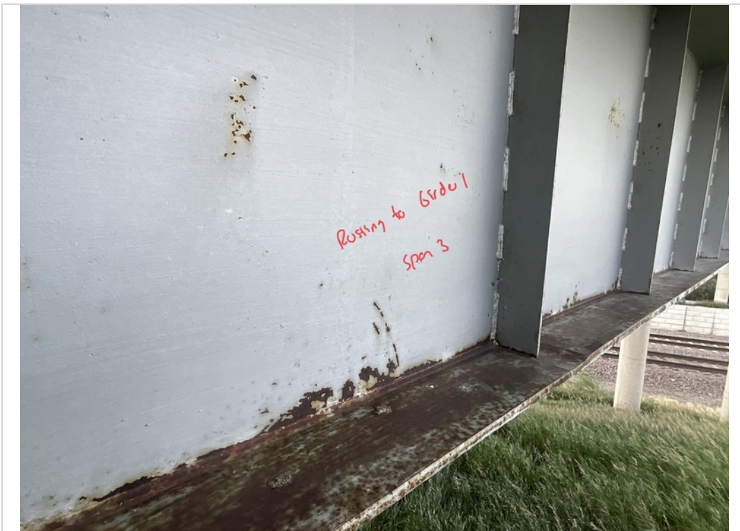
Facing SW. Rusting to Bottom flange to Girder 1 in Span 3.
