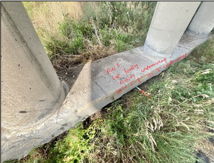
Facing NW and Downward. Continued Erosion and Undermining to Pier 2 Cap Footing in-between Columns 3 and 4.
