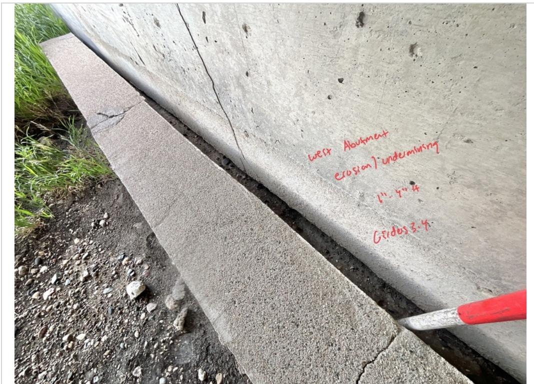
Facing SW and Downward. Continued Erosion along West Abutment from Girders 3 to 4.
