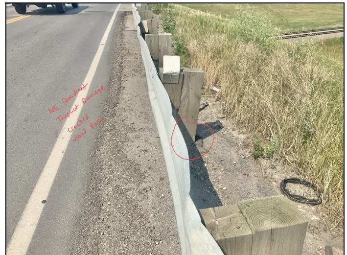
Facing West. Vehicle Impact Damage with cracked wood post within NE Quadrant.
