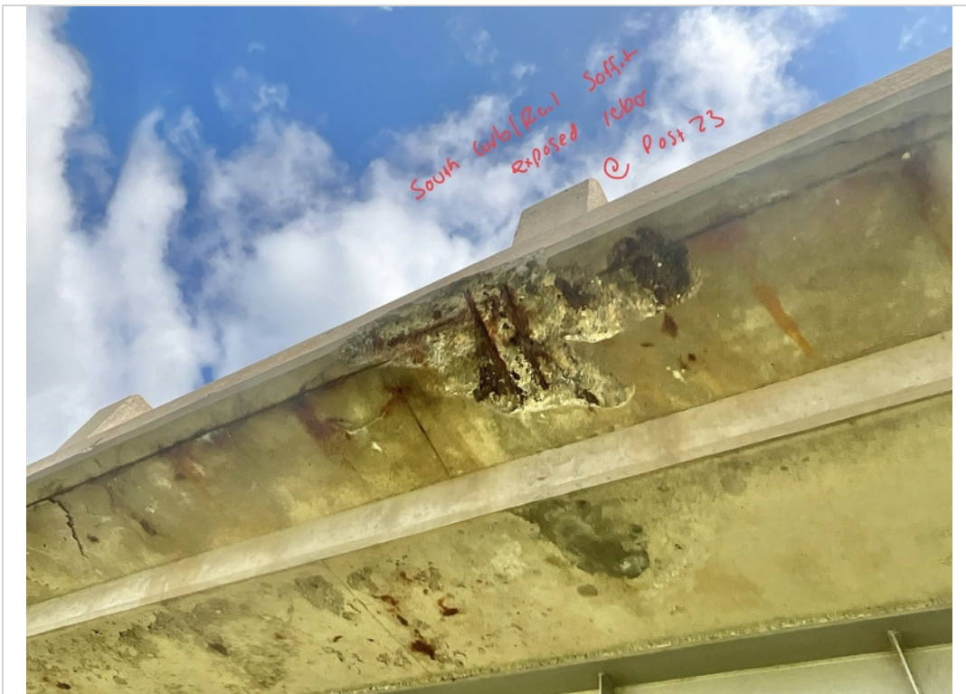
Facing NW and Upwards. Spalling with Exposed Rebar to South Railing at Post 23.
