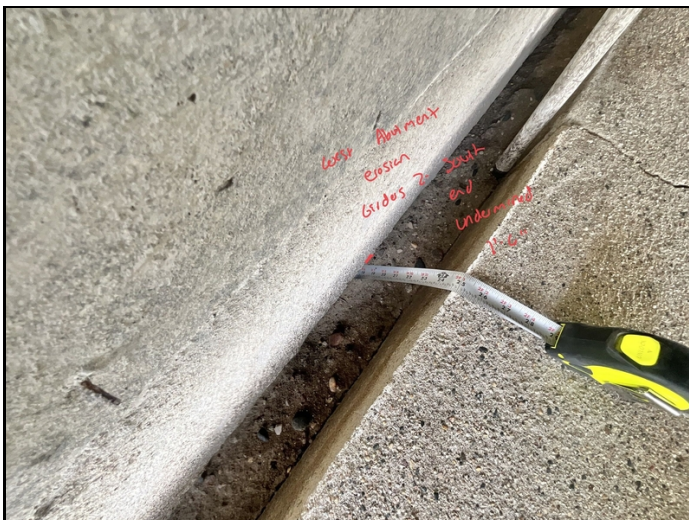
Facing NW and Downward. Erosion and Undermining Depth to West Abutment.
