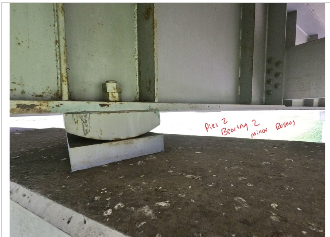
Facing NE. Pier 2 Bearing 2 Minor Rusting.
