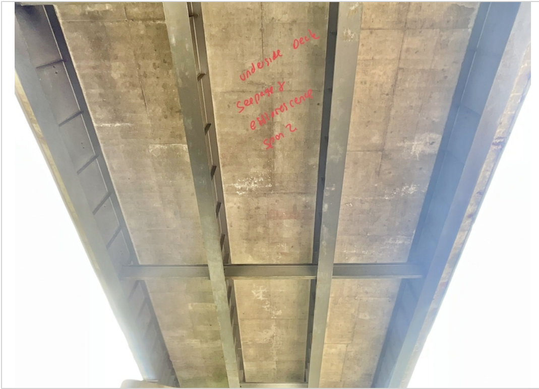
Facing East and Upwards. Underside Deck Seepage and Efflorescence in Span 2.
