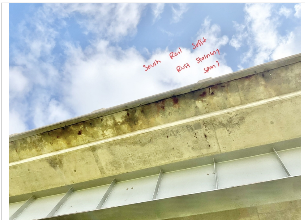
Facing North and Upwards. Rust Staining to South Curb Soffit in Span 1.
