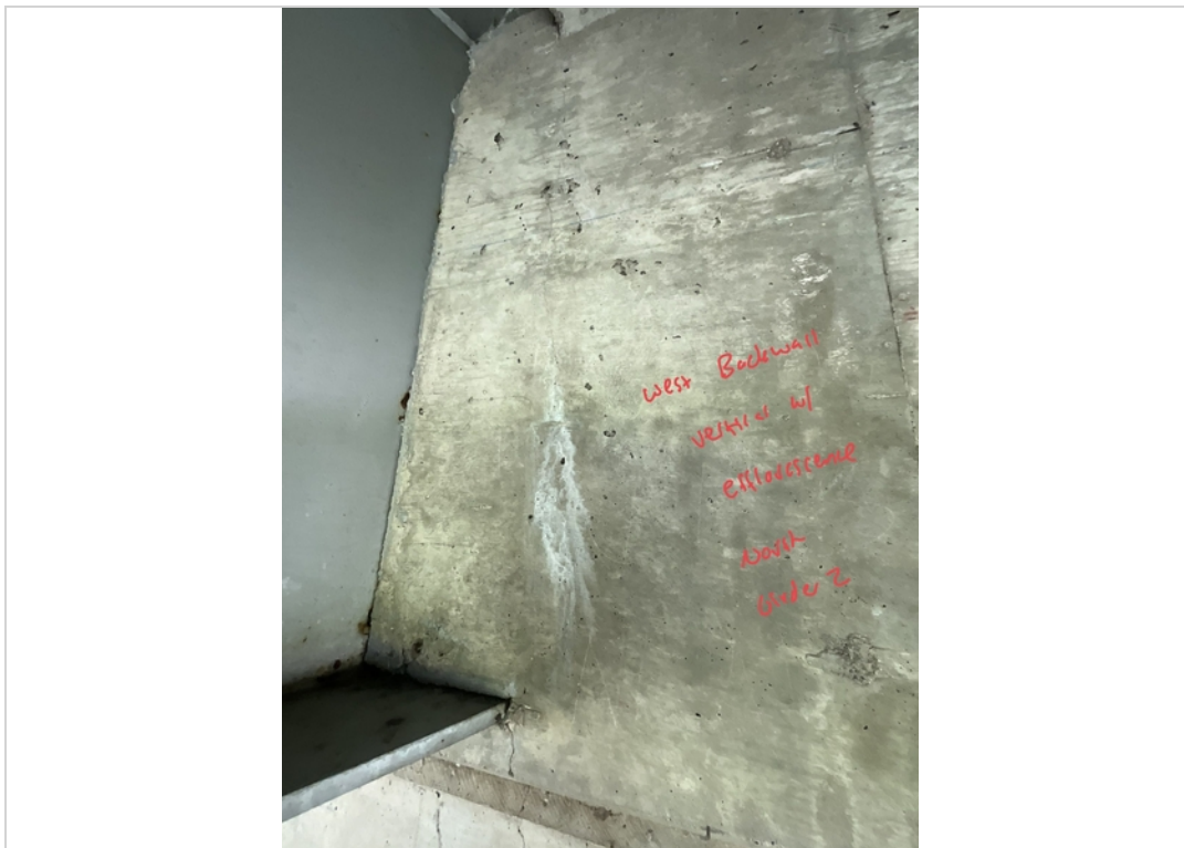
Facing SW. Vertical Crack with some seepage and efflorescence to West Backwall North of Girder 2.
