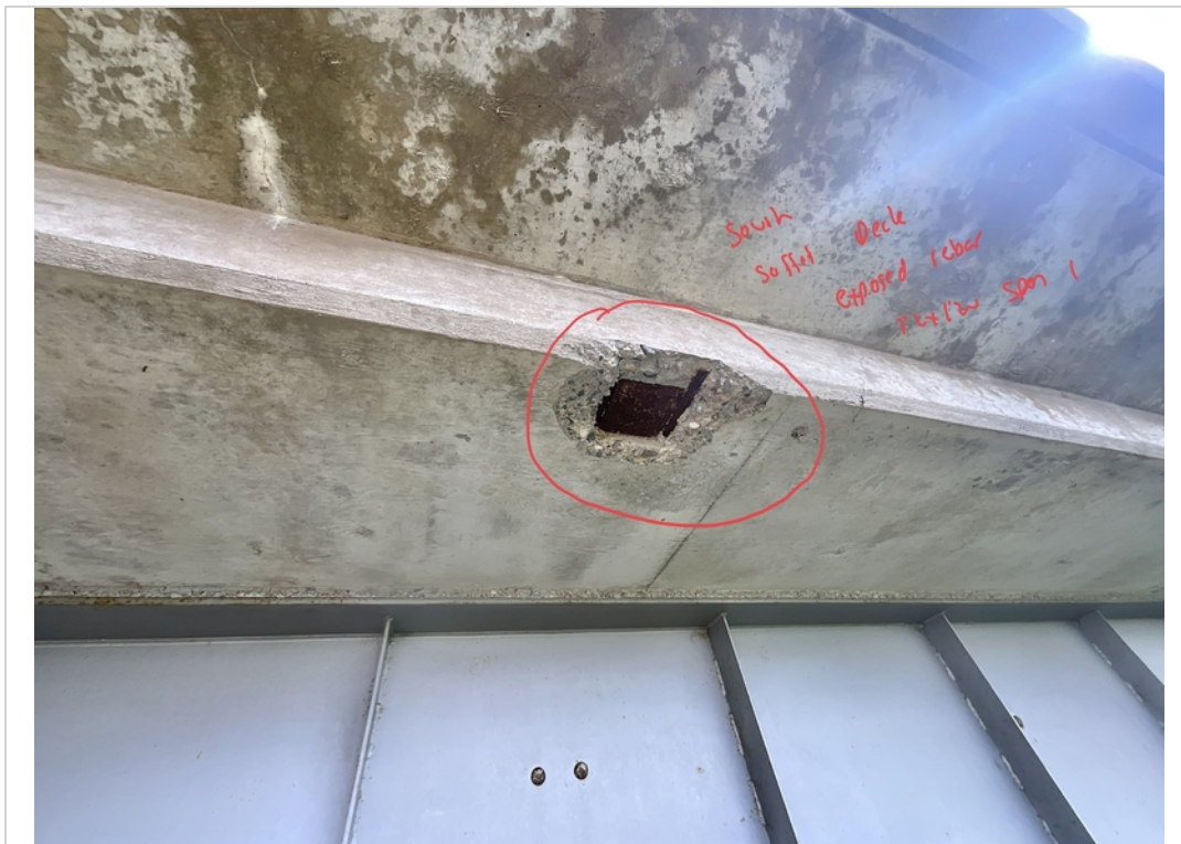
Facing South and Upwards. Exposed Rebar to South Deck Soffit in Span 1.
