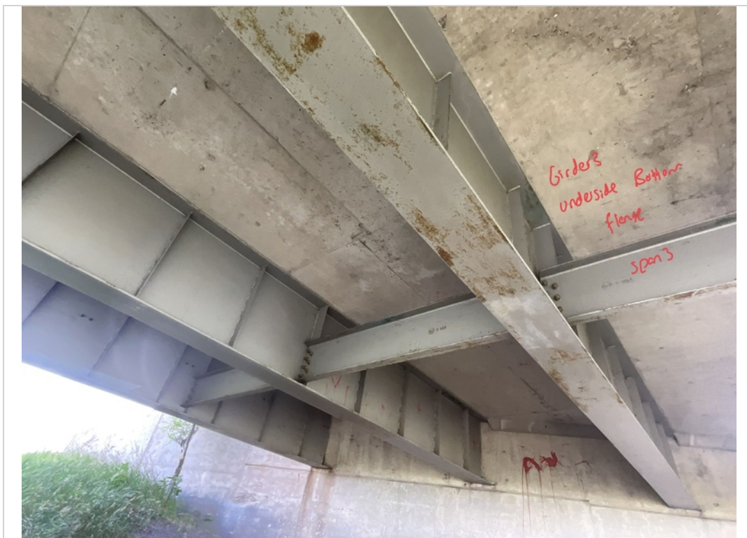
Facing NE and Upwards. Rusting to underside bottom flanges of Girders in Span 3.
