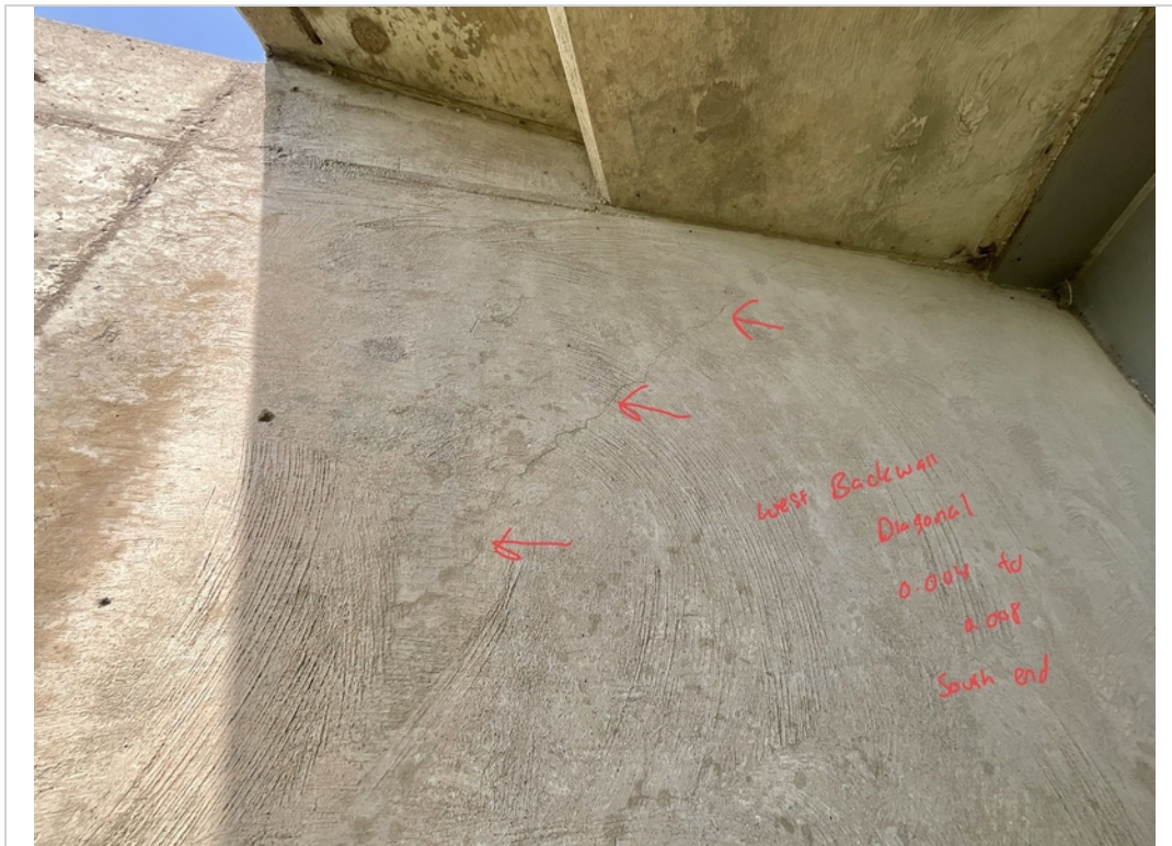
Facing West and Upwards. Diagonal Crack to West Backwall South End.
