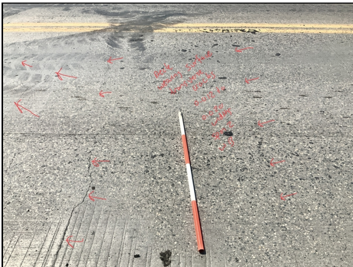
Facing South and Downward. Transverse cracking to Deck Wearing Surface in the WB Lane of Span 2.
