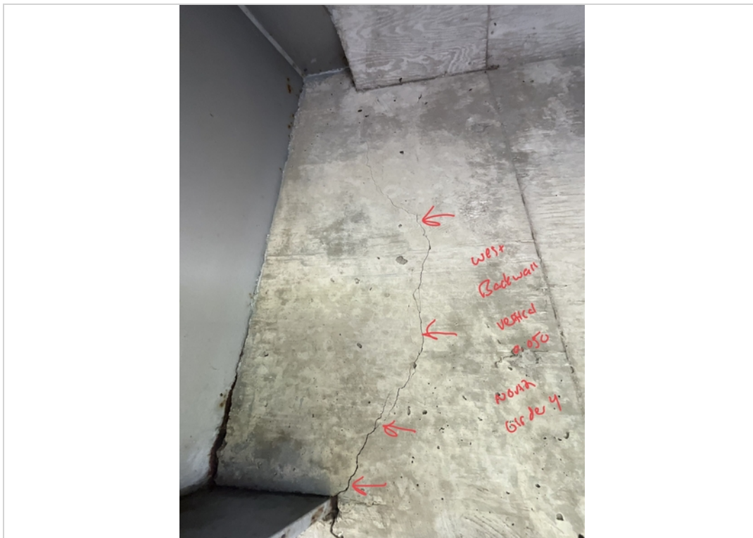
Facing West. Vertical Crack to West Backwall North of Girder 1.
