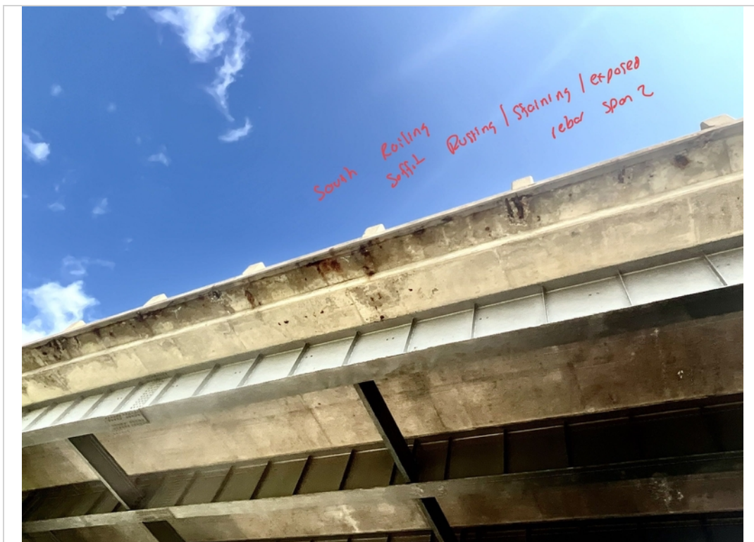
Facing North and Upwards. South Curb Soffit with Rust Staining in Span 2.
