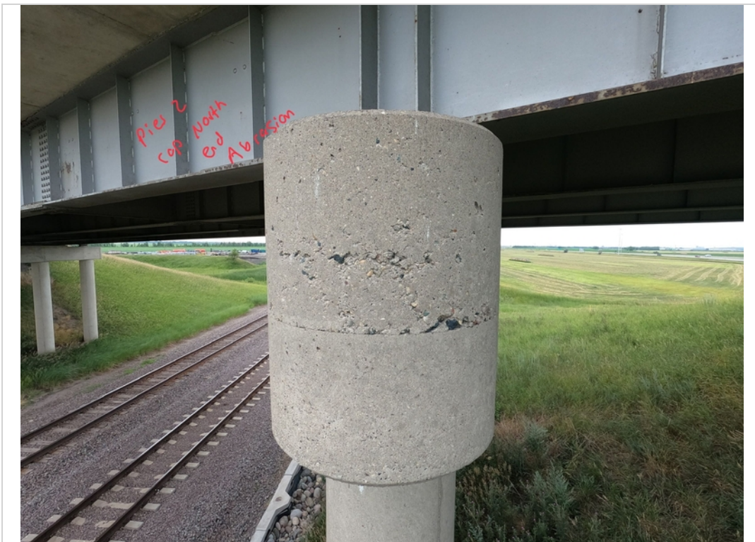
Facing South. Abrasion to Pier 2 Cap North End.
