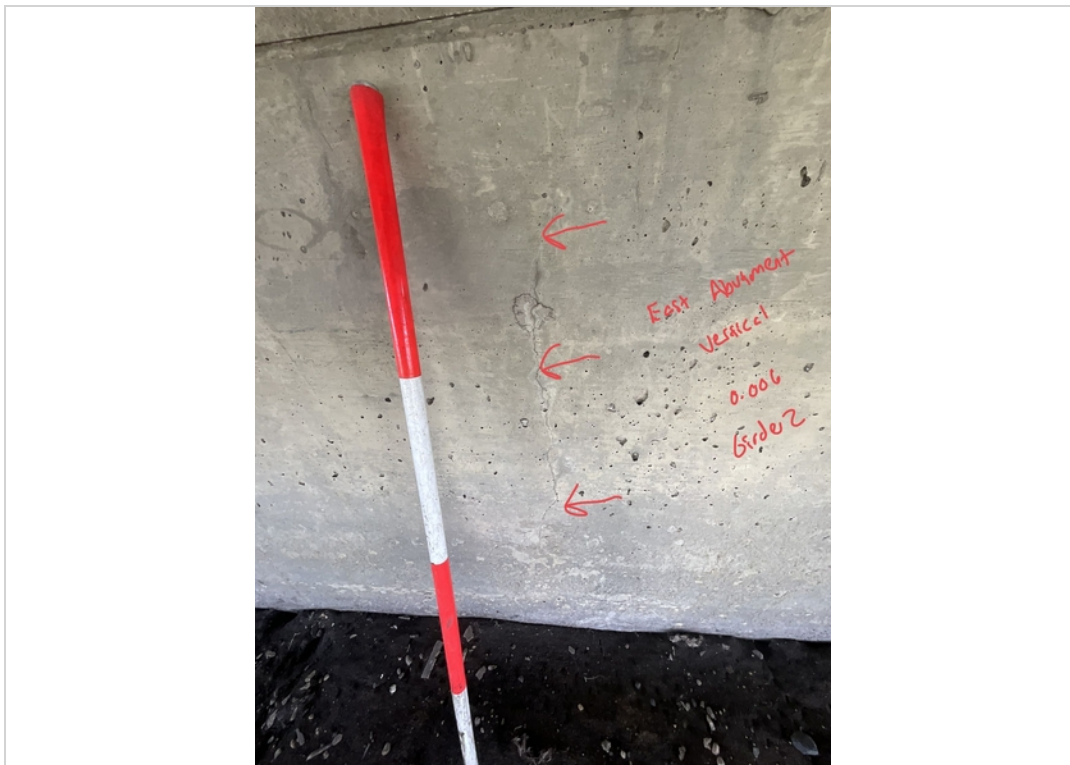
Facing East. Vertical Crack to East Abutment under Girder 2.
