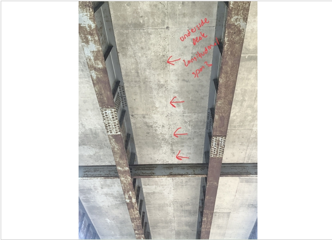
Facing East and Upwards. Longitudinal Crack to Underside Deck in Span 3 along CL.
