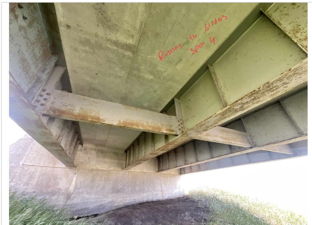
Facing SE. Rusting to Girders in Span 4.
