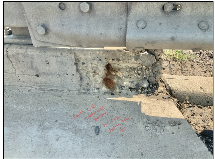
Facing South. Moderate Spalling to South Curb at SW Corner.
