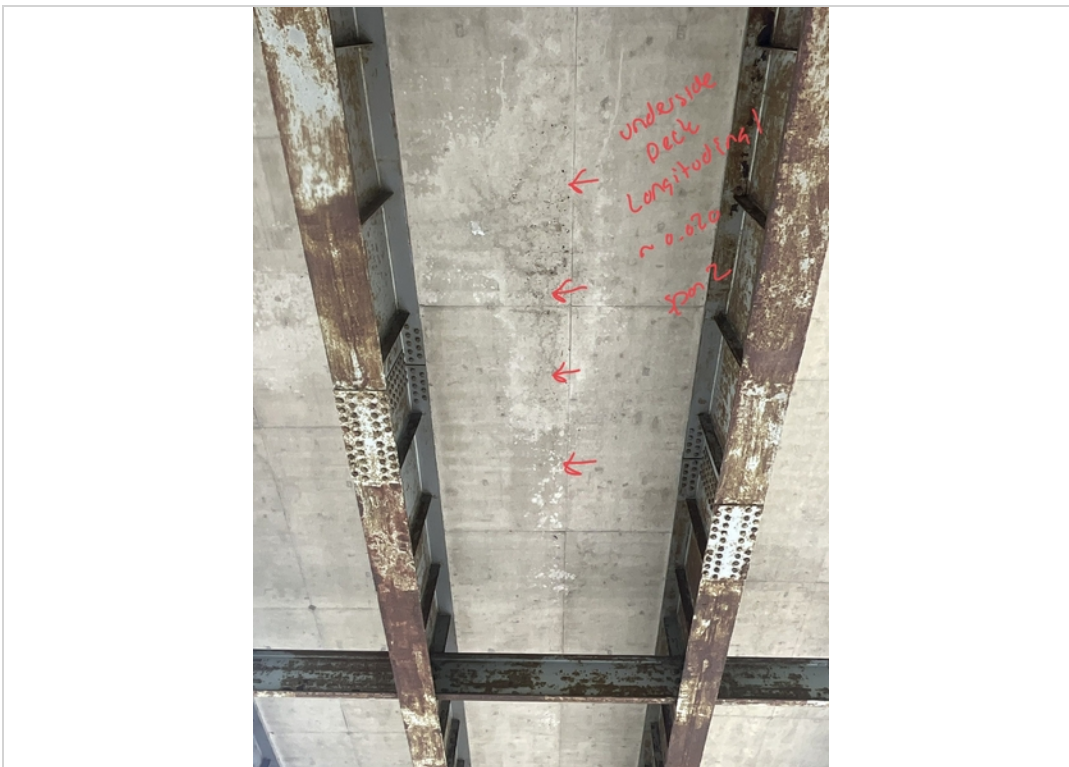
Facing East and Upwards. Longitudinal Crack to Underside Deck CL in Span 2.
