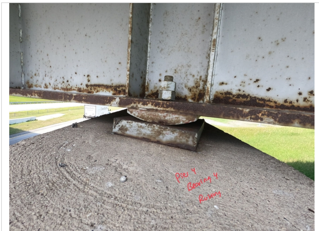
Facing North. Pier 4 Bearing 4 Rusting.
