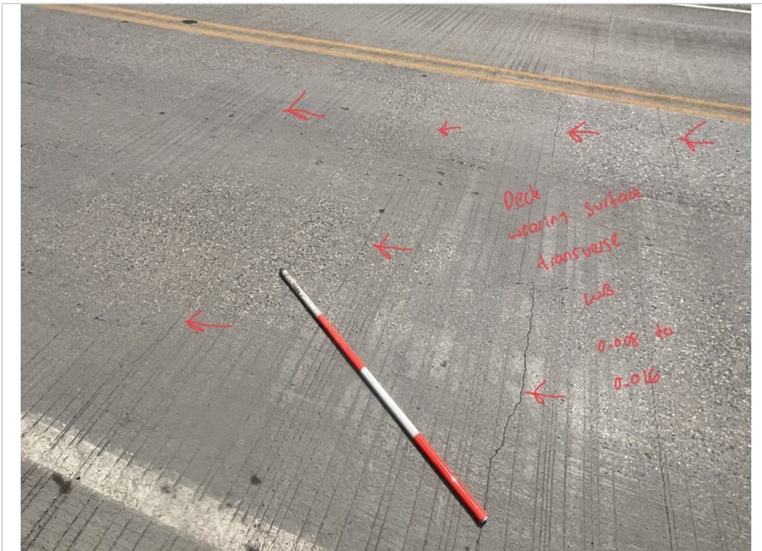
Facing South and Downward. Patterned Transverse Cracking to Deck Wearing Surface WB Lane.
