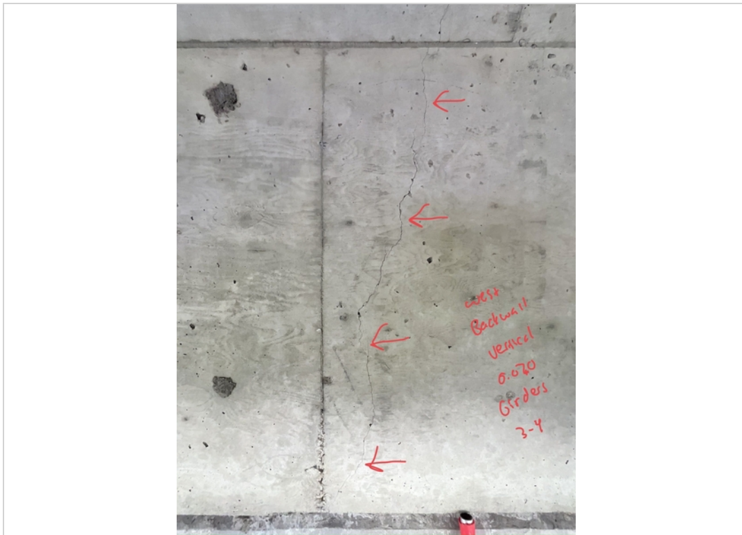
Facing West. Vertical Crack to West Backwall in-between Girders 3 and 4.
