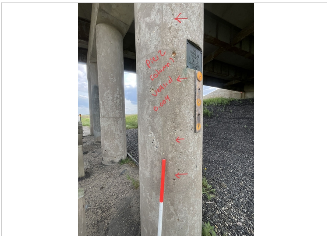
Facing SW. Minor Vertical Crack to Pier 2 Column 1.
