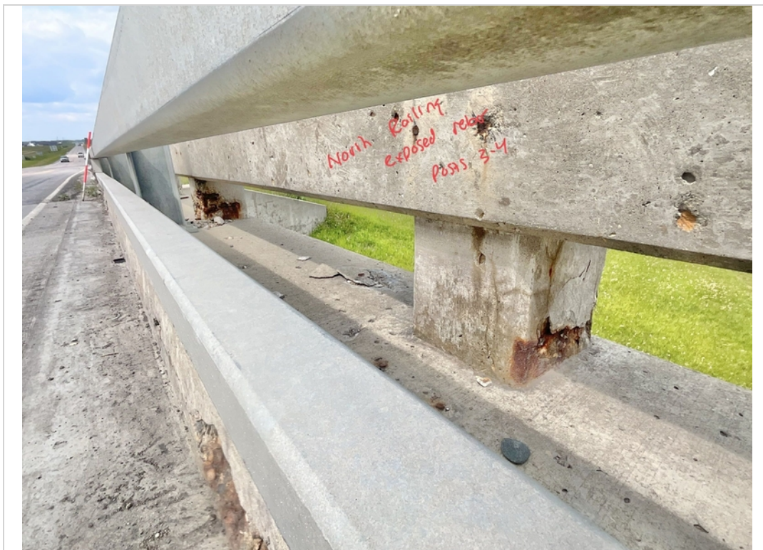
Facing NW. Exposed Rebar to North Railing Posts 3 and 4.
