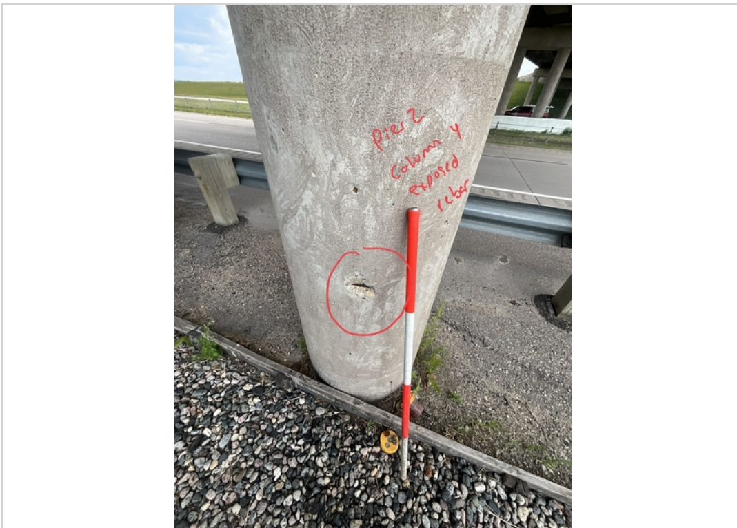
Facing NE. Pier 2 Column 4 Exposed Rebar.
