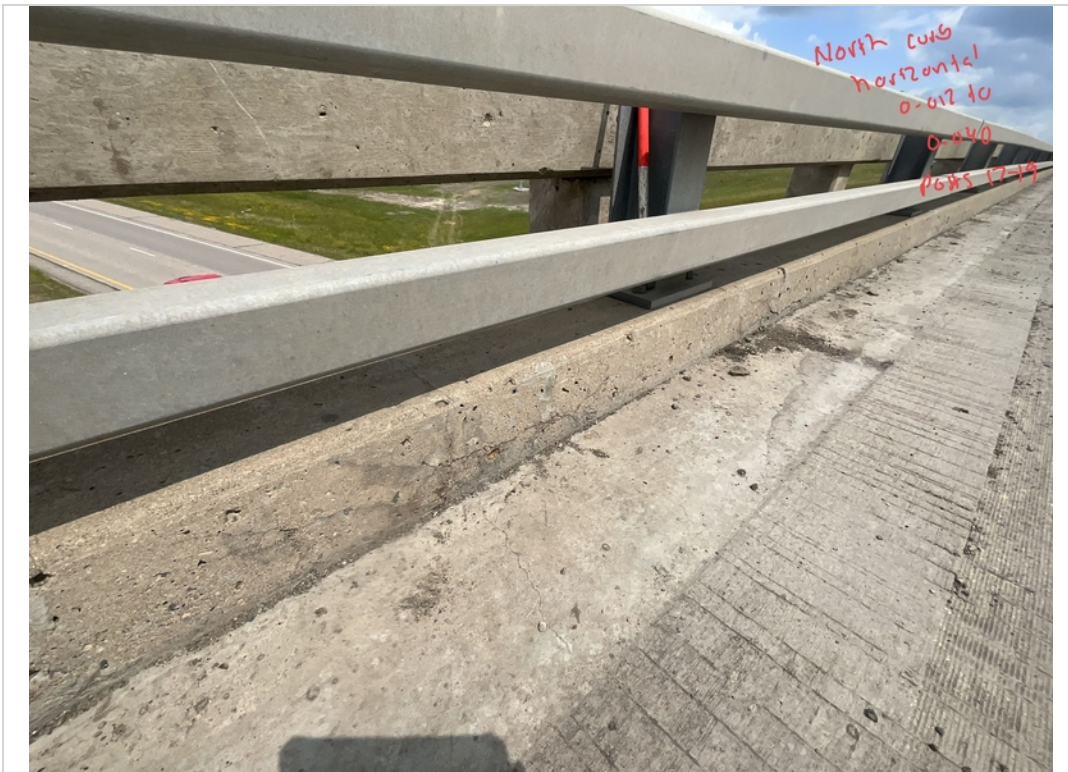
Facing NE. Continued Horizontal Cracking to Face of North Curb from Posts 17-19.
