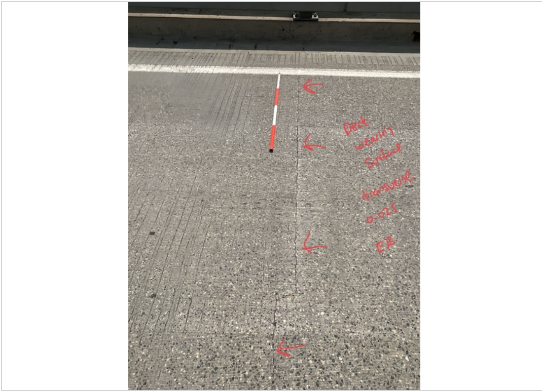
Facing South and Downward. Transverse Crack to Deck Wearing Surface EB Lane.
