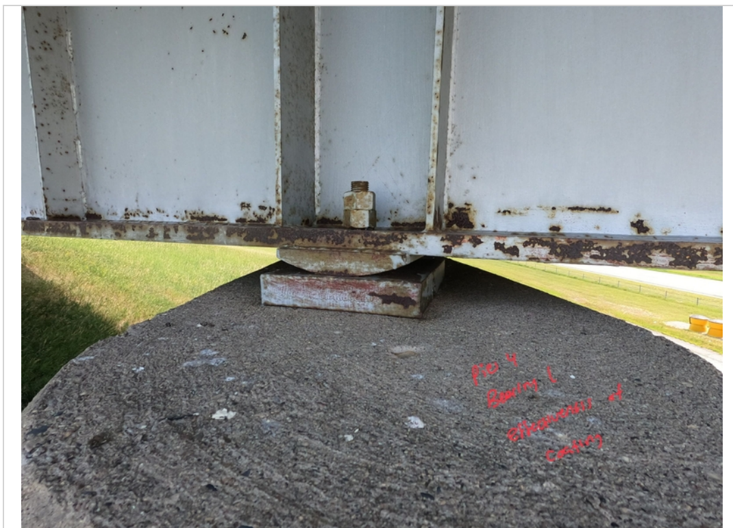
Facing South. Pier 4 Bearing 1 Effectiveness of Coating.
