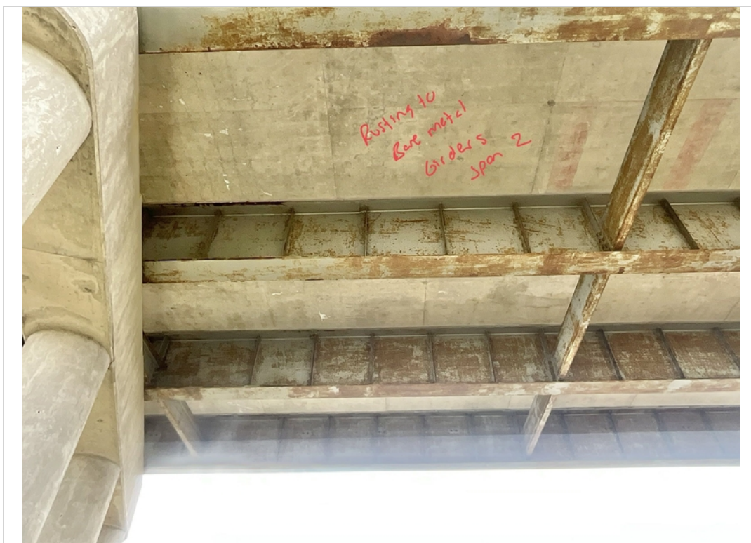
Facing South and Upwards. Rusting to Bare Metal to Girders in Span 2.
