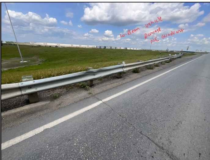
Facing NE. Another View of the Vehicle Impact Damage to W-Beam within NE Quadrant.
