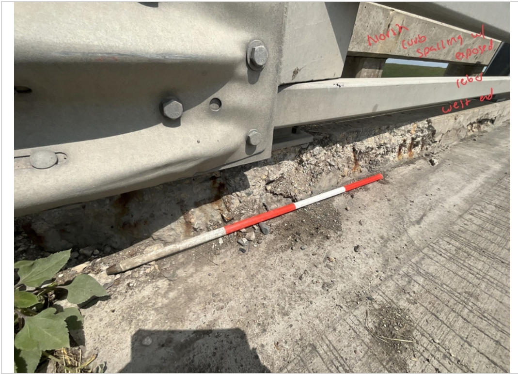
Facing NE. Moderate area of Spalling with Exposed Rebar to North Curb at West End.
