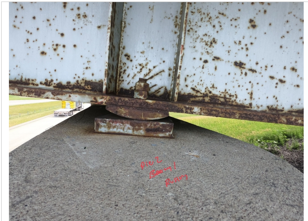
Facing South. Pier 2 Bearing 1 Rusting.
