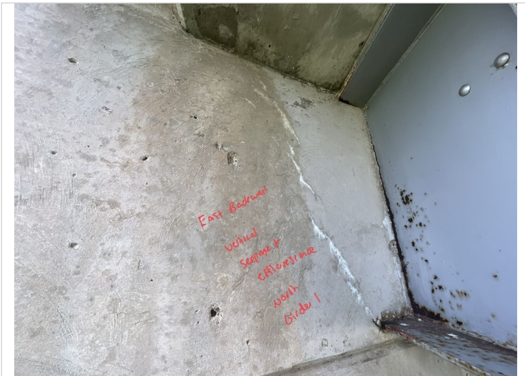
Facing SE. Vertical Crack with seepage and efflorescence to East Backwall North of Girder 1.
