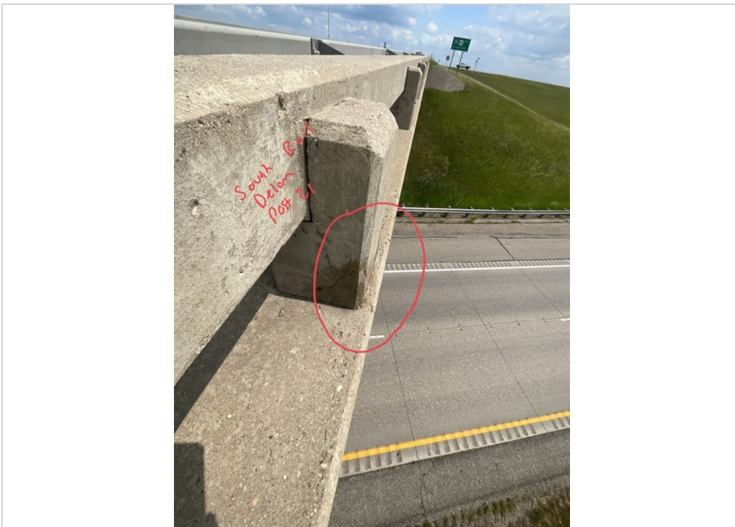
Facing East. Delamination to South Railing Post 21.
