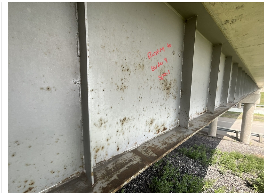
Facing NE. Rusting to Girder 4 in Span 1.
