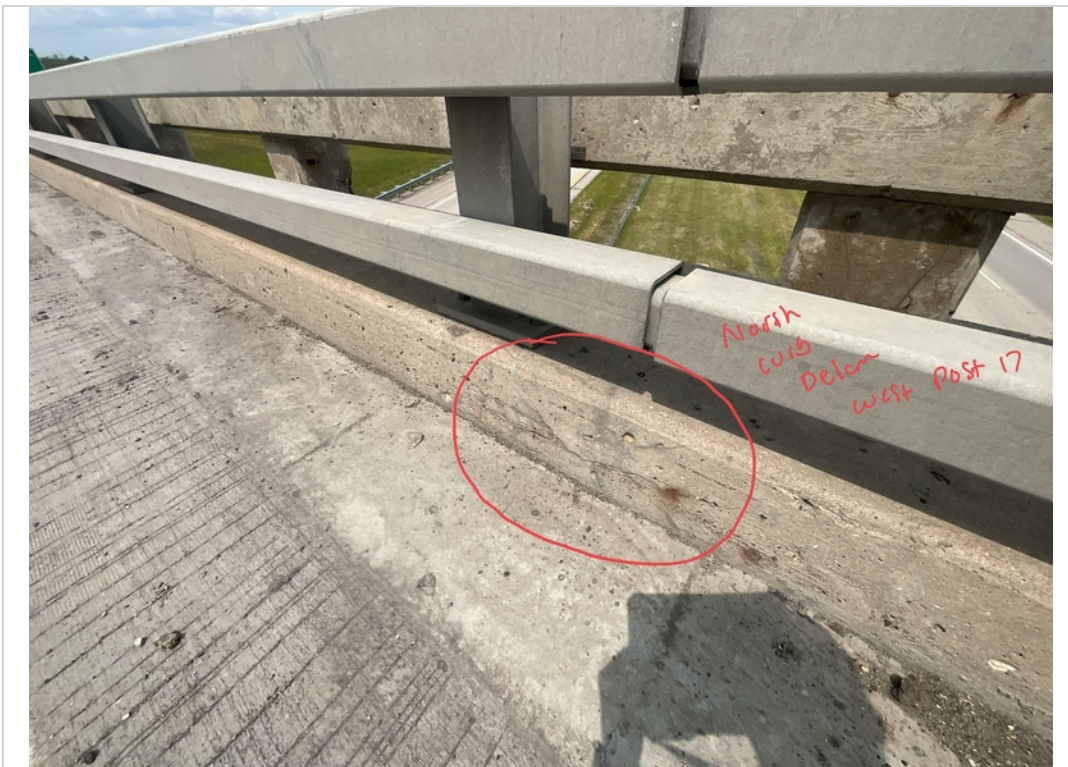
Facing NW. Delamination to Face of North Curb near Post 17.
