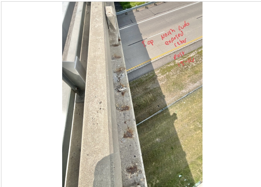
Facing West and Downward. Exposed Rebar to Top of North curb from Posts 15-16.
