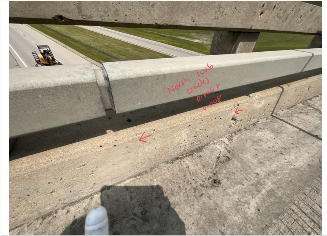
Facing North. Minor Cracks typical to North Curb.
