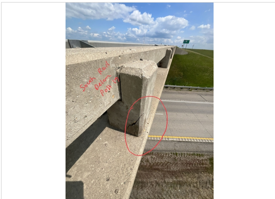
Facing East. Delamination to South Railing Post 17.
