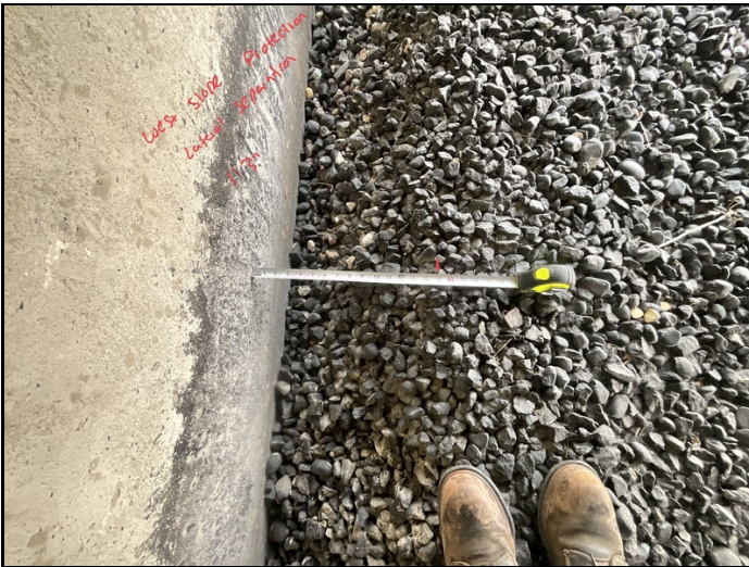
Facing North and Downward. West Slope Protection with Lateral Separation.
