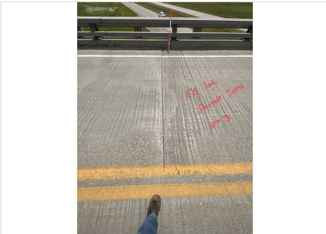
Facing South and Downward. Pourable Joint to EB Lane in Span 4.
