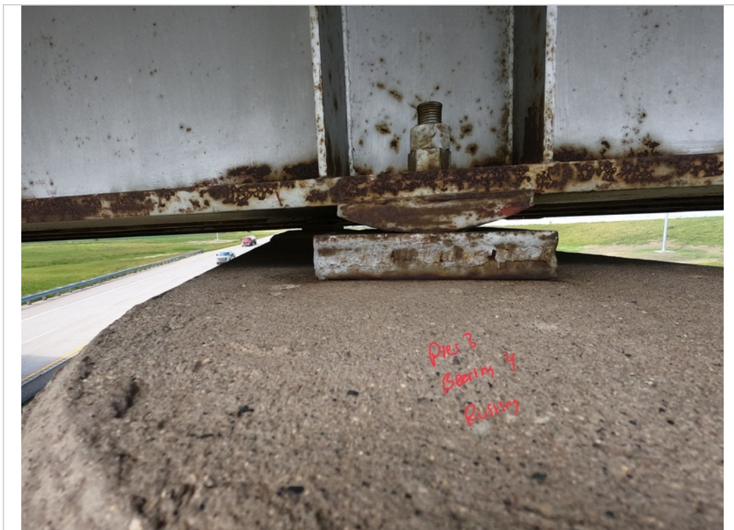
Facing North. Rusting to tPier 3 Bearing 4.
