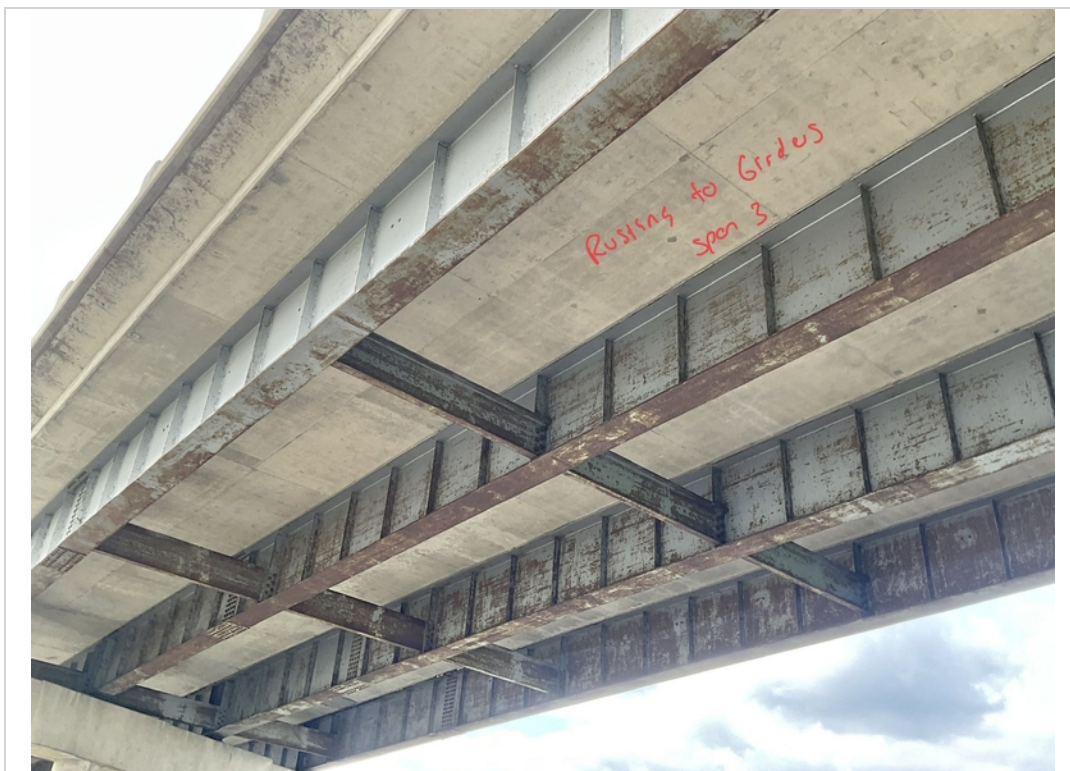
Facing NW and Upwards. Rusting to Girders in Span 3.
