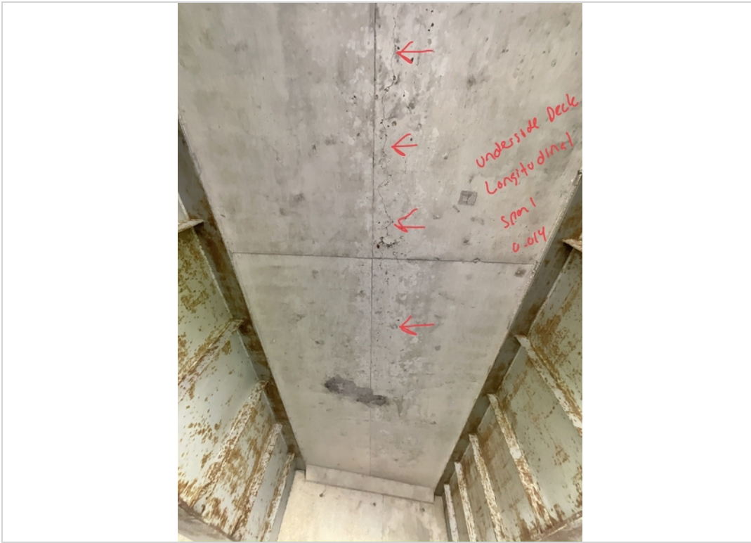
Facing West and Upwards. Longitudinal Crack along CL of Underside Deck in Span 1.
