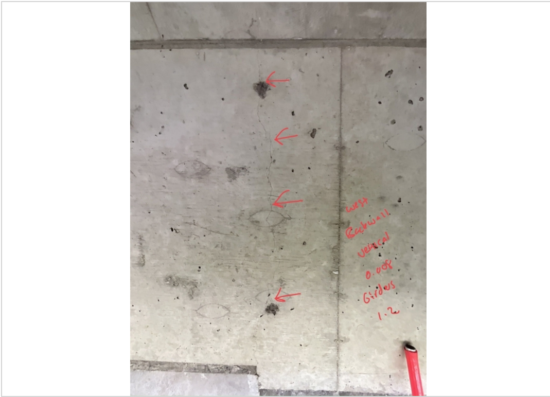
Facing West. Vertical Crack to West Backwall in-between Girders 1 and 2.
