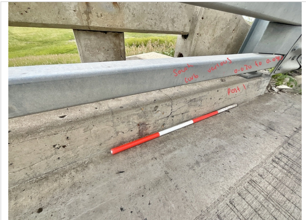
Facing SW. Various Cracks to South curb near Post 1.
