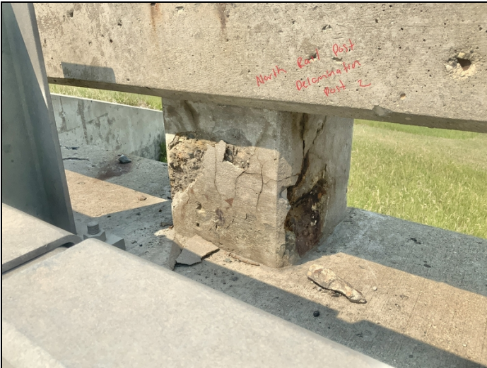
Facing NW. Spalling with Exposed Rebar to North Rail at Post 2.
