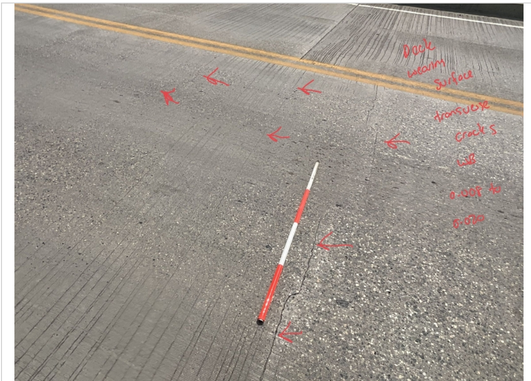
Facing South. Continued Patterned Transverse Cracking to Deck Wearing Surface.
