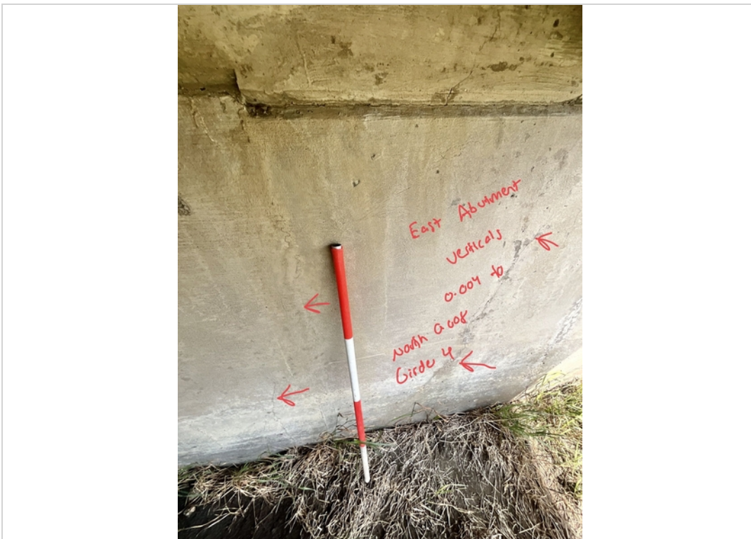
Facing East. Attempting to show minor vertical cracks to East Abutment North of Girder 4.
