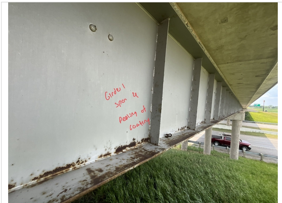
Facing West. Peeling of Coating to Girder 1 in Span 4.
