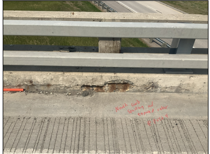
Facing North. Spalling with Exposed Rebar to North Curb at Post 4.
