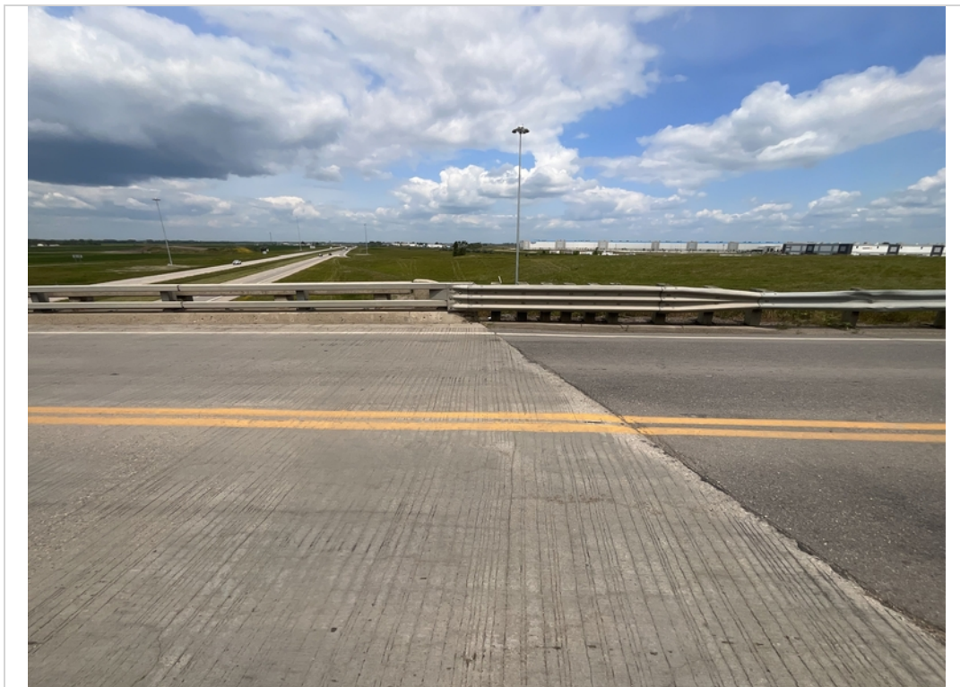
Facing North. Guardrail Transition at NE Corner. Similar at SE Corner.
