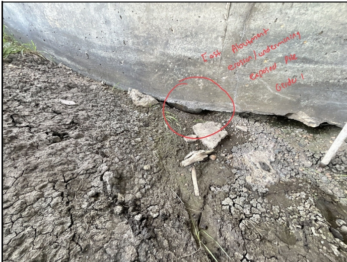
Facing East. Erosion area under East Abutment Exposing 1 Pile.
