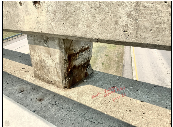
Facing NW. Spalling with Exposed Rebar to North Railing at Post 20.
