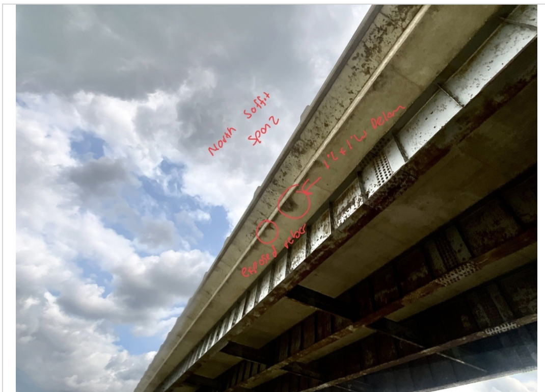
Facing SE and Upwards. Areas of Delamination and Exposed Rebar to North Soffit in Span 2.
