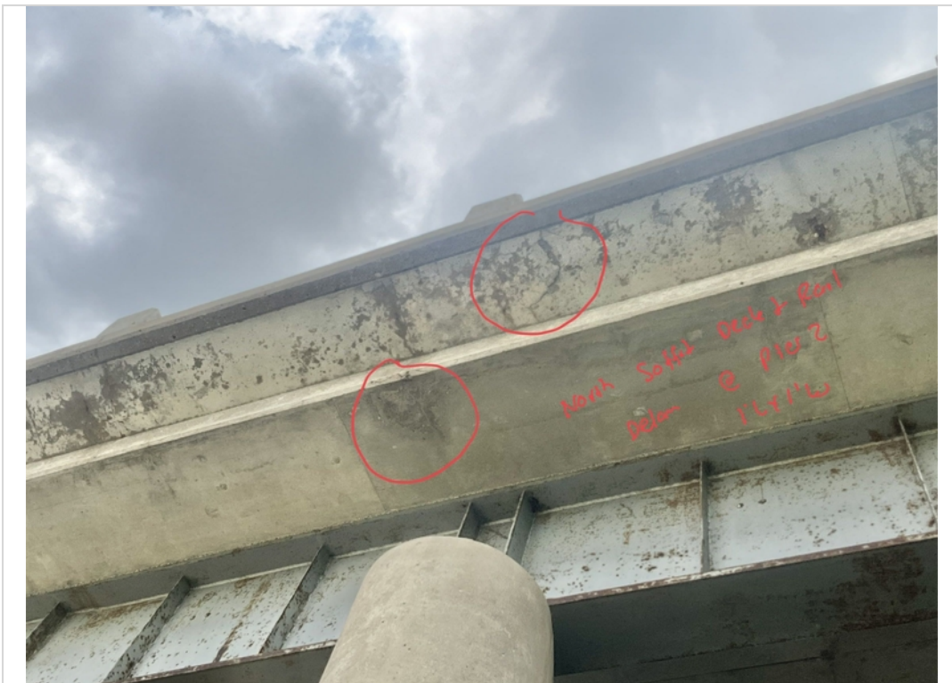
Facing South and Upwards. Delamination to North Soffit of Deck and Railing near Pier 2.
