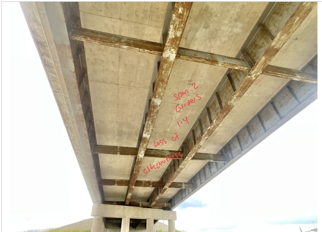
Facing West and Upwards. Loss of Effectiveness to coating system Girders in Span 2.
