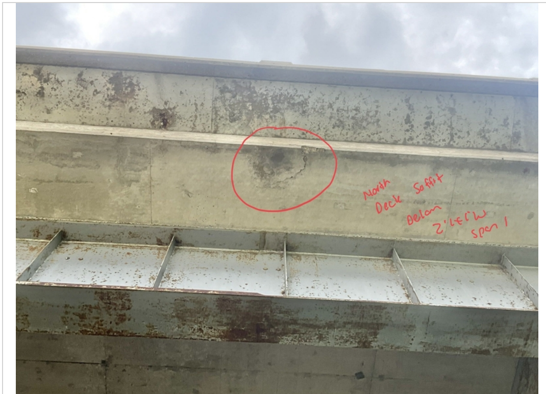
Facing South and Upwards. Delamination to North Soffit in Span 1.
