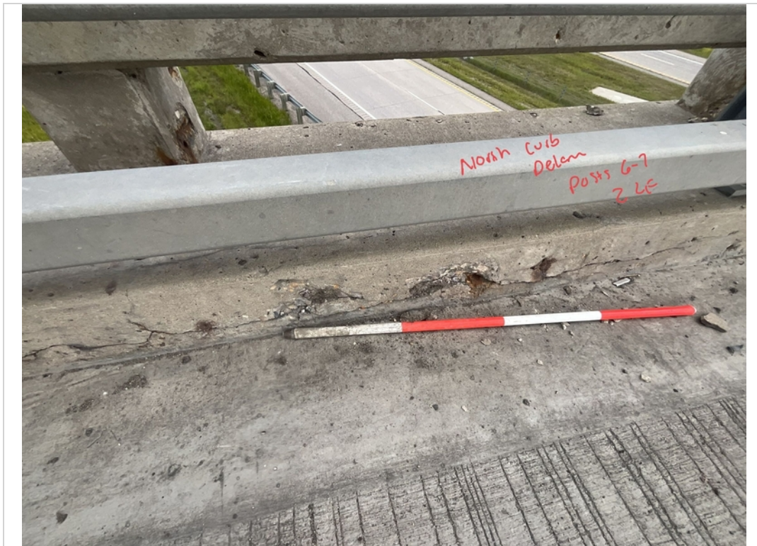
Facing North. Delamination to North Curb face from Posts 6-7.
