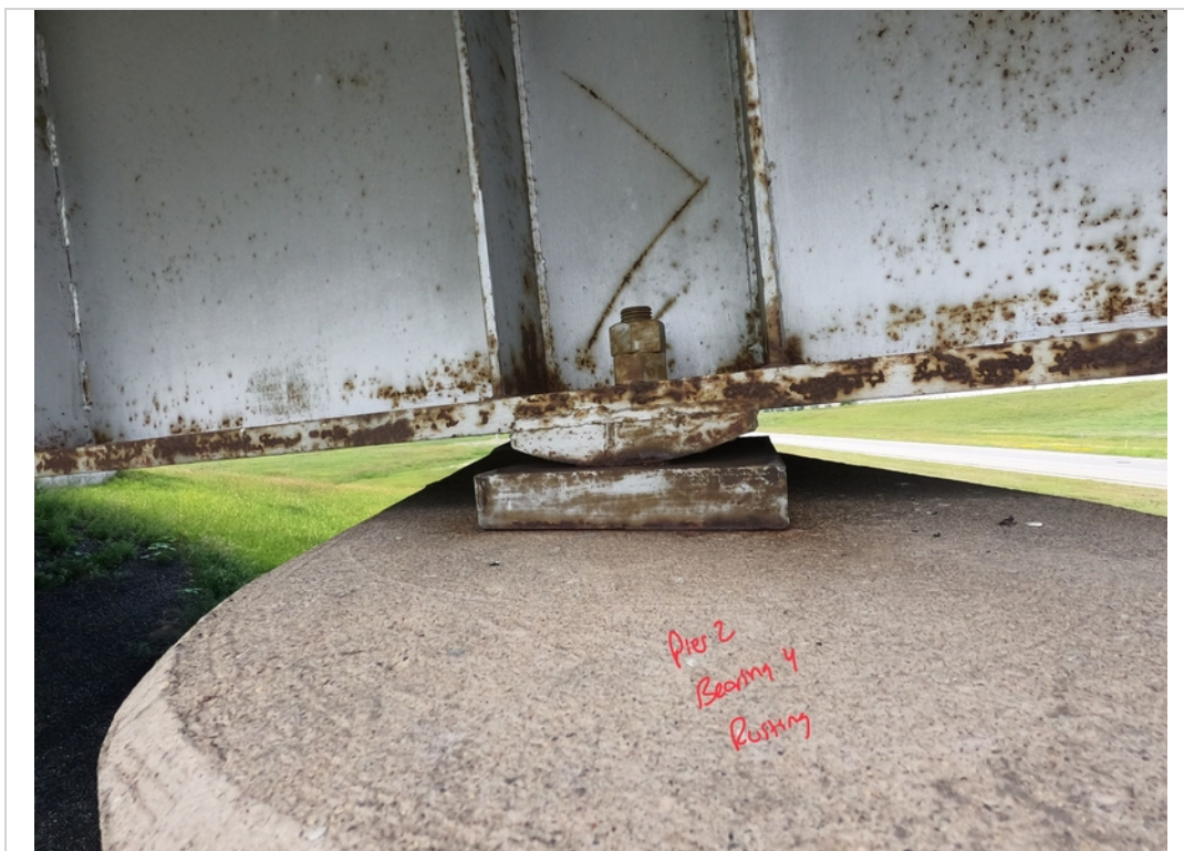
Facing North. Pier 2 Bearing 4 Rusting.
