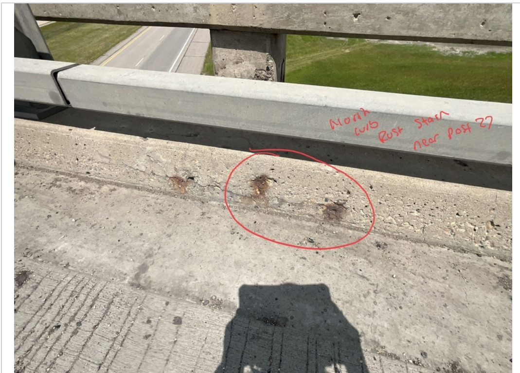
Facing North and Downward. Rust Staining to North Curb near Post 27.
