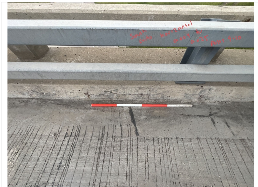
Facing South and downward. Horizontal Crack to Face of South Curb from Posts 9-10.
