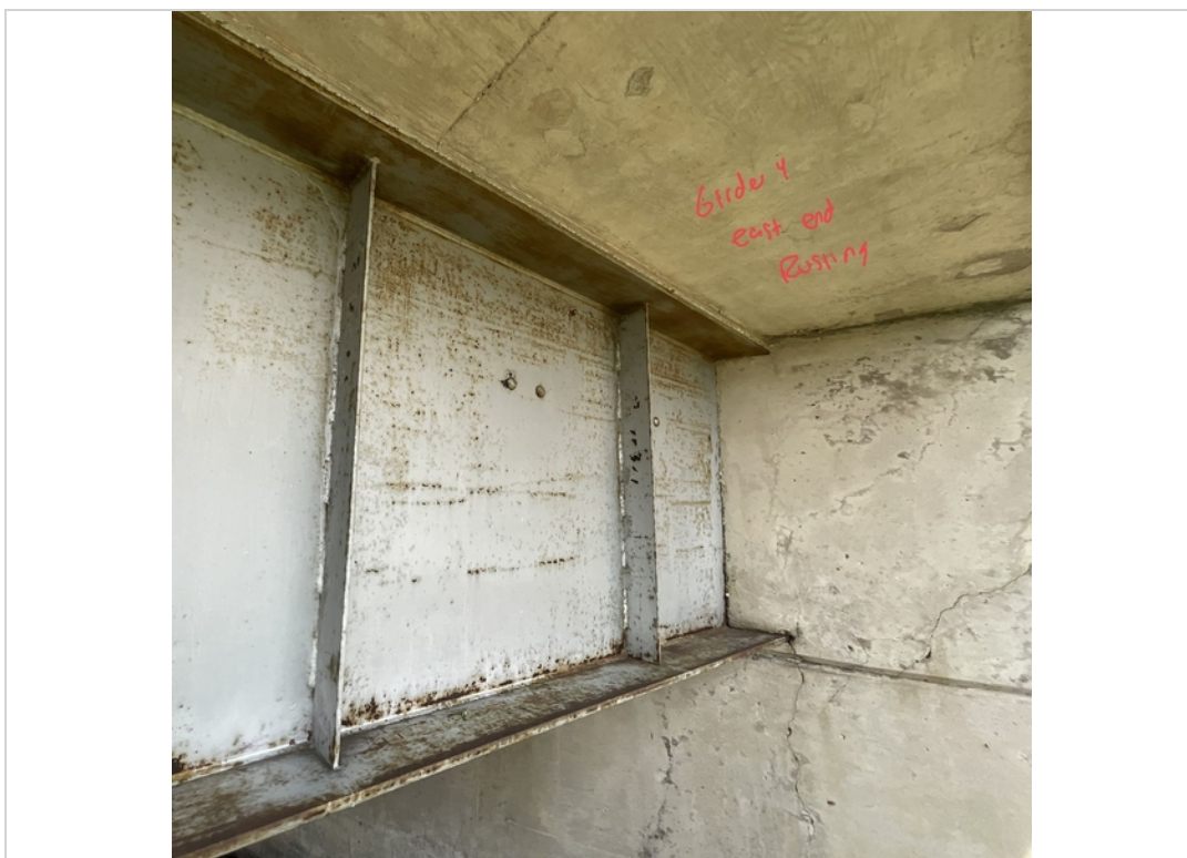
Facing NE. Rusting to Girder 4 near East End.
