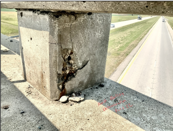
Facing NW. Spalling to North Railing at Post 22.
