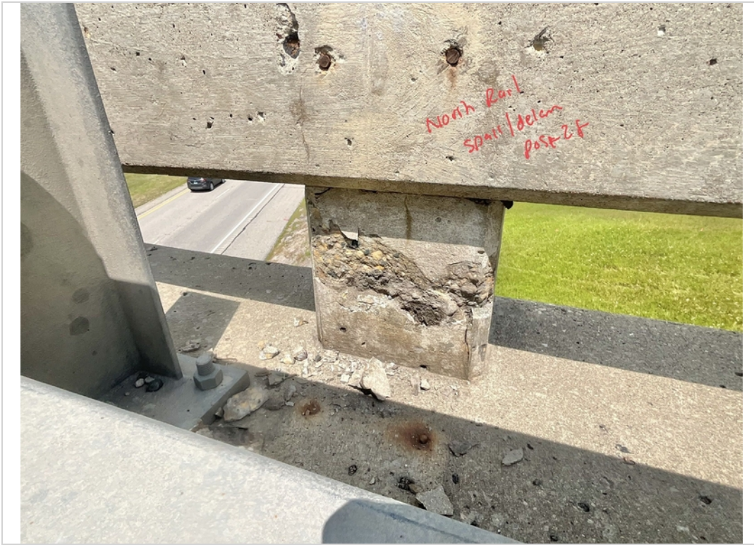
Facing North. Delamination/Spalling to North Railing Post 31.
