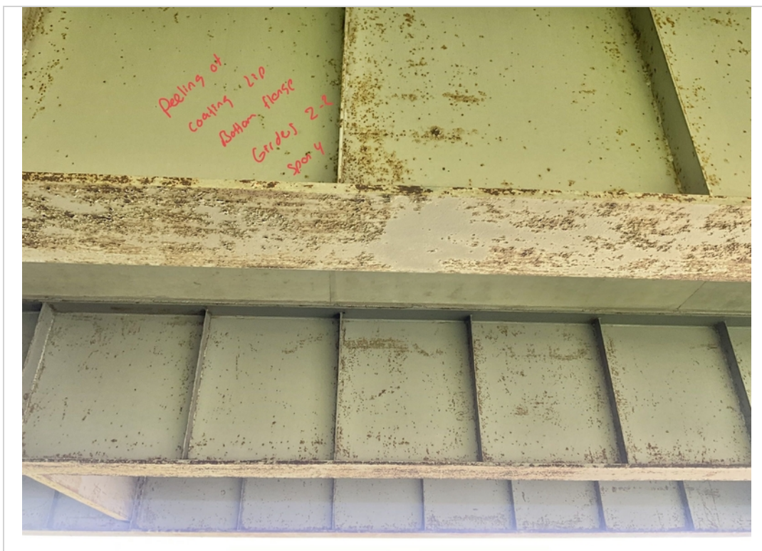
Facing South and Upwards. Peeling of Coating to Lips of Bottom Flanges of Girders in Span 4.
