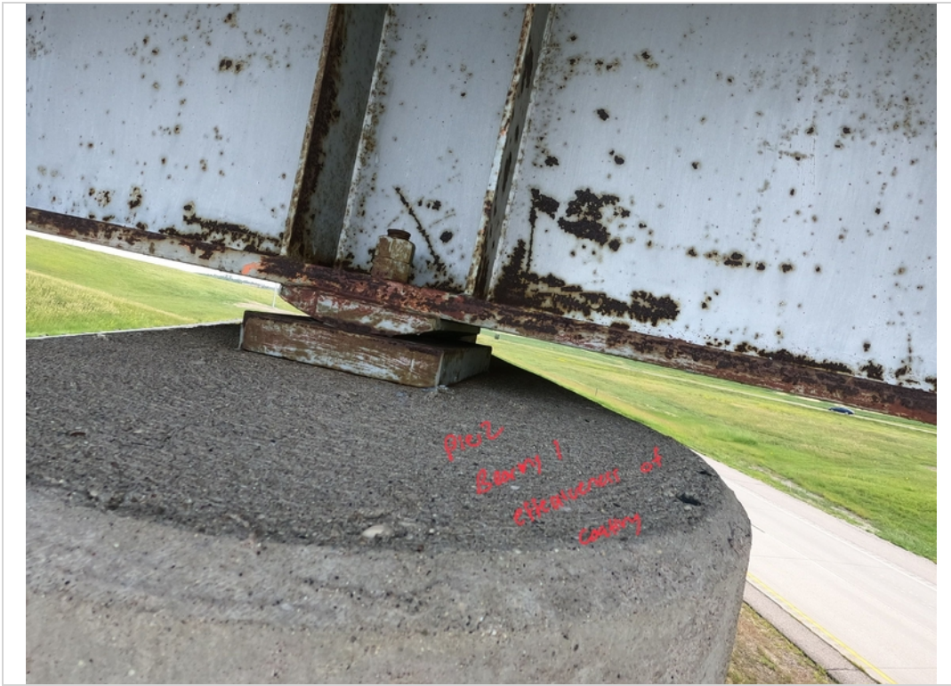
Facing South. Pier 2 Bearing 1 Effectiveness of Coating.
