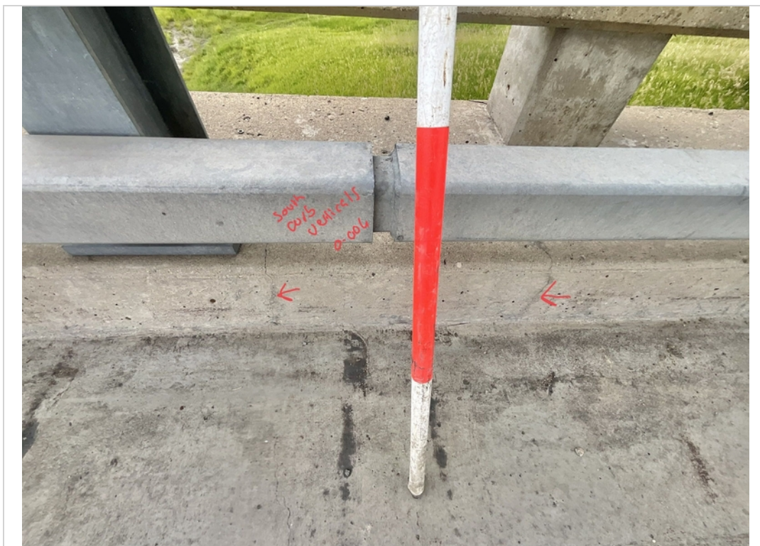
Facing South and Downward. Typical Cracks to South Curb.
