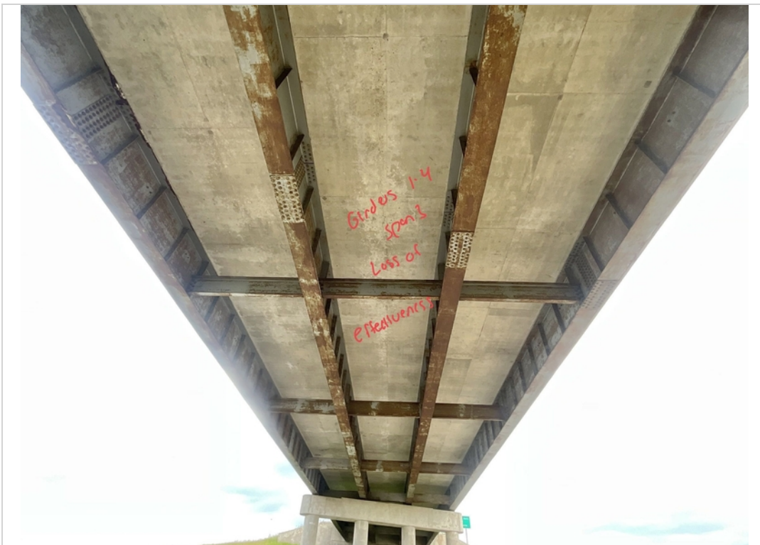
Facing East and Upwards. Loss of effectiveness of Girders 1-4 in Span 3.
