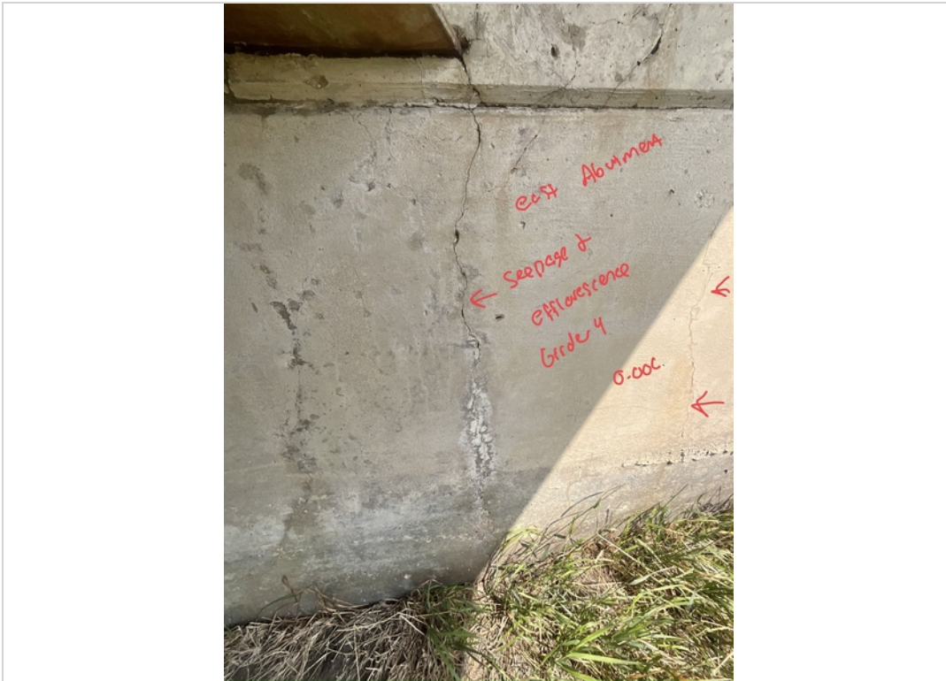
Facing East. Vertical Crack with 1 crack having Seepage and Efflorescence to East Abutment under Girder 4.
