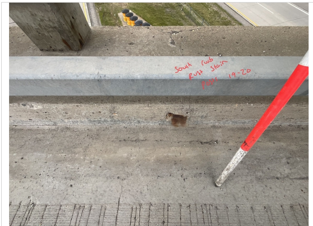
Facing South and Downward. Rust Stain to Face of South Curb from Posts 19-20.
