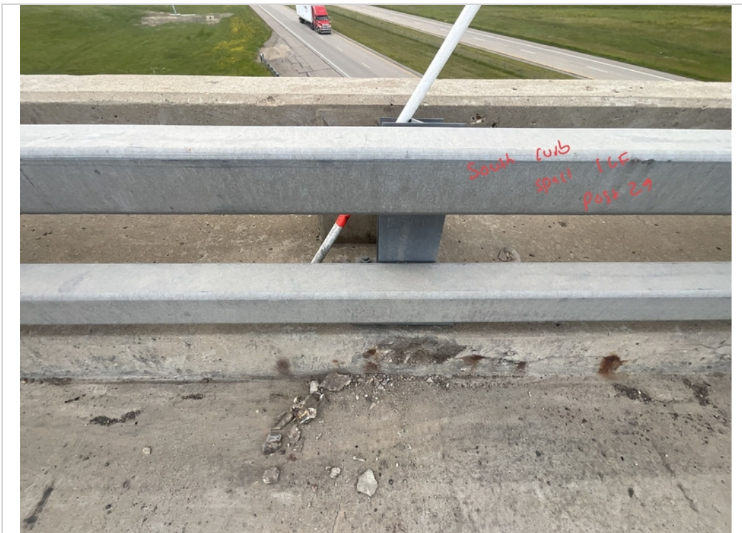
Facing South. Spall to Face of South Curb at Post 29.
