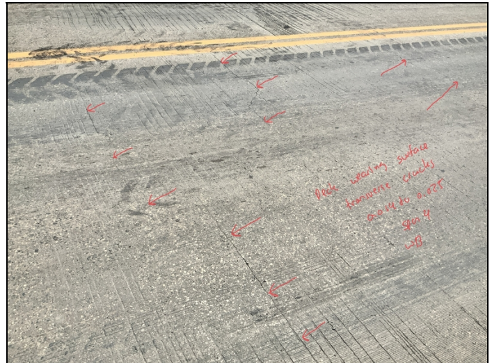
Facing SW and Downward. Transverse cracking to Deck Wearing Surface of the WB Lane of Span 4.
