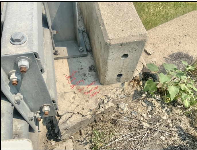
Facing East and Downward. Spalling to South Curb at West End.
