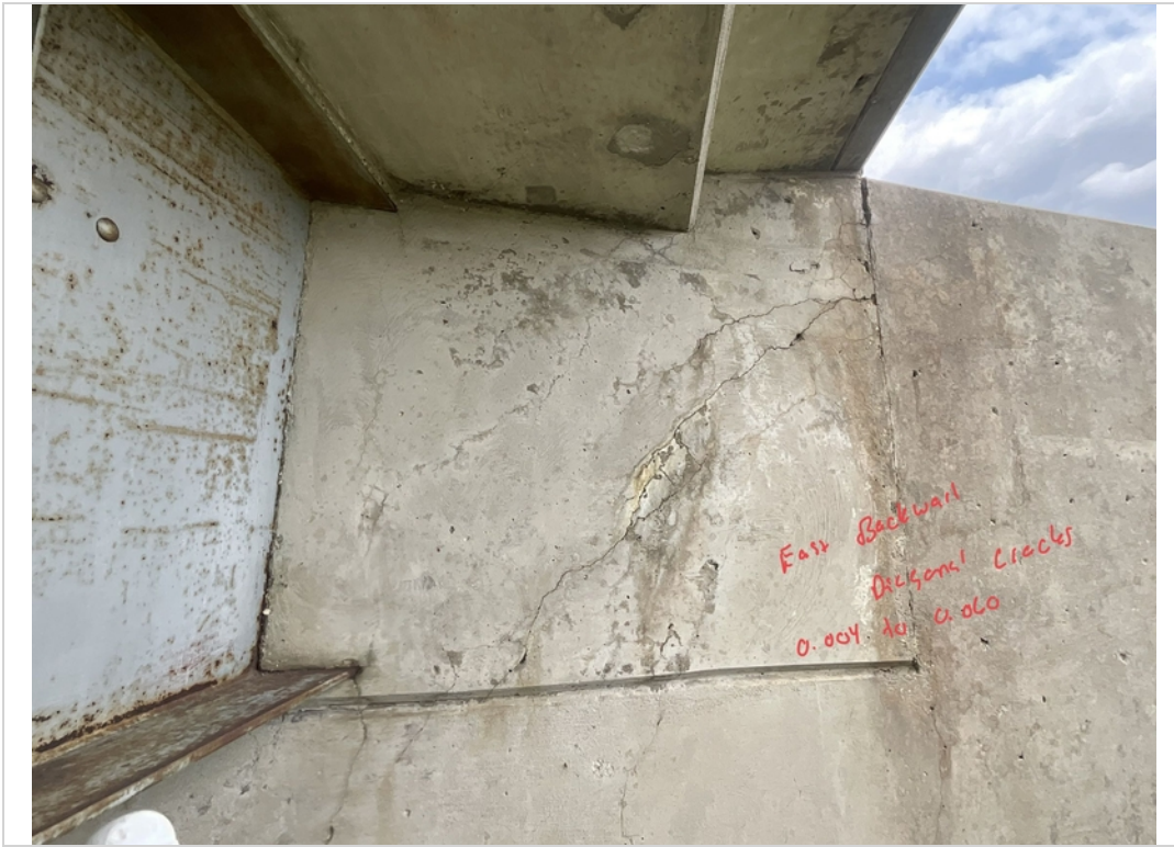
Facing East. Area of Moderate Cracking to East Backwall South End.
