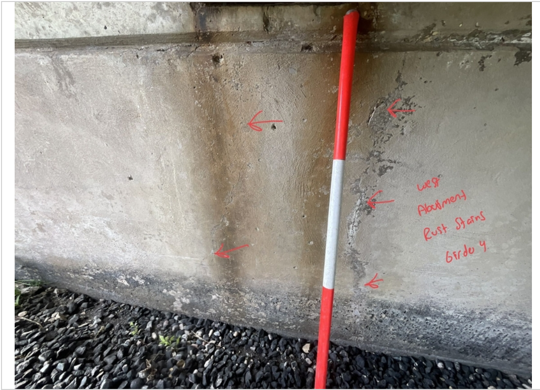
Facing West. Rust Stains to West Abutment under Girder 4.
