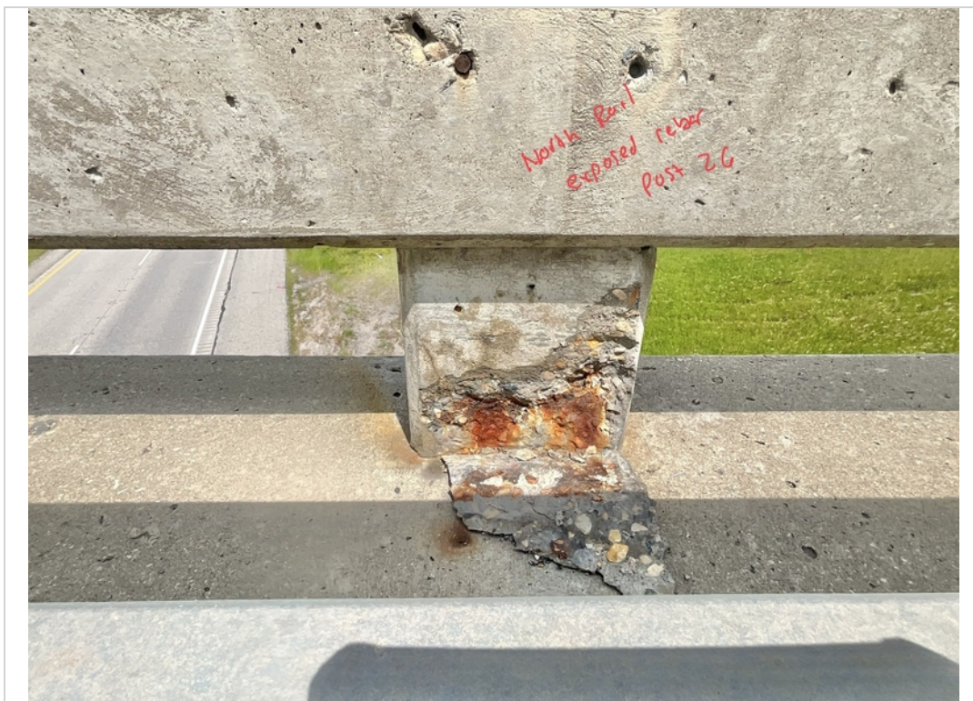
Facing North. Exposed Rebar to North Railing Post 26.
