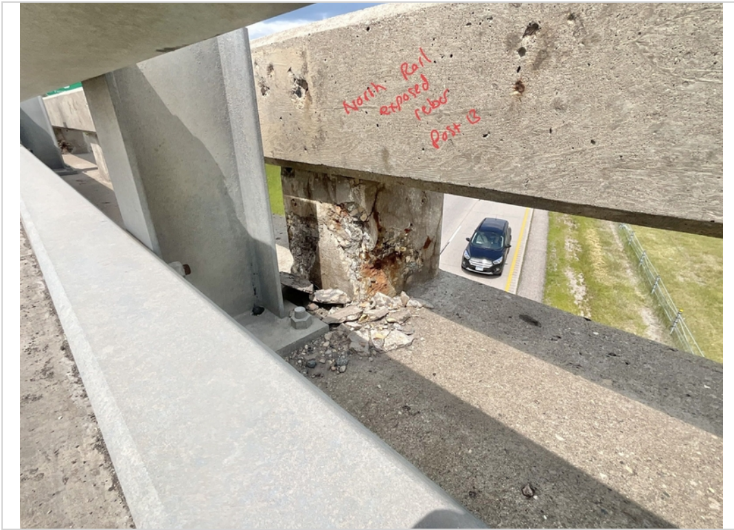
Facing NW. Spalling with Exposed Rebar to North Railing at Post 13.
