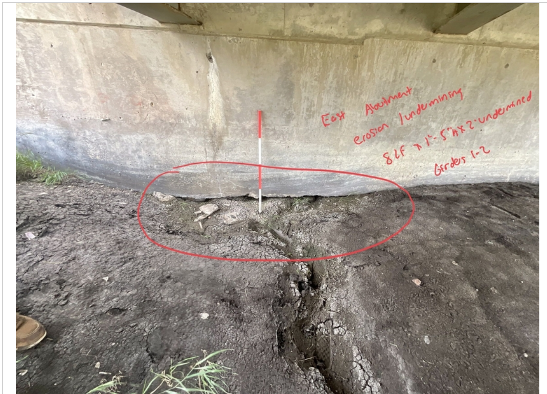
Facing East. Continued Erosion area to East Abutment.
