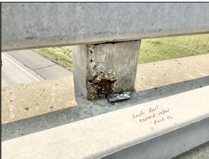
Facing South. Exposed Rebar to South Railing Post 12.
