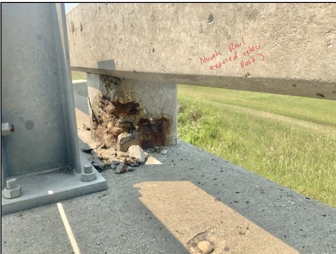
Facing NW. Spalling with Exposed Rebar to North Railing at Post 3.
