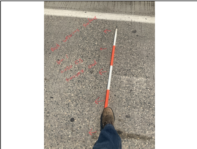
Facing South and Downward. Transverse Crack to Deck Wearing Surface in the EB Lane of Span 1.
