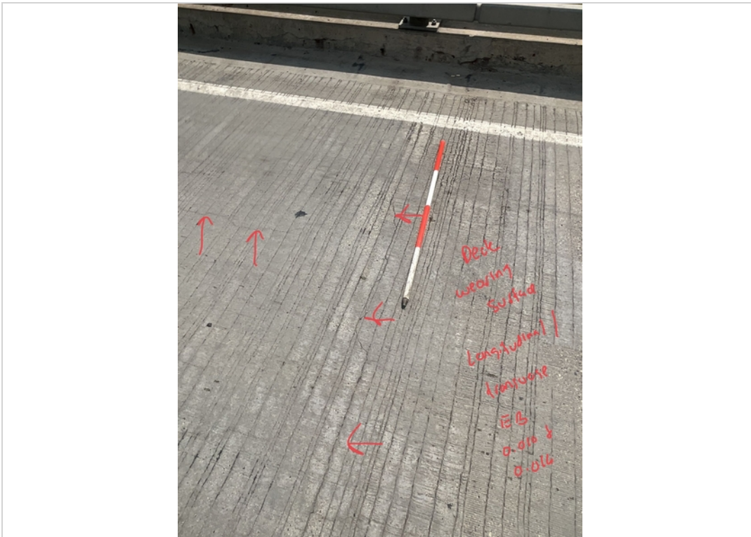
Facing South and Downward. Longitudinal Cracks to Deck Wearing Surface EB Lane.
