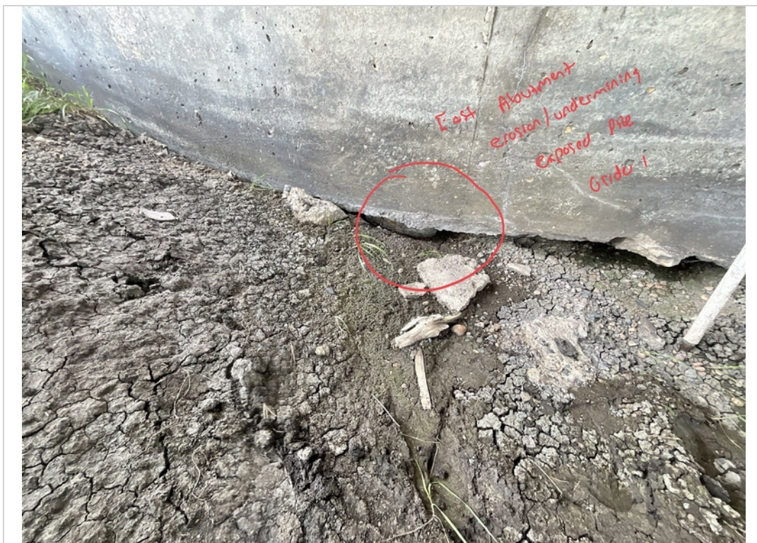
Facing East. Erosion area under East Abutment Exposing 1 Pile.
