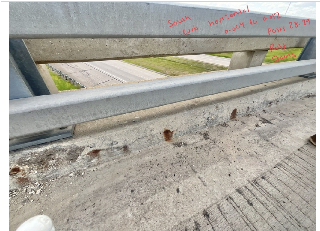
Facing South. Rust stains with Horizontal Cracks to Face of South Curb from Posts 28-29.
