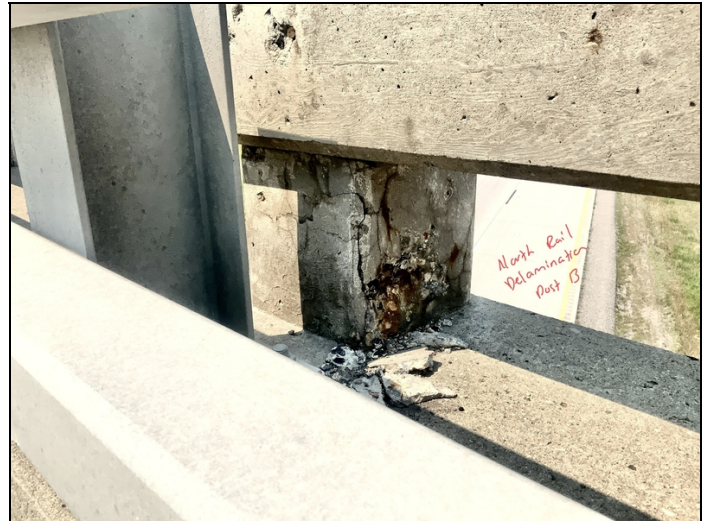
Facing NW. Spalling with Exposed Rebar to North Railing at Post 13.
