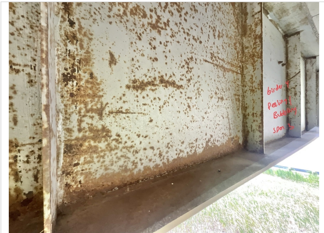
Facing SW. Peeling and Bubbling of Coating to Girder 3 in Span 4.
