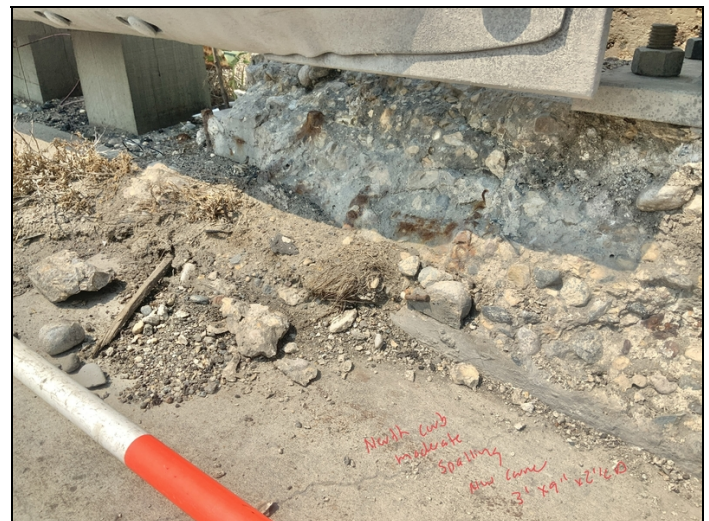
Facing NW. Moderate Spalling to North Curb near SW Corner.
