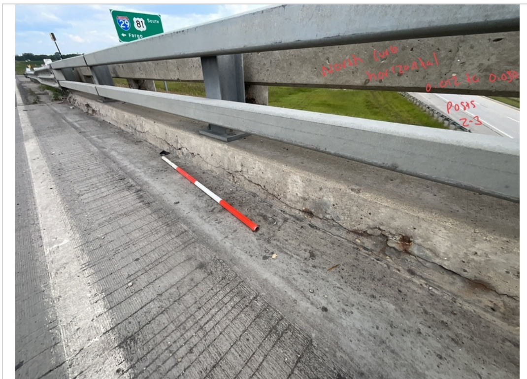
Facing NW. Horizontal Crack to Face of North Curb from Posts 2-3.
