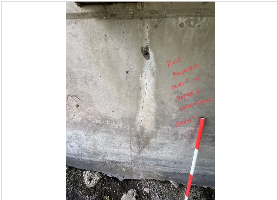
Facing East. Vertical Crack with seepage and efflorescence to East Abutment under Girder 1.
