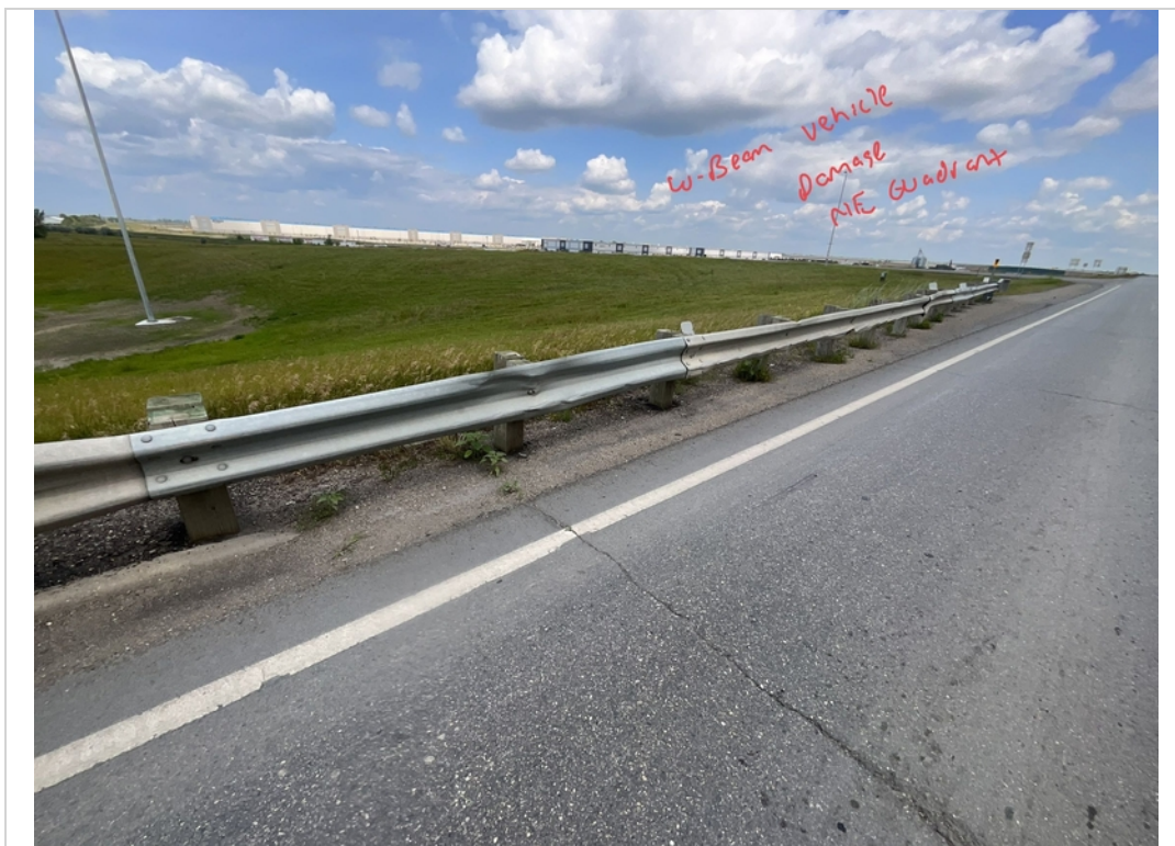
Facing NE. Another View of the Vehicle Impact Damage to W-Beam within NE Quadrant.
