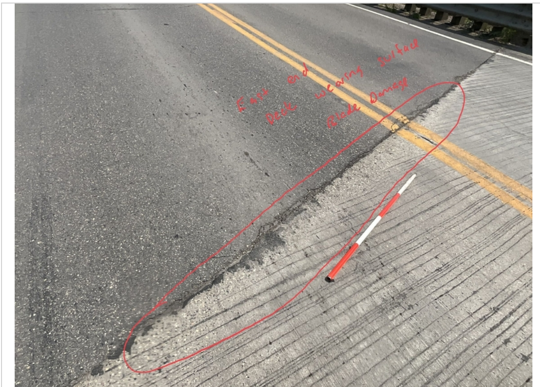
Facing SE and Downward. Minor Blade Damage to East End of Deck Wearing Surface
