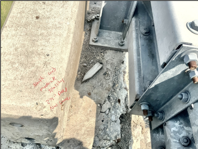
Facing East and Downward. Another View of the Moderate Spalling to North Curb near West End.
