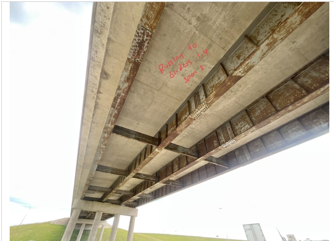
Facing SE and Upwards. Rusting to Girders 1-4 in Span 2.
