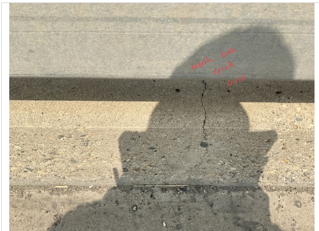
Facing North and Downward. Typical Crack to North curb.
