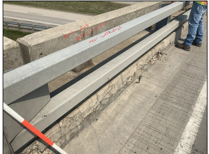
Facing NE. Spalling and Delamination to North Curb near West End.
