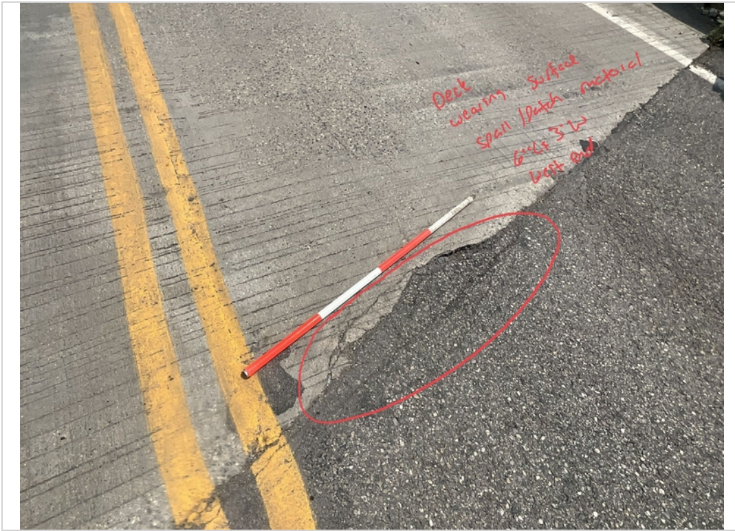
Facing SE and Downward. Spall to West End of Deck Wearing Surface EB Lane.
