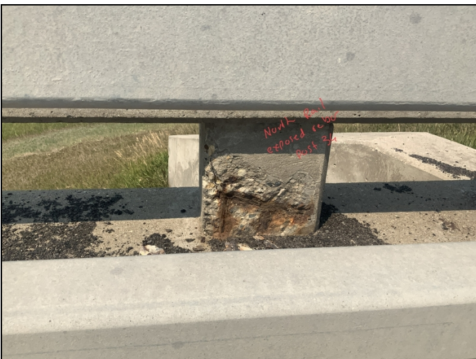
Facing North. Exposed Rebar to North Railing at Post 36.
