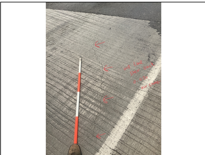
Facing SW and Downward. Shear Crack to Deck Wearing Surface near NW Corner.
