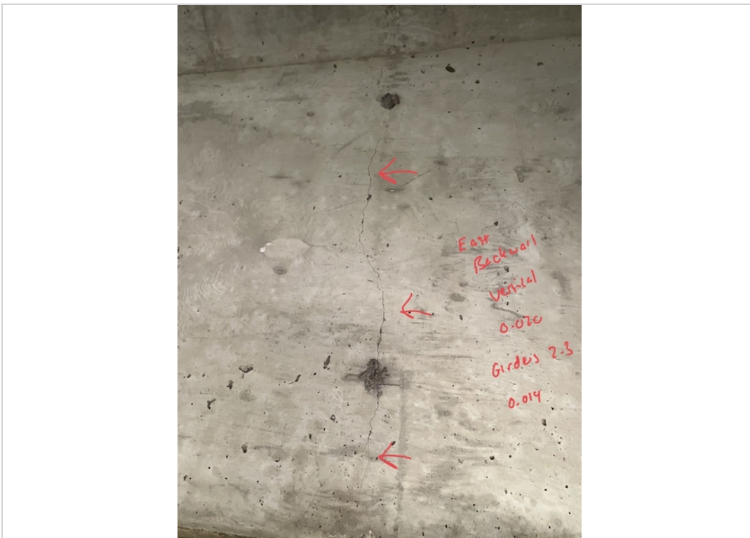
Facing East. Vertical Crack to East Backwall in-between Girders 2 and 3.
