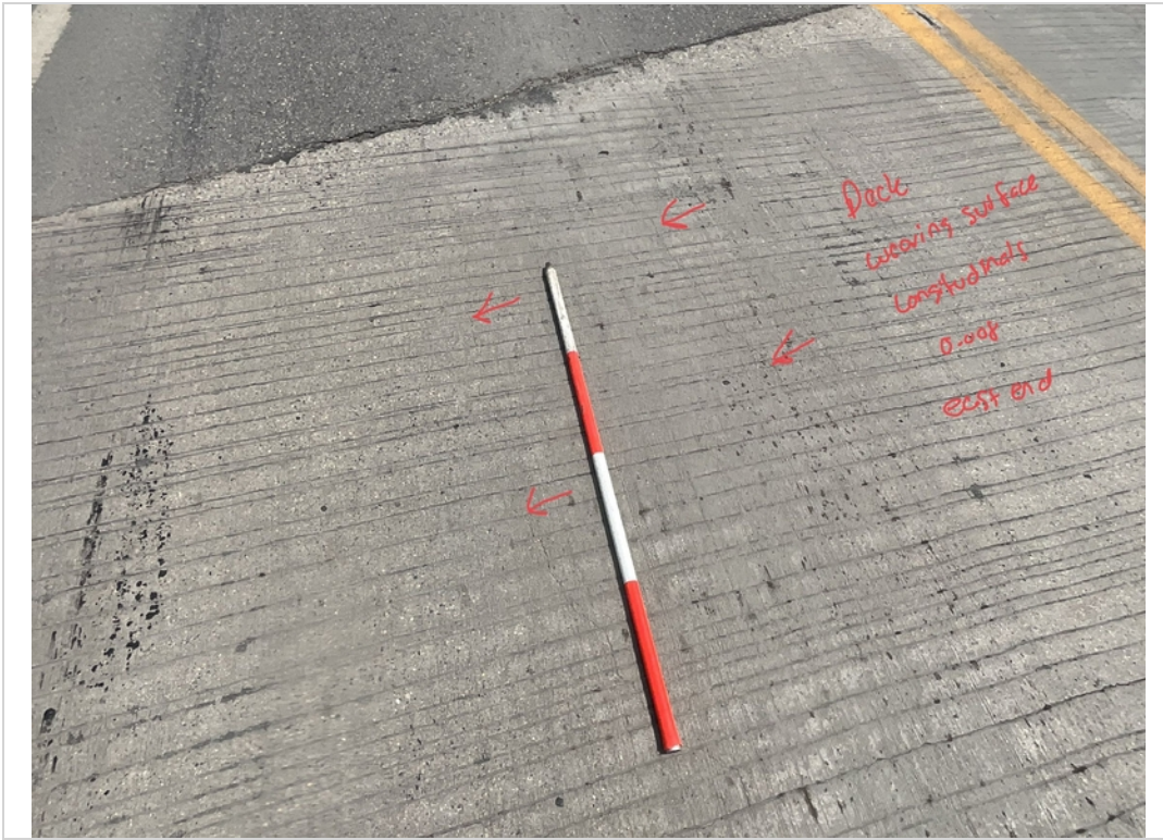
Facing East and Downward. Attempting to show minor longitudinal Cracks to Deck Wearing Surface East End.
