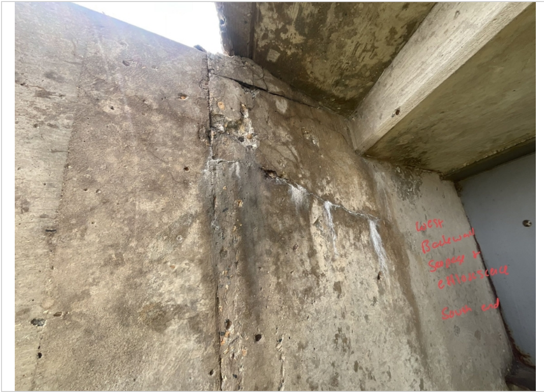
Facing NW and Upwards. Cracks with seepage and efflorescence to West backwall South End.
