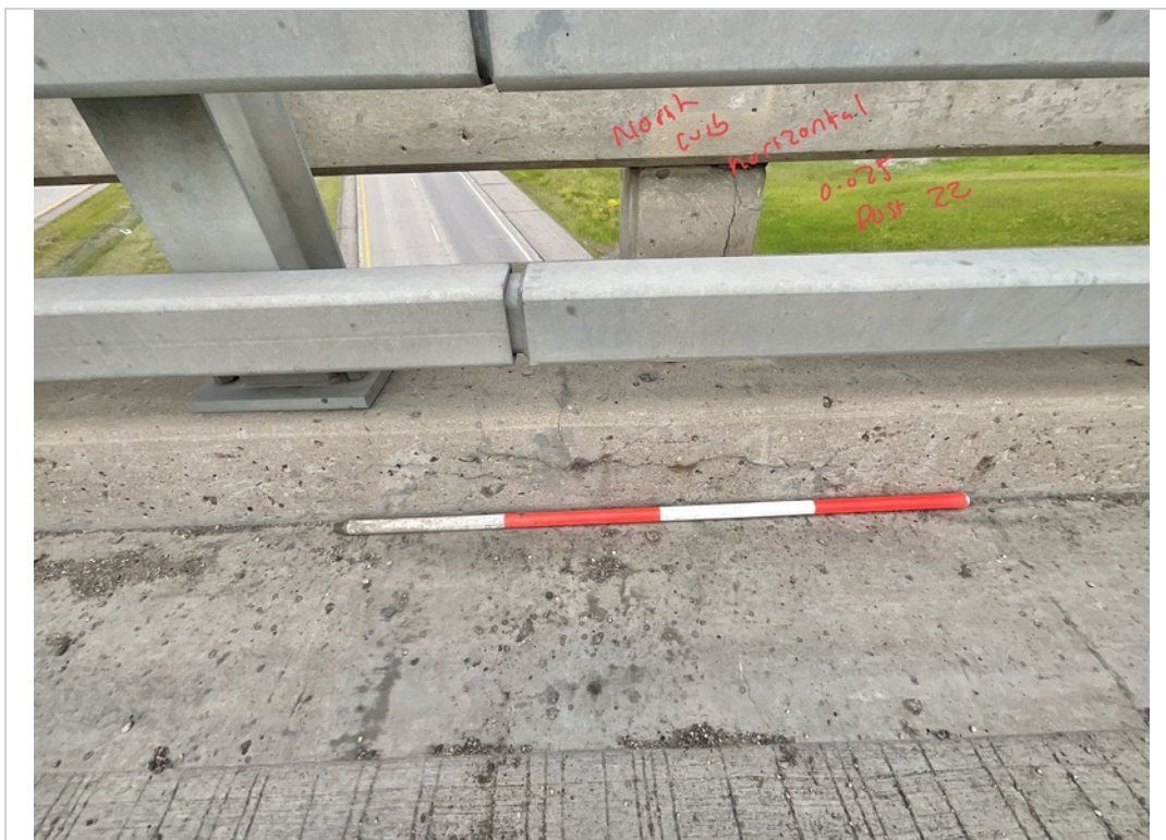
Facing North. Horizontal Crack to Face of North Curb at Post 22.
