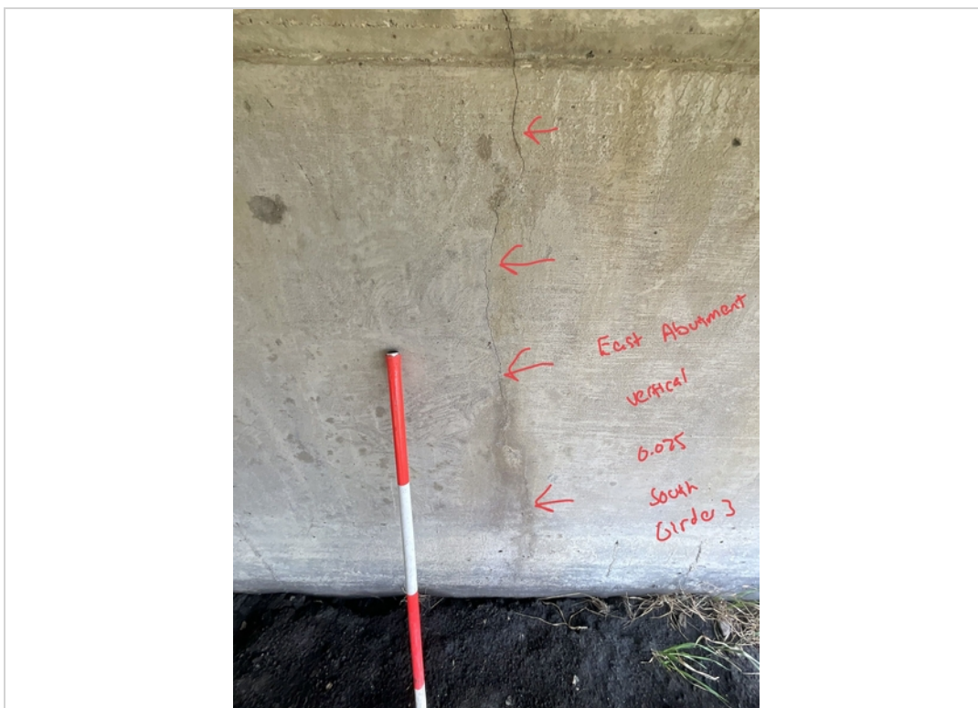
Facing East. Minor Vertical Crack to East Abutment South of Girder 3.
