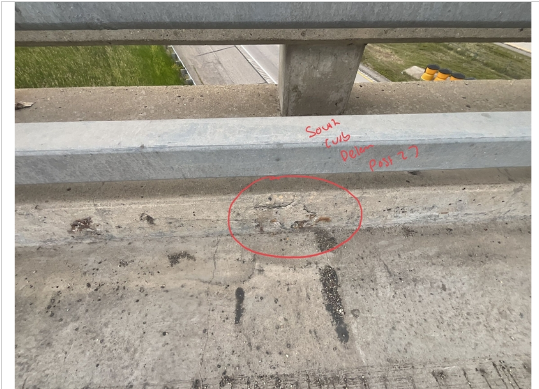
Facing South. Delam to Face of South Curb near Post 27.
