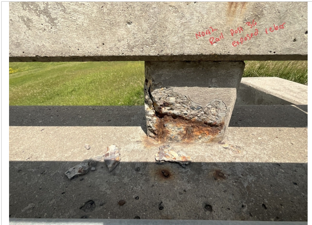
Facing North. North Rail Post 26 with Exposed Rebar.
