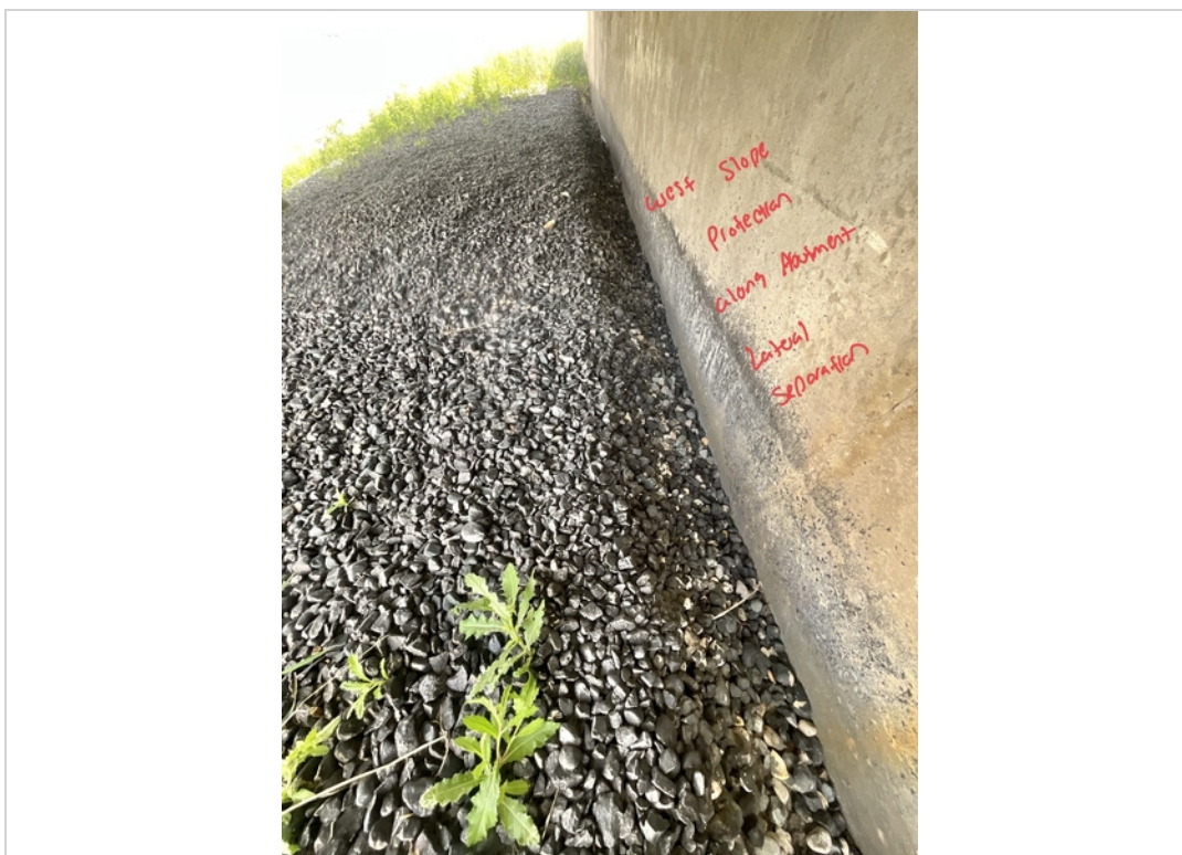
Facing South. West Slope Protection along Abutment with Lateral Separation.
