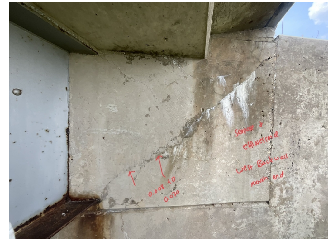
Facing West. Diagonal Crack with seepage and efflorescence to West Backwall North End.
