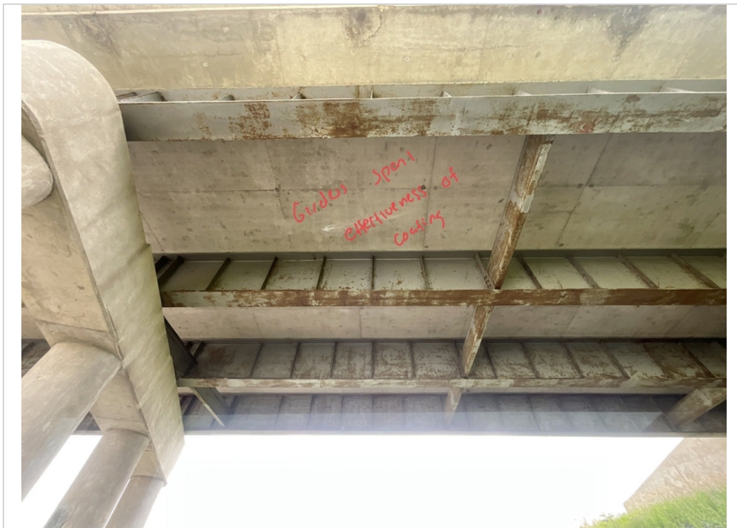
Facing South and Upwards. Effectiveness of Coating to Girders in span 1.
