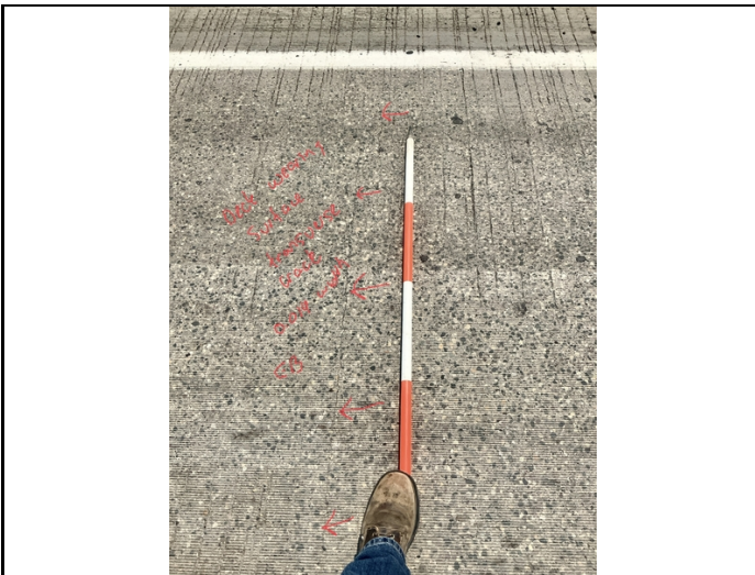
Facing South and Downward. Deck Wearing Surface Transverse Crack to EB Lane.
