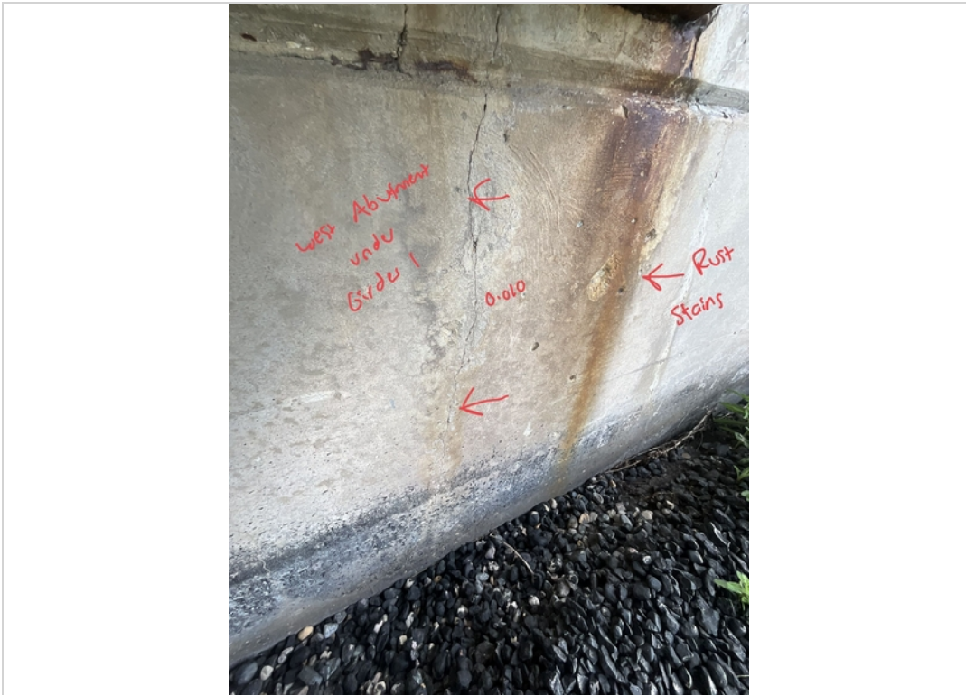
Facing NW. Vertical Crack with Rust stains to West Abutment under Girder 1.
