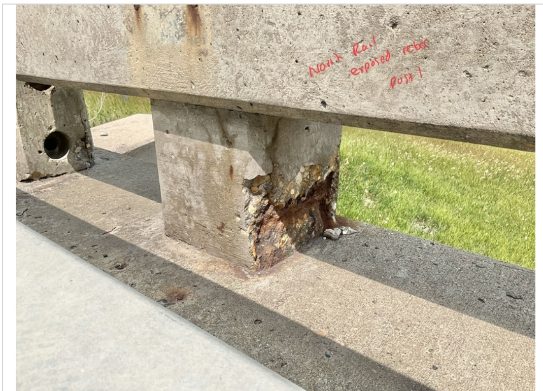
Facing NW. Exposed Rebar to North Railing Post 1.
