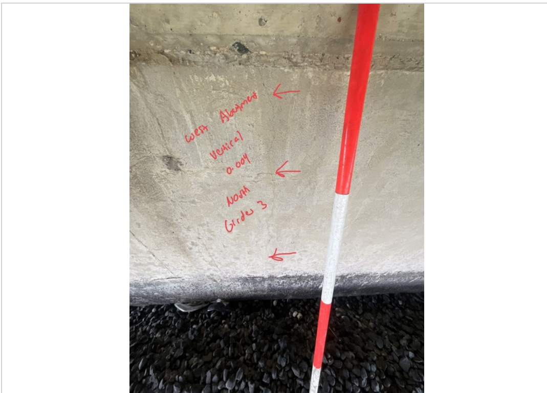
Facing West. Minor Vertical Crack to West Abutment North of Girder 3.
