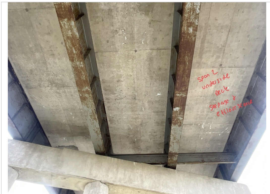
Facing East and Upwards. Underside Deck Seepage and Efflorescence Span 2.
