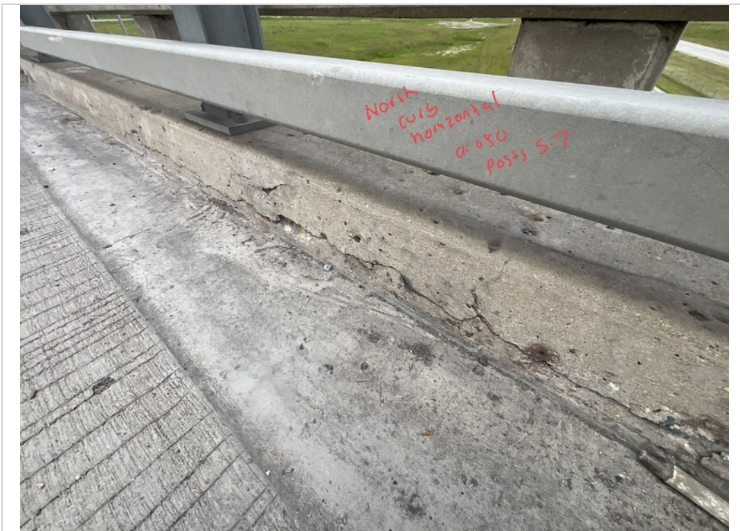
Facing NW. Horizontal Crack to Face of North Curb from posts 5-7.
