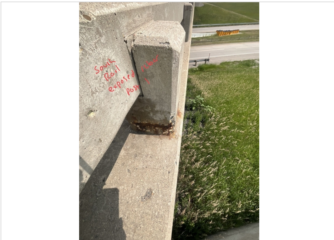
Facing East. Exposed Rebar to South Railing at Post 1.
