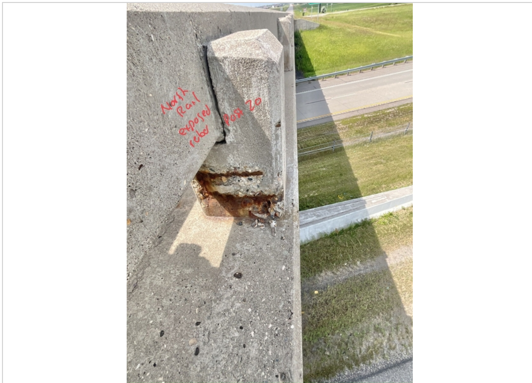
Facing West. Exposed Rebar to North Railing Post 20.
