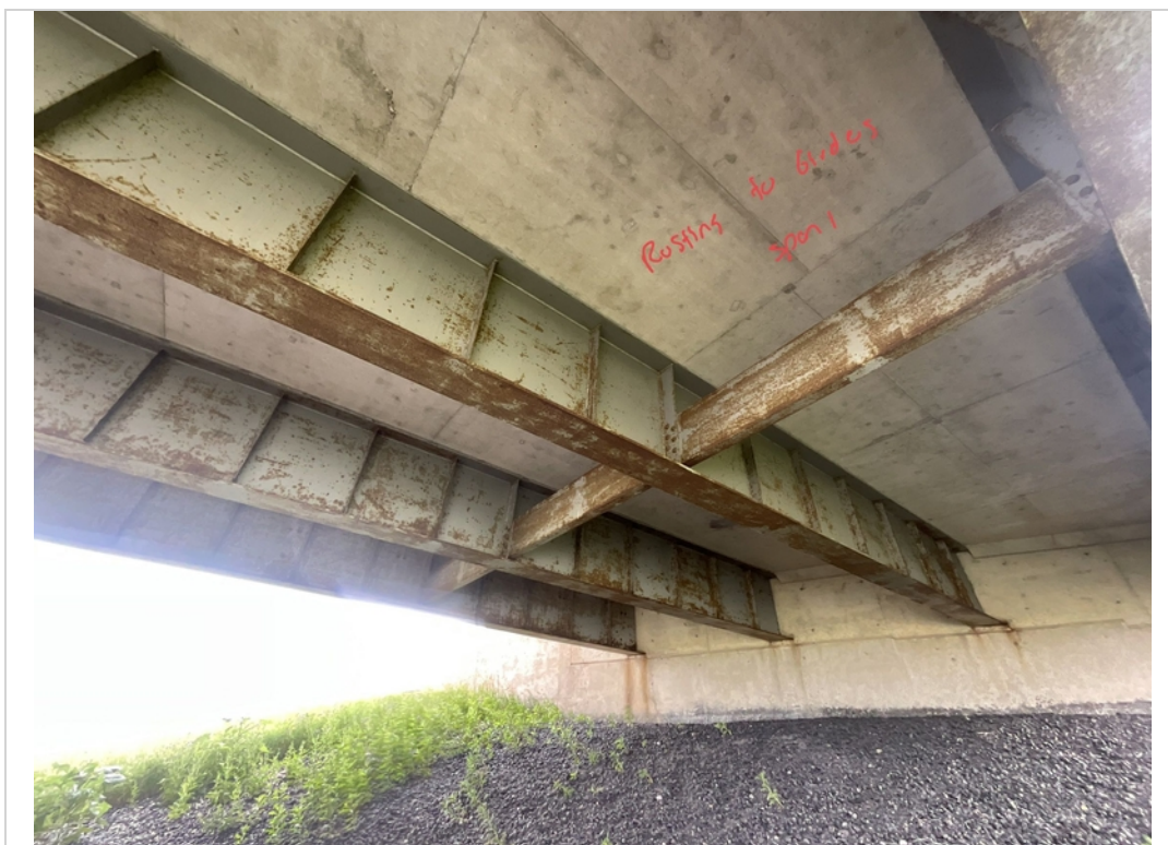
Facing SW. Rusting to Girders in Span 1.
