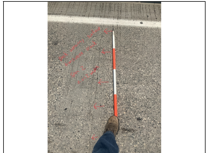
Facing South and Downward. Transverse Crack to Deck Wearing Surface in the EB Lane of Span 2.
