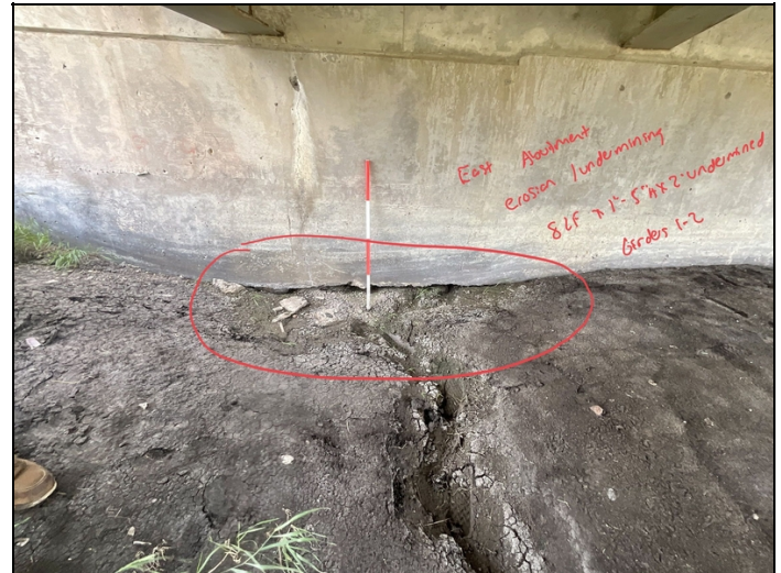
Facing East. Continued Erosion area to East Abutment.
