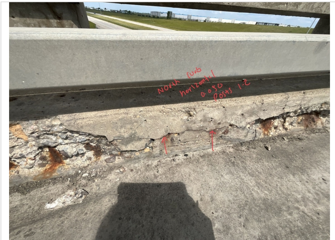
Facing North. Horizontal Crack to Face of North curb from Posts 1-2.
