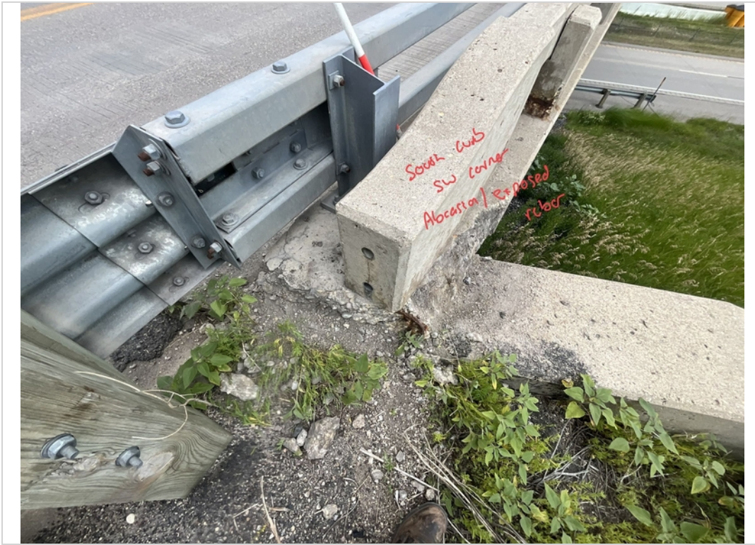
Facing East and Downward. Moderate Abrasion to South Curb at SW Corner.
