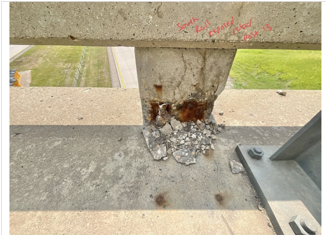
Facing South. South Railing Post 13 with Exposed Rebar.
