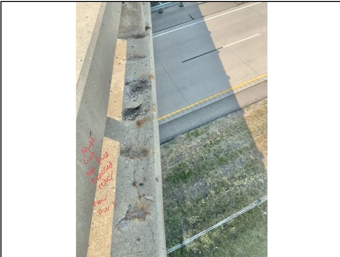
Facing West and Downward. Exposed Rebar to Top of North Curb near Pier 3.
