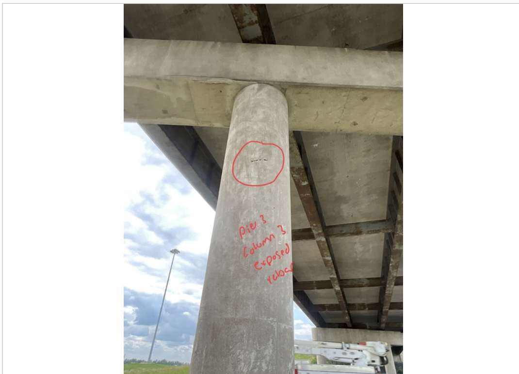
Facing West and Upwards. Exposed Rebar to Pier 3 Column 3.
