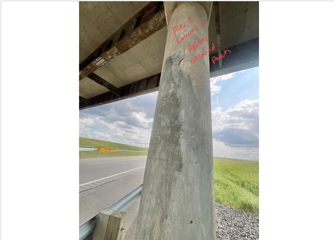
Facing SE and Upwards. Unsound Patch with Delamination to Pier 2 Column 3.
