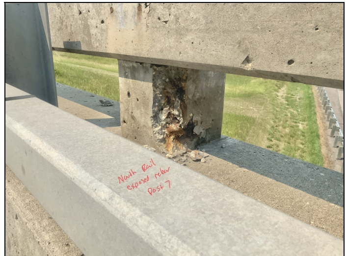
Facing NW. Spalling with Exposed Rebar to North Rail Post 7.
