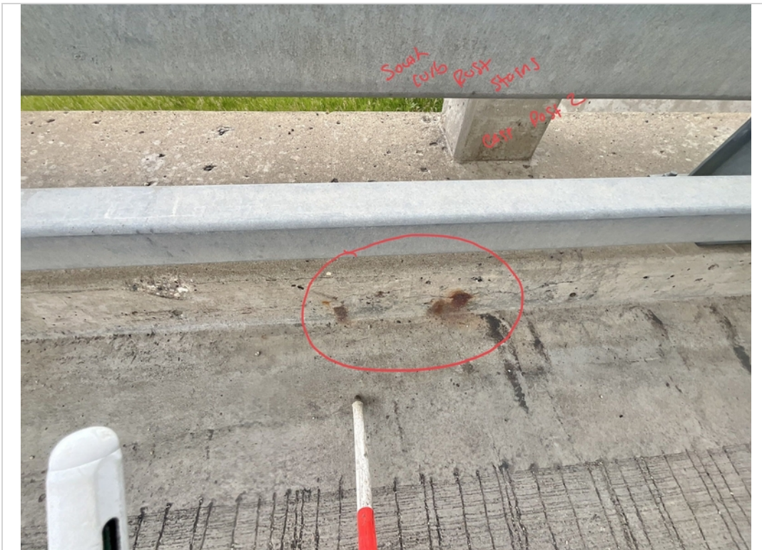
Facing South and Downward. Rust stains to South Curb.
