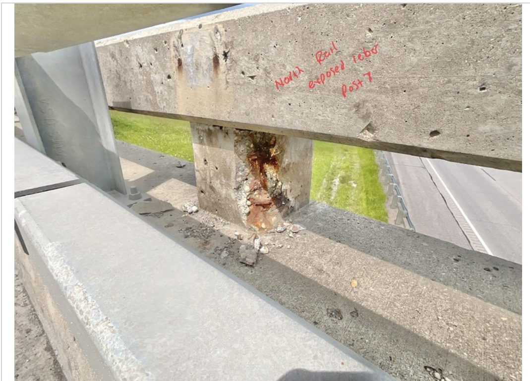
Facing NW. Exposed Rebar to North Railing at Post 7.
