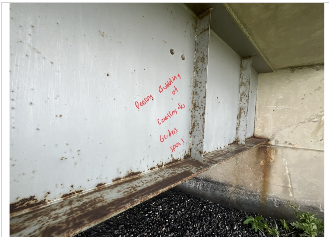
Facing SW. Peeling of Coating to Girder 1 in Span 1 near West End.
