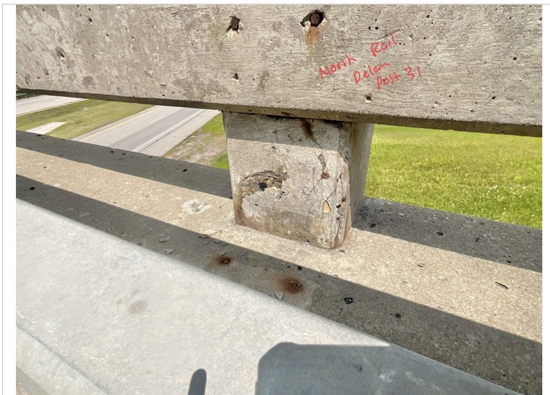
Facing North. Delamination to North Railing Post 31.
