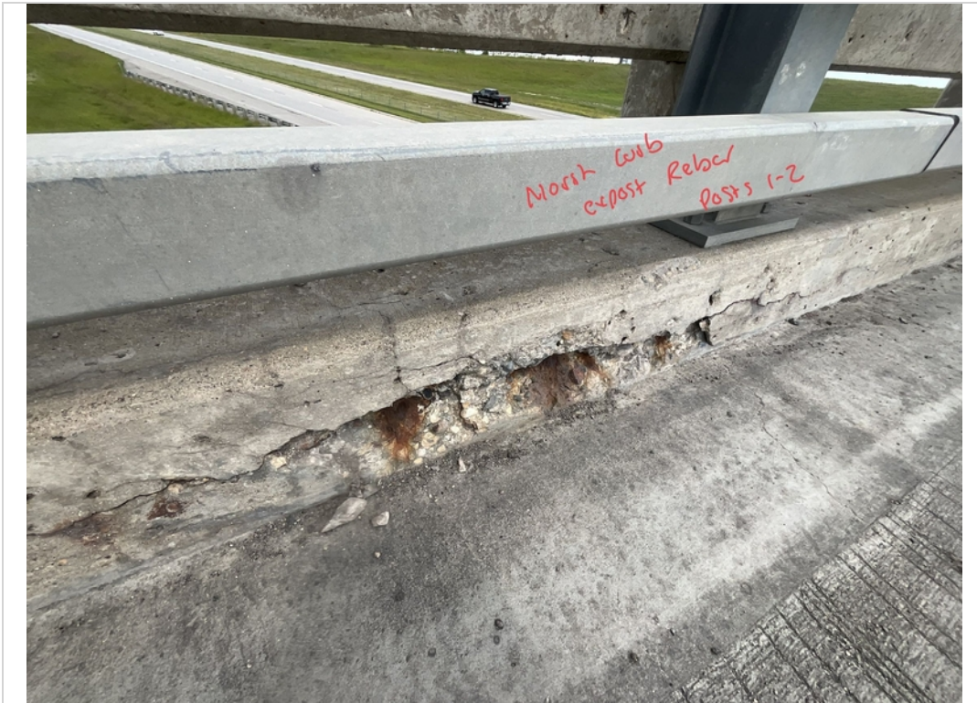
Facing NE. Spalling with Exposed Rebar to Face of North Curb from Posts 1-2.
