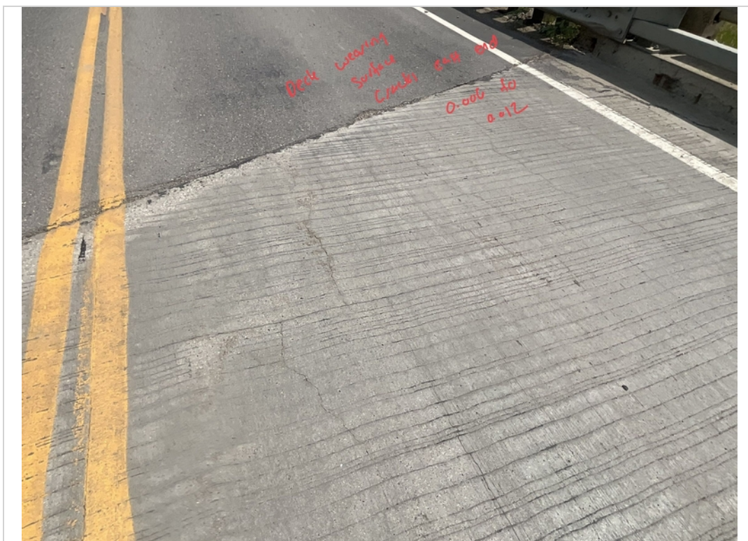
Facing East and Downward. Minor Area of various Cracks to Deck Wearing Surface East End.
