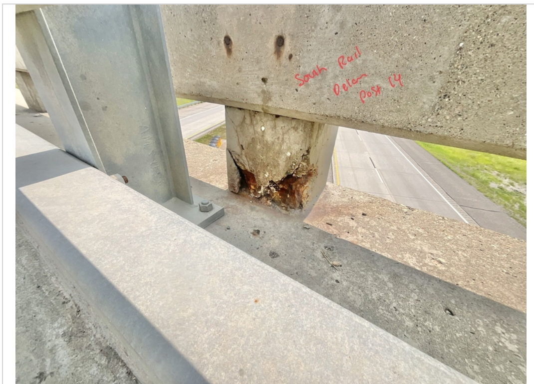
Facing SE. Delamination to South Railing Post 14.
