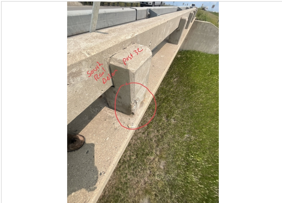
Facing NE. Delamination to South Railing at Post 32
