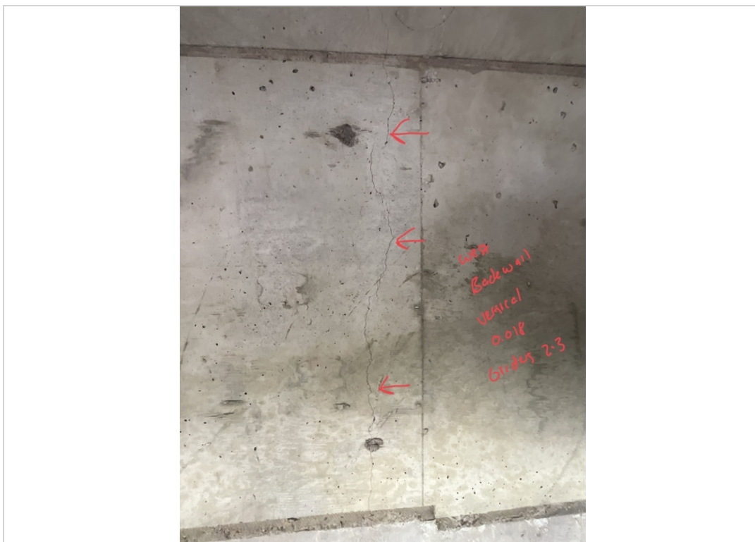
Facing West. Vertical Crack to West Backwall in-between Girders 2 and 3.
