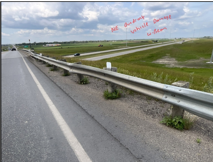
Facing NW. Vehicle Impact Damage to NE W-Beam.
