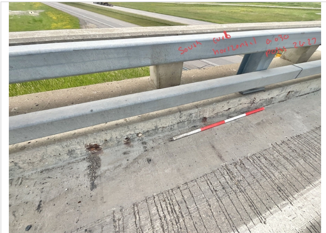
Facing SW and Downward. Continued Horizontal Crack to Face of South Curb from Posts 26-27.
