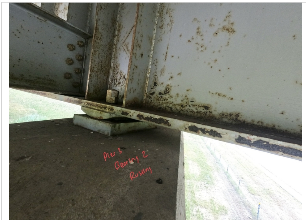
Facing SE. Pier 3 Bearing 2 Rusting.
