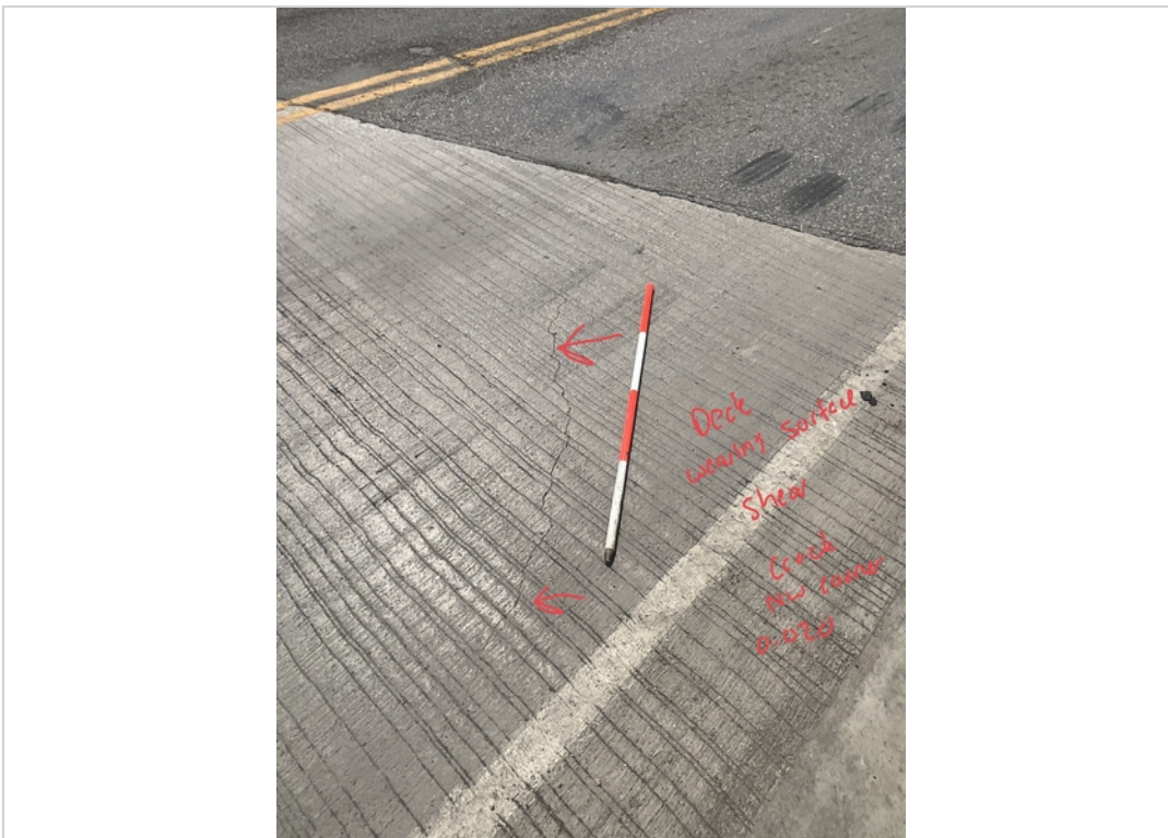
Facing SW and Downward. Shear Cracks to Deck Wearing Surface NW Corner.
