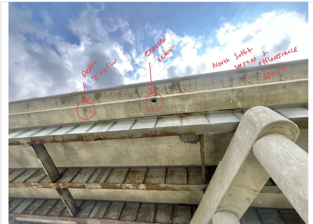
Facing South and Upwards. Delamination and Exposed Rebar to North Soffit in Span 3.
