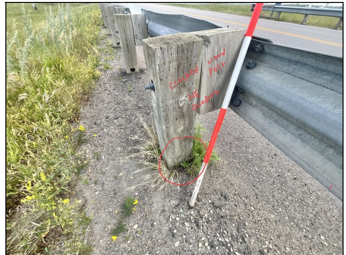
Facing East. Cracked Wood Post within NE Quadrant.
