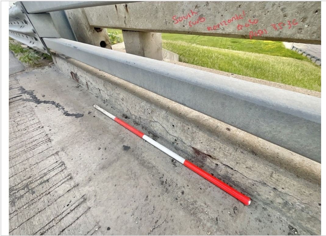
Facing SE. Horizontal Cracks to Face of South Curb from Posts 35-36.
