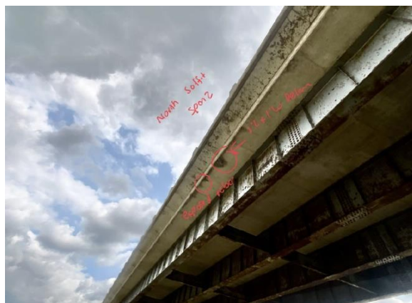
Figure 8. 29-69.374 Underside of Deck Girder Rust and Exposed Rebar
