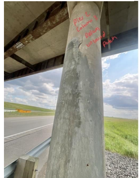
Figure 3. 29-69.374 Column Delamination
