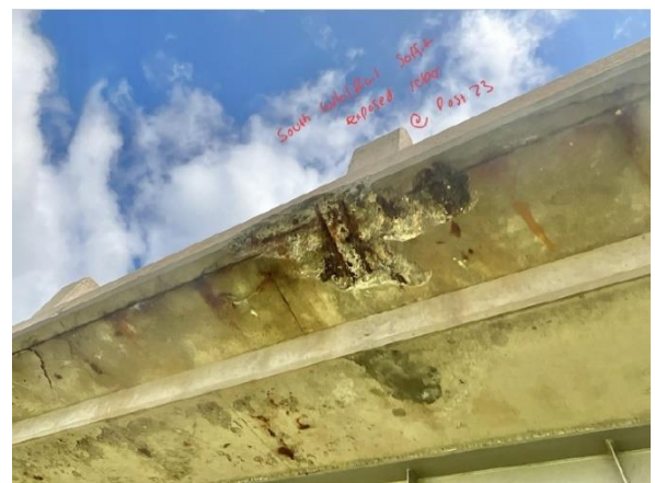
Figure 4. 29-69.374 N Curb/Rail Soffit Exposed Rebar
