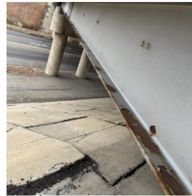
Figure 12. Concrete Buckling - I-94 Exit 152
