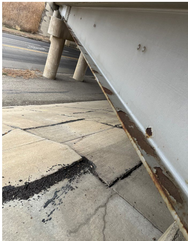
FIGURE 13: PAINT CONDITION OF THE SOUTH FASCIA BEAM OF THE WESTBOUND BRIDGE (11/9/2022)
