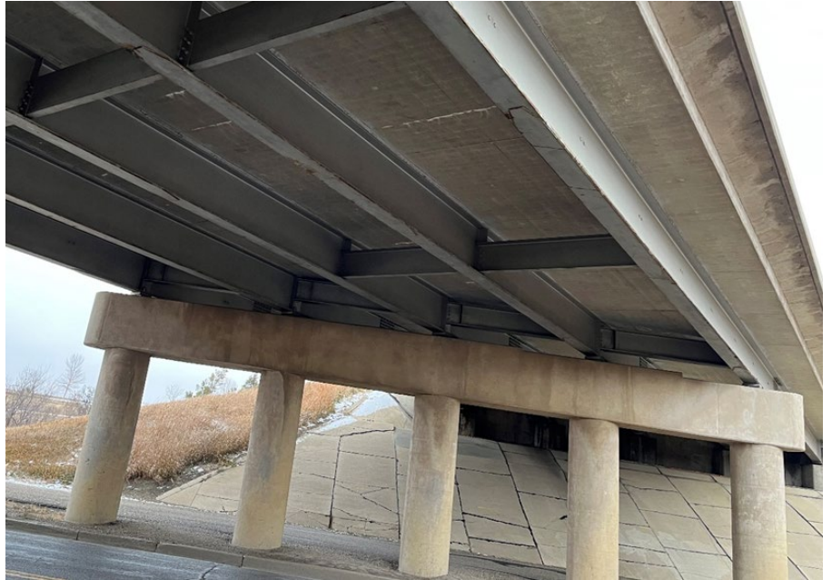
FIGURE 12: TRANVERSE CRACKS WITH EFFLORESCENCE ON THE UNDERSIDE OF THE DECK (11/9/2022)
