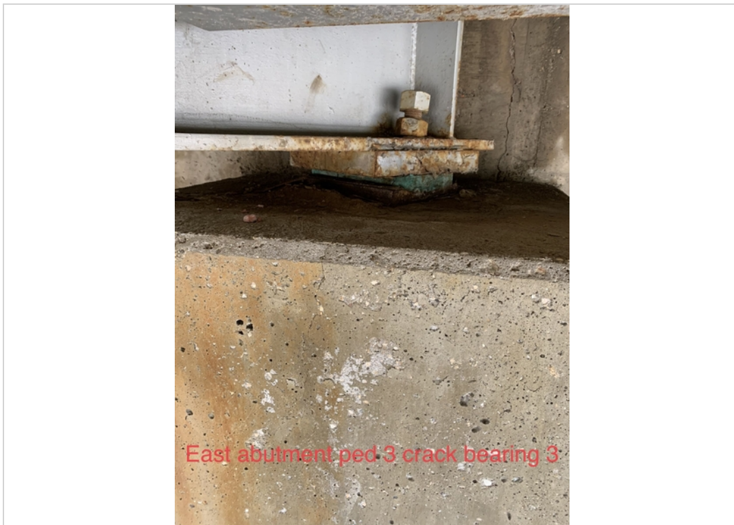
East abutment ped 3 bearing 3
