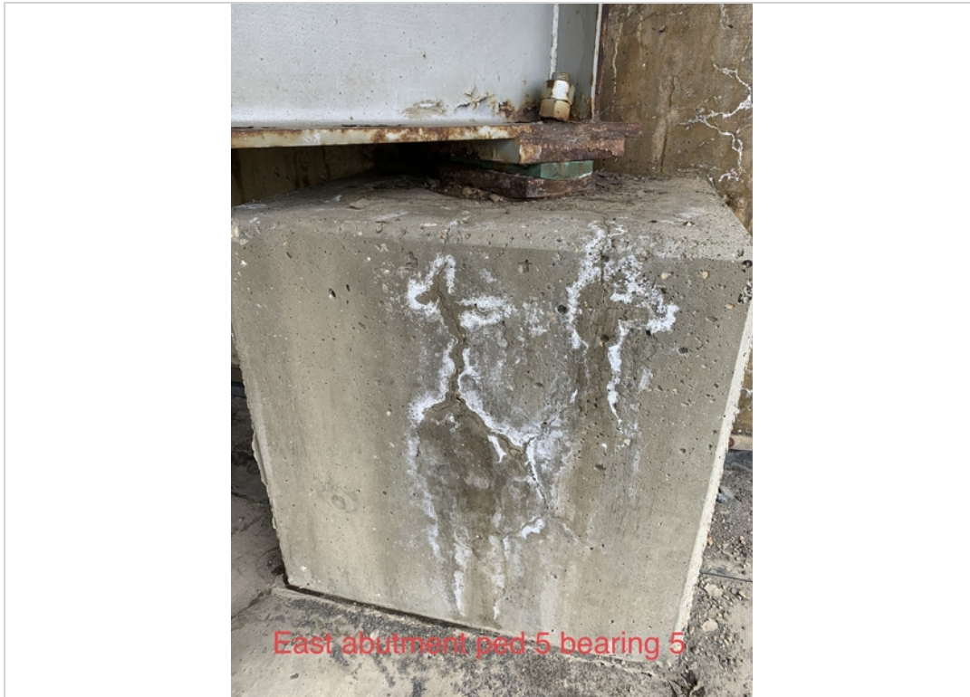
East abutment ped 5 bearing 5
