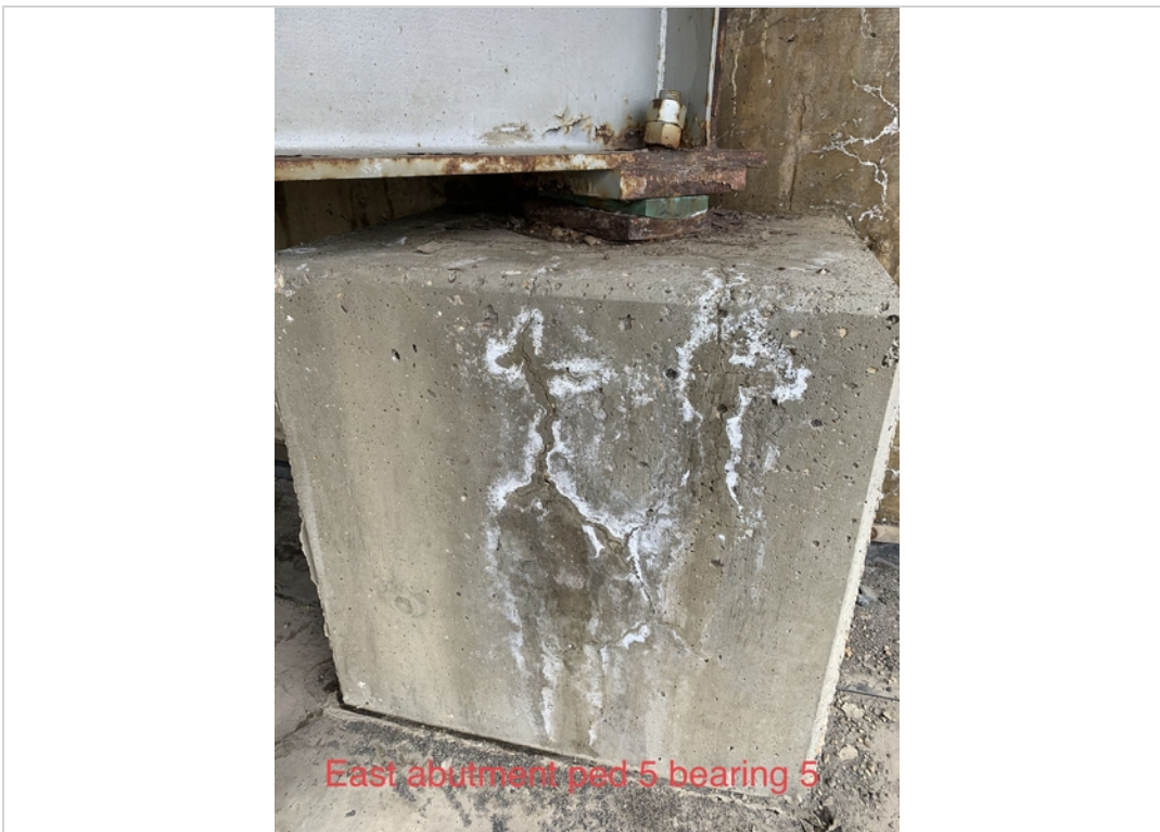
East abutment pad 5 bearing 5
