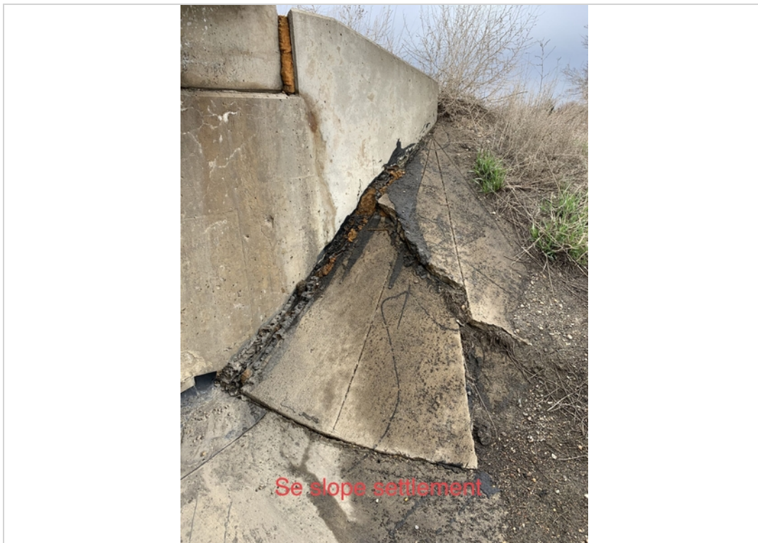
SE slope protection settlement
