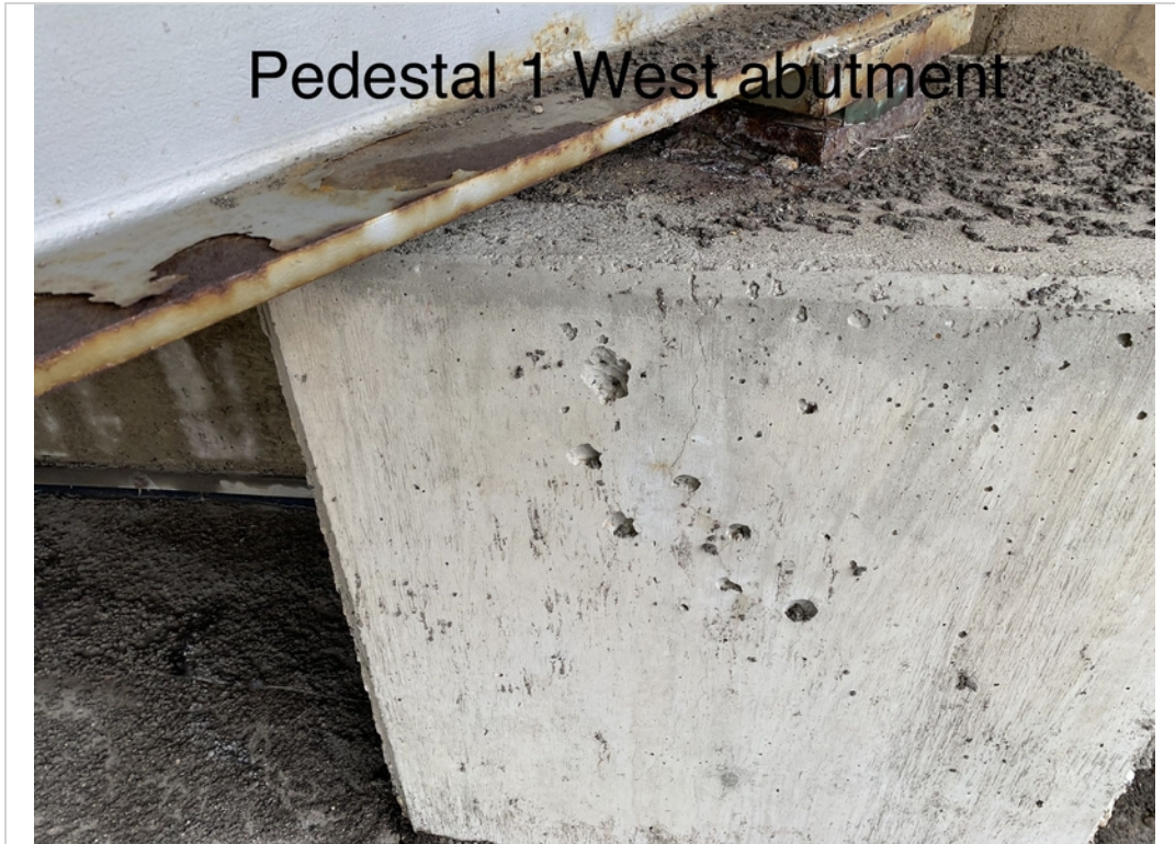
Ped 1 west abutment crack
