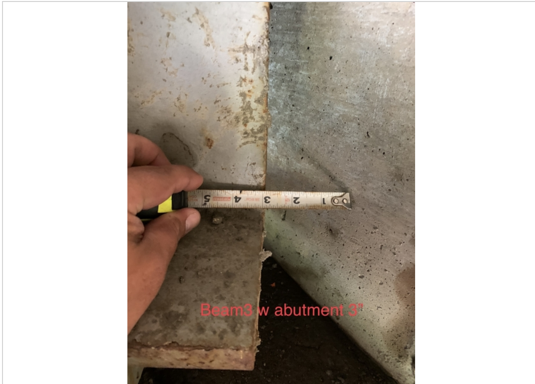
Beam 3 west abutment 3"
