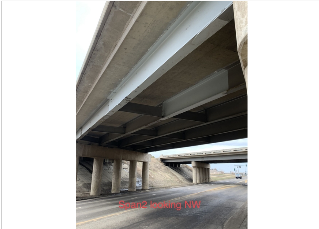
Span2 looking NW
