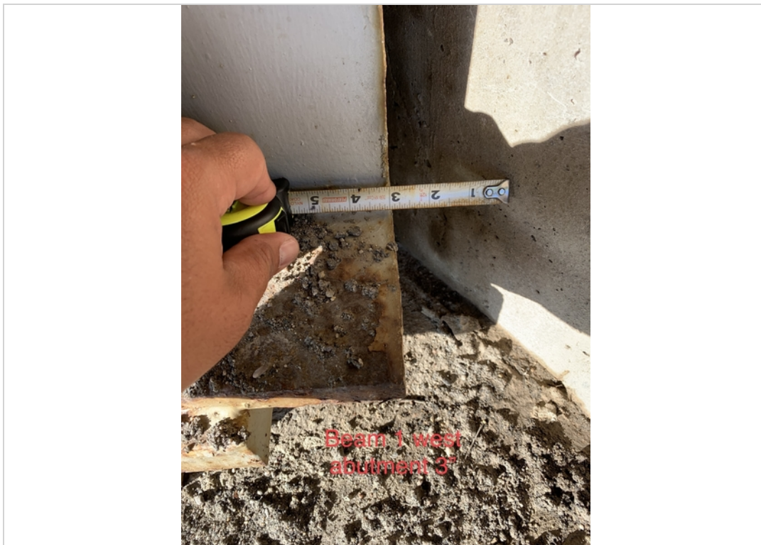
Beam 1 west abutment 3"
