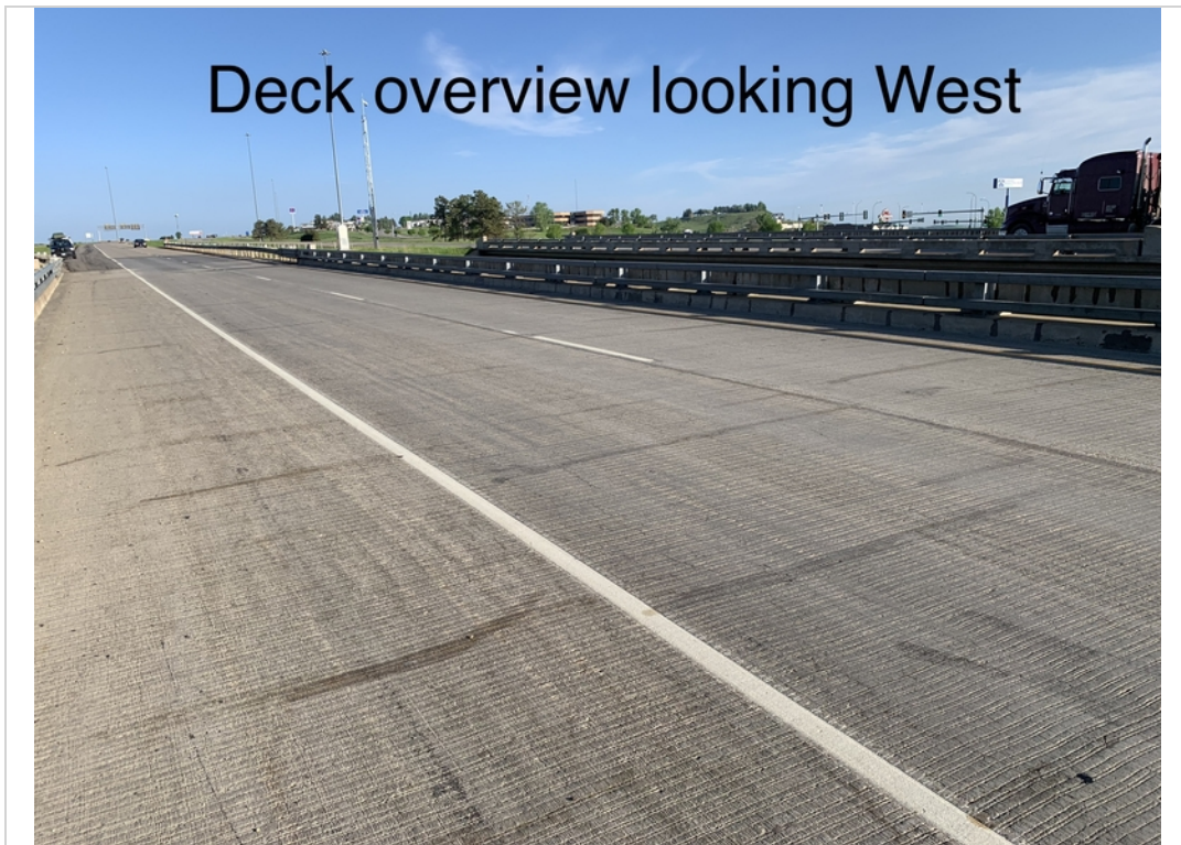
Deck view looking west
