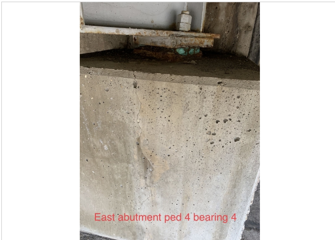
East abutment ped 4 bearing 4
