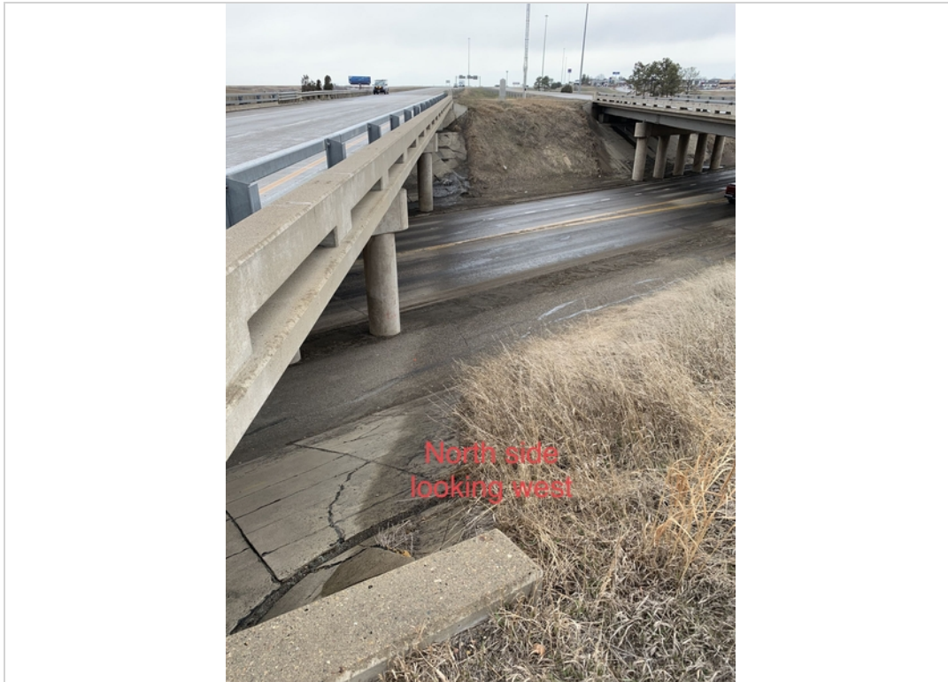
North side looking west
