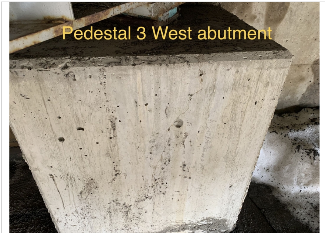
Ped 3 west abutment crack
