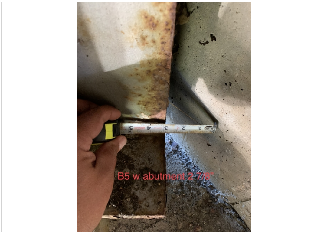
Beam 5 west abutment 2 7/8"
