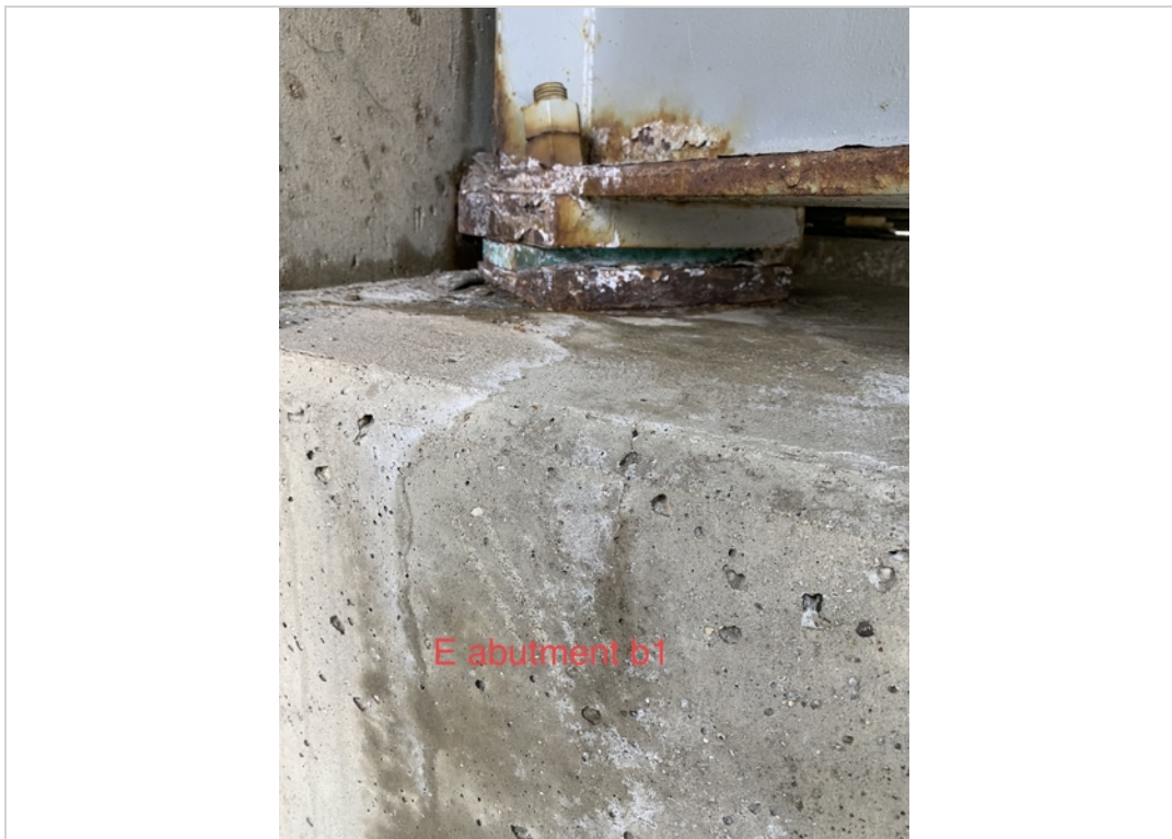
East abutment bearing 1
