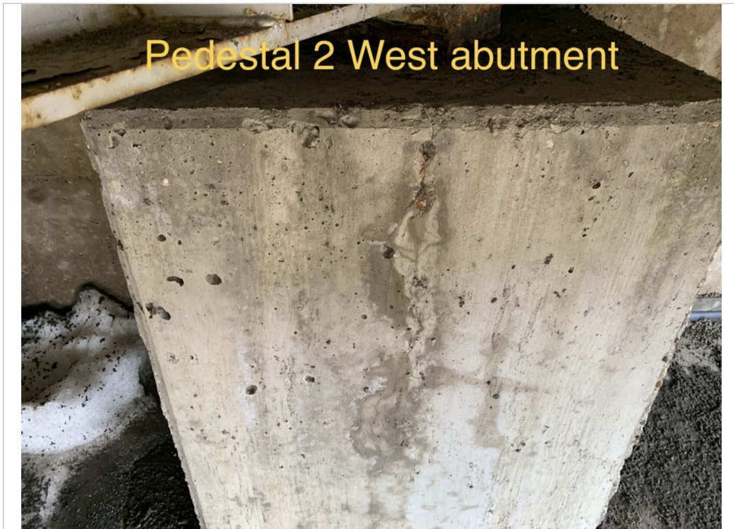
Ped 2 west abutment
