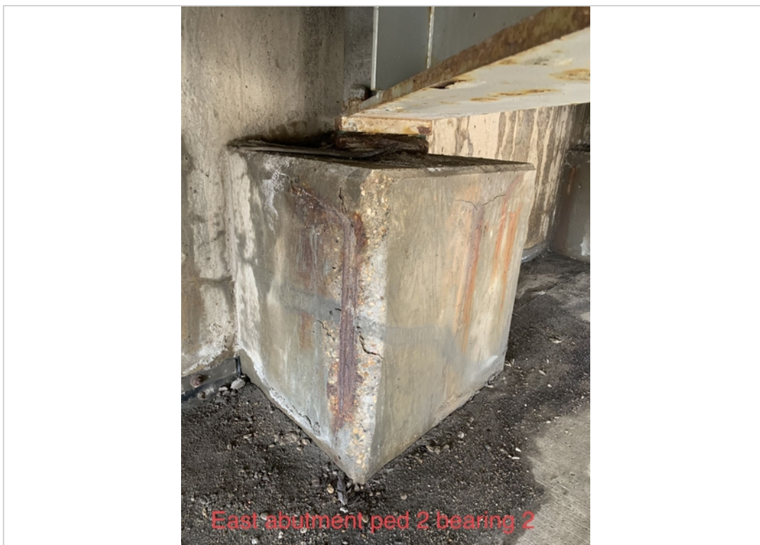
East abutment ped 2 exposed rebar and bearing 2
