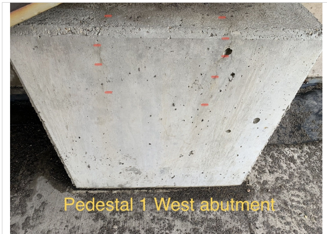
Ped 1 west abutment cracks
