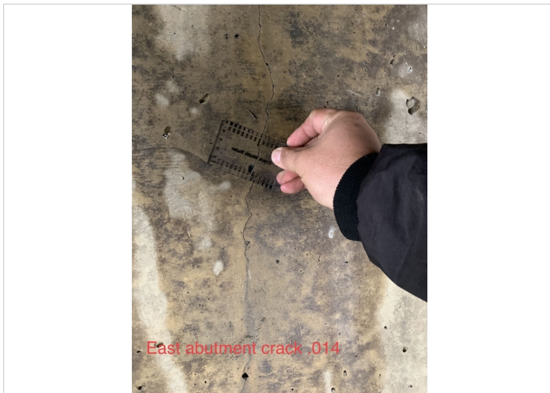
East abutment crack .014
