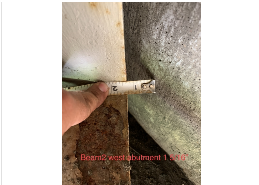
Beam 2 west abutment 1 5/16"
