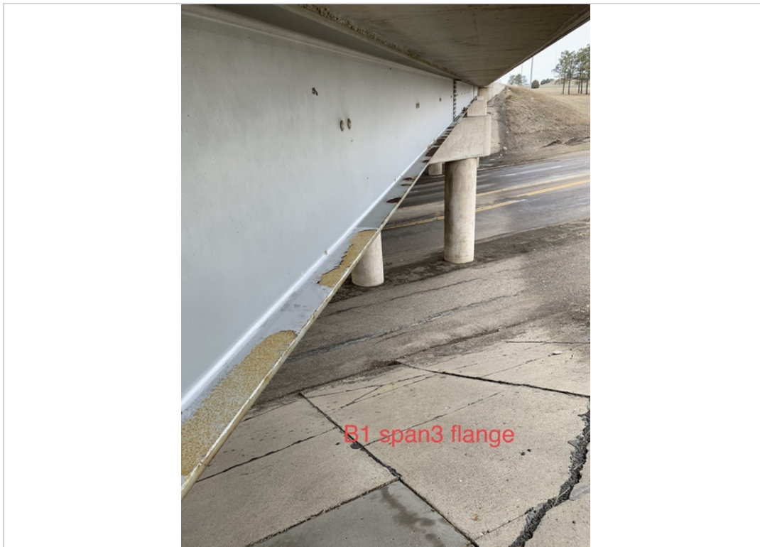
Beam 1 span 3 flange corrosion
