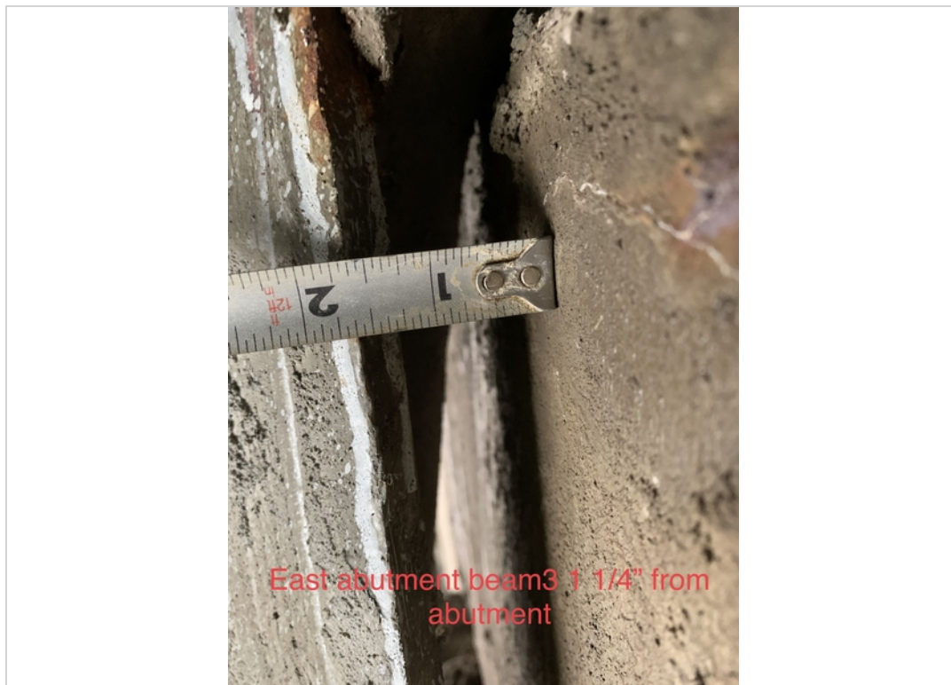
East abutment beam 4 , 1 1/4"from abutment
