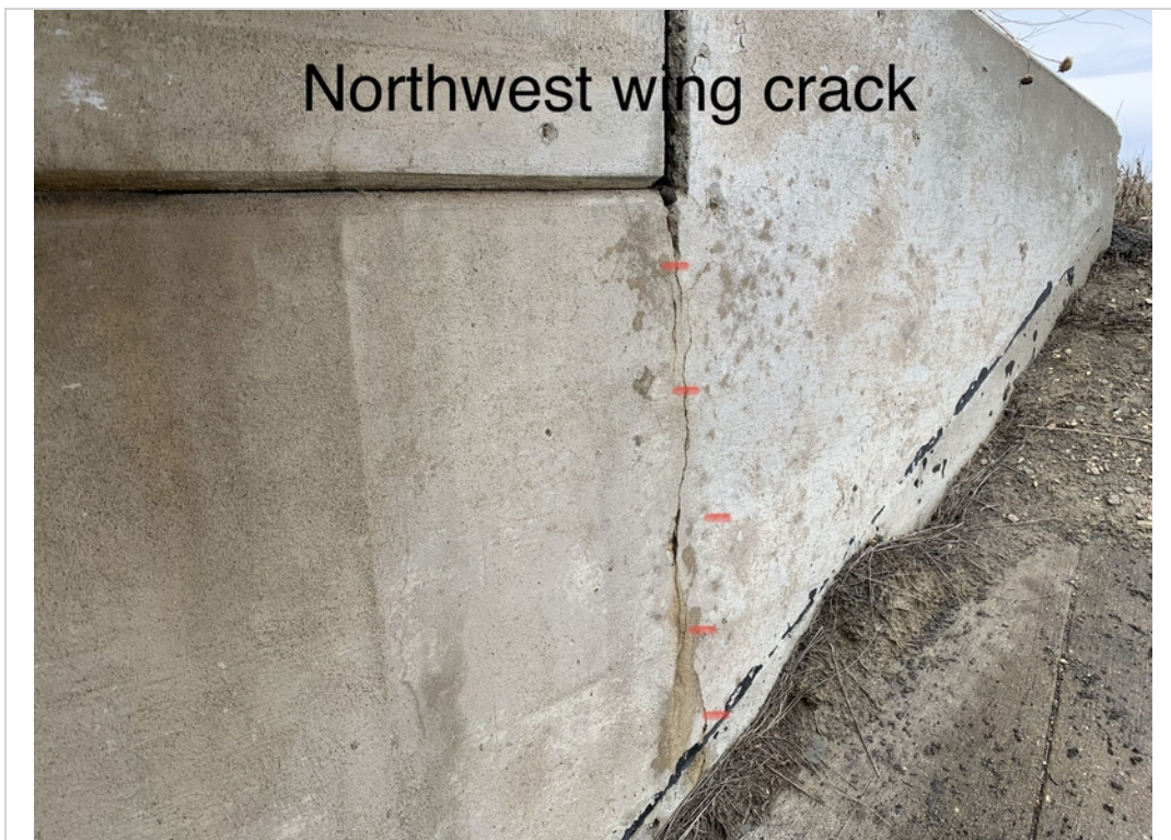
NW wing crack
