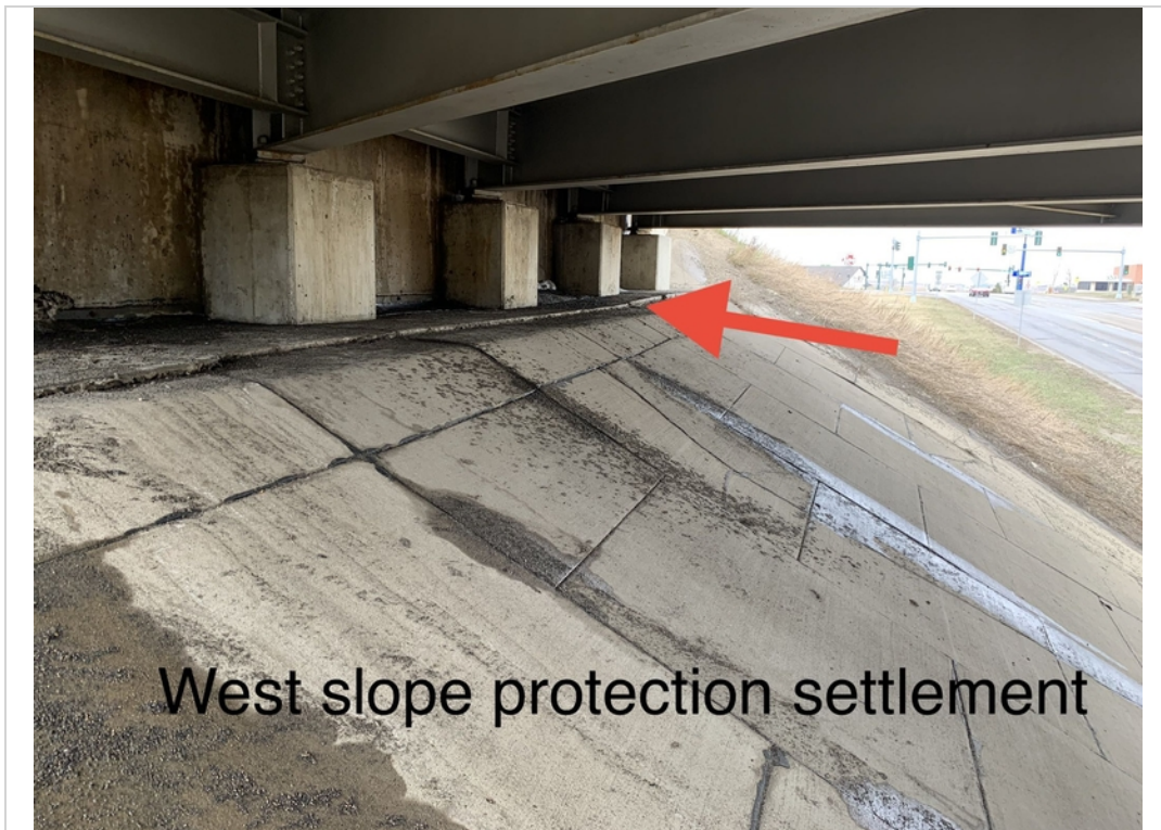
West slope protection settlement
