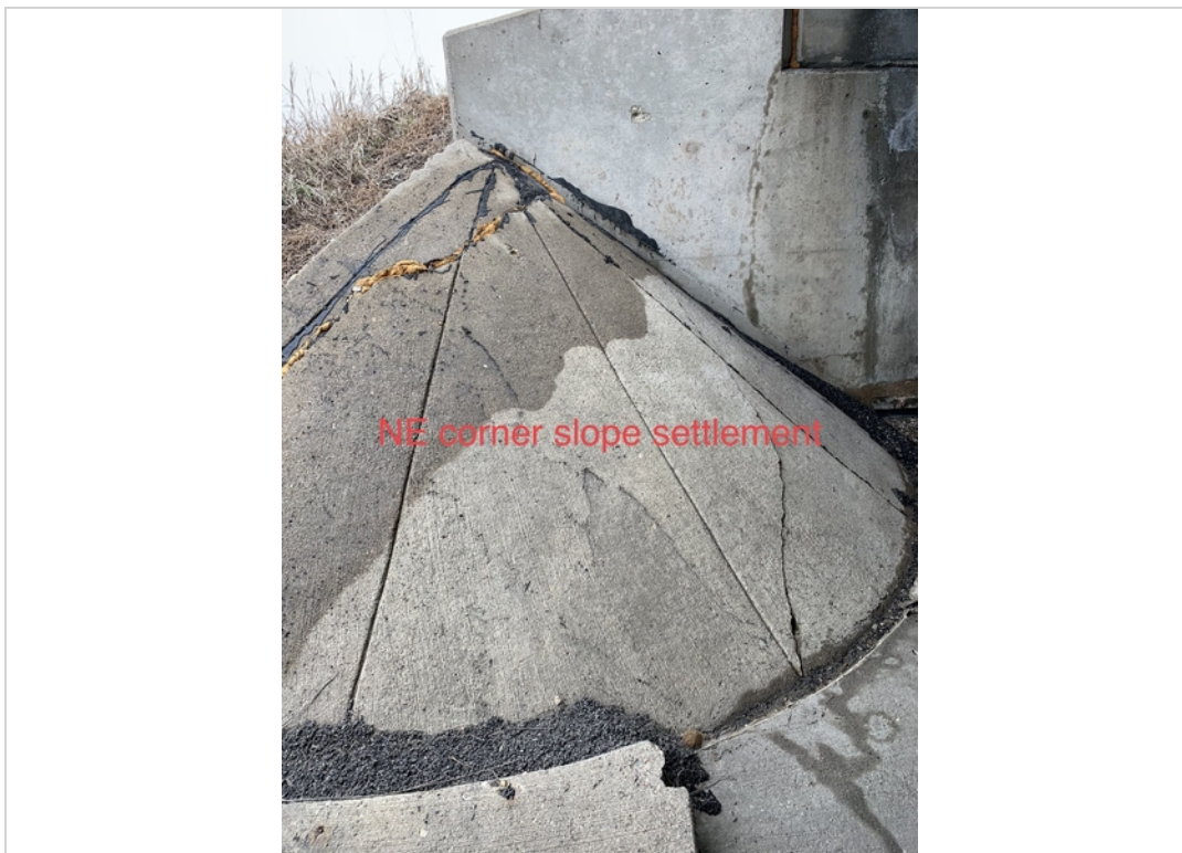
NE corner slope protection settlement
