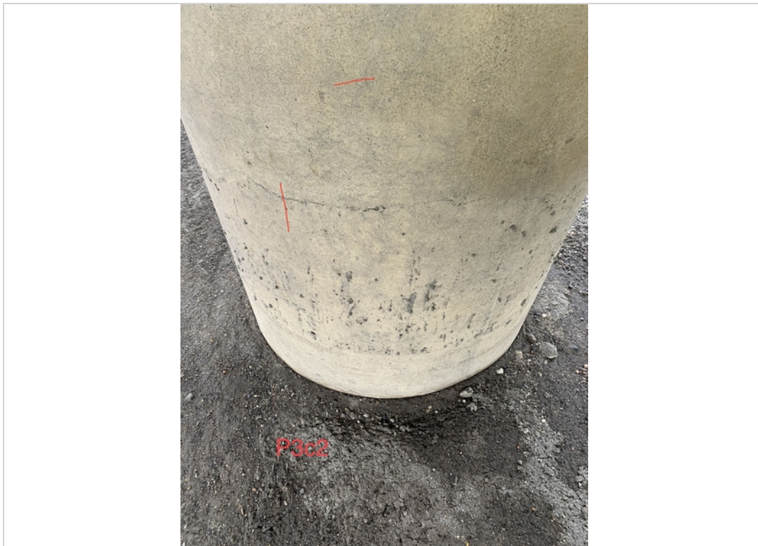
Pier 3 column 2 cracks
