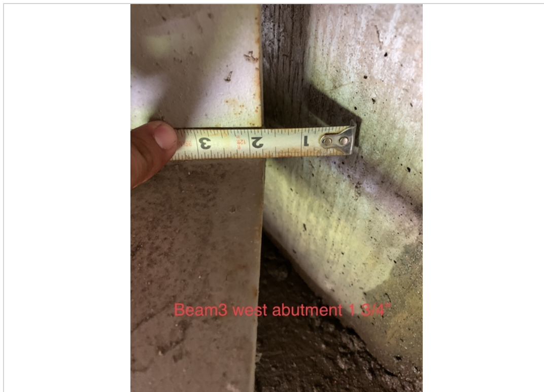
Beam 3 west abutment 1 3/4"
