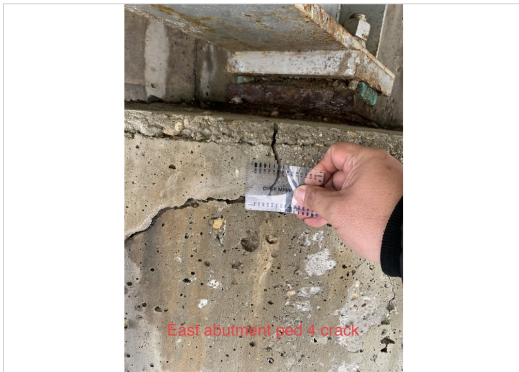
East abutment pier 4 crack
