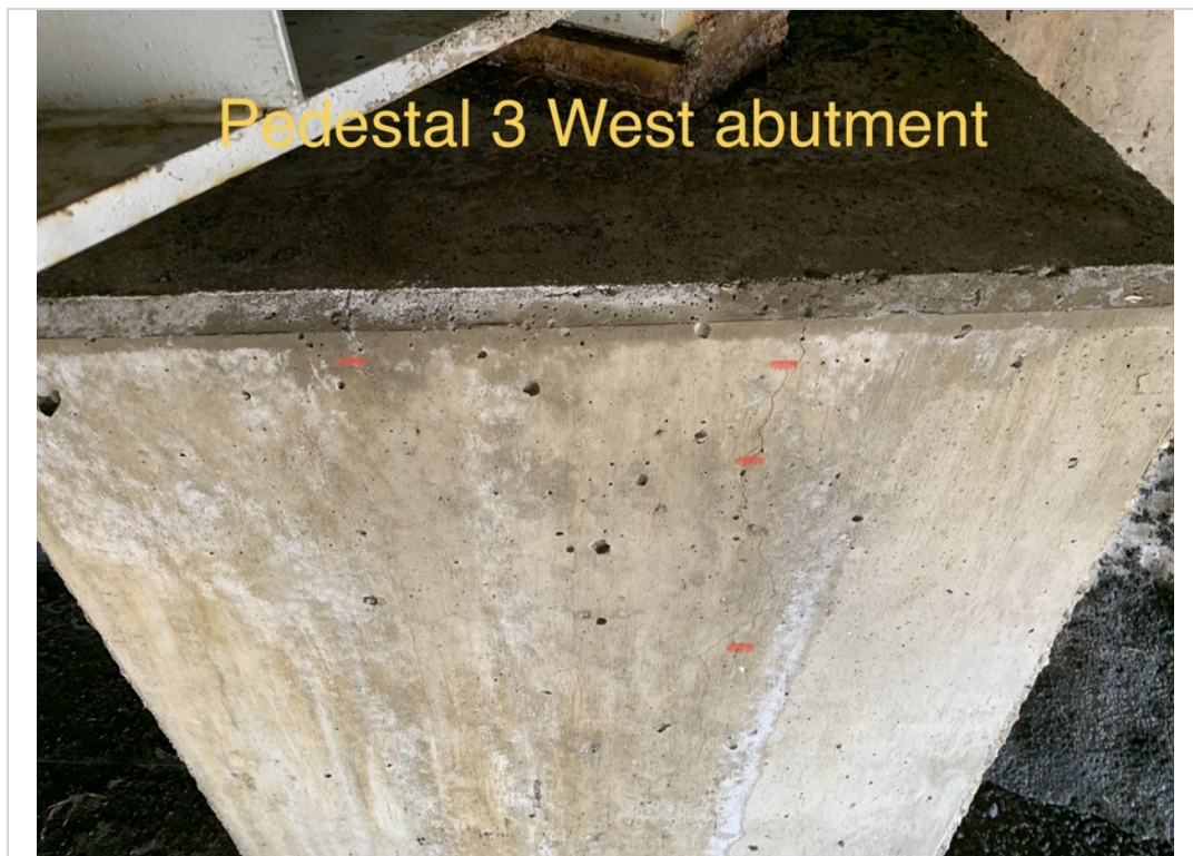
Ped 3 crack west abutment
