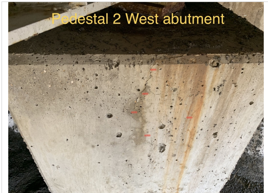
Ped 2 west abutment crack
