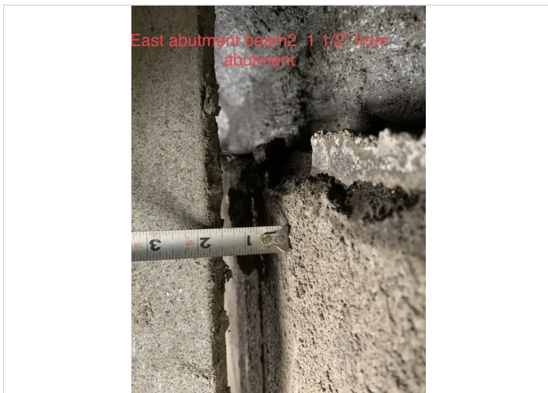
East abutment beam 2 , 1 1/2" from abutment
