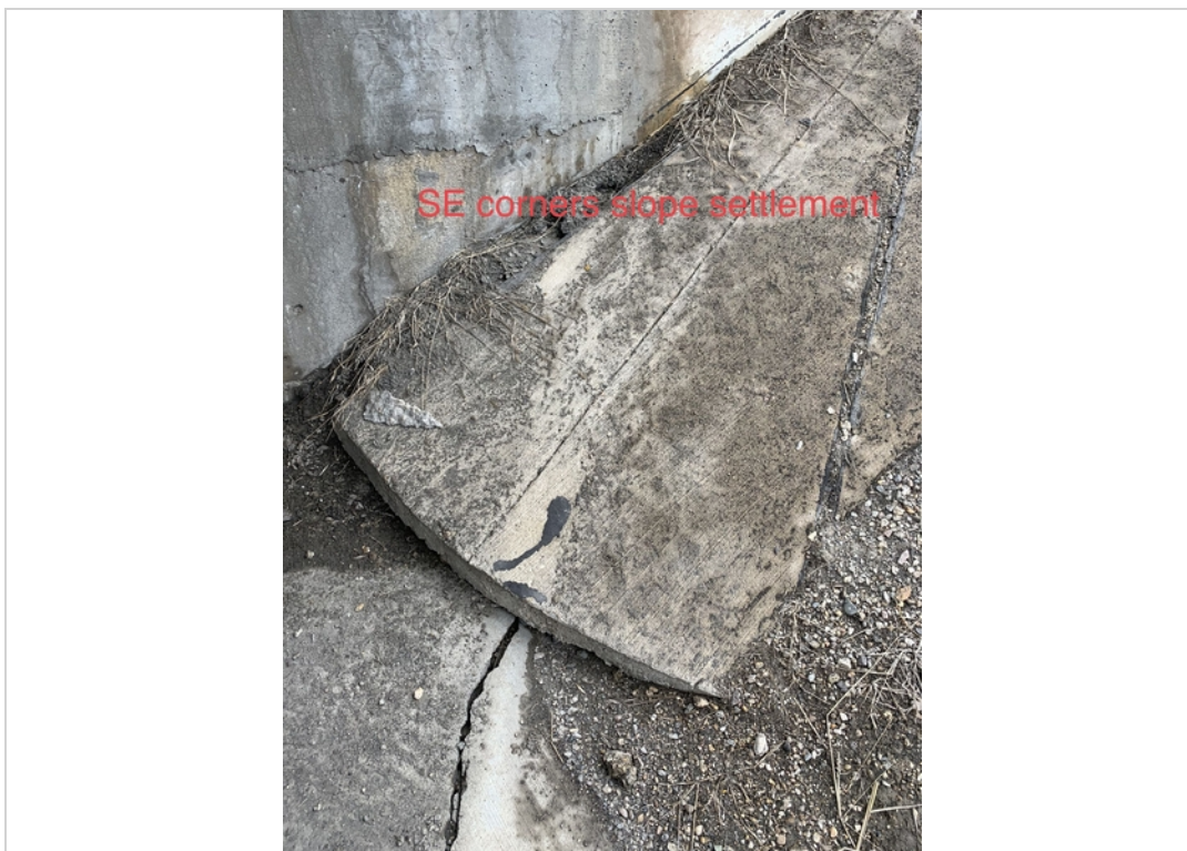
SE corner slope protection settlement
