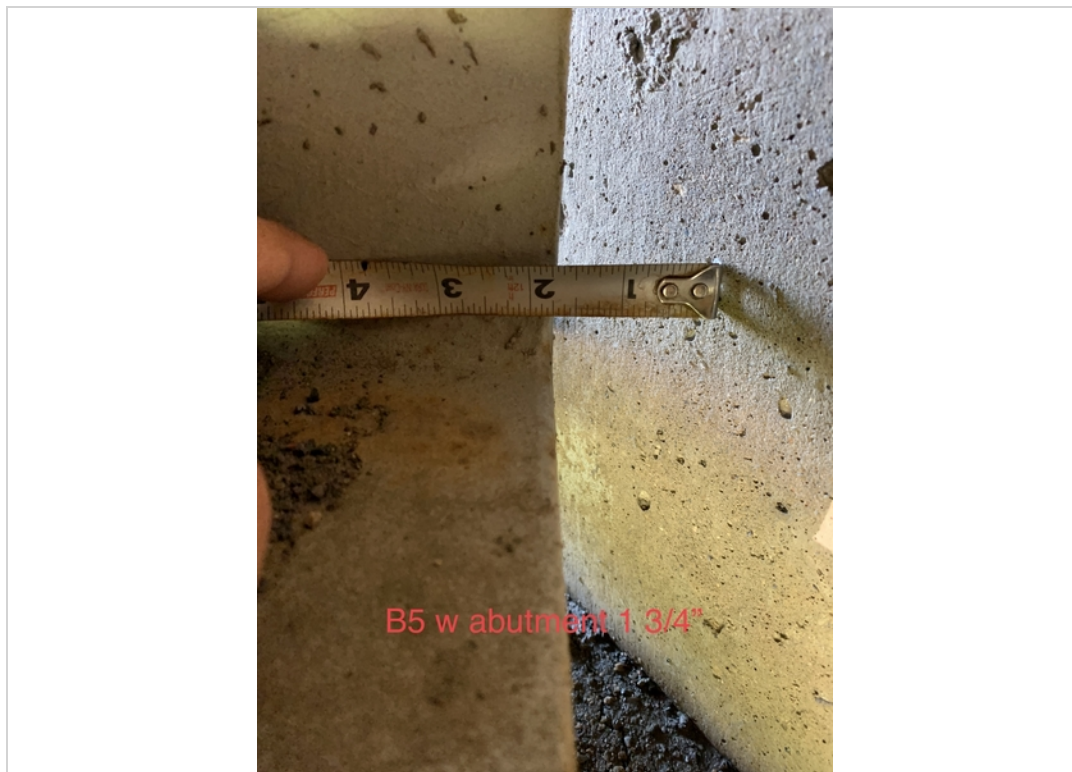
Beam5 west abutment 1 3/4"
