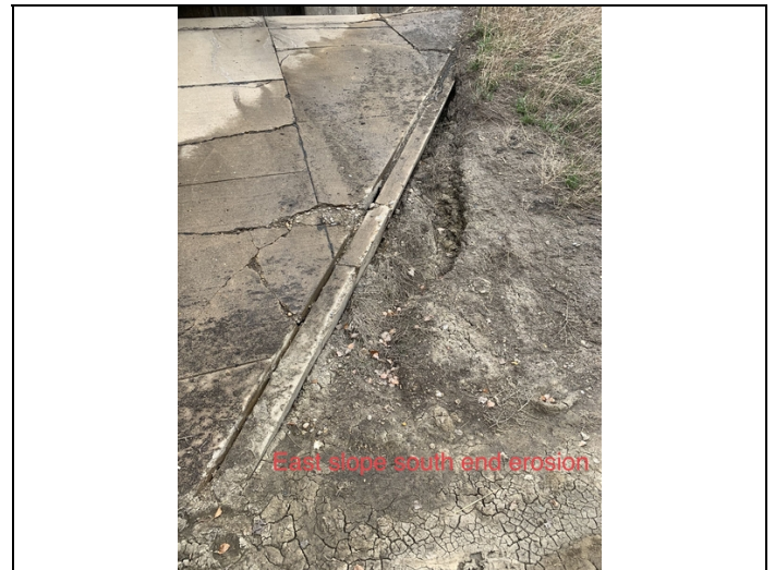
East slope south end erosion
