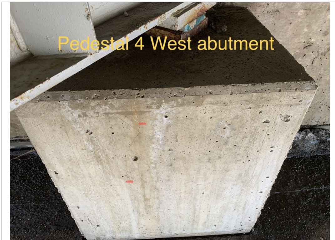
Ped 4 crack west abutment
