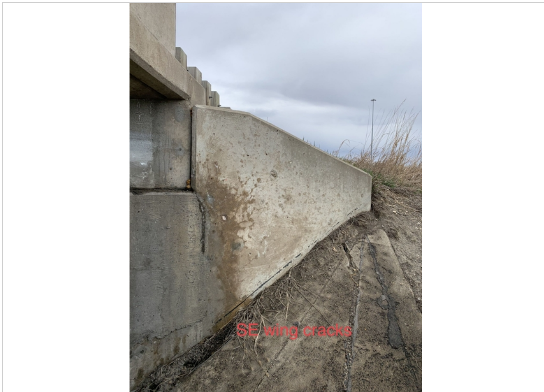
SE wing cracks
