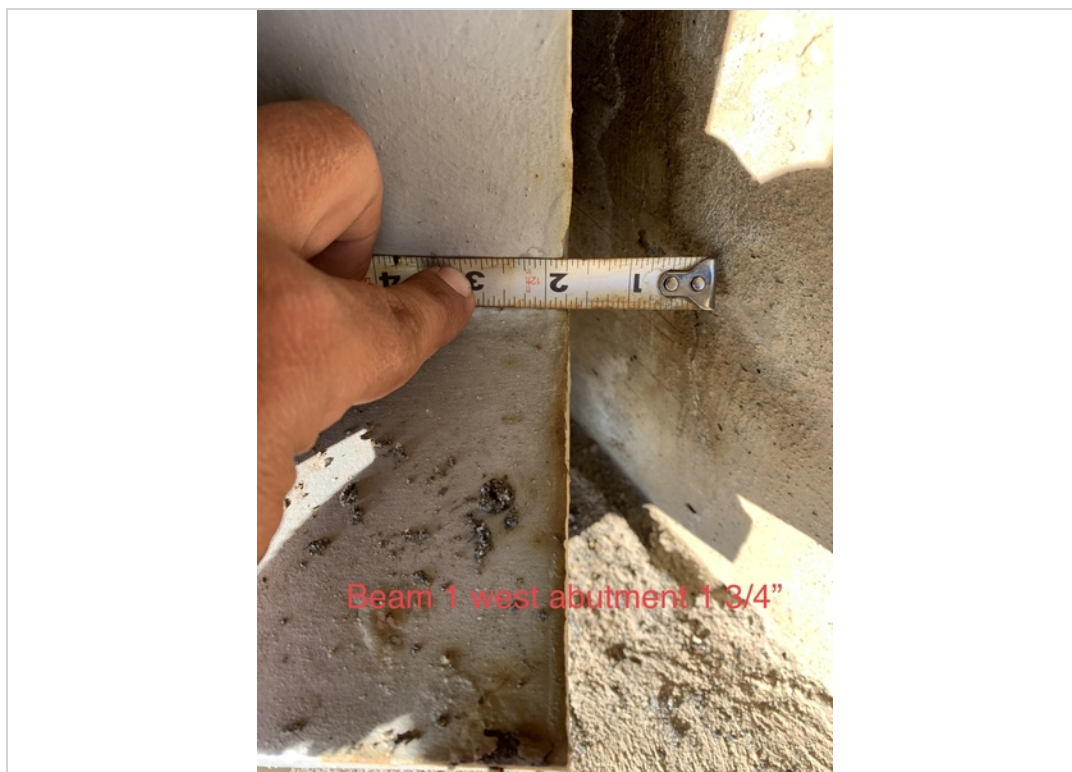
Beam 1 west abutment 1 3/4"
