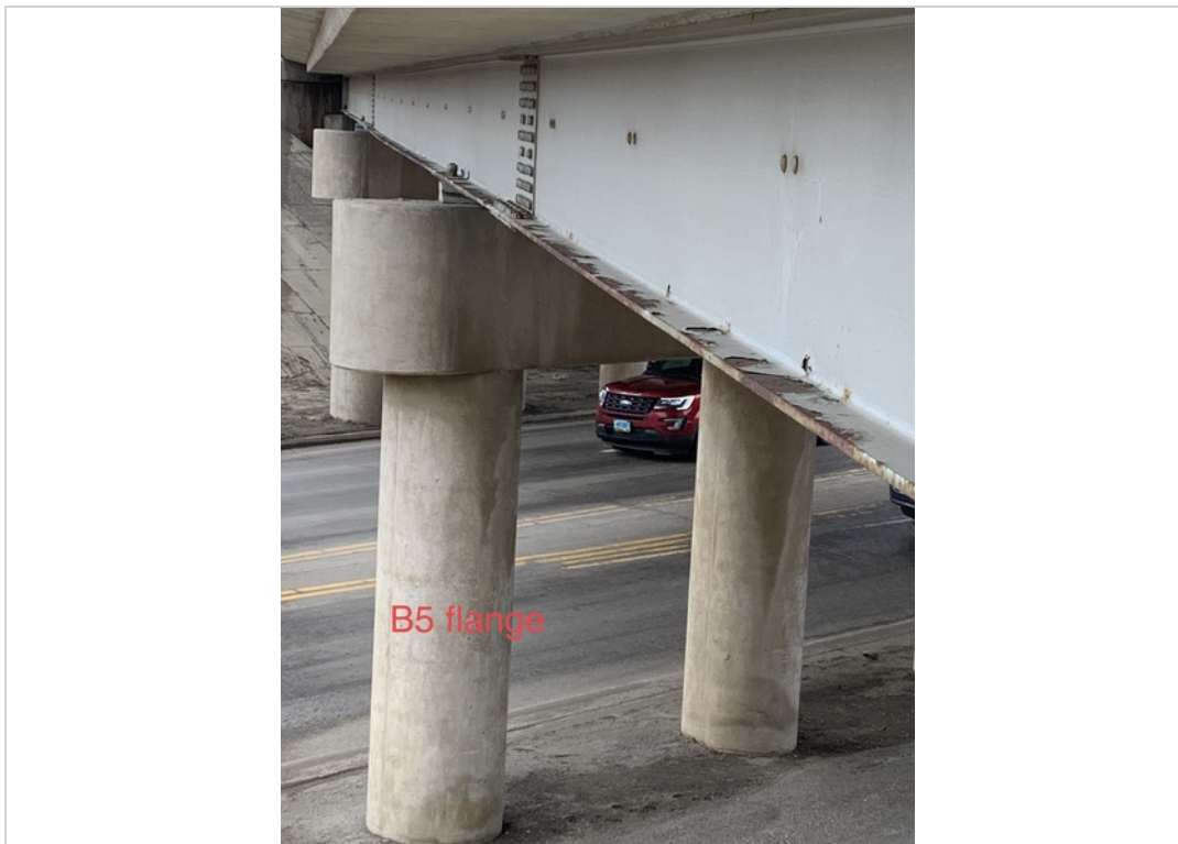
Beam 5 flange corrosion
