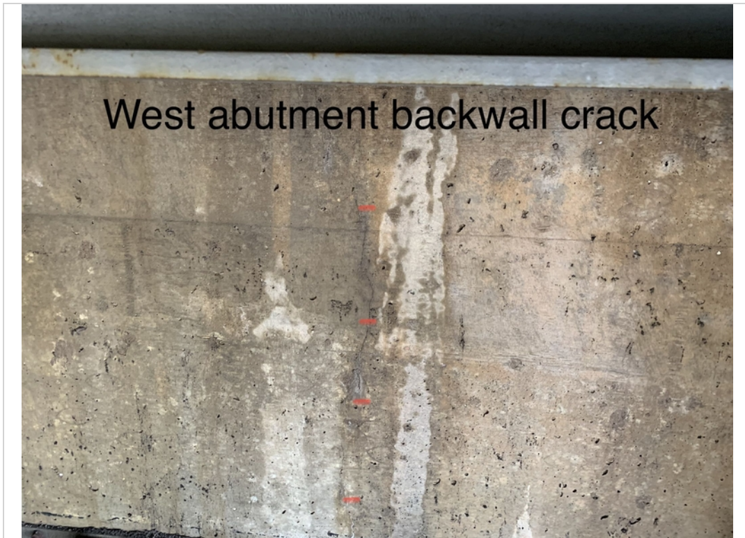
West abutment backwall crack
