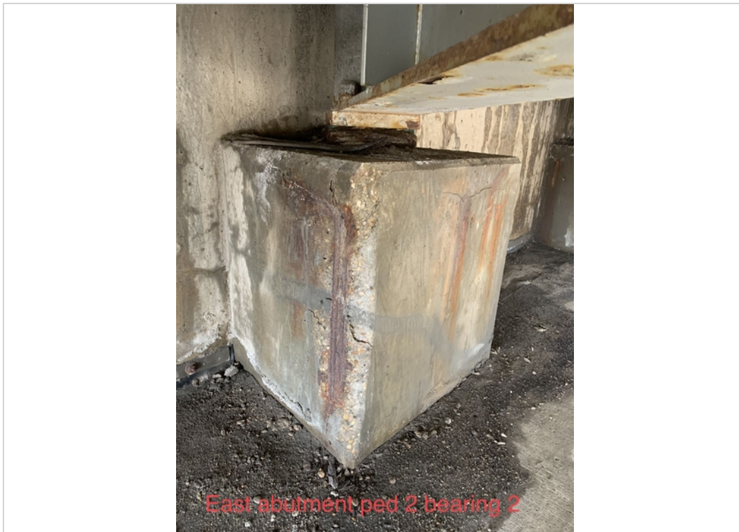
East abutment ped 2 exposed rebar and bearing 2
