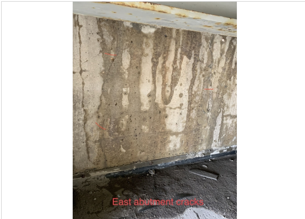
East abutment cracks
