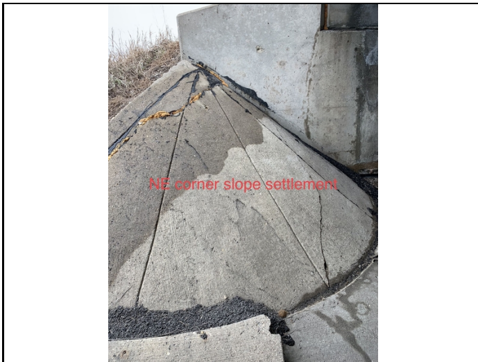
NE corner slope protection settlement
