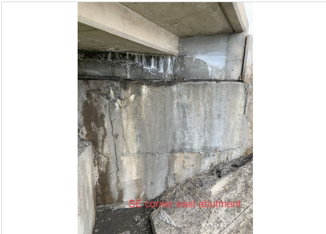
SE corner east abutment cracks efflorescence
