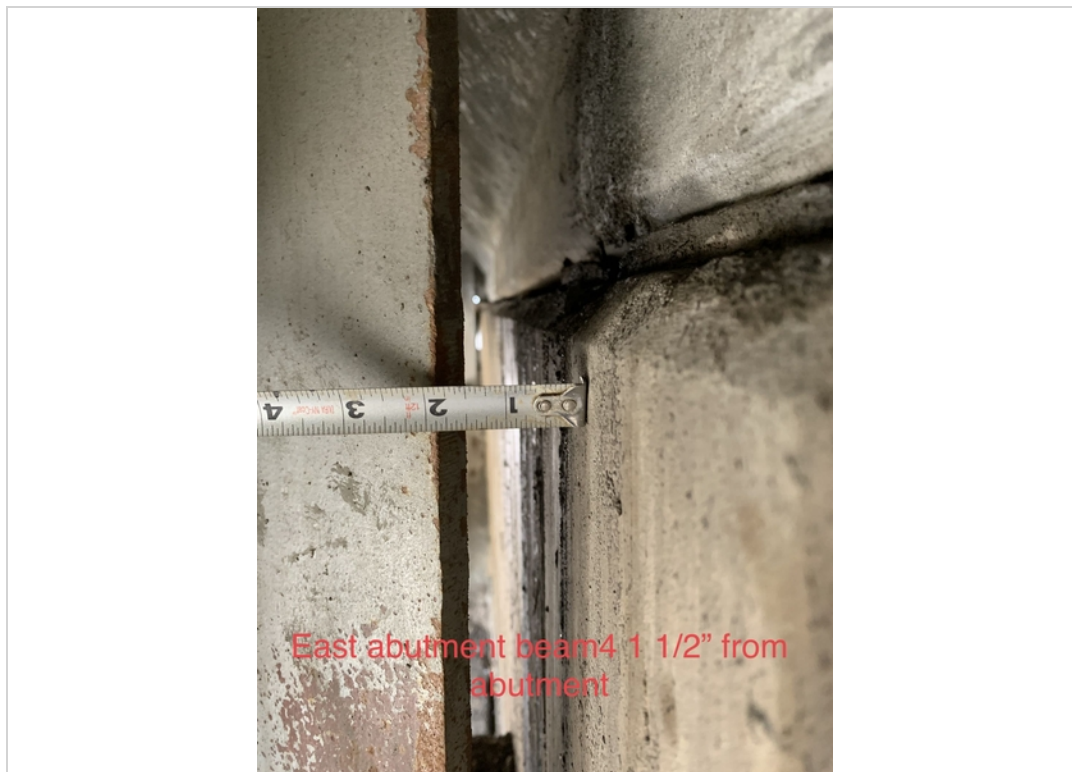
East abutment beam 4 , 1 1/2" from abutment
