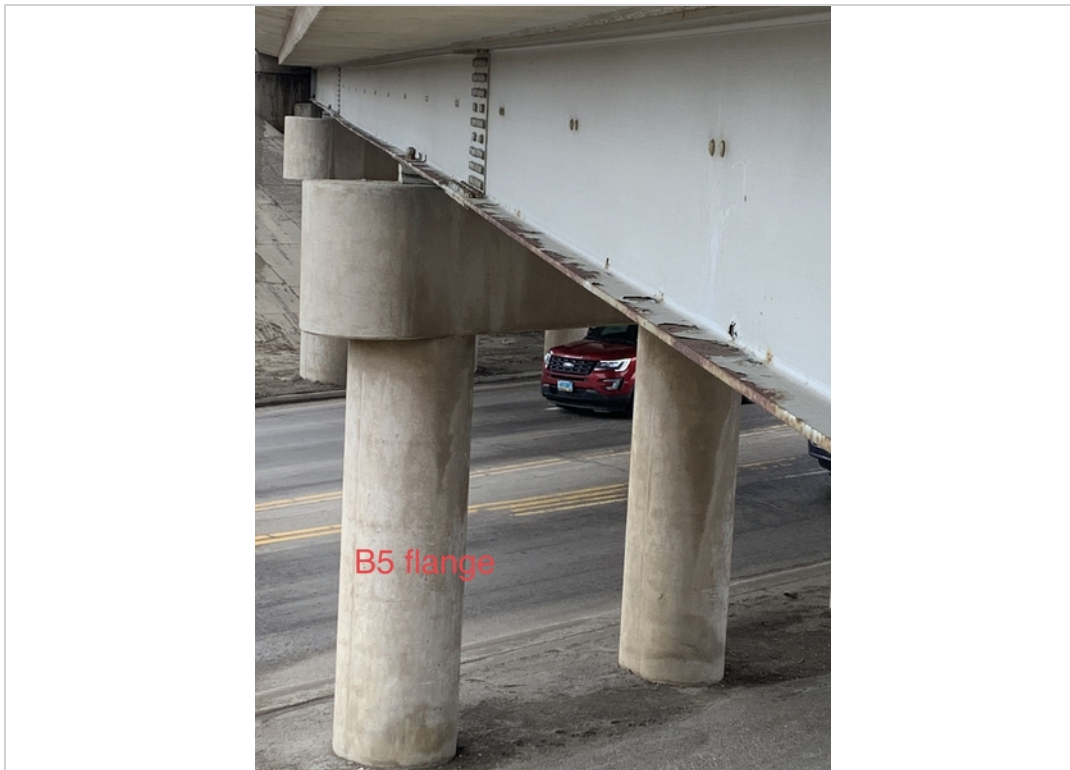
Beam 5 flange corrosion
