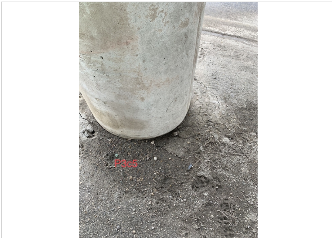
Pier 3 column 5 delam
