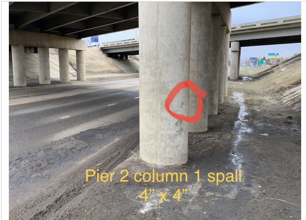
Pier 2 column 1 spall 4"x4"
