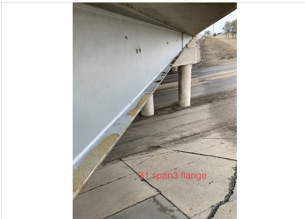
Beam 1 span 3 flange corrosion
