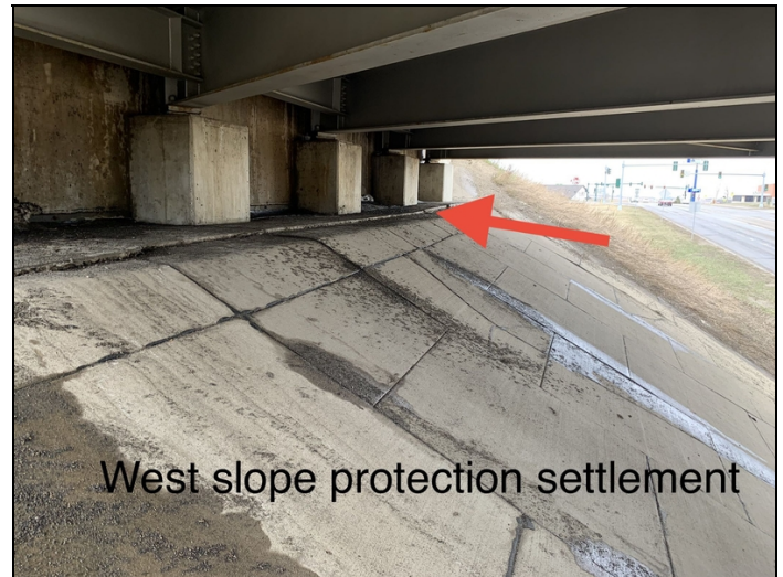
West slope protection settlement
