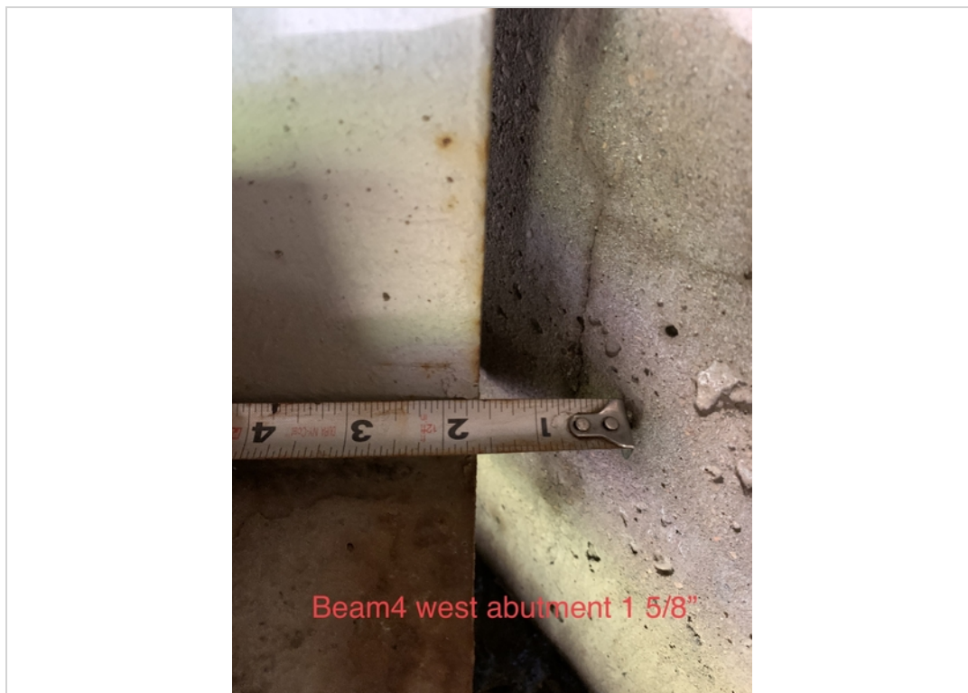
Beam 4 west abutment 1 5/8"
