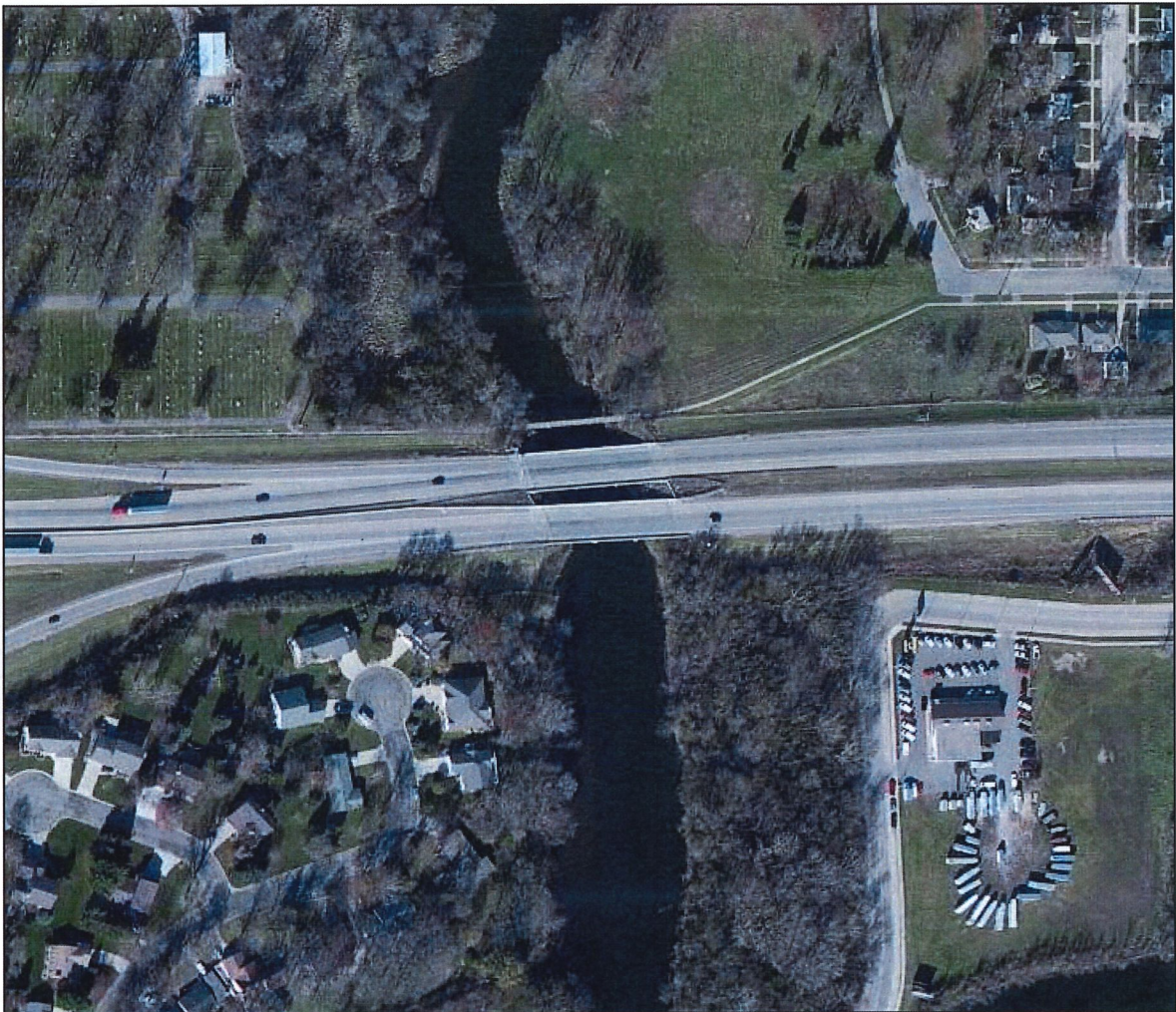
Figure 5. Cedar River Bridges - Bridge #6868 and 6869
