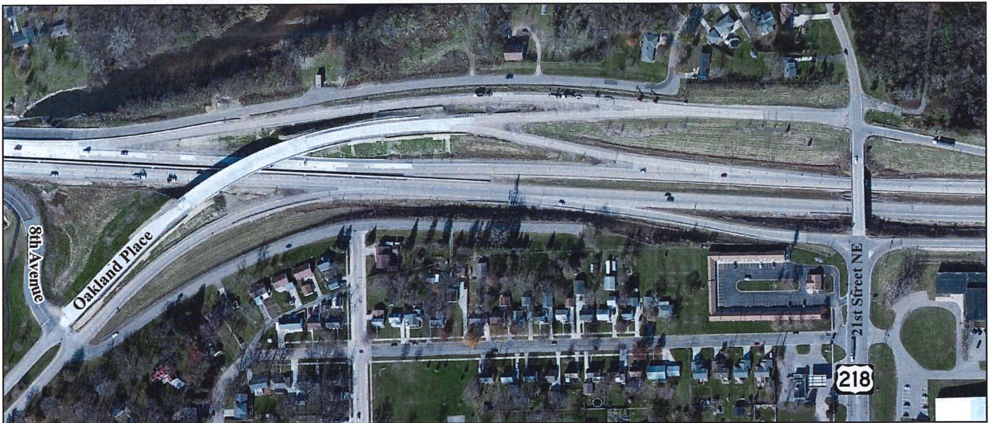
Figure 7. US 218 South/21st Street NE/Oakland Place Interchange - Bridge #9201
