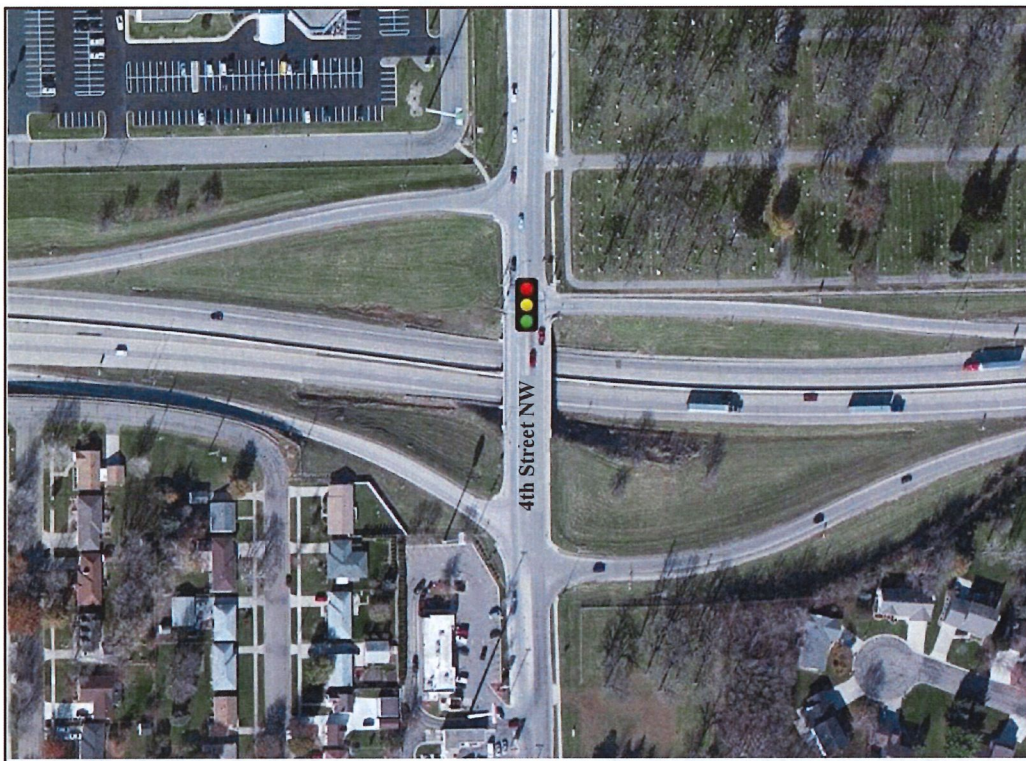
Figure 4. 4th Street NW Interchange - Bridge #9180
