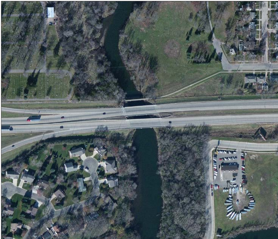
Figure 5. Cedar River Bridges - Bridge #6868 and 6869
