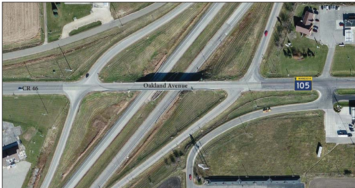
Figure 2. TH 105/Oakland Avenue Interchange - Bridge #9183
