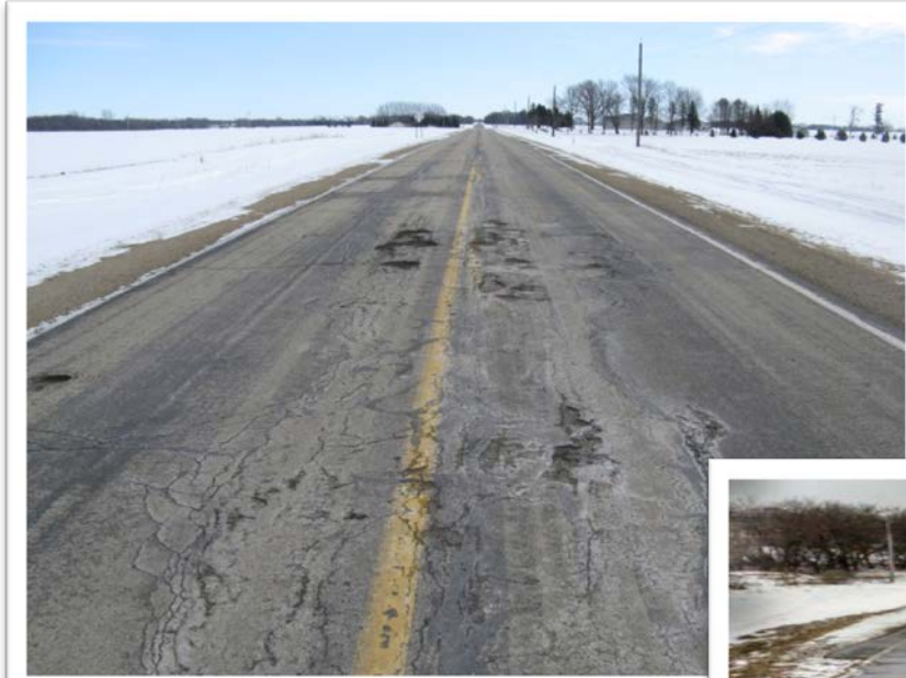
CR 58 – East of Transfer Station Surfaced in 1990
