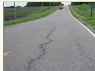
PCI = 38 POOR
