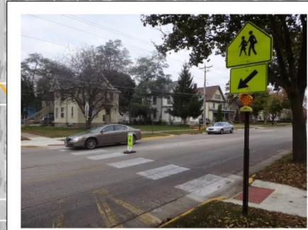
The flashing beacon across 4th St at 7th Ave should be upgraded to a modern Rectangular Rapid Flash Beacon to increase yielding compliance.
