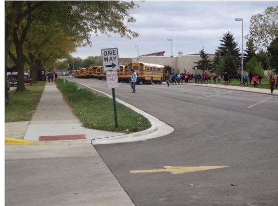
Ellis students head to the bus loop, one of the few places with ADA compliant curb ramps.
