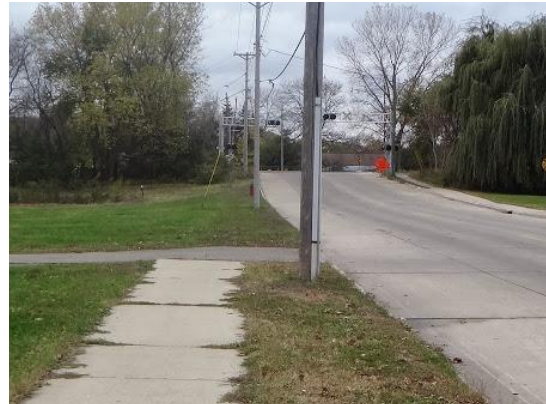
The sidewalk on the south side of 4th Ave SE ends as it approaches the railroad crossing.
