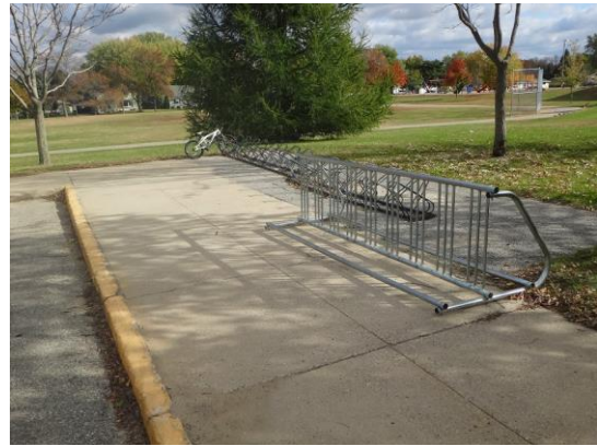
Comb style bicycle racks are provided. Alternative rack styles allow improved bicycle security.
