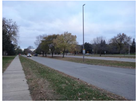
W Oakland Avenue and its two frontage roads (Service Drive and 1st Avenue SW) are a barrier for
