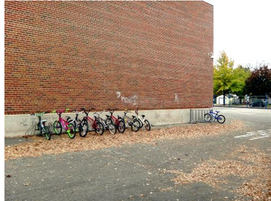
Bicycle racks are present on the south side of the school site.
