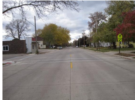
Motor vehicle traffic moves quickly along Oakland Avenue E, which runs along the north side of Neveln. Traffic calming measures may want to be investigated along this corridor to improve safety.
