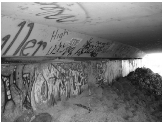
Figure 7. Graffiti and concreted rip rap at the east abutment. Debris on the bridge seats of both abutments appears to be the result of past failure of expansion joint glands.
