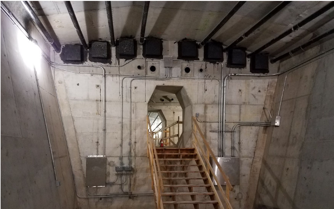
Figure 3.9 – Draped Tendon Anchorages
