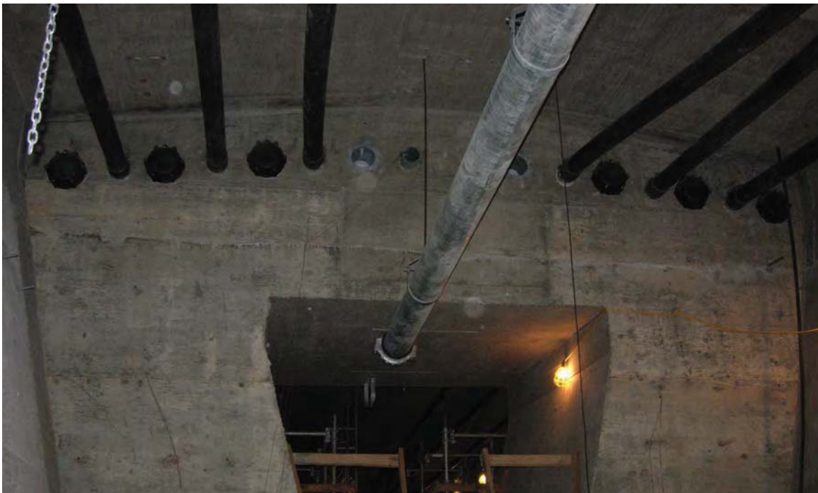
Figure 3.13 –Draped Tendon Anchorages
