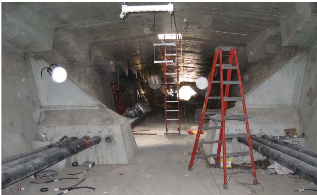
Figure 2.13 – Span 1 External Draped Tendons
