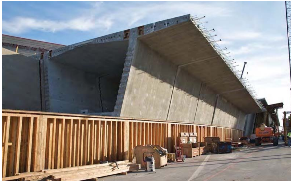
Figure 2.9 – Segment Casting
