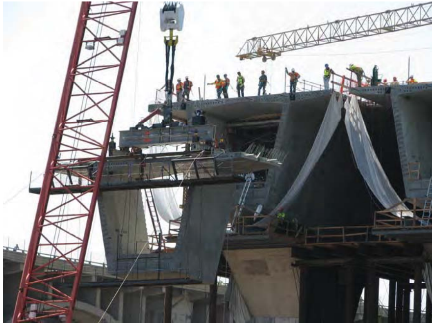
Figure 2.10 – Crane Erecting Segments (Span 2)
