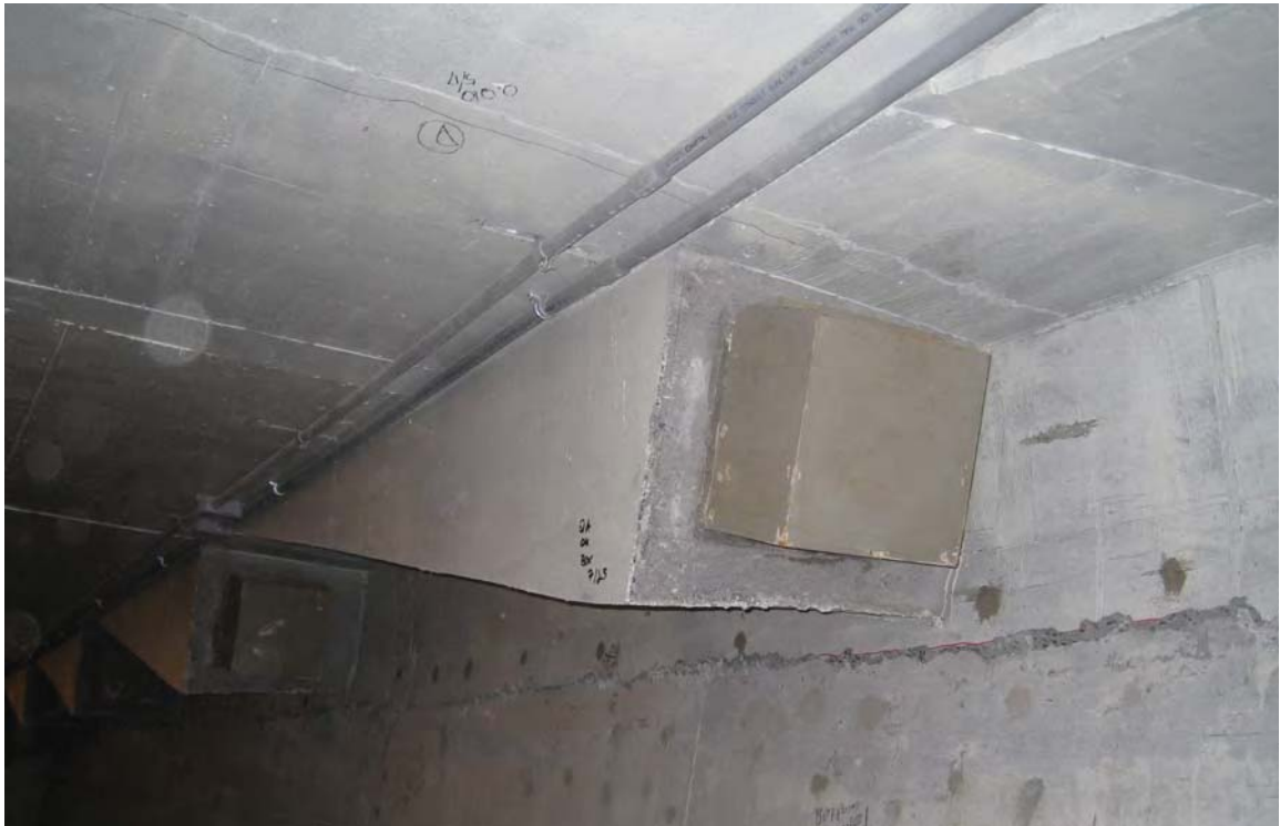
Figure 3.12 – Internal Tendon Anchor Blocks
