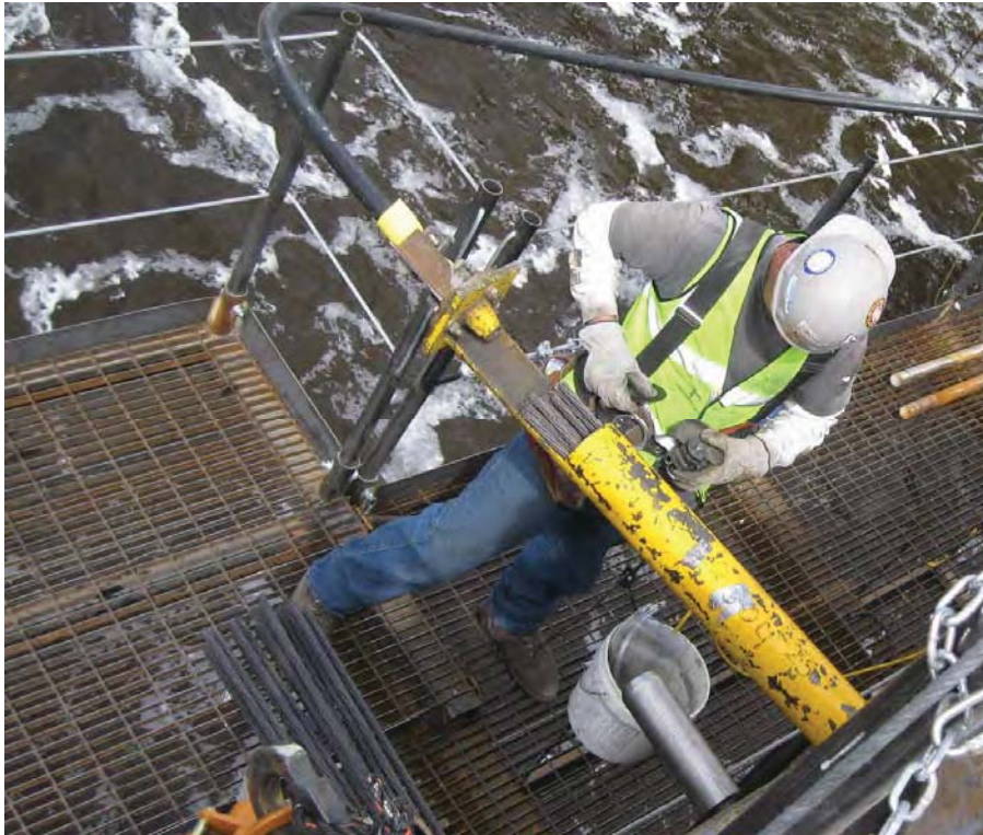
Figure 2.12 – Multi-Strand Cantilever PT Strand
