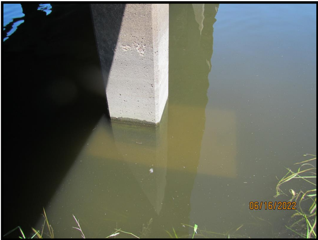
50-277-015_2022_24_CDI_West Bent Column #1 (South) Exposed Footing
