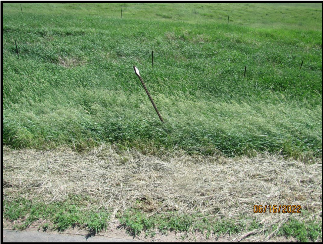
50-277-015_2022_6_CDI_4 th SW Approach Delineator Bent
