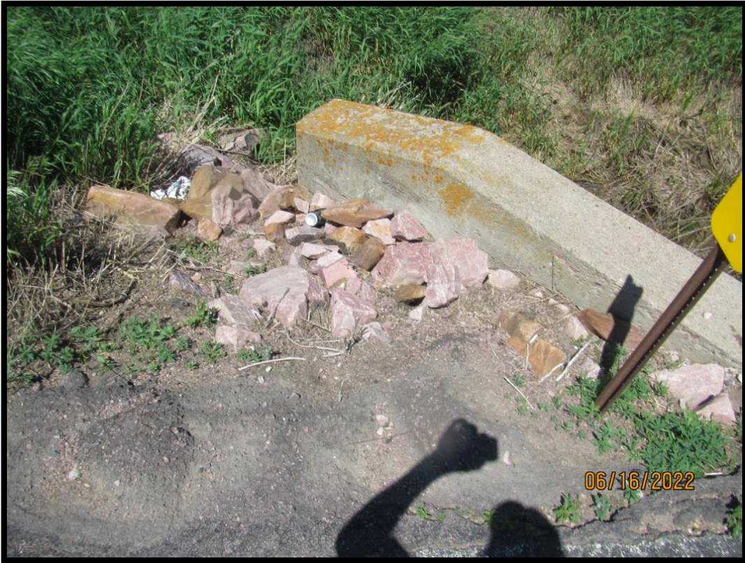
50-277-015_2022_29_CDI_Riprap behind NW Wingwall
