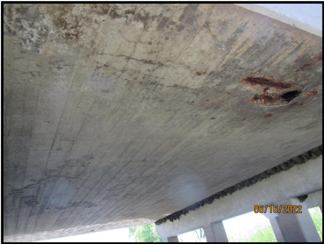
50-277-015_2022_18_CDI_Underside of Slab Span #3
