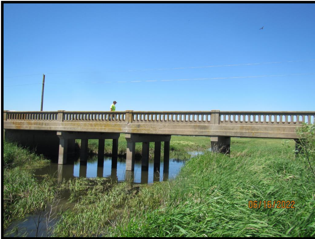
50-277-015_2022_3_CDI_Profile looking North
