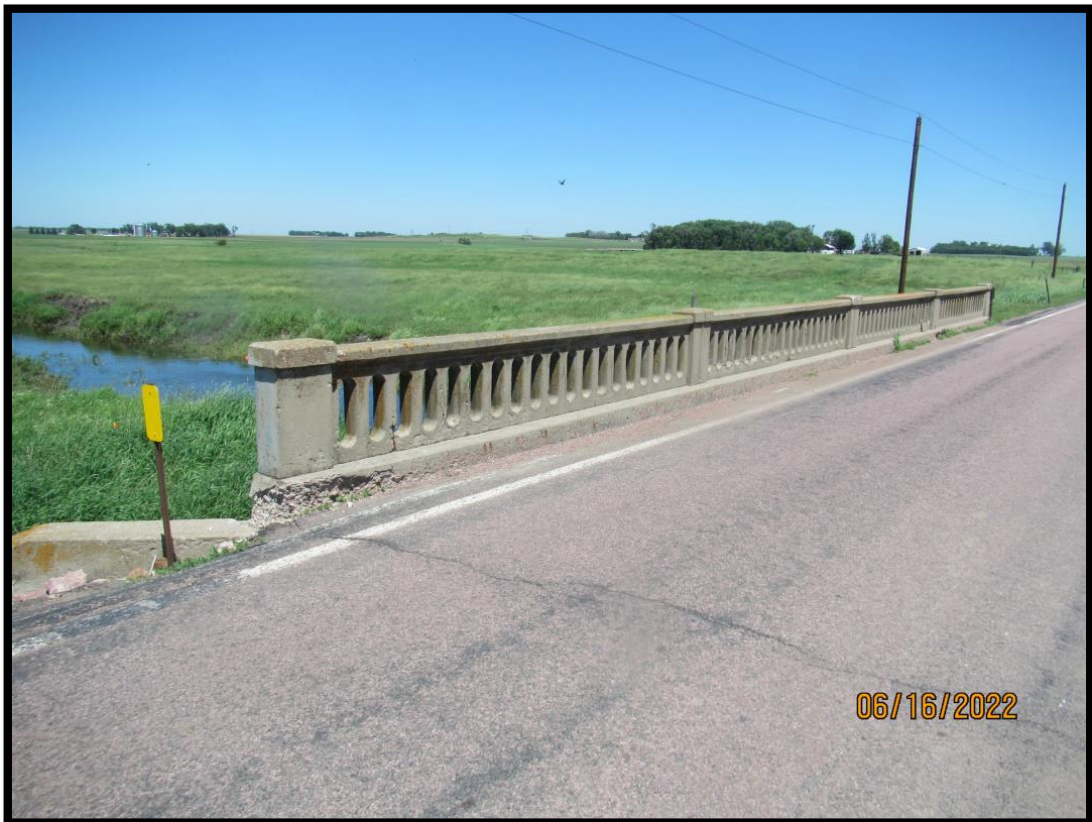
50-277-015_2022_14_CDI_North Bridge Rail
