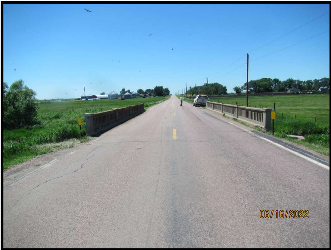
50-277-015_2022_2_CDI_Approach looking West
