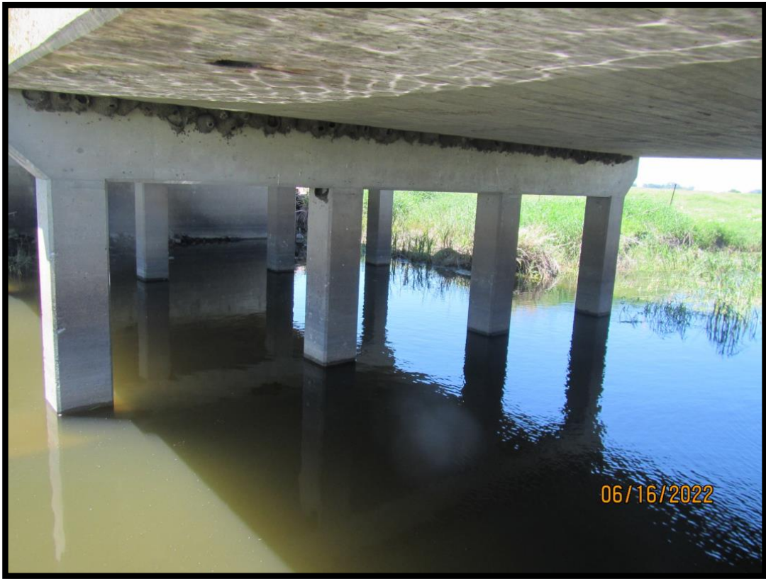
50-277-015_2022_23_CDI_Typical Configuration of Bent
