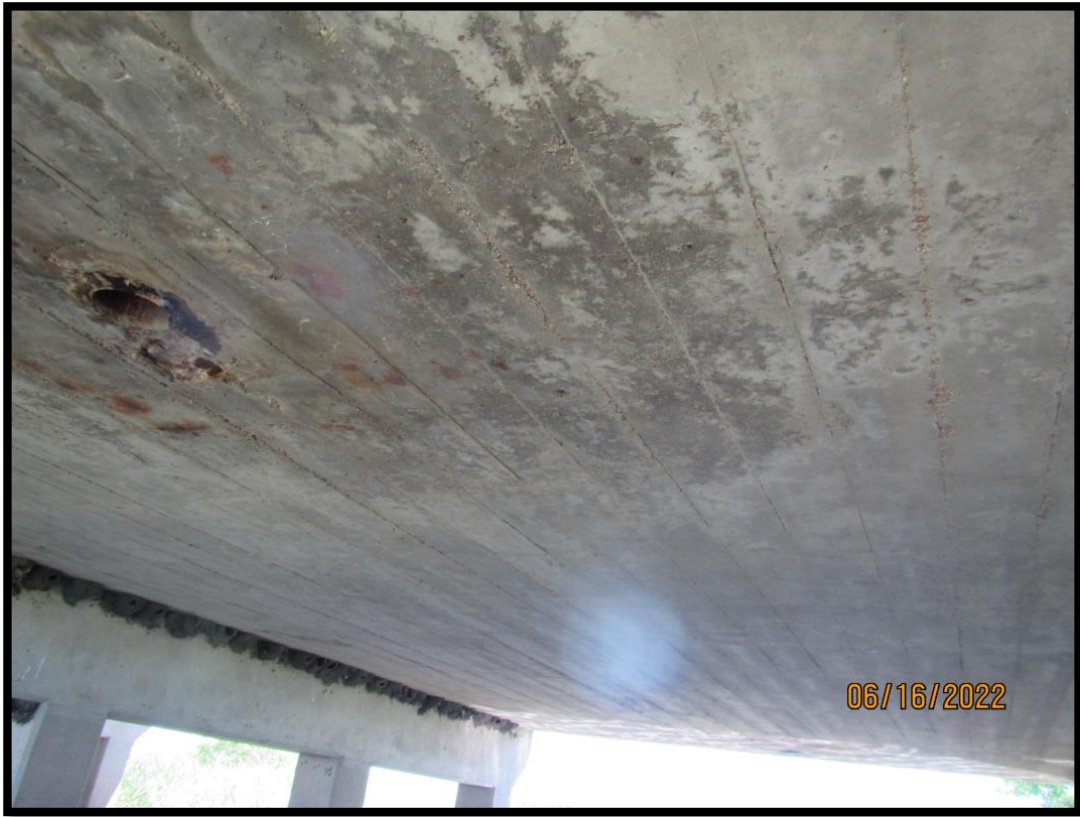
50-277-015_2022_17_CDI_Underside of Slab Span #2
