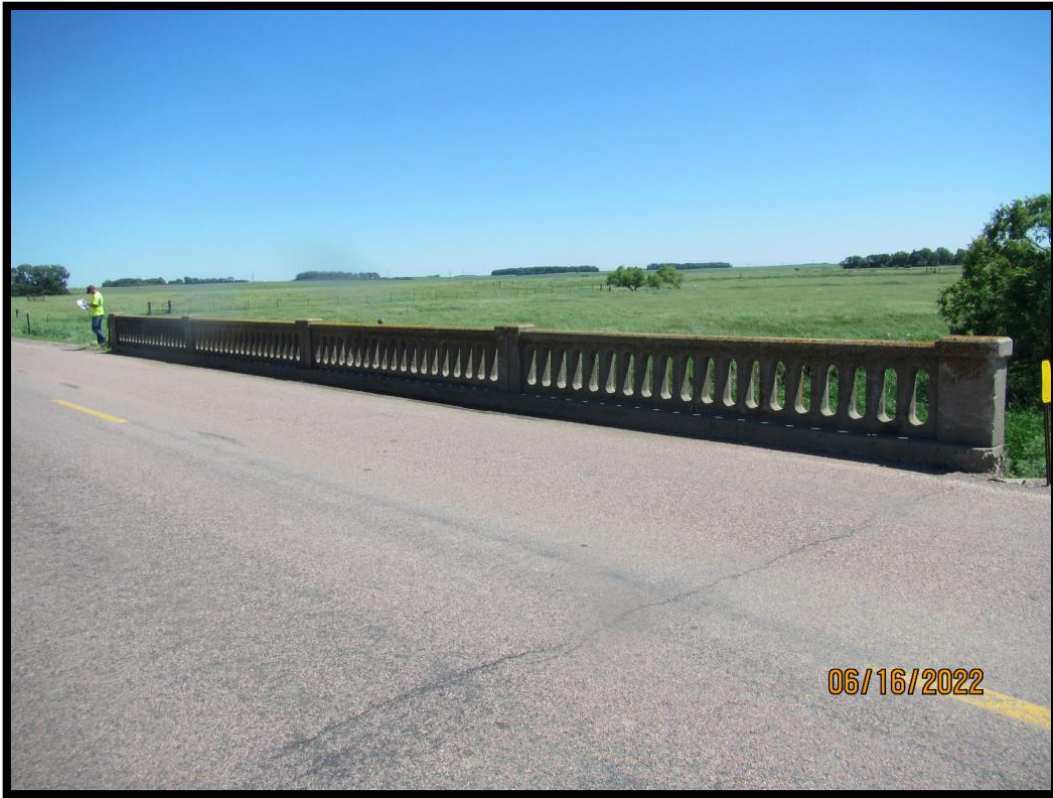
50-277-015_2022_15_CDI_South Bridge Rail
