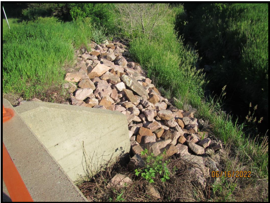
50-216-015_2022_28_CDI_Riprap along NW Channel Bank
