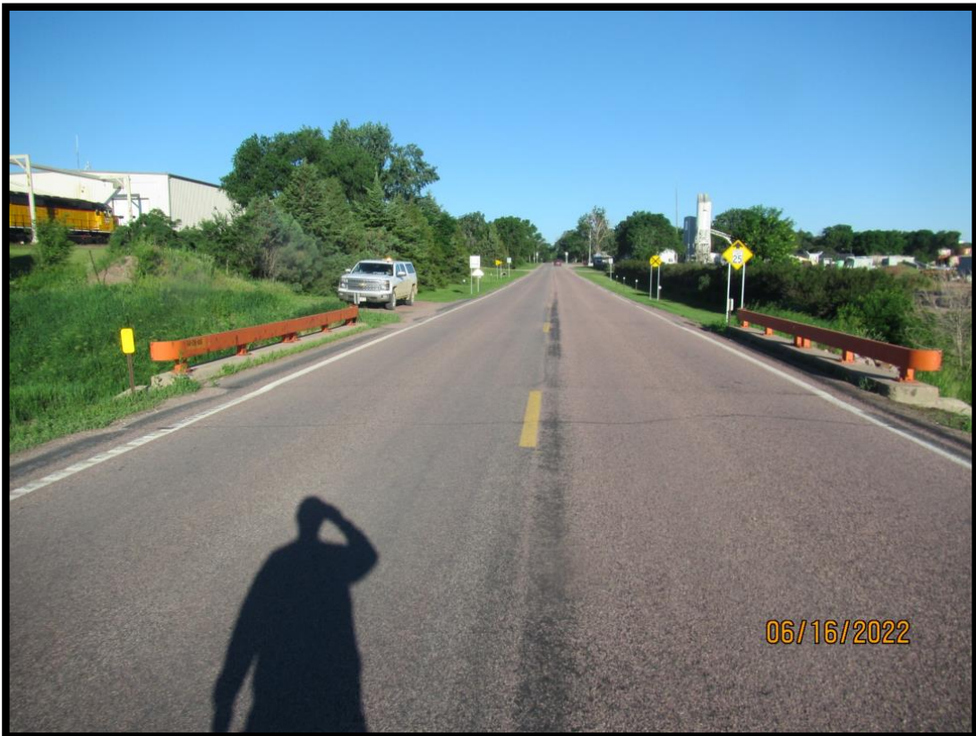
50-216-015_2022_2_CDI_Approach looking West
