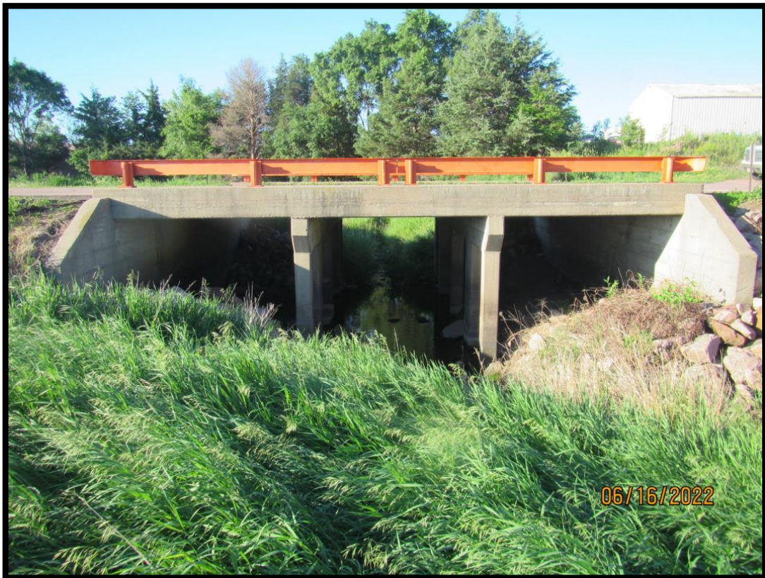
50-216-015_2022_4_CDI_Profile looking South
