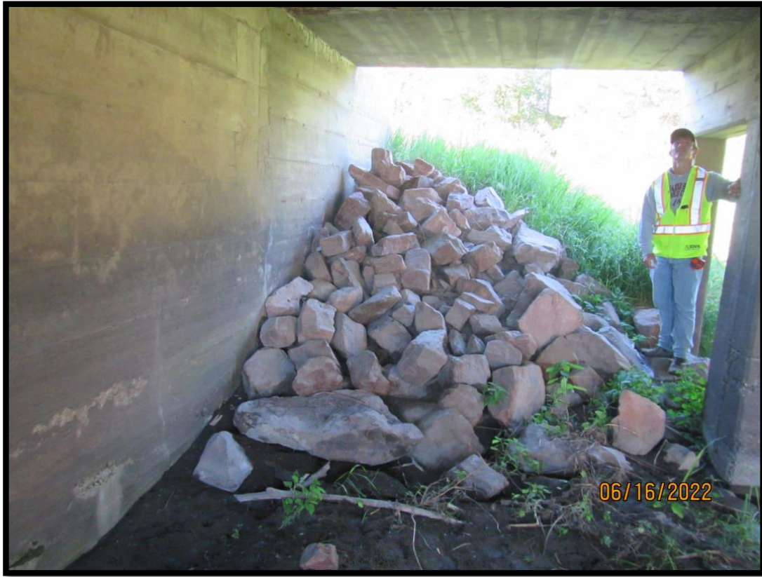
50-216-015_2022_29_CDI_Riprap in front of SE Wingwall
