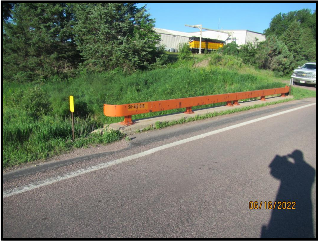
50-216-015_2022_9_CDI_South Bridge Rail
