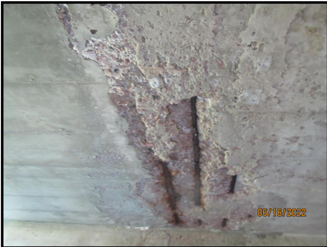
50-216-015_2022_12_CDI_Underside of Existing Slab, South side of East Span
