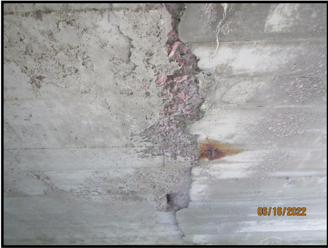
50-216-015_2022_13_CDI_Underside of Existing Slab, North side of East Span
