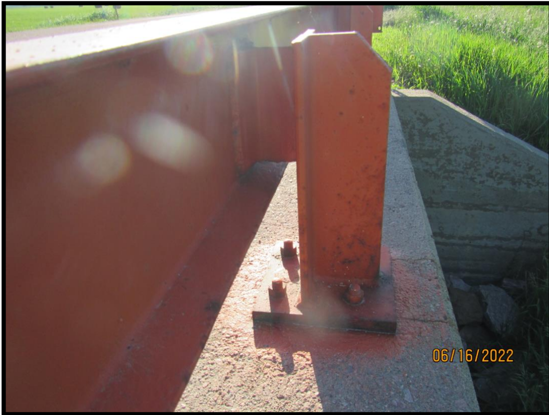
50-216-015_2022_11_CDI_Typical Rail Post Condition
