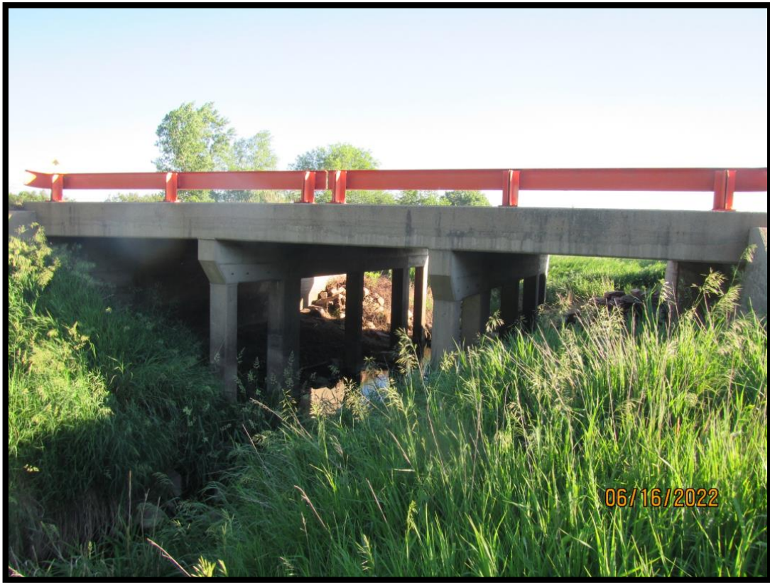
50-216-015_2022_3_CDI_Profile looking North
