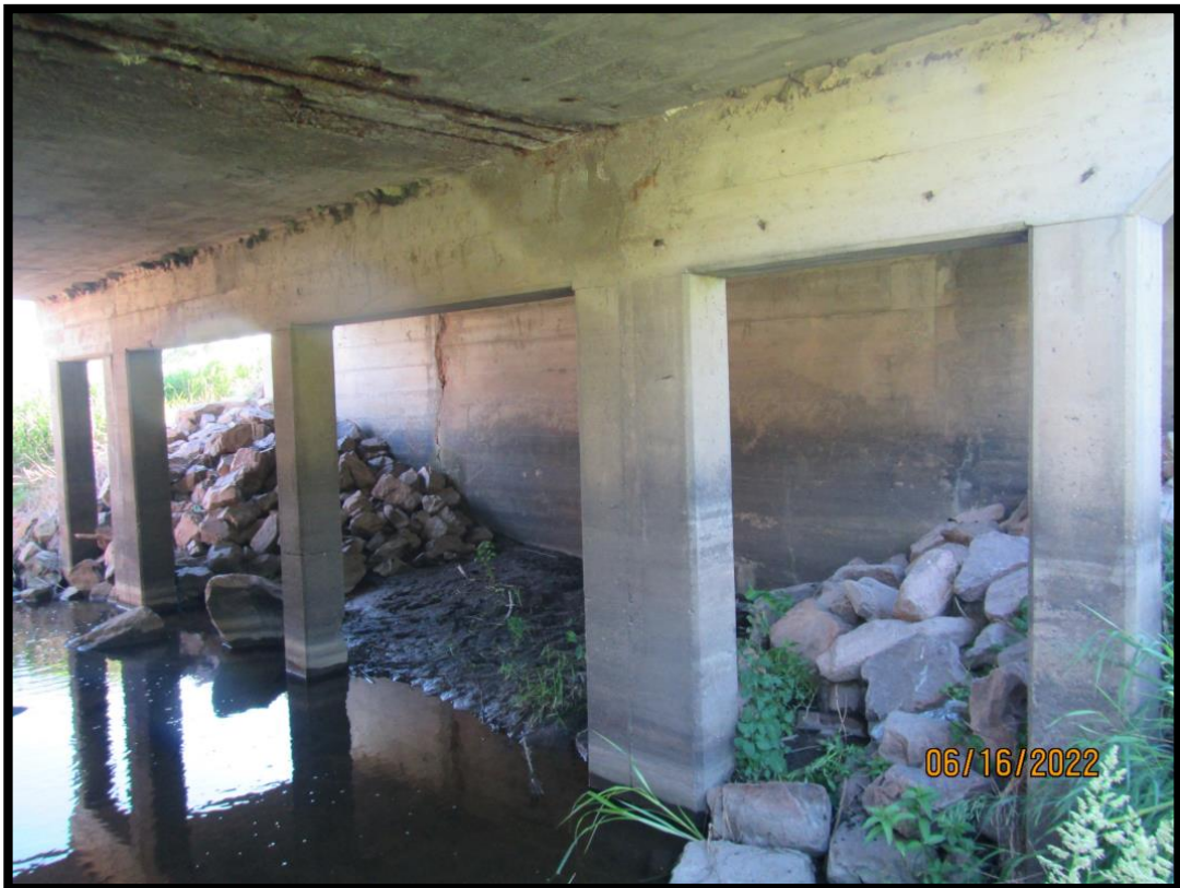
50-216-015_2022_22_CDI_Typical Configuration of Bent
