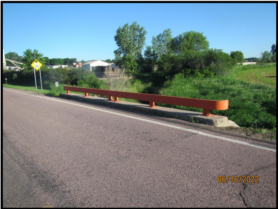
50-216-015_2022_10_CDI_North Bridge Rail
