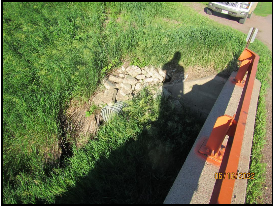
50-216-015_2022_5_CDI_CMP Culvert Outlet at SW Corner of Structure
