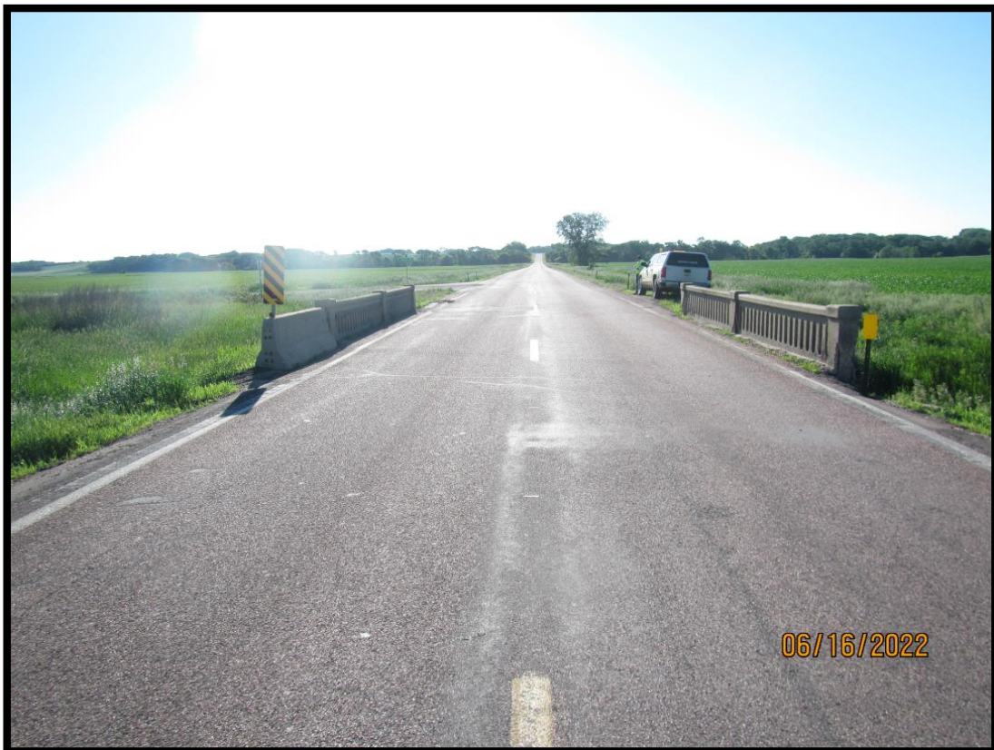
50-219-015_2022_2_CDI_Approach looking East
