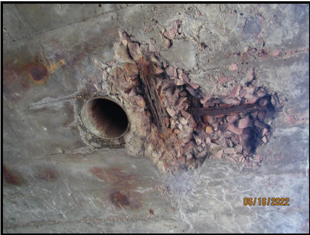
50-277-015_2022_20_CDI_Underside of Slab Span #4 Spall with Exposed Rebar at North Deck Drain
