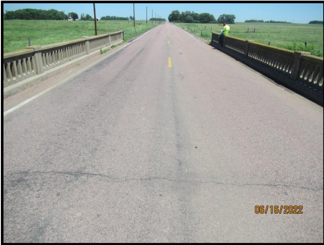
50-277-015_2022_7_CDI_Top of Bituminous Overlay looking East
