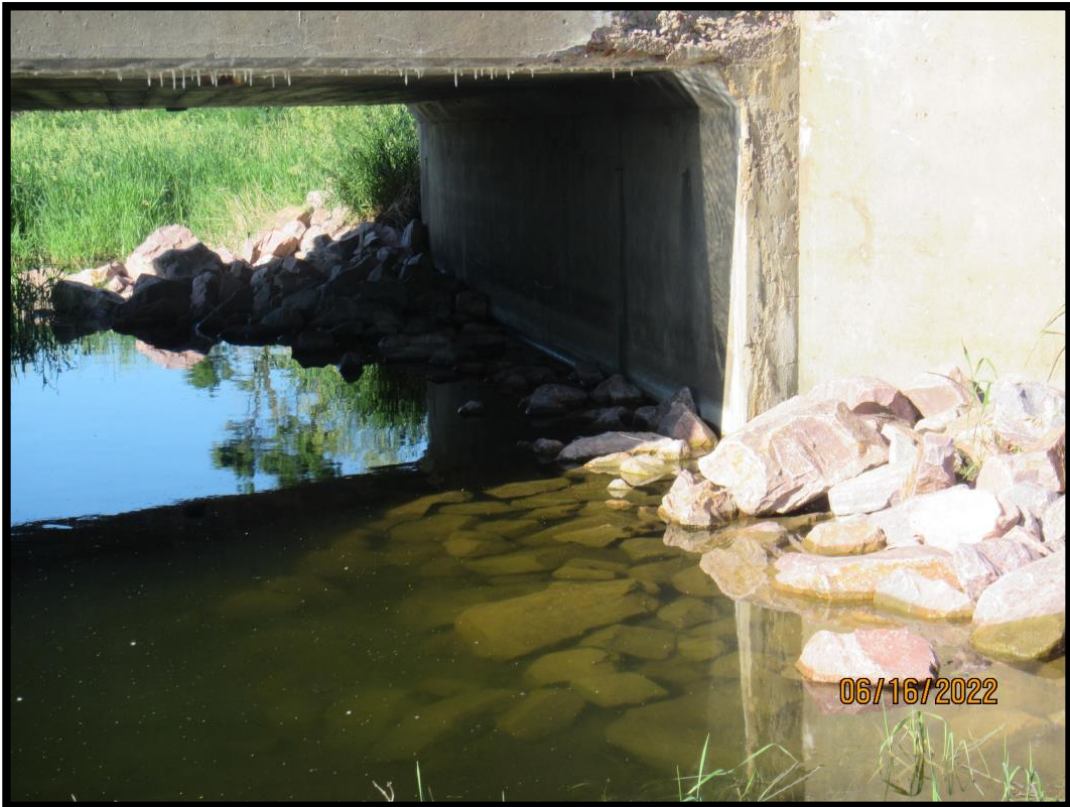
50-219-015_2022_28_CDI_Riprap in front of West Abutment
