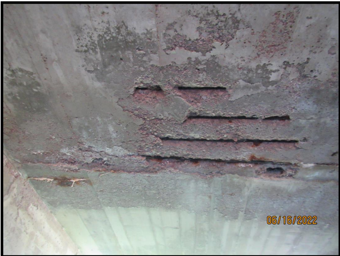
50-216-015_2022_16_CDI_Underside of Existing Slab, South side of West Span
