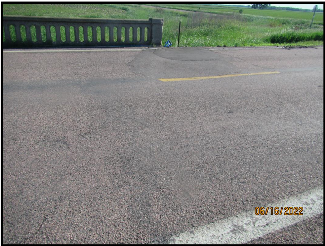
50-219-015_2022_8_CDI_Bituminous Patch at NE Bridge end
