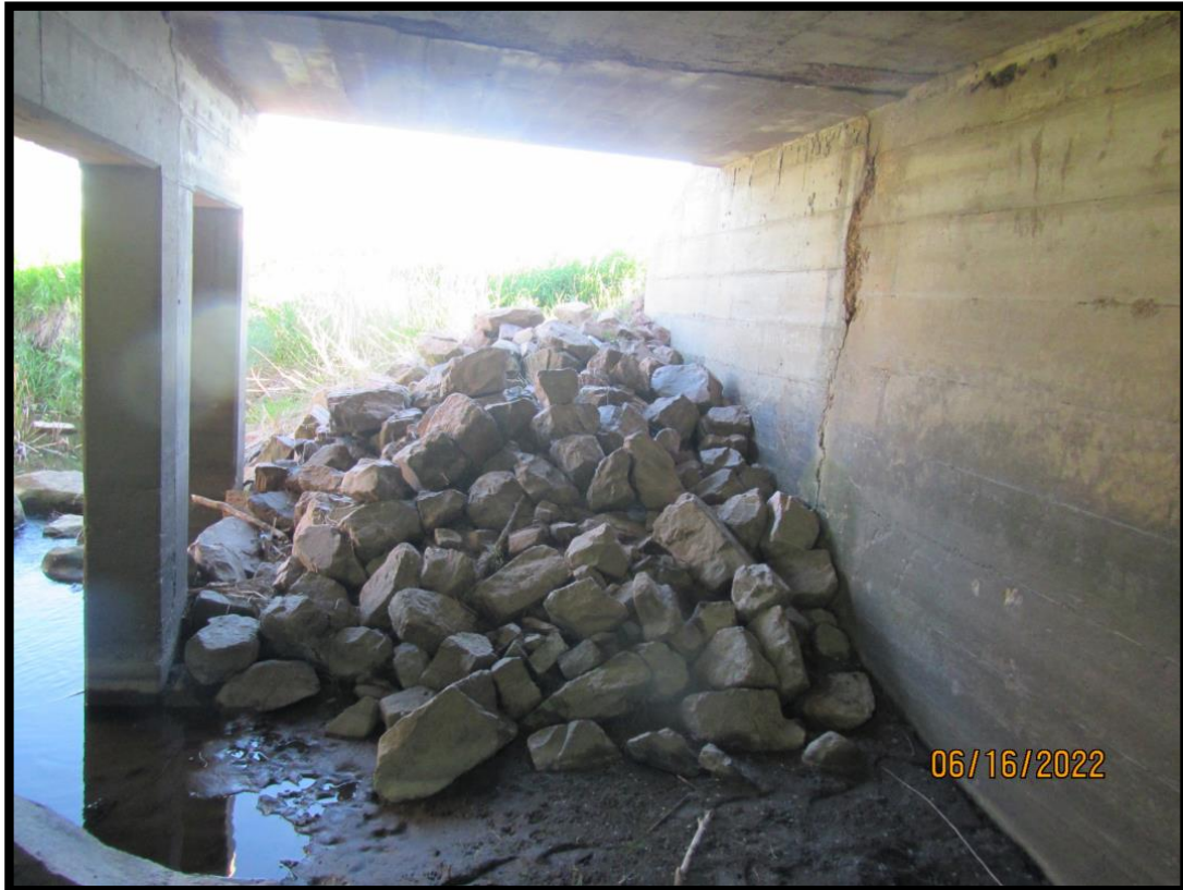
50-216-015_2022_30_CDI_Riprap in front of NE Wingwall
