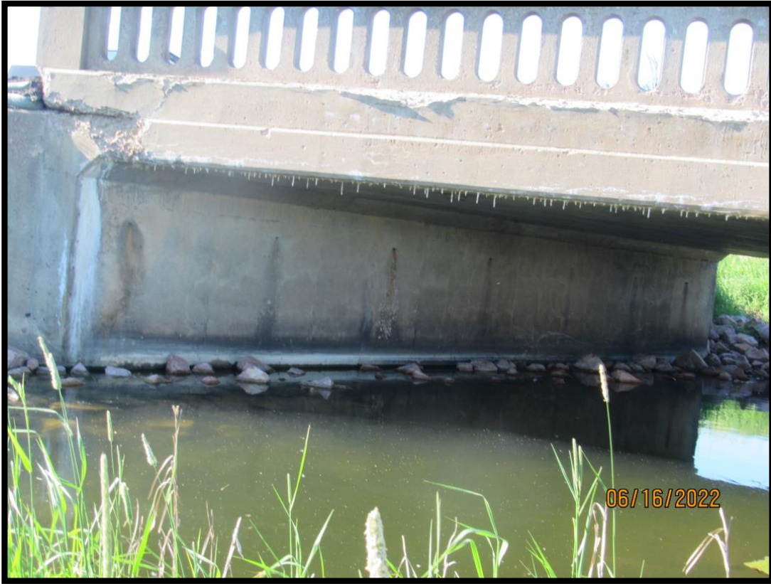
50-219-015_2022_29_CDI_Riprap in front of East Abutment
