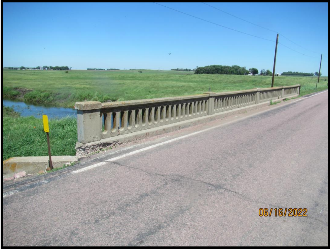
50-277-015_2022_14_CDI_North Bridge Rail
