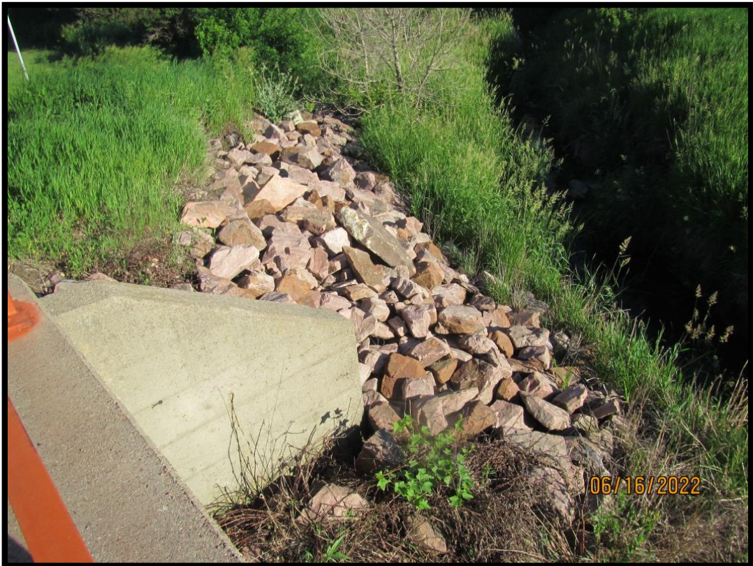
50-216-015_2022_28_CDI_Riprap along NW Channel Bank
