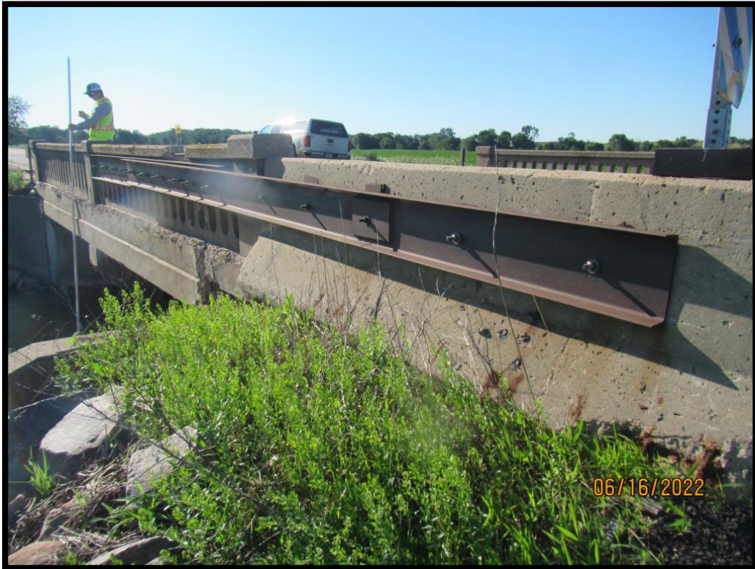
50-219-015_2022_16_CDI_Steel Channel Attached to Backside of NW Railing
