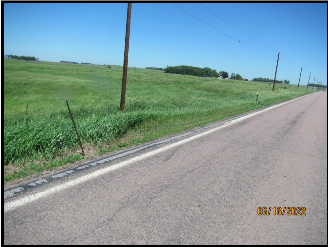
50-277-015_2022_5_CDI_1 st NE Approach Delineator Bent
