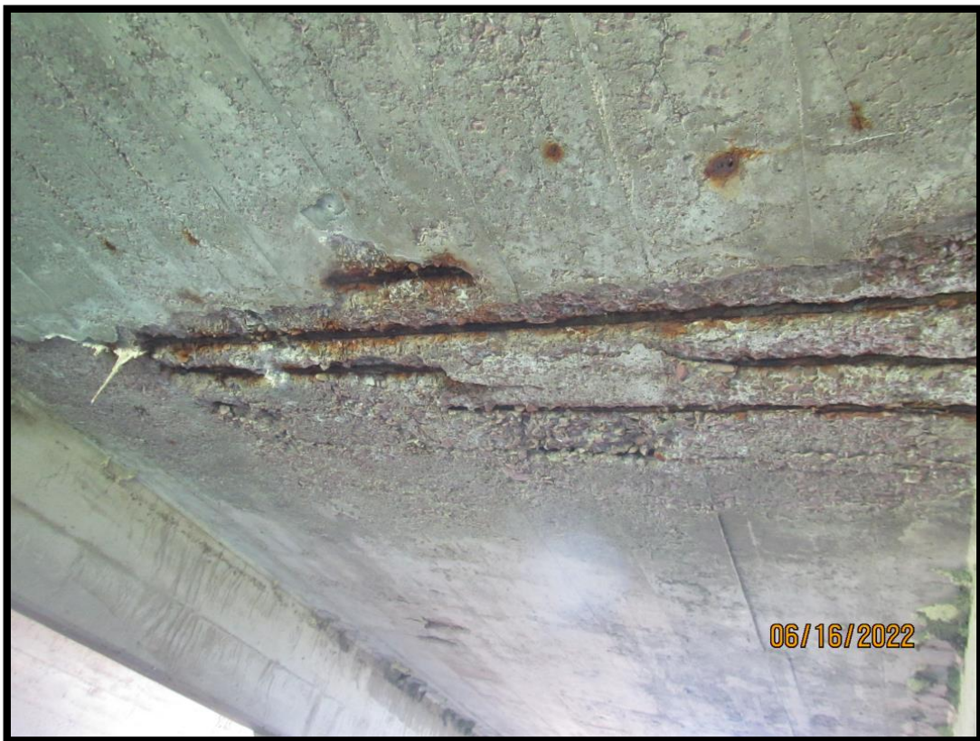
50-216-015_2022_14_CDI_Underside of Existing Slab, South side of Center Span
