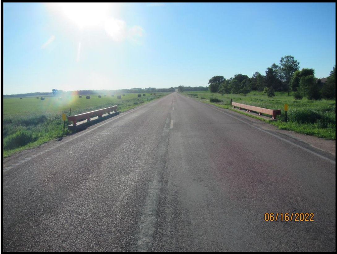
50-216-015_2022_1_CDI_Approach looking East
