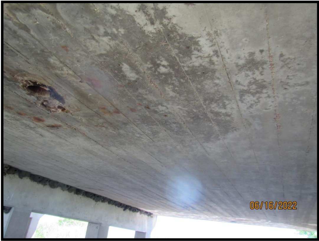
50-277-015_2022_17_CDI_Underside of Slab Span #2
