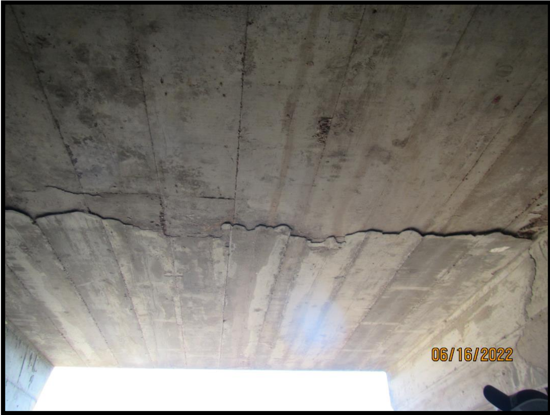
50-216-015_2022_17_CDI_Underside of Existing Slab, North side of West Span
