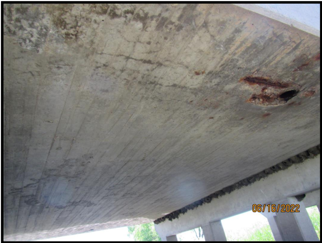
50-277-015_2022_18_CDI_Underside of Slab Span #3
