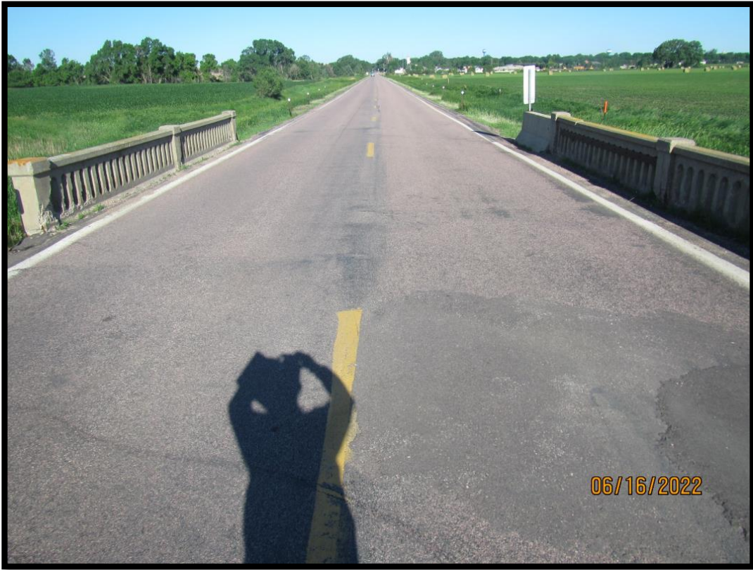
50-219-015_2022_7_CDI_Top of Bituminous Overlay looking West
