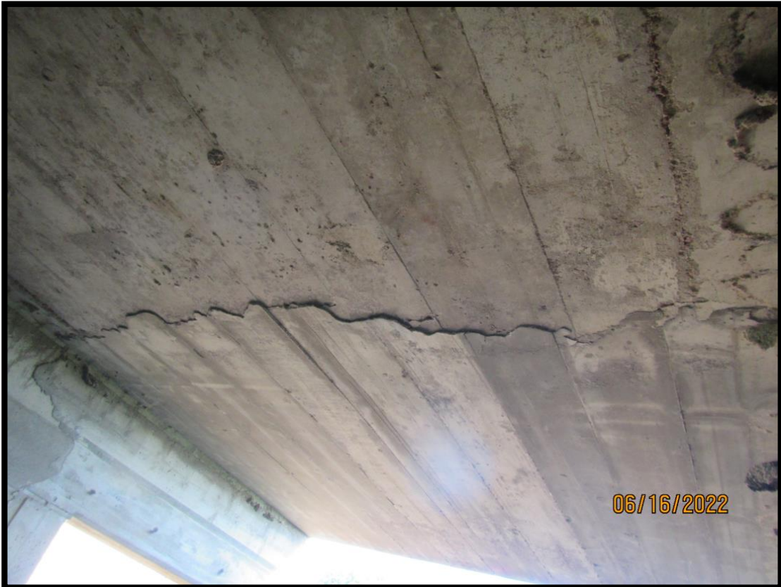
50-216-015_2022_15_CDI_Underside of Existing Slab, North side of Center Span
