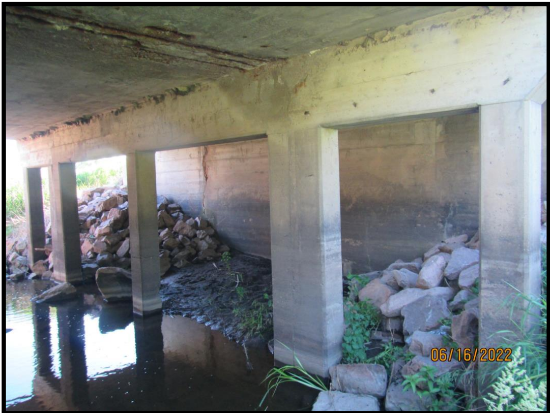
50-216-015_2022_22_CDI_Typical Configuration of Bent
