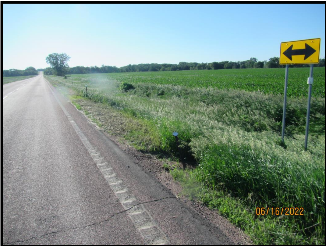
50-219-015_2022_5_CDI_1 st NE Approach Delineator Missing
