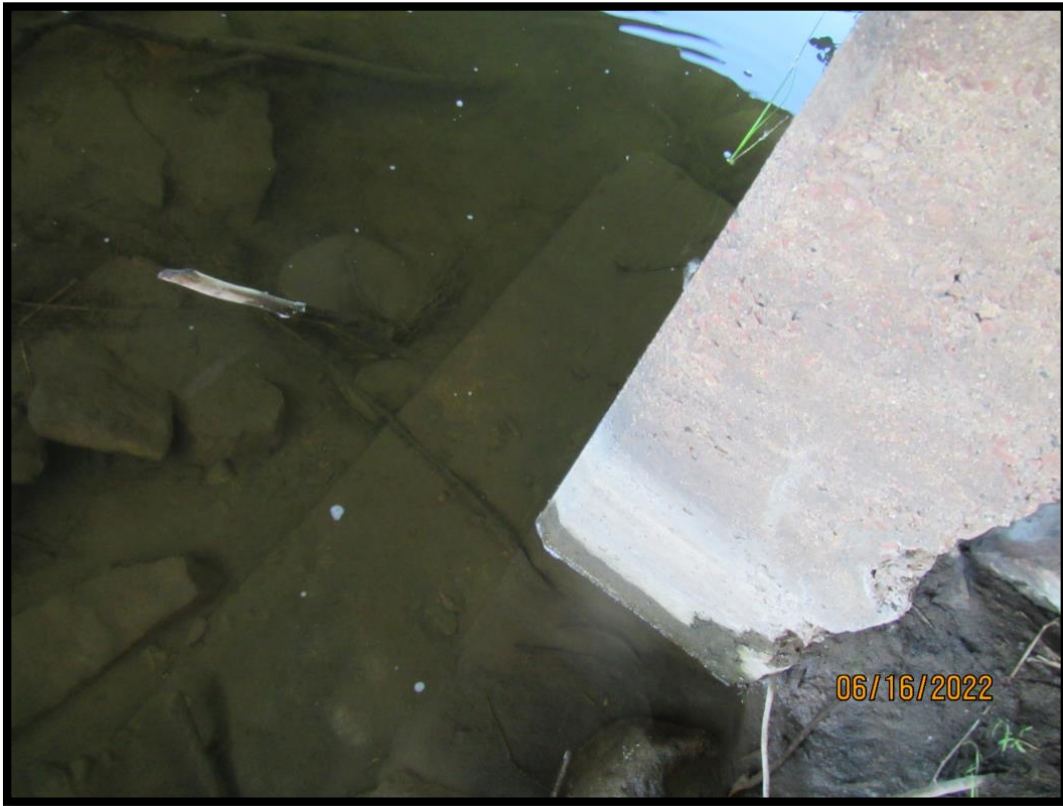
50-216-015_2022_25_CDI_Typical Exposed Concrete Footing (West Bent Column #3 shown)
