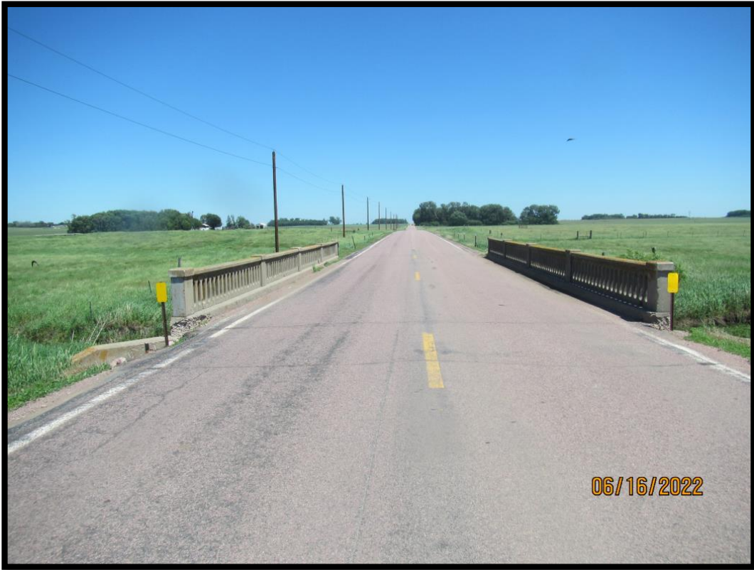
50-277-015_2022_1_CDI_Approach looking East
