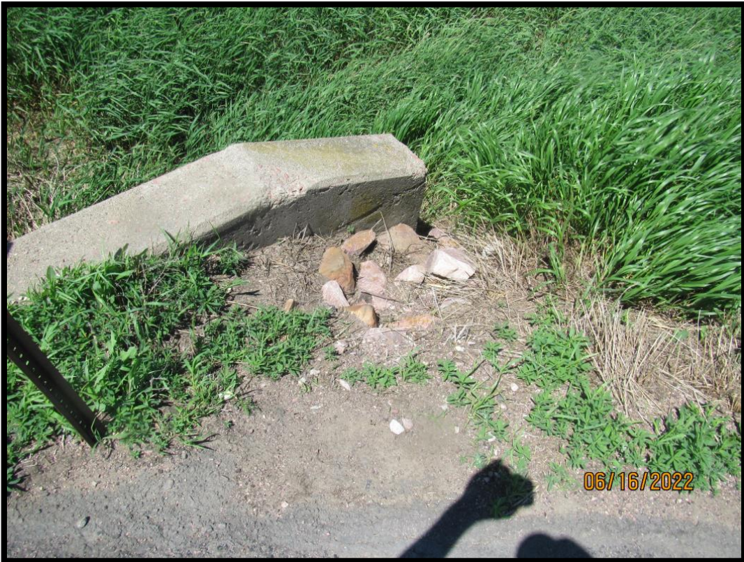
50-277-015_2022_30_CDI_Riprap behind NE Wingwall
