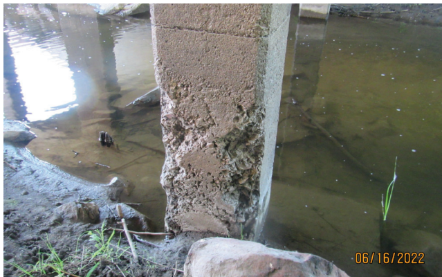
Figure 3 50-216-015 Column Honeycombing
