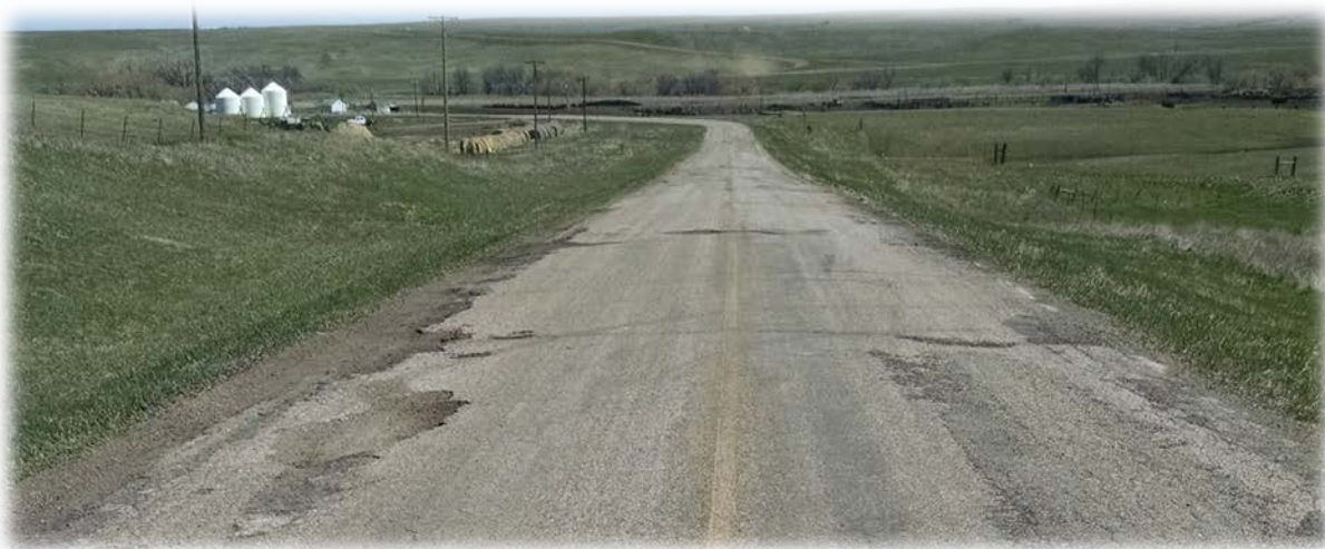
Photo of a PASER Rating 3 Road on the Standing Rock Reservation
