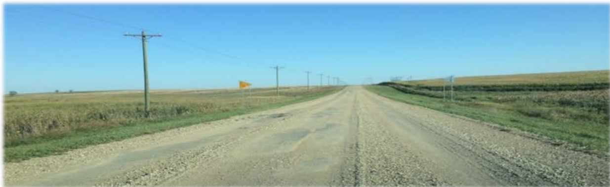
Example Photo of a PASER Rating 2 Road
