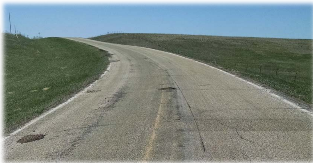
Photo of Pavement Condition on a Standing Rock Reservation Road
