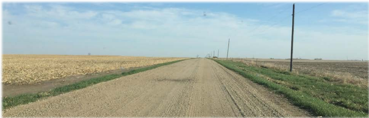
Example Photo of a PASER Rating 1 Road
