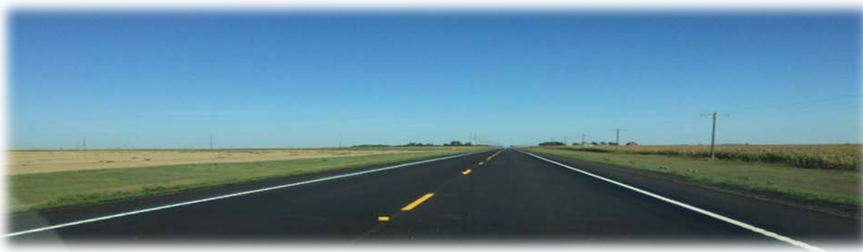
Example Photo of a PASER Rating 10 Road
