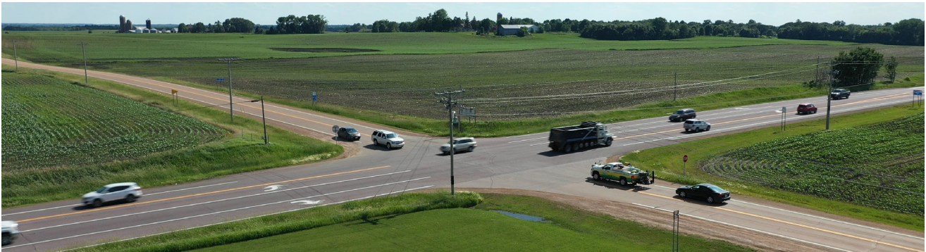
US 212 and County Highway 43
