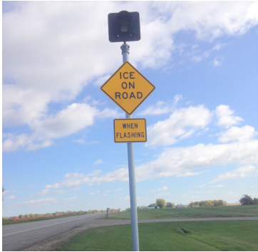
Figure 16 Blow Ice Warning System Sign
