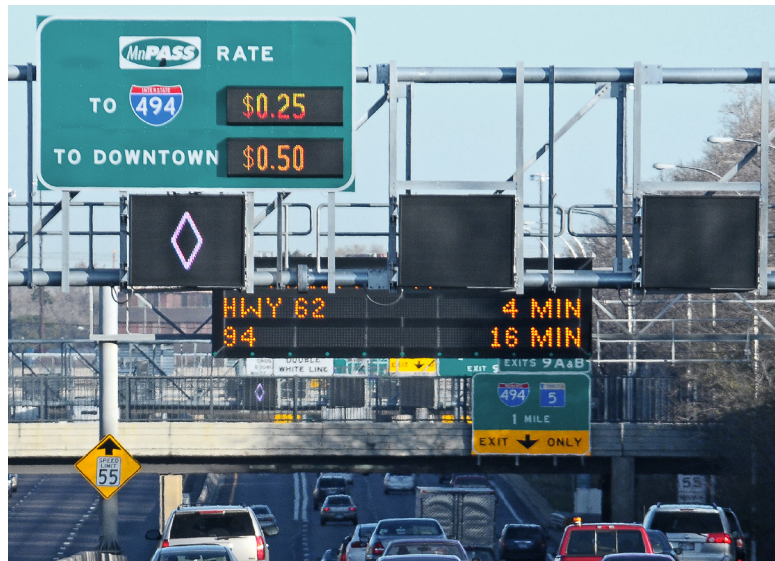
Figure 6-11: Overhead Sign Structure
