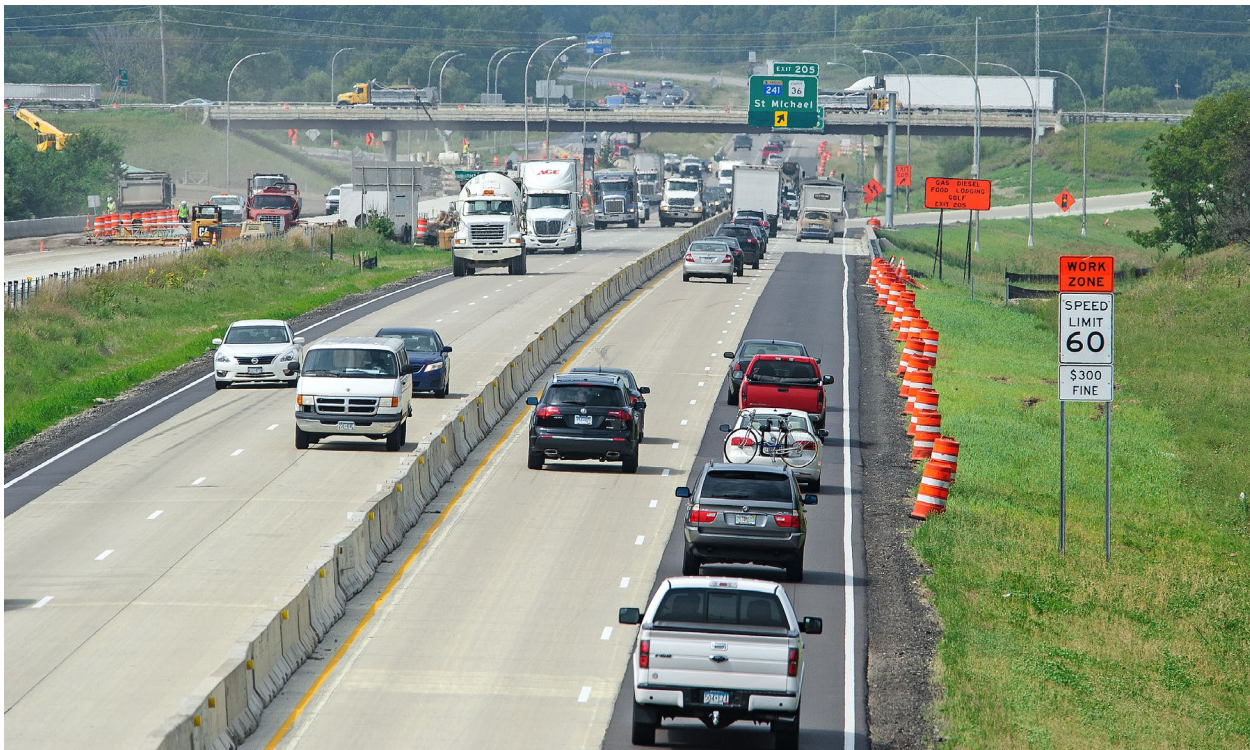
Construction along I-94 near TH 241. Source: District 3 Staff
